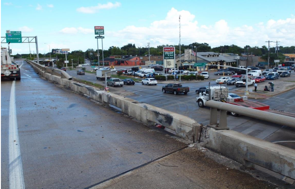
Figure 3 – View of the bridge rail after impact by the HISD school bus looking to the southeast
