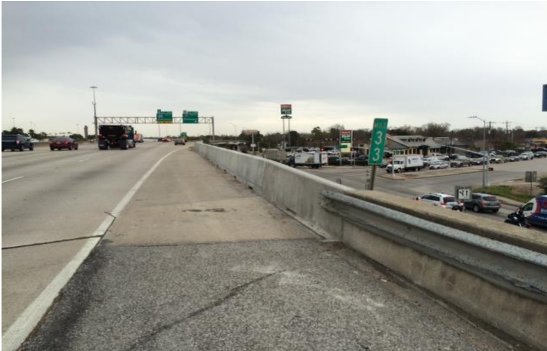
Figure 6 – New single-sloped concrete traffic rail installed by the TxDOT Houston District after the crash looking to the southeast (Source: TxDOT Houston District)
