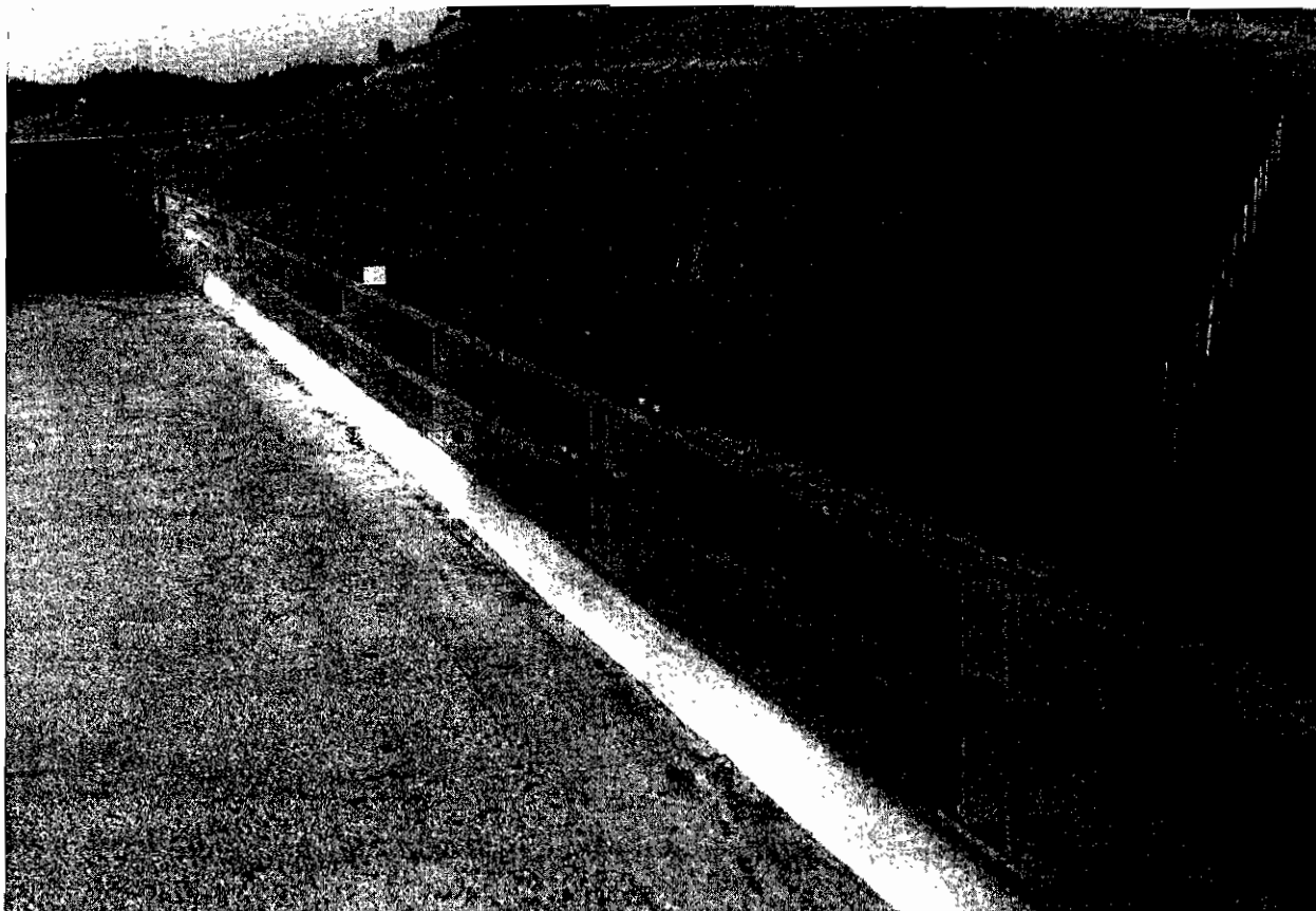
FIGURE 7.2 Wyoming two-tube bridge railing
