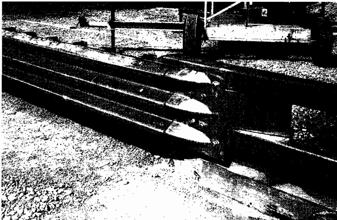
FIGURE 7.20a Thrie-beam transition to curb-mounted steel post and beam bridge railing
