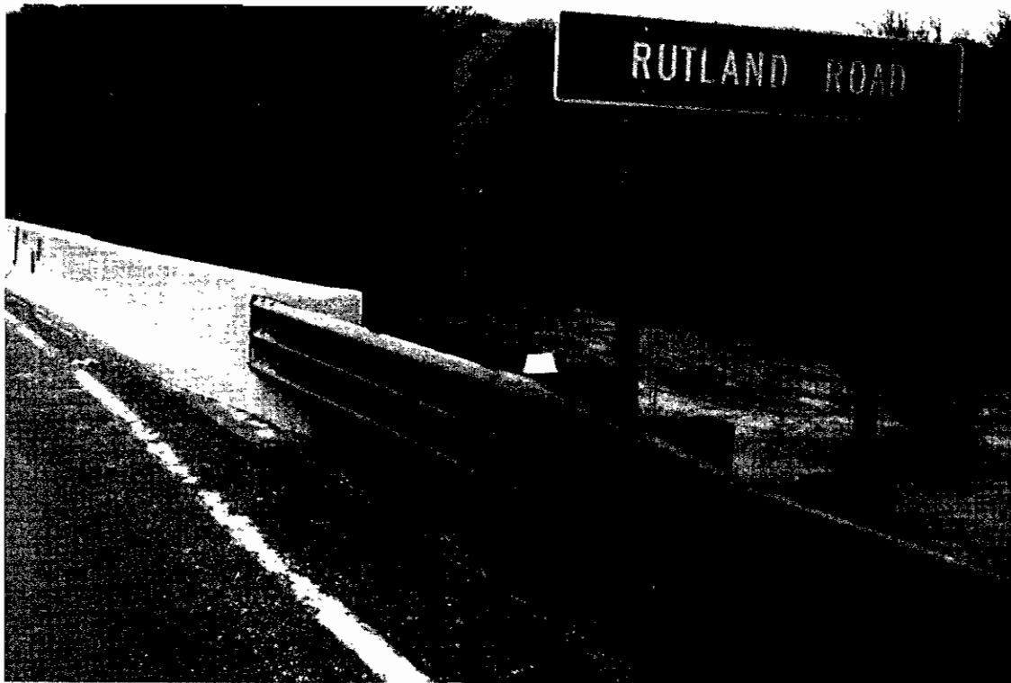
FIGURE 7.19 Thrie-beam transition to modified concrete safety shape
