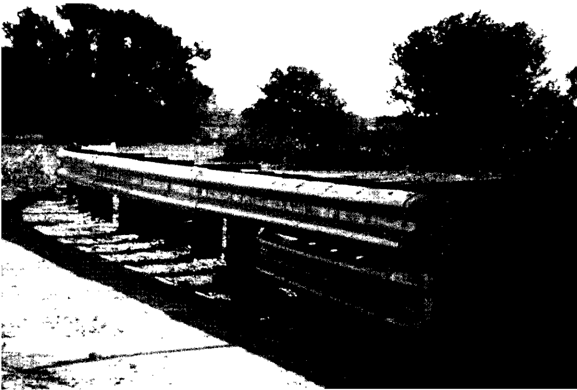
FIGURE 7.17 W-beam transition to vertical concrete rail
