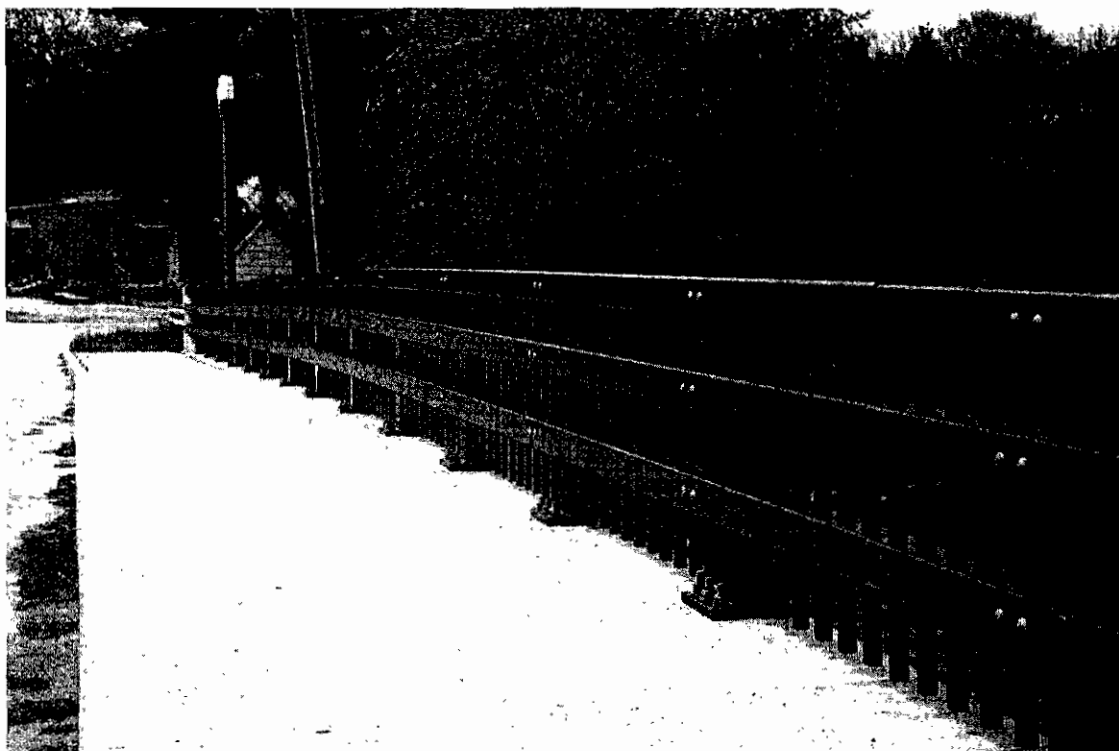
FIGURE 7.3 Massachusetts S3 steel bridge railing
