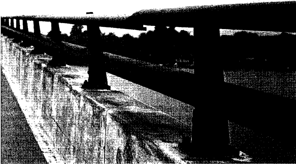
FIGURE 7.10 Lack of continuity in railing
