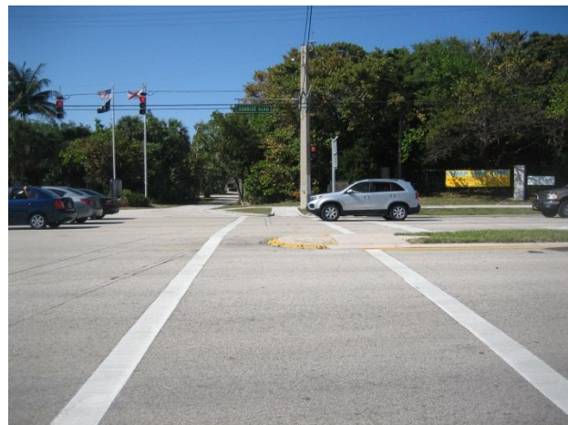
Photograph 2: Crosswalk on the east side (looking north)
