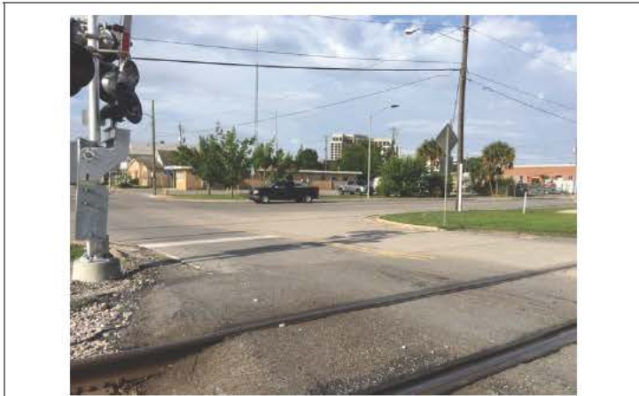
Photo No. 3 View Southwest.
