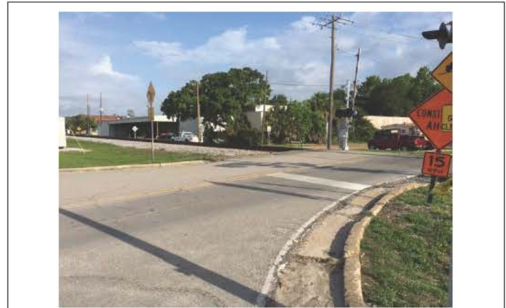
Photo No. 4 View Northwest.
