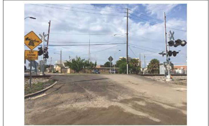
Photo No. 2 View Southwest.
