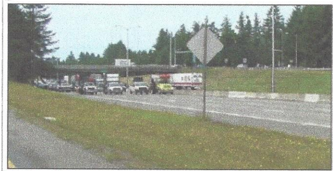
A Rolling Roadblock Using Maintenance Vehicles with PCMS and Arrow Panels
