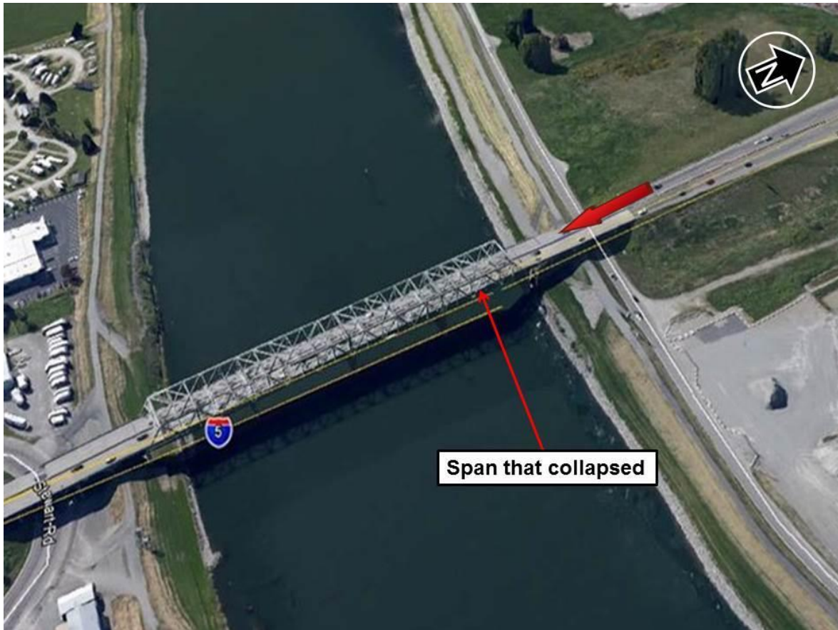
Figure 4. Aerial view, looking west, at the Skagit River (through-truss) Bridge before the span collapse. The span that collapsed is labeled, and the large red arrow shows the southbound direction of travel of the oversized combination vehicle. (Image captured by Google Earth.)
