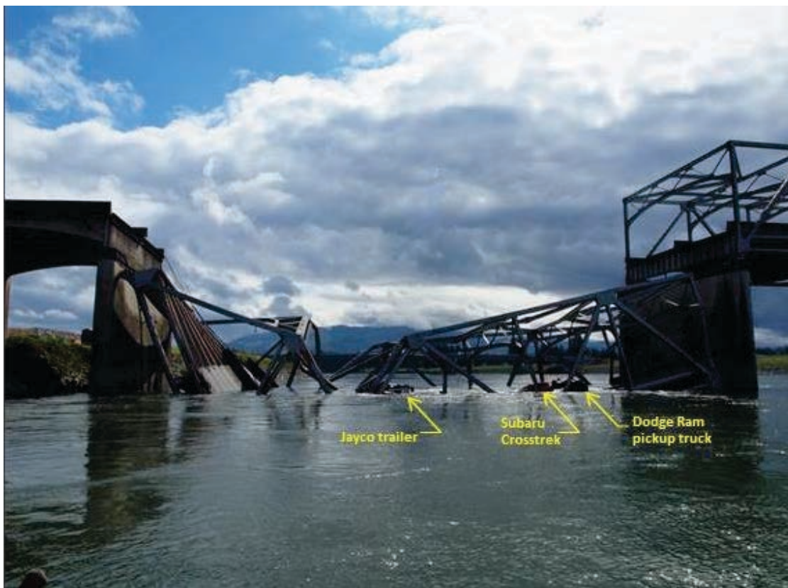
Figure 6. Bridge span 8 in the Skagit River.
