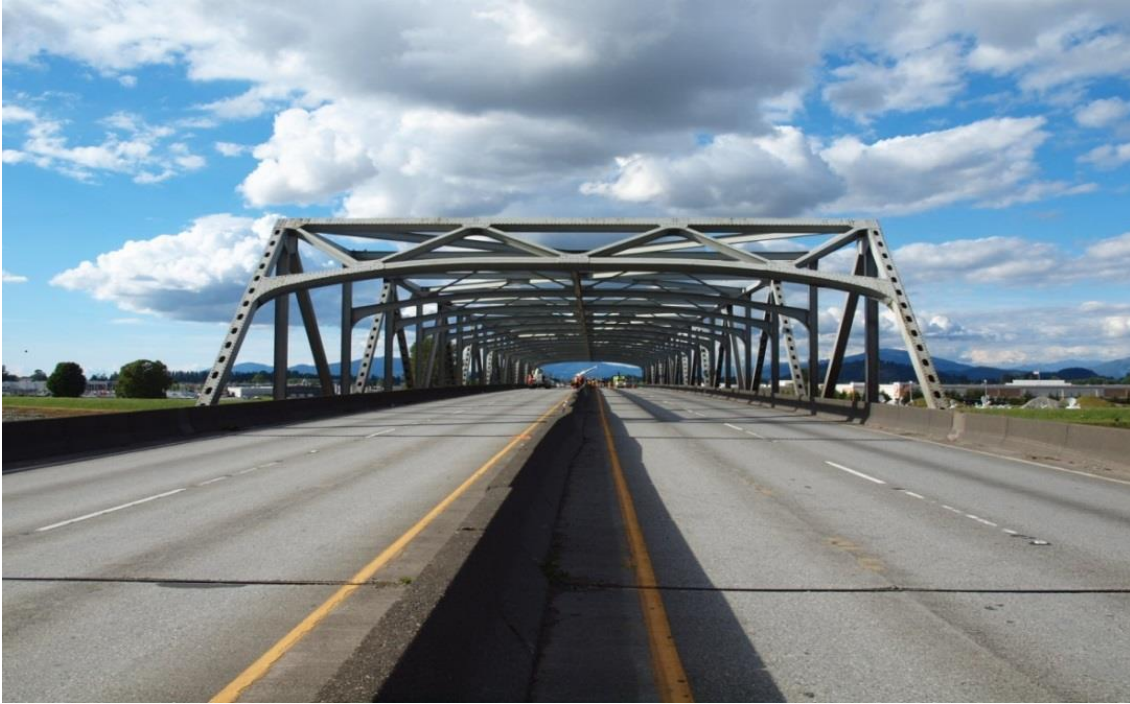
Figure 5. Looking northward at the Skagit River Bridge on May 24, 2013. The through-truss structure is the portion above the roadway.
