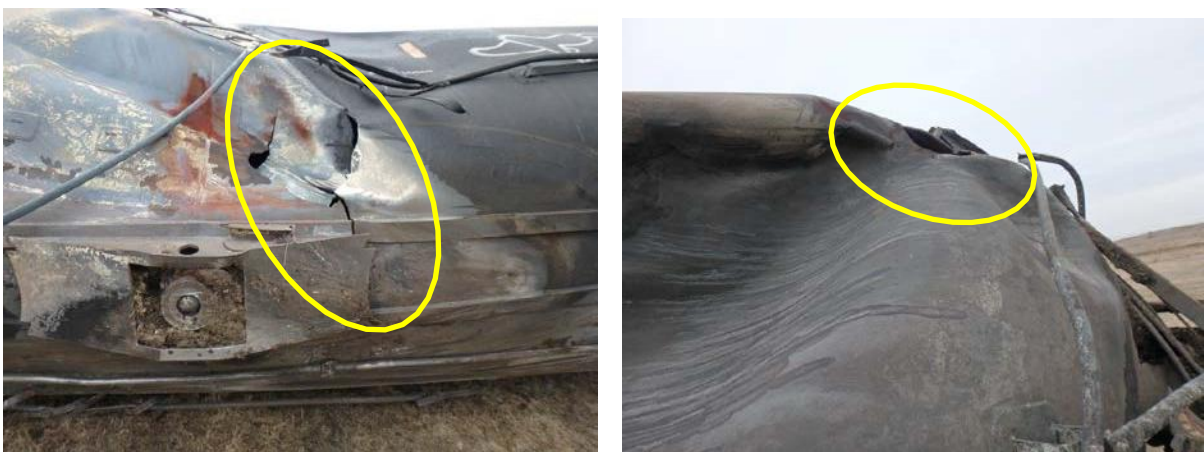
Figure 21 CTCX 731383 shell puncture (left circled) and B-end head fracture (right circled), staging area, March 12, 2017.
