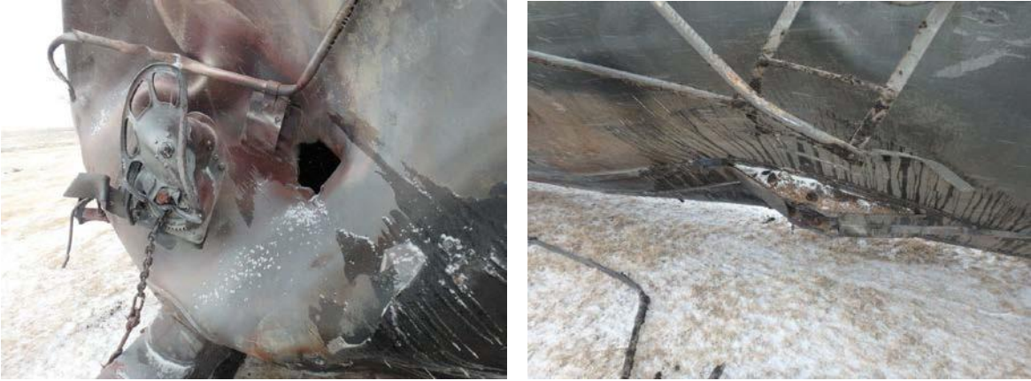
Figure 15: GATX 203812 / TAEX 2909, punctured B-end head (left) and bottom dent over the bottom outlet valve (right), staging area, March 12, 2017.
