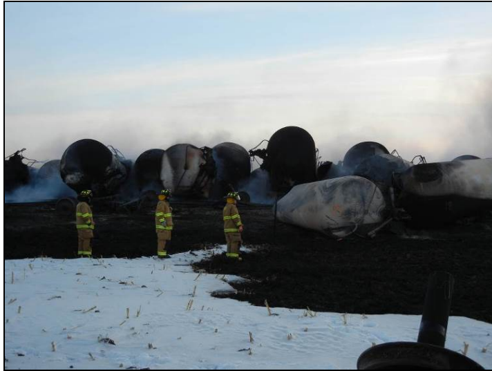
Figure 16: Image of derailment taken from the North.
