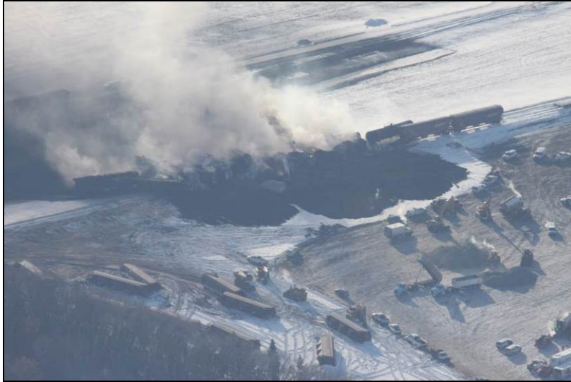
Figure 4: Aerial image of accident site taken from the Northeast. (Photograph courtesy of the US Customs and Border Patrol)
