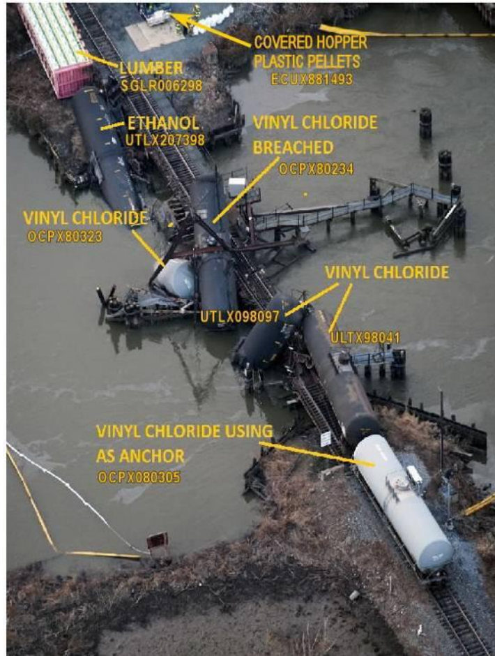
Figure 4 - Aerial image (from the East) of the train derailed on the Paulsboro movable bridge. (Photograph courtesy of the United States Coast Guard)
