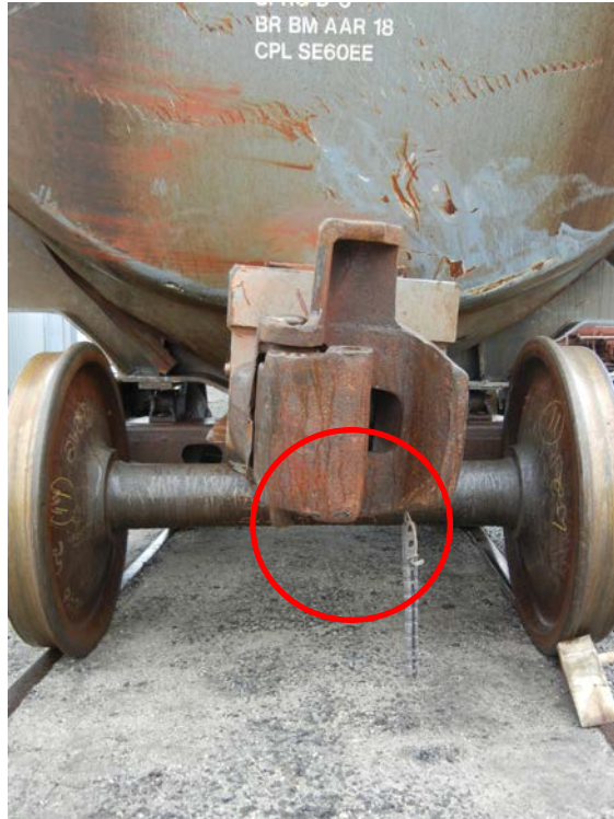
Figure 15: Broken bottom shelf (highlighted in red) of A-end SE60EE double-shelf coupler on tank car OCPX 80323.
