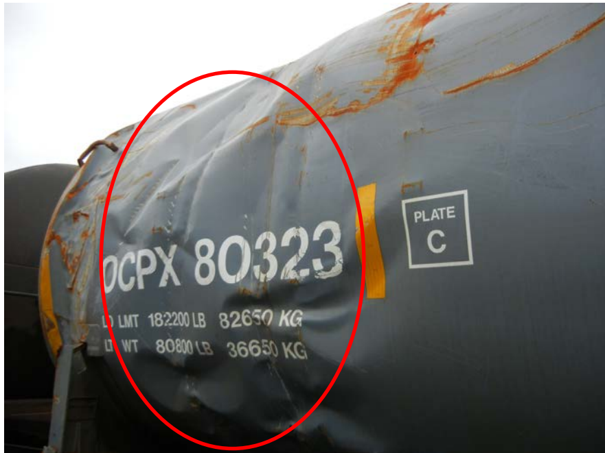
Figure 8: Damage to the B-right side (including damage caused by crane operations – highlighted in red) of tank car OCPX 80323.
