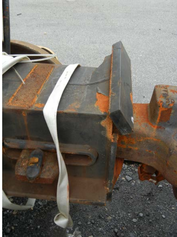
Figure 6: Damage to B-end striker plate and stub sill from a different angle.
