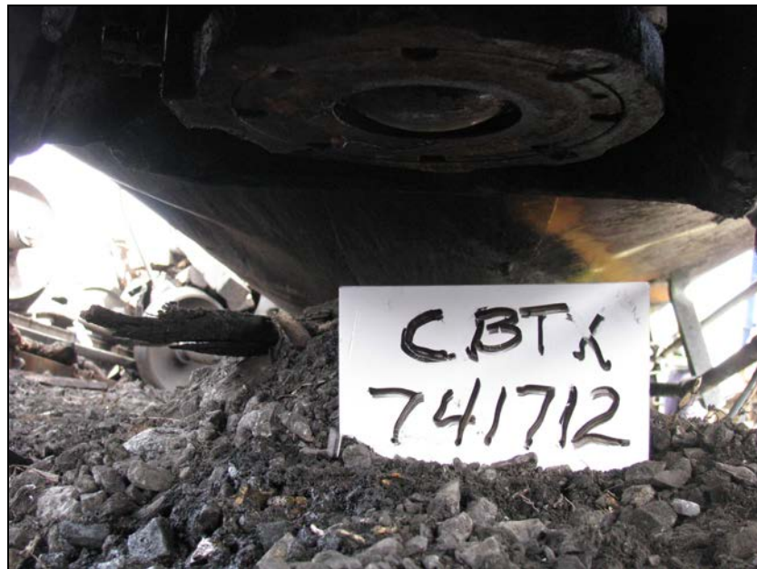
Figure 15: Sheared off bottom outlet nozzle of CBTX 741712.
