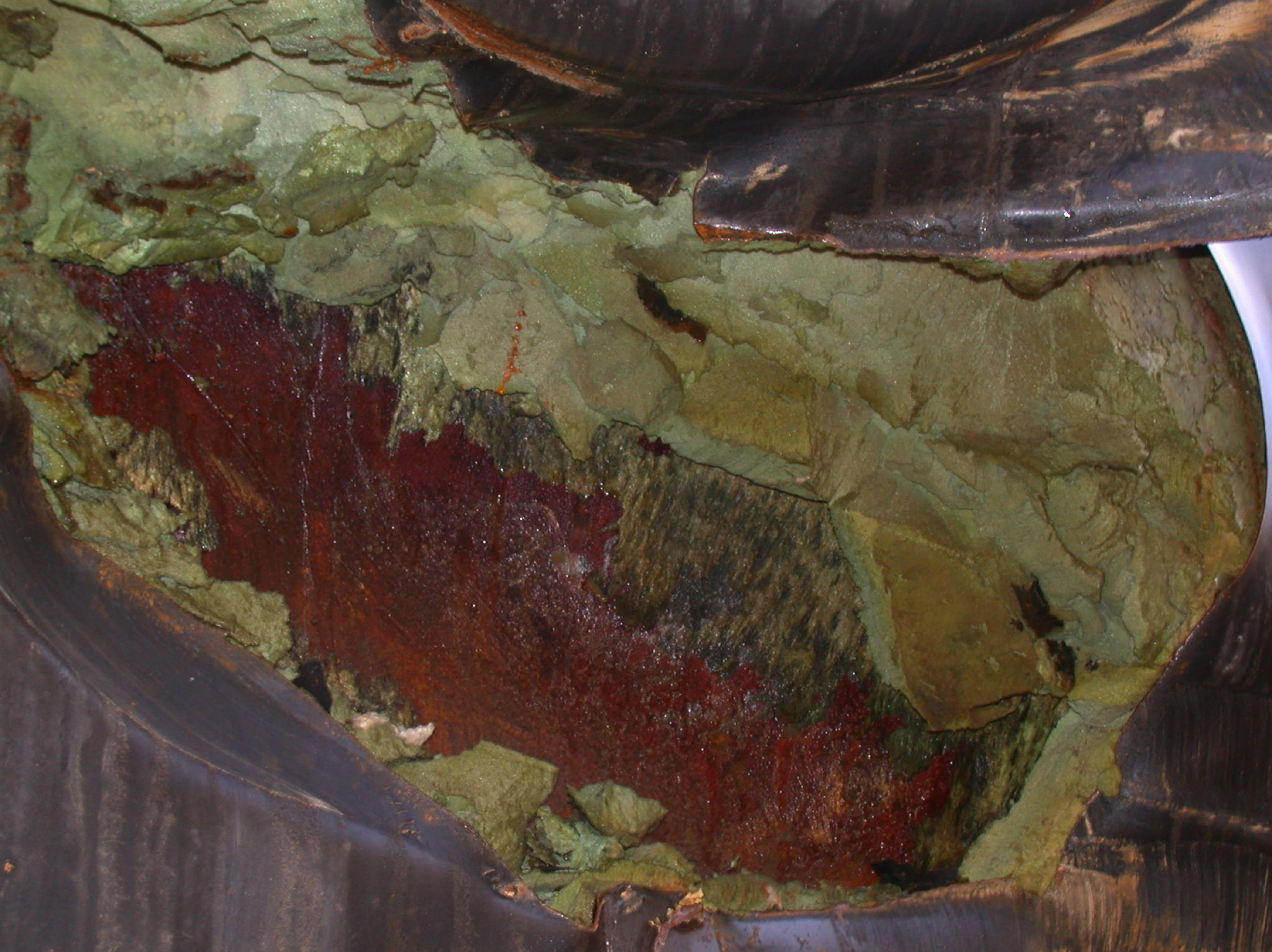
Haz/Mat Appx J - GATX 17105 Left Side at A-end - Markings and Severe Dent
