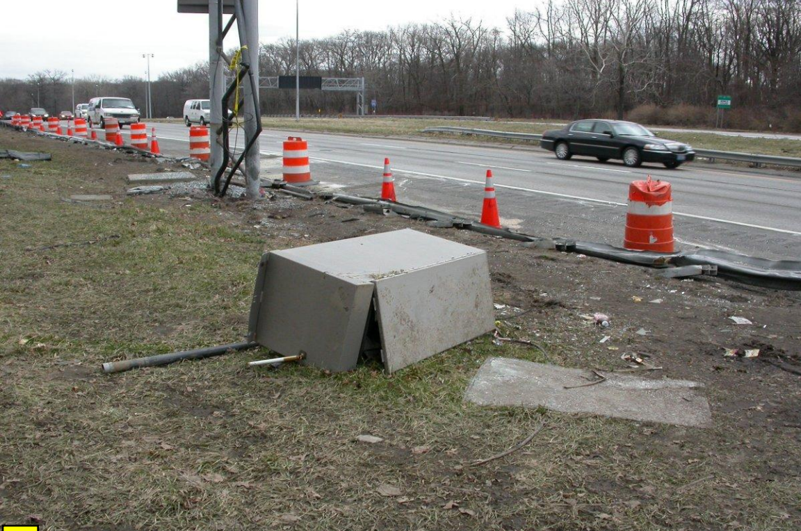
Y Photo-17, Illustrating the final rest of the cabinet after the accident
