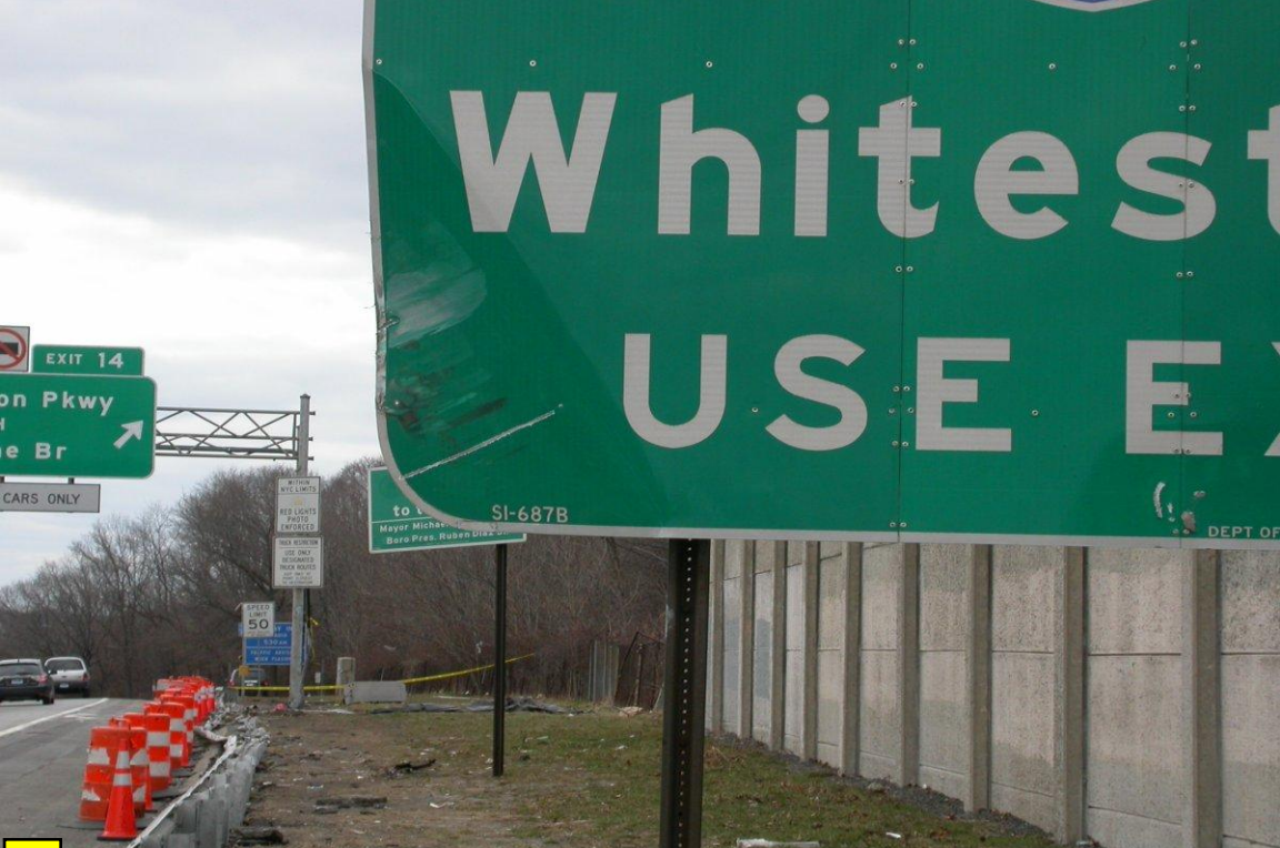
Y Photo-12, Illustrating the damage to lower left hand corner of Sign #2
