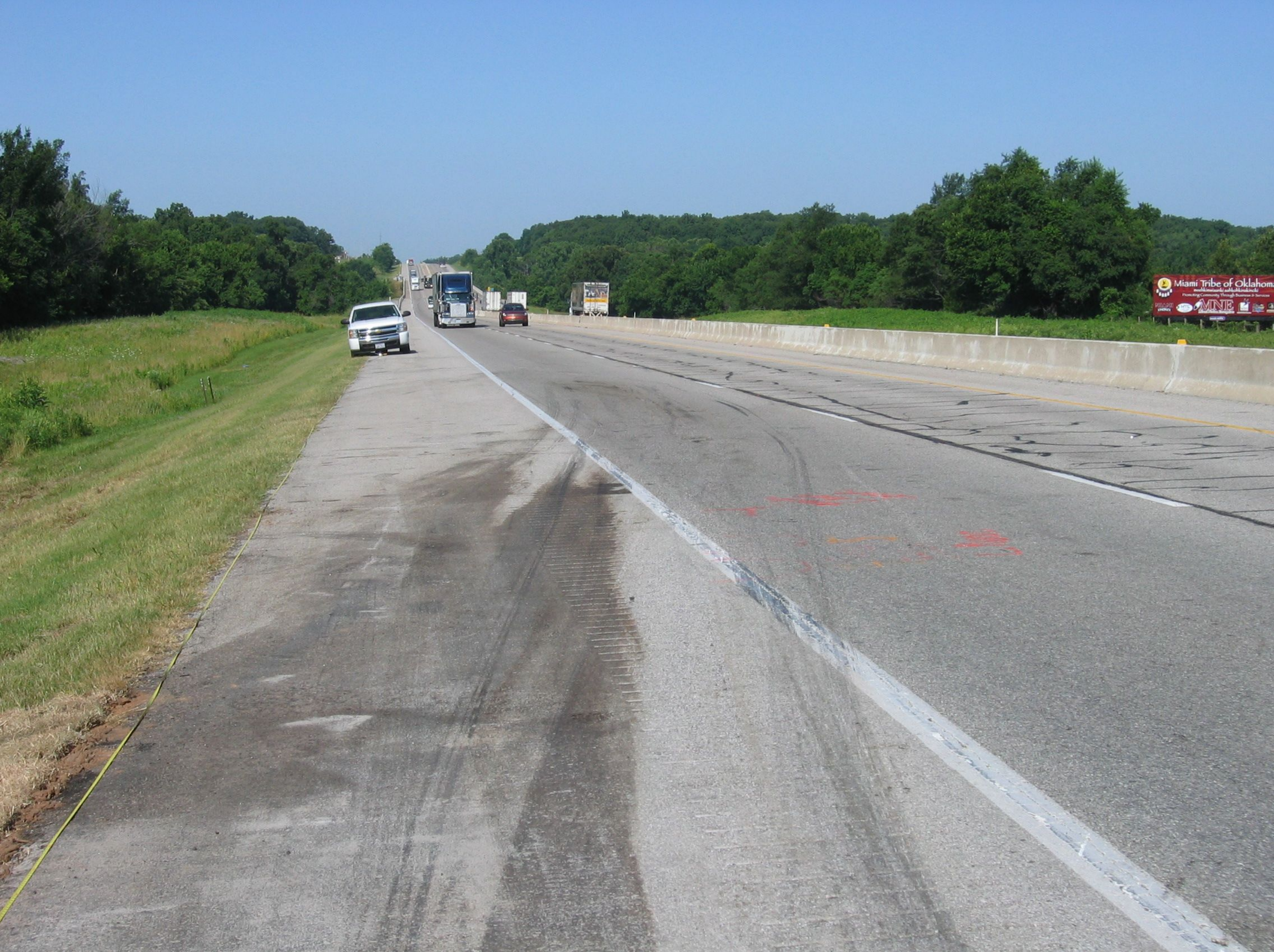
HWY Photo 15, Additional Opposite Direction View of Pavement Gouges and Tire Marks
