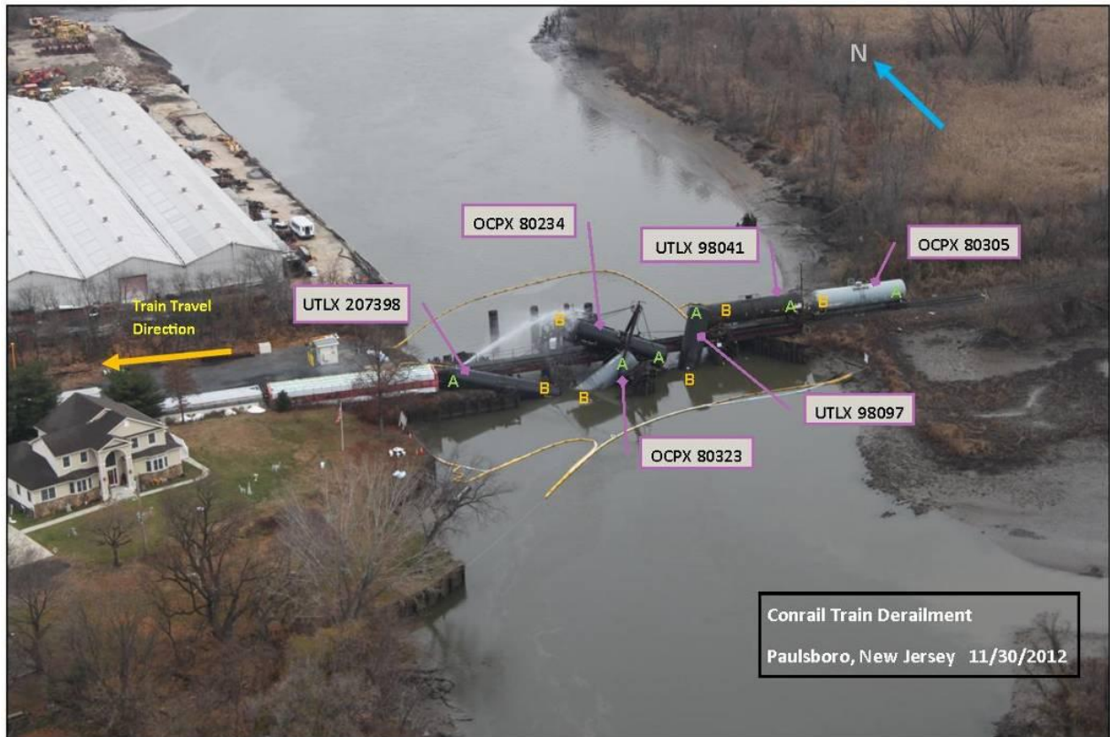
Figure 3 - Aerial photograph (from the South) of the train derailment on the movable bridge in Paulsboro on December 1, 2012. (Photograph courtesy of the New Jersey State Police)
