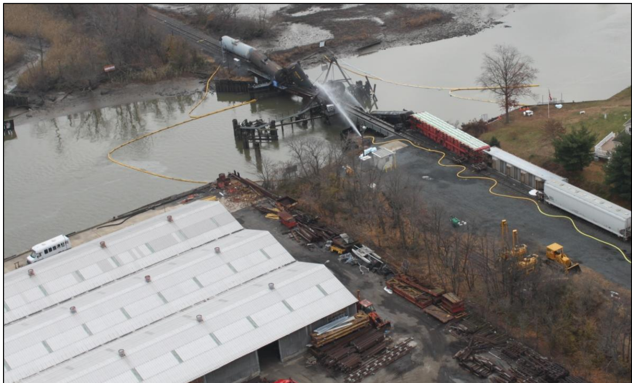
Figure 1-Aerial Photo of the Derailment
