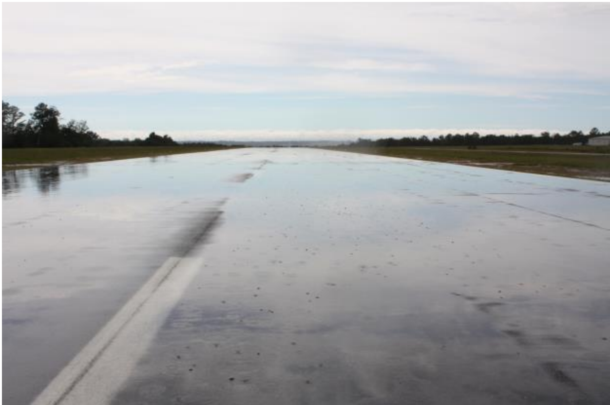
Photo 2: Ponding Following a Rain shower Looking West on Runway 28 (Courtesy of the Operator)
