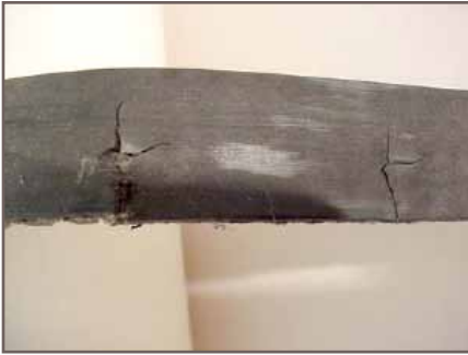
Figure 19 - Tensile cord failure from debris
