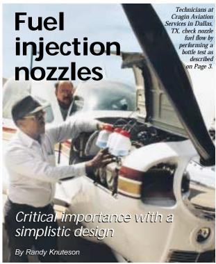
Livery fuel injection system made today requires that a calibrated device be used to accurately deliver a precise amount of fuel to each cylinder at the exact instant fuel is needed for combustion.
