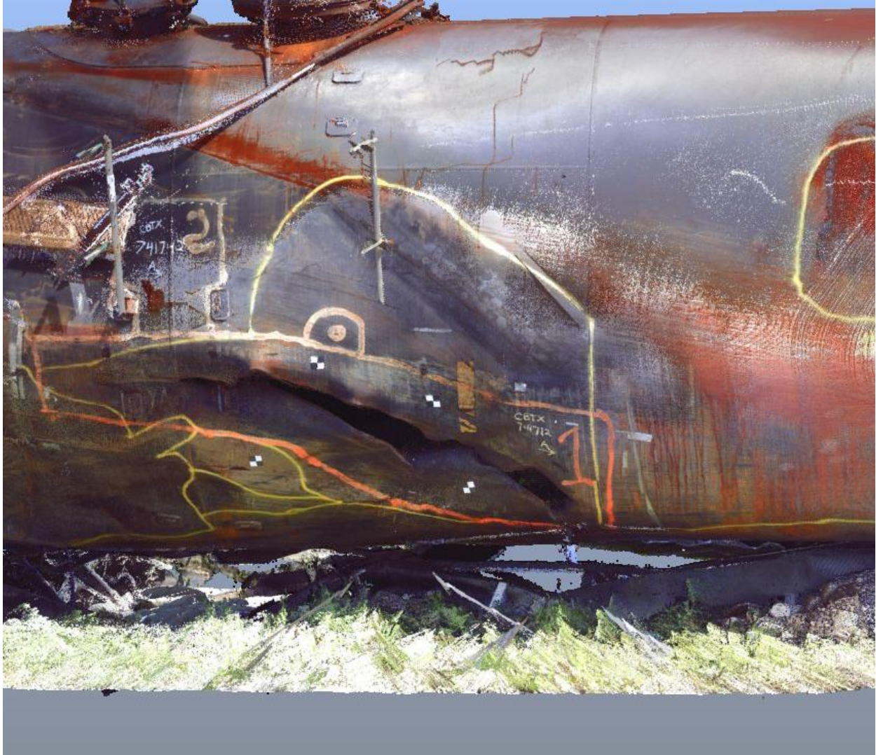
Figure 3: An image from the 3D laser scanner point cloud showing a close-up of the gash in the found on the left side of tank car CBTX 741712. Prior to the accident the tank car was traveling B-end leading.
