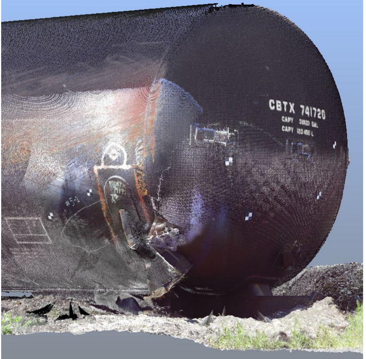
Figure 6: An image from the 3D laser scanner point cloud showing a close-up image of the A-end of car CBTX 74720 and the damage to left side bolster. Prior to the accident the tank car was traveling B-end leading.
