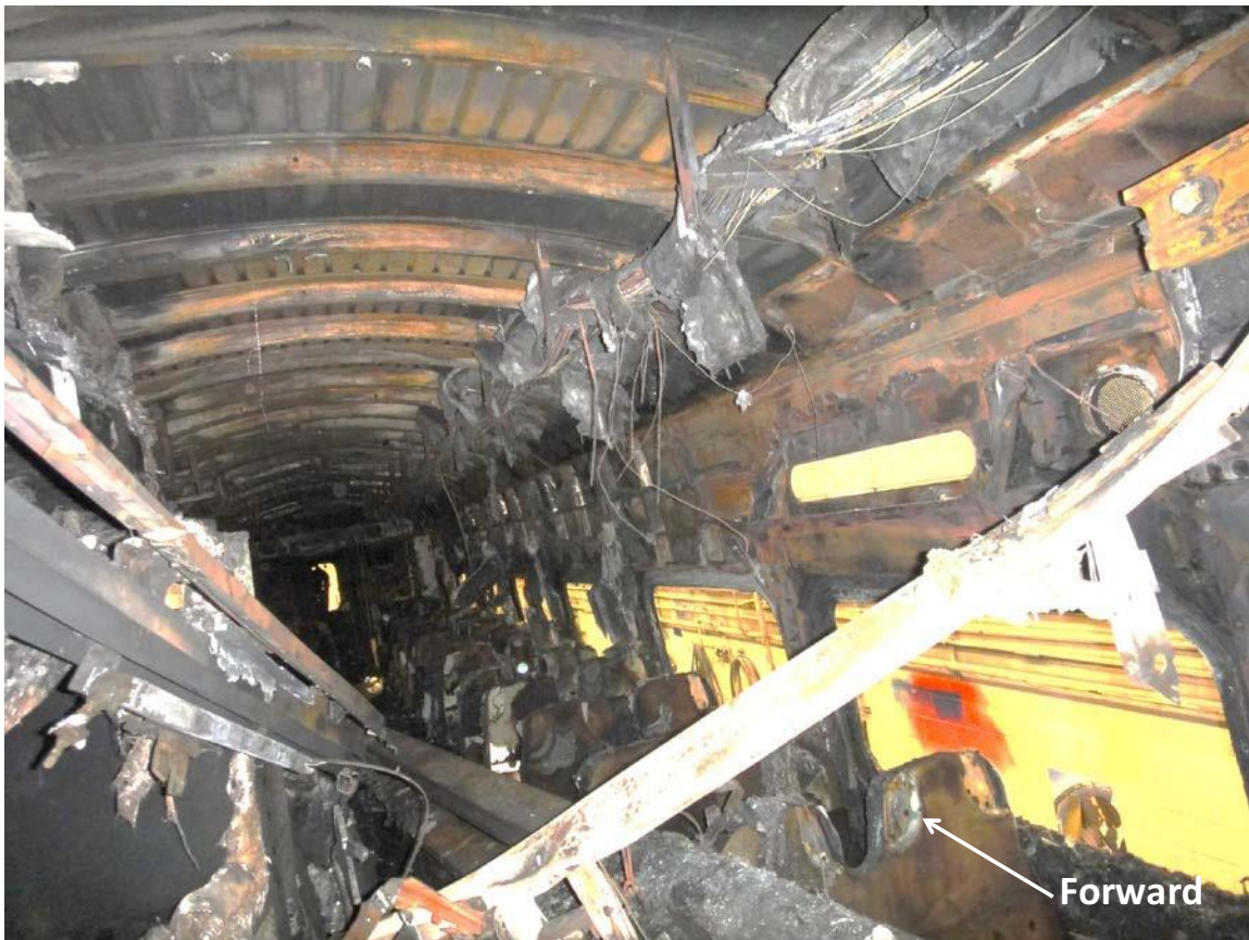
Figure 23. Section of cable run near the right rear passenger door.
