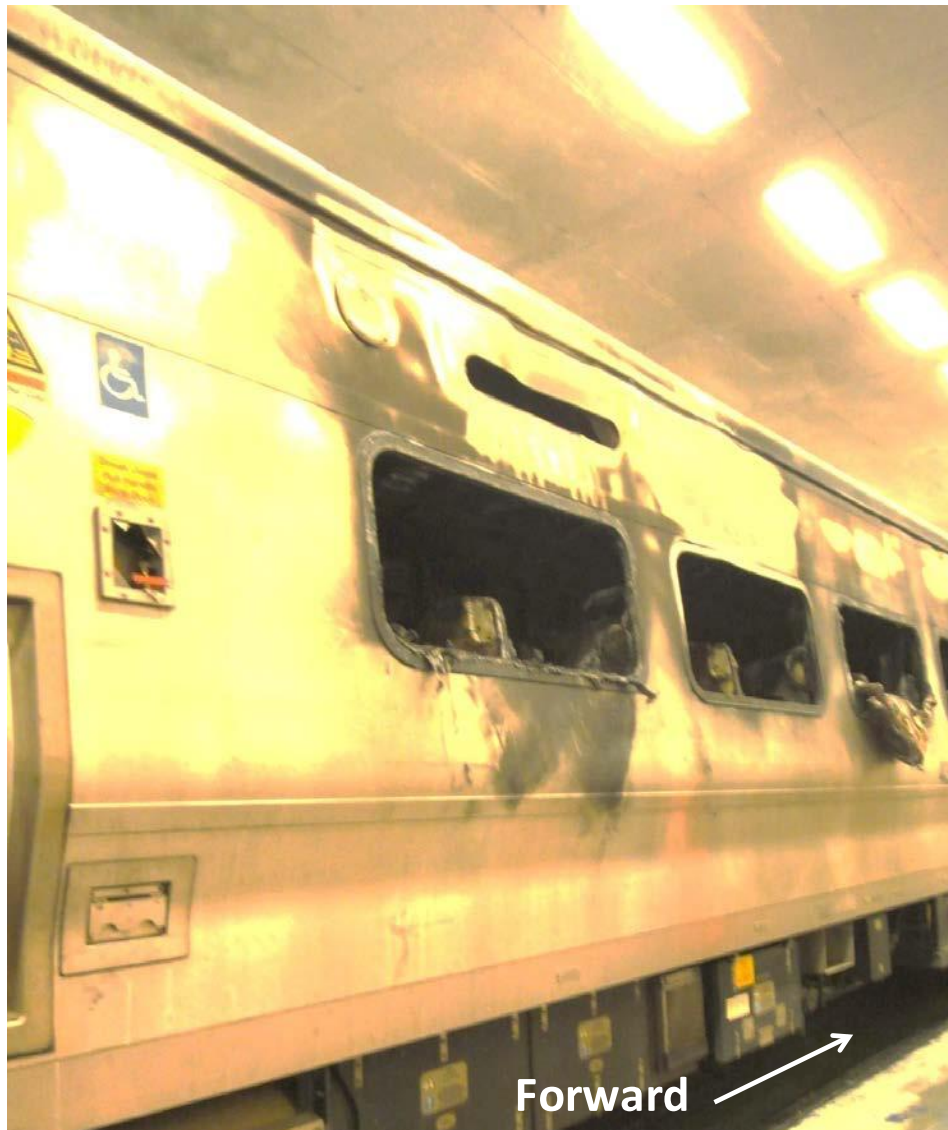
Figure 13. Right side exterior from fifth (R5) to seventh (R7) window.
