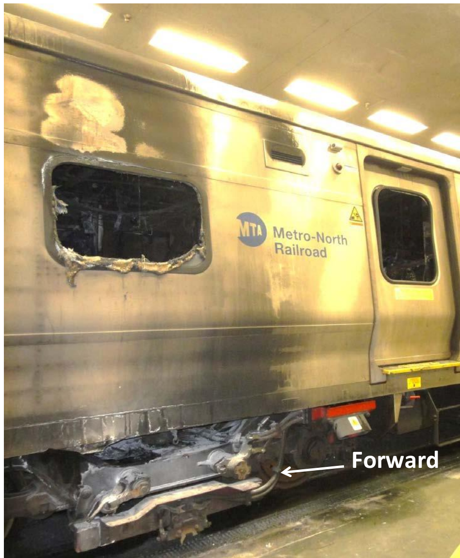
Figure 6. Left side section of exterior car body between L1 window and F-end passenger door.
