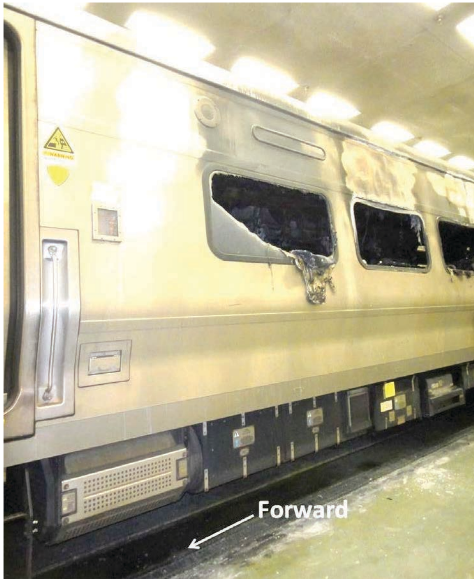
Figure 7. Left side exterior from F-end passenger door to fourth (L4) window.
