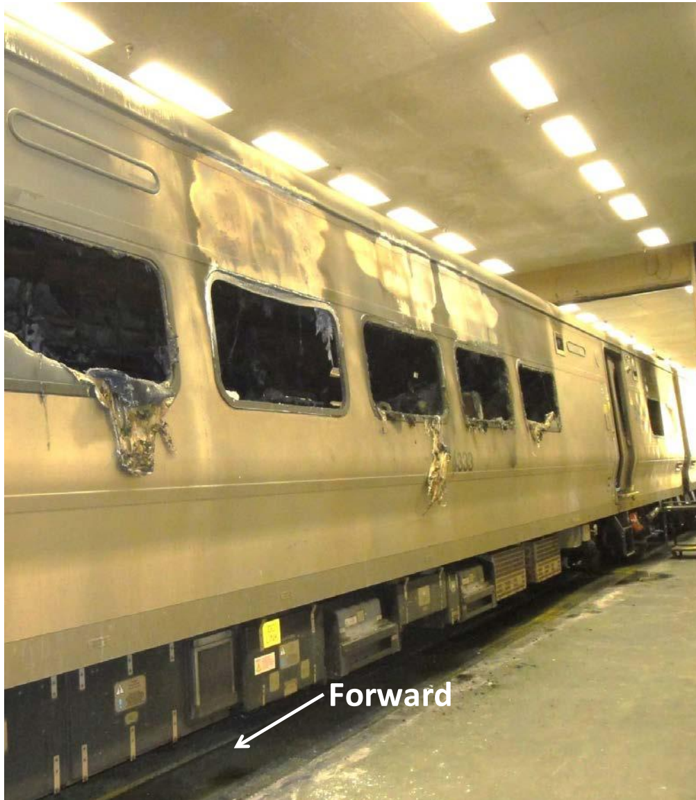
Figure 8. Left side exterior from second (L2) window to sixth (L6) window.
