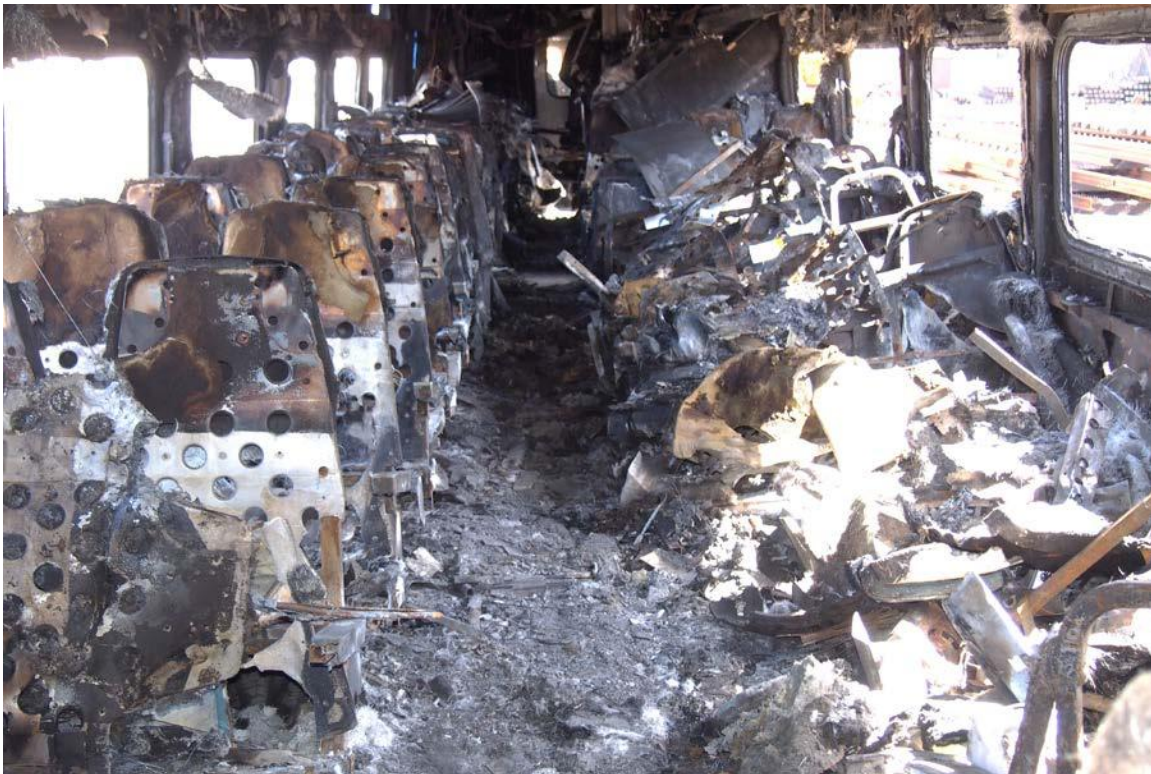
Figure 17. Passenger Compartment - Overall interior of MN 4333 after the removal of the injected rail.
