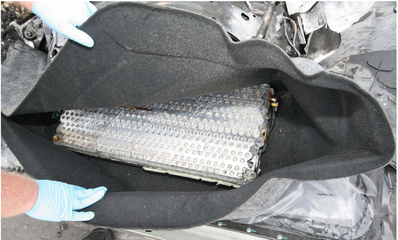
Figure 9: Battery module without fire damage.
