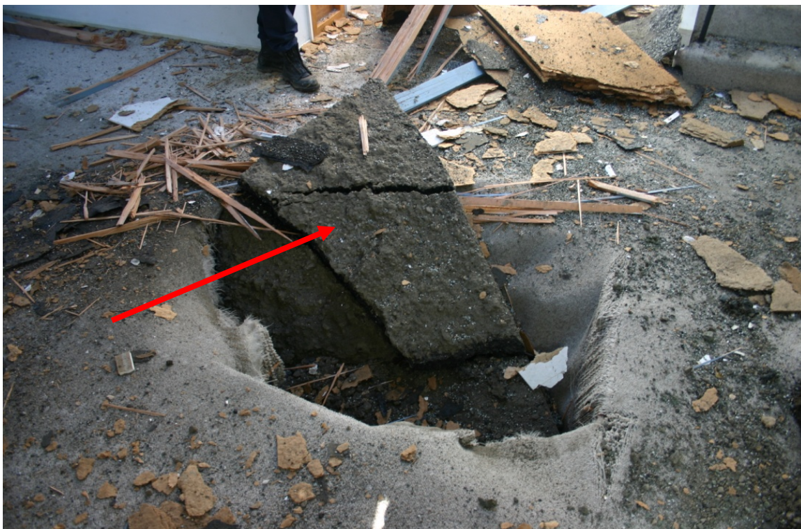
Figure 8. Picture of asphalt debris (highlighted with a red arrow) that penetrated the roof of a house near the accident site.
