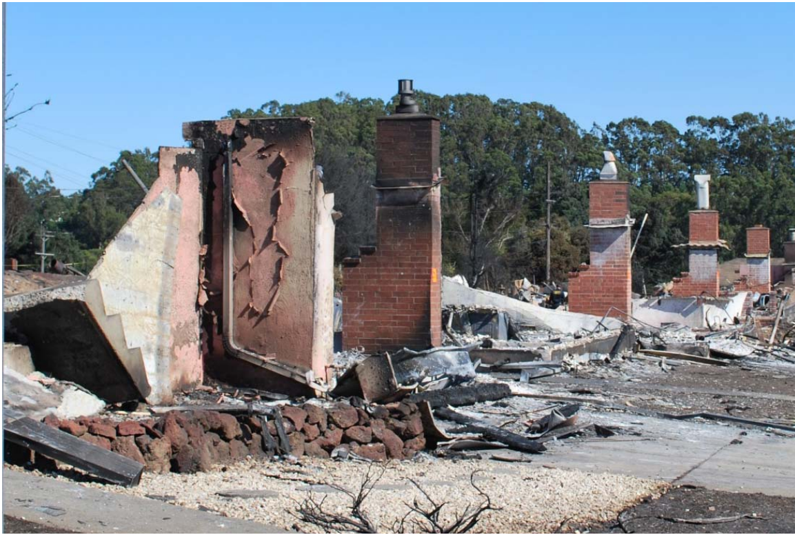
Figure 5. A row of four destroyed houses on Claremont Avenue.
