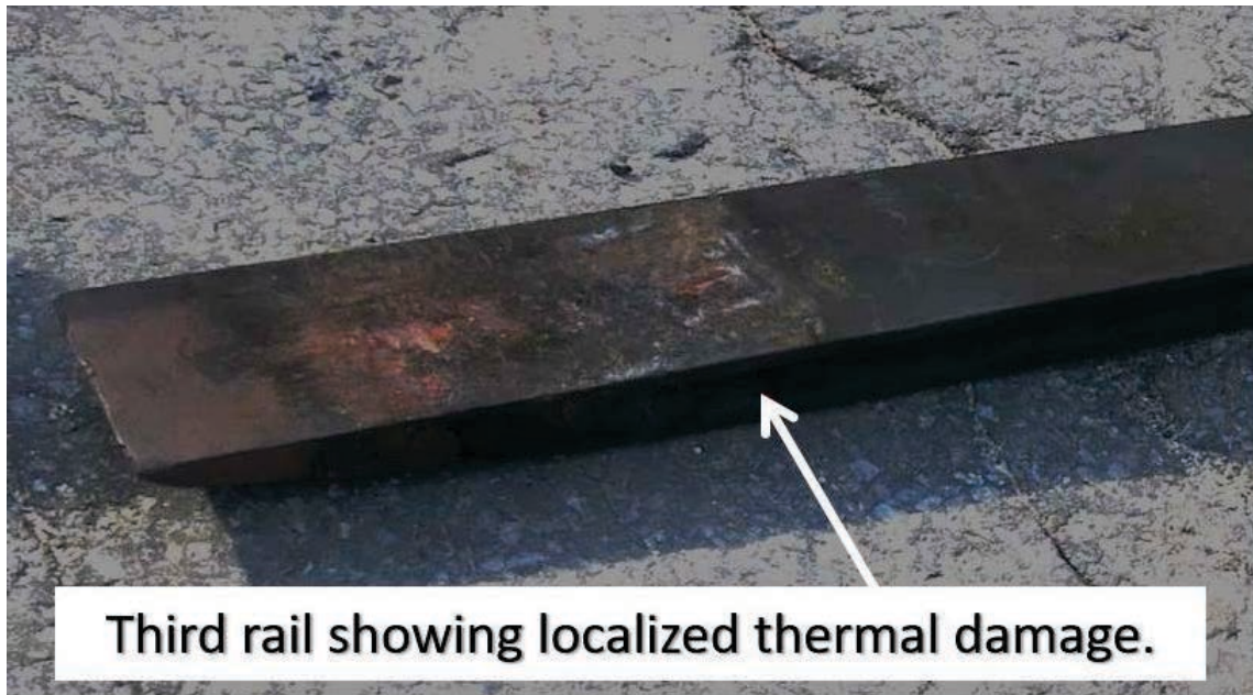
Figure 20. Localized thermal damage to the third rail nose piece surface removed from the lead railcar.
