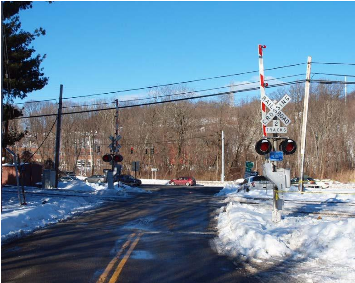
Figure 10. Approach of the Commerce Street grade crossing, facing northeast.
