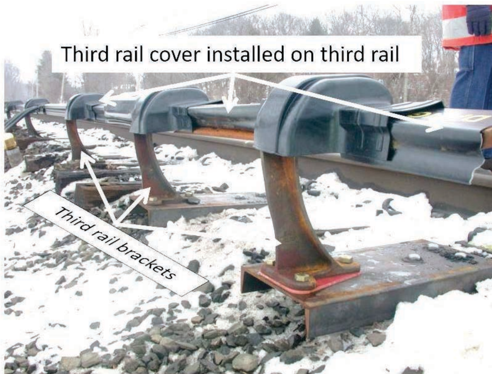
Figure 13. Metro-North's third rail configuration.
