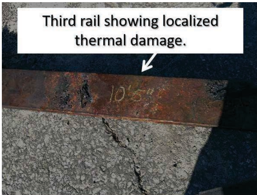
Figure 21. Localized thermal damage to the surface of the third rail removed from the SUV.
