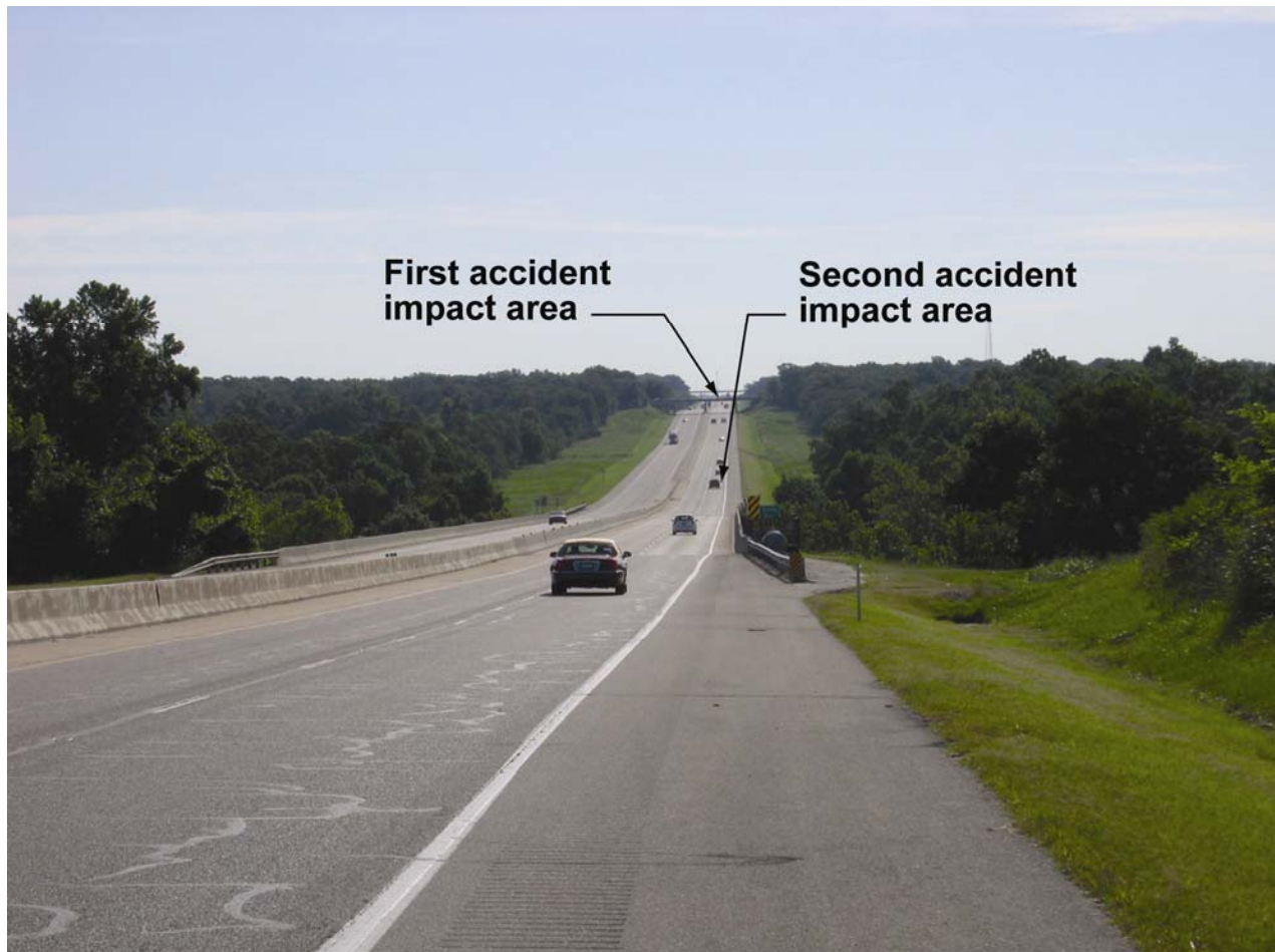
Figure 6. View of I-44 eastbound, showing the sites of the June 26, 2009, accidents.
