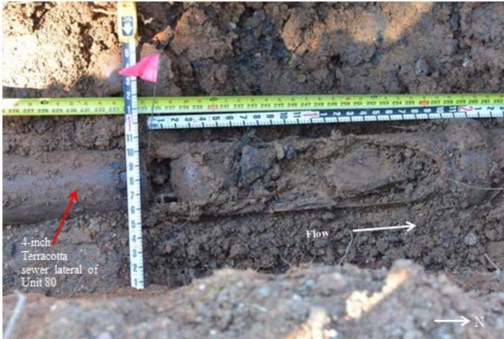
Figure 15: Measured damage section on the 4-inch" east end sewer lateral to Unit 80. Source: HABD Insurance Forensic Excavations
