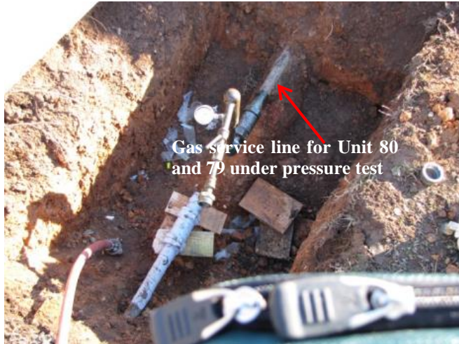
Figure 21: Gas flow isolation point where pressure tests of the branched services of Units 79 and 80 measured by pressure gauge and recorded on pressure chart.
