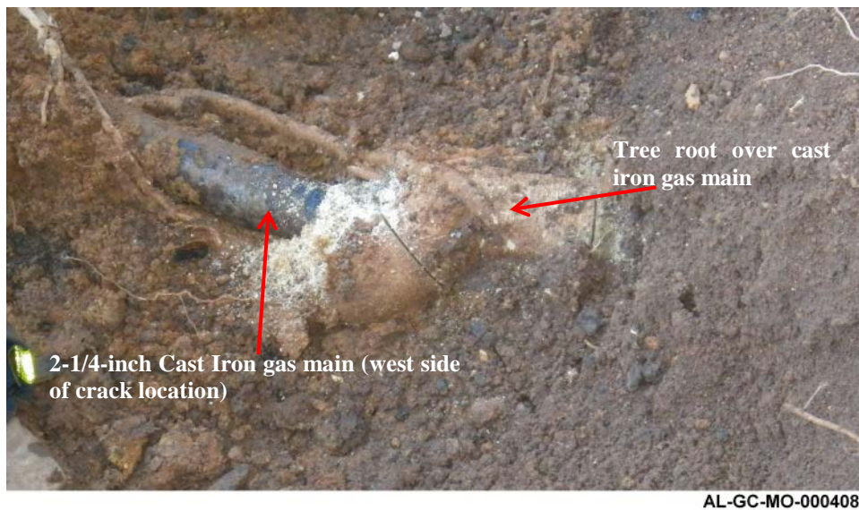
Figure 19: Tree root at the point of crossing 2-1/4-inch cast iron main opposite Unit 80. Source: Alagasco
