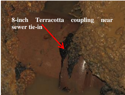
Figure 13: 8-inch male and female sewer main coupling with coal tar coating.
