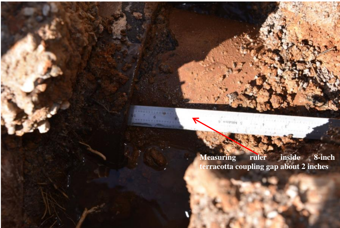
Figure 14: 8-inch sewer main with gap in the coupling. Source: HABD Insurance Forensic Excavations.
