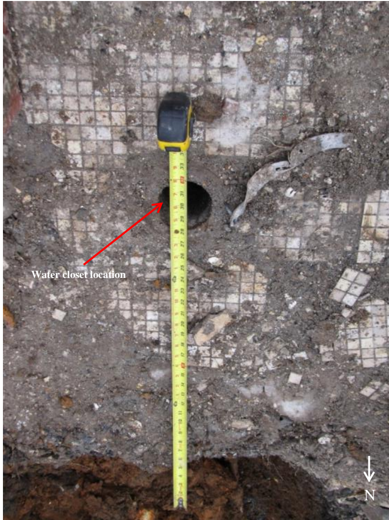
Figure 7: Water closet drain is positioned about 30 inches from east foundation wall of Unit 80.
