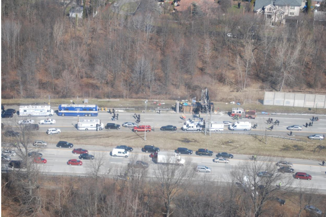
Figure 2. Aerial view of I-95 and accident site. (Source: New York State Police [NYSP].)
