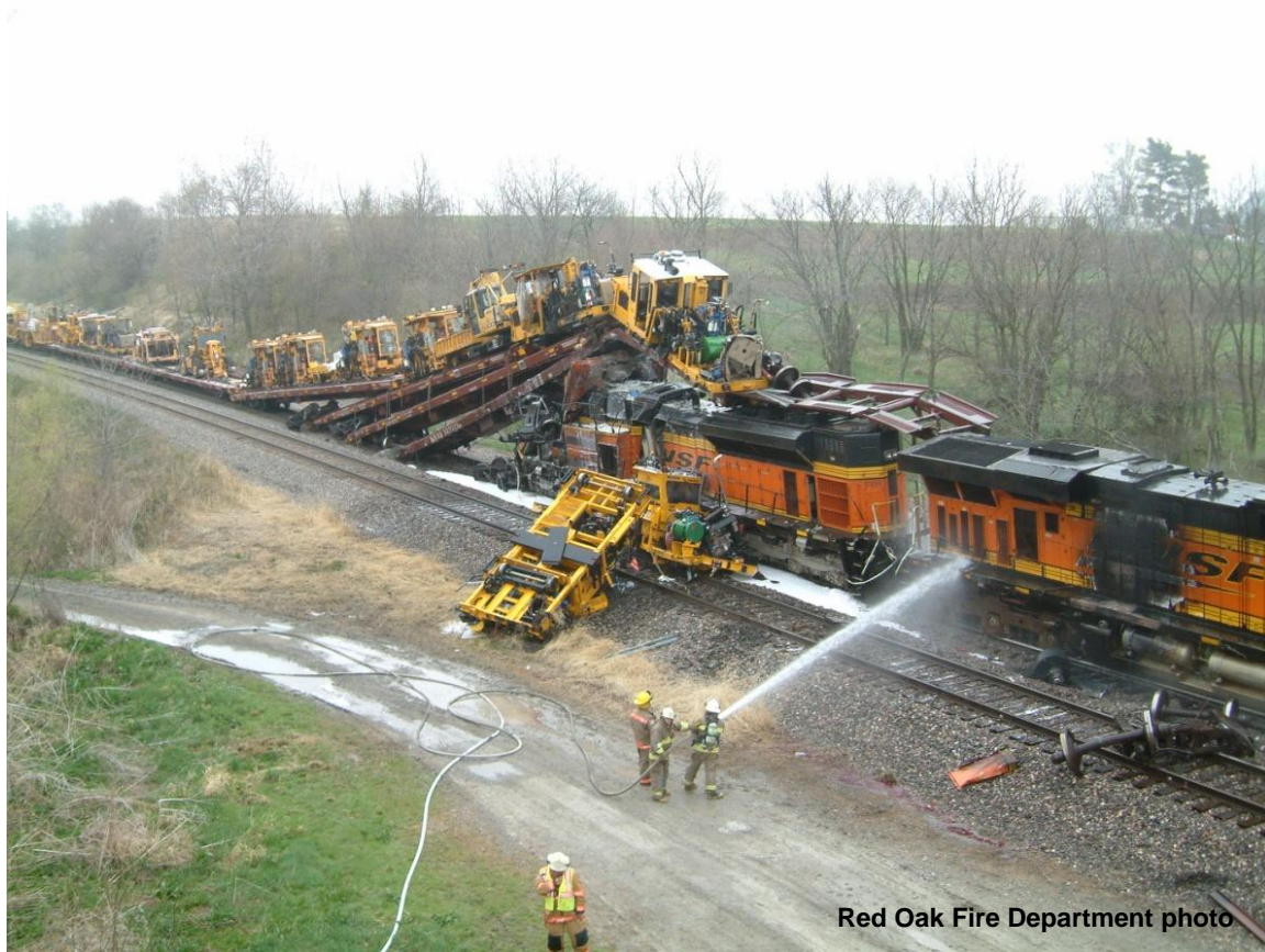
Figure 22. Red Oak Fire Department applying foam after collision.
