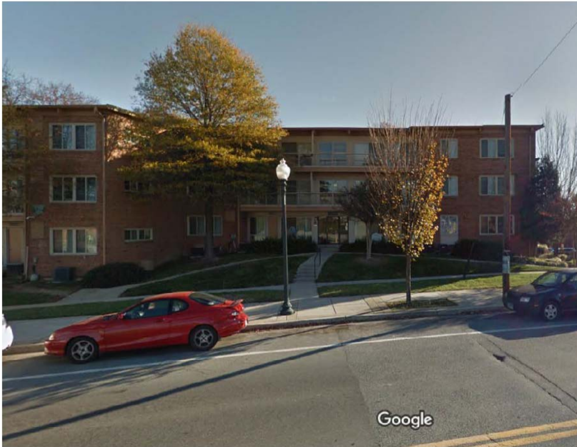
Figure 1. The accident location, 8701 Arliss Street, before the August 10, 2016, explosion. (Photograph from Google Earth, dated November 2015.)
