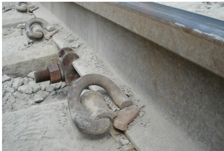
Figure 10: Insulator between pandrol clip and rail base of the type without metal insert. Note that insulator has slipped above base of rail on field side.
