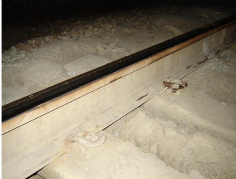
Figure 7: Marks on gage side of base of low rail at POD
