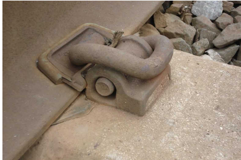
Figure 9: Insulator between pandrol clip and rail base of the type with metal insert. Note that insulator has slipped above base of rail on field side.
