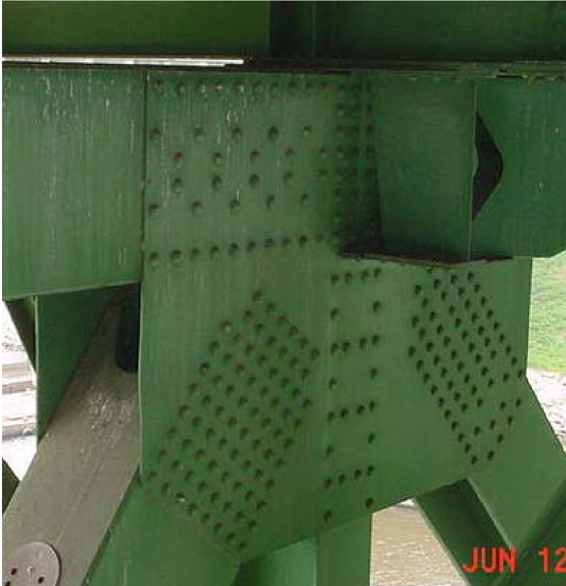
Figure 63. Picture of U10'E connection taken on 12 June 2003.
