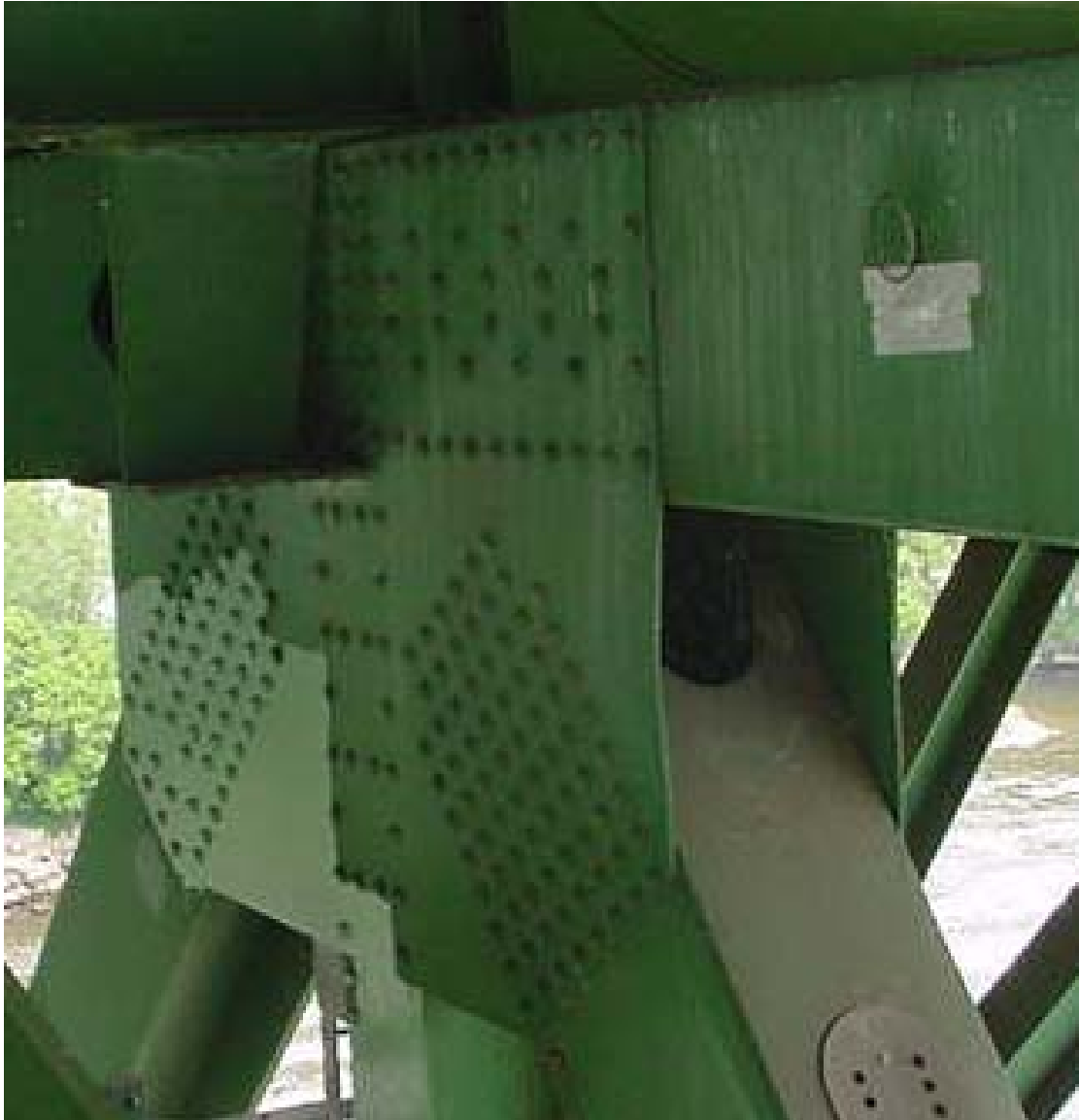
Figure 61. Picture of U10E connection taken on 12 June 2003.
