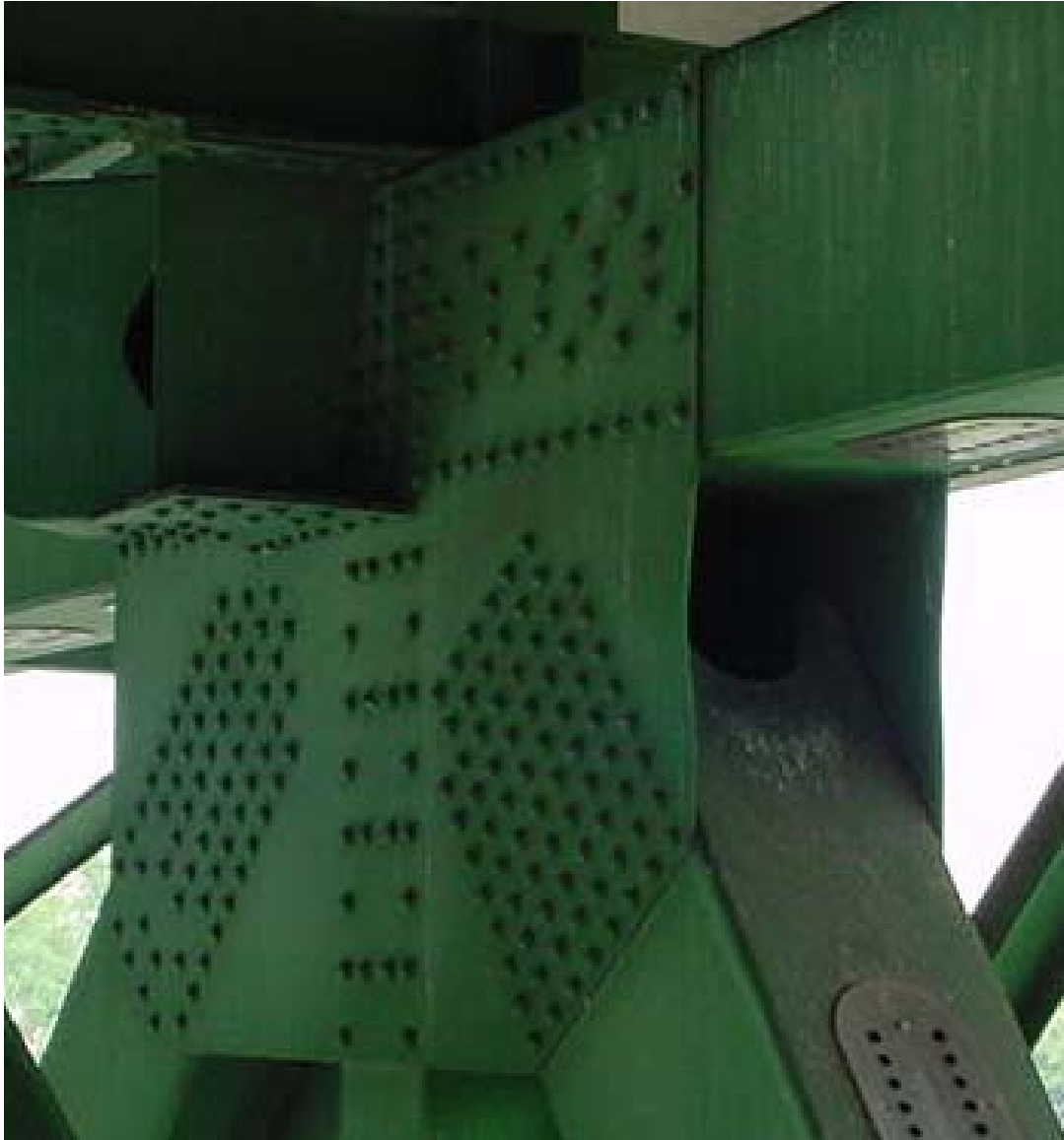
Figure 64. Picture of U10'W connection taken on 10 June 2003.
