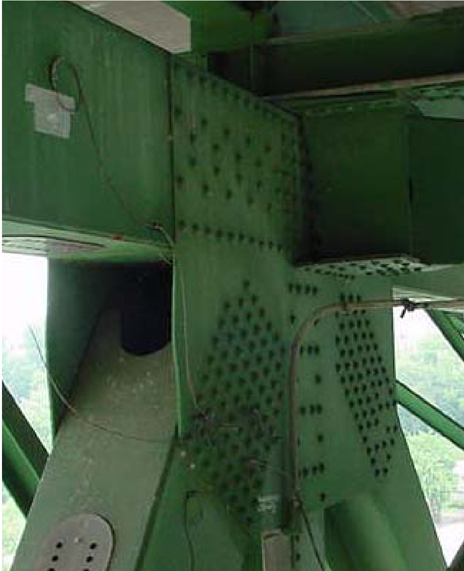
Figure 62. Picture of U10W connection taken on 10 June 2003.
