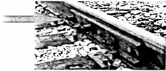
STANDARD RAIL JOINT BAR
