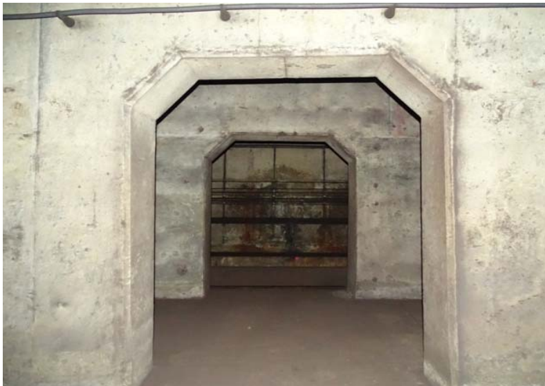
Photograph No. 15 Storage area, section 2, middle portion.
