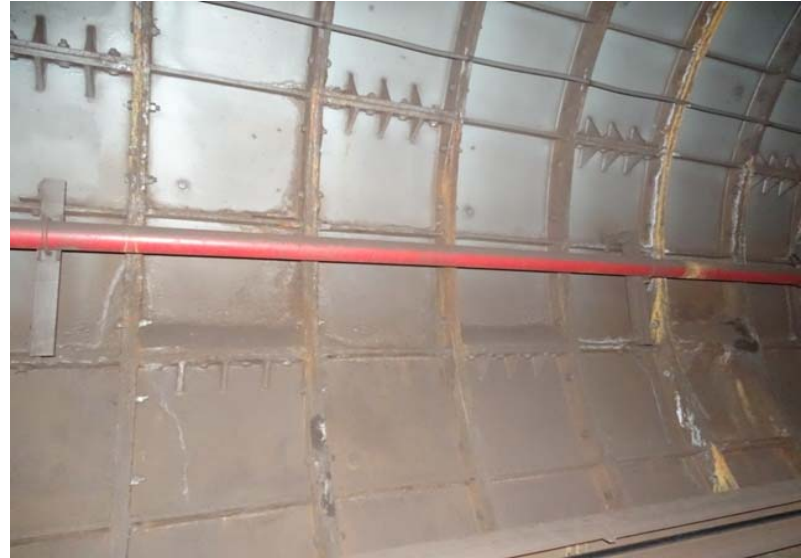
Photograph No. 2 Station 69+70, east wall.
