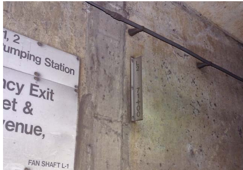
Photograph No. 72 Station 71+00 - marker for L2 71+00.
