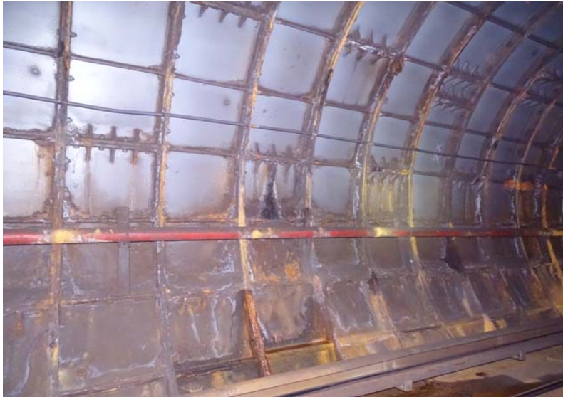
Photograph No. 21 Station 70+10, east wall.
