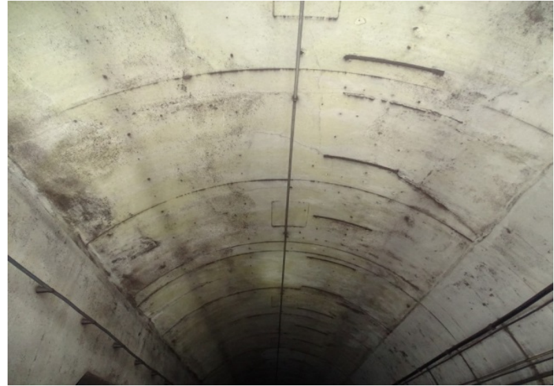
Photograph No. 566 Station 78+50, ceiling.
