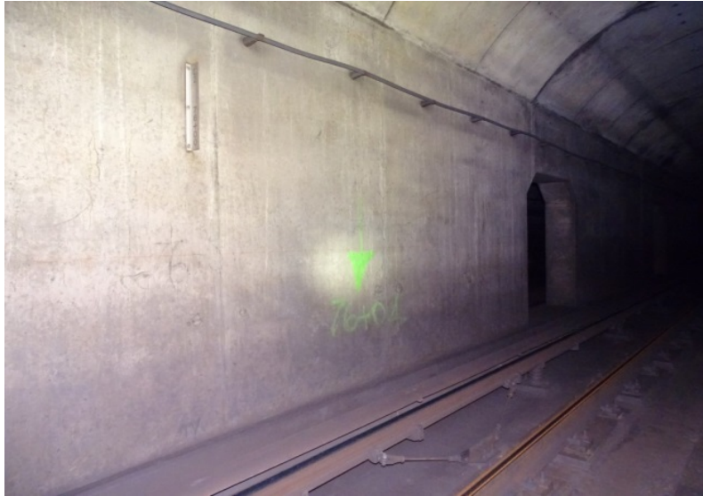
Photograph No. 421 Station 76+00, east wall.
