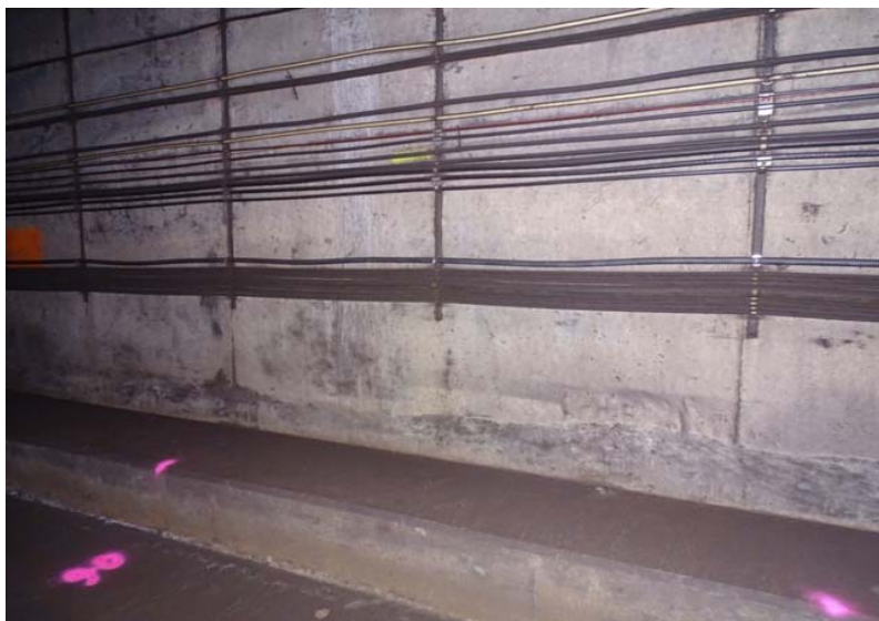
Photograph No. 267 Station 73+80, lower portion of west wall.
