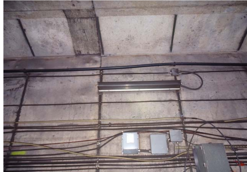
Photograph No. 142 Station 72+00, upper portion of west wall.
