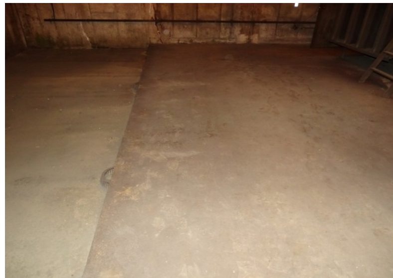
Photograph No. 174 Upper fan room floor, north section, center portion.
