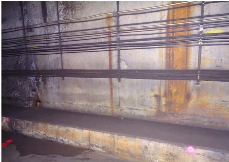
Photograph No. 89 Station 71+20, lower portion of west wall.
