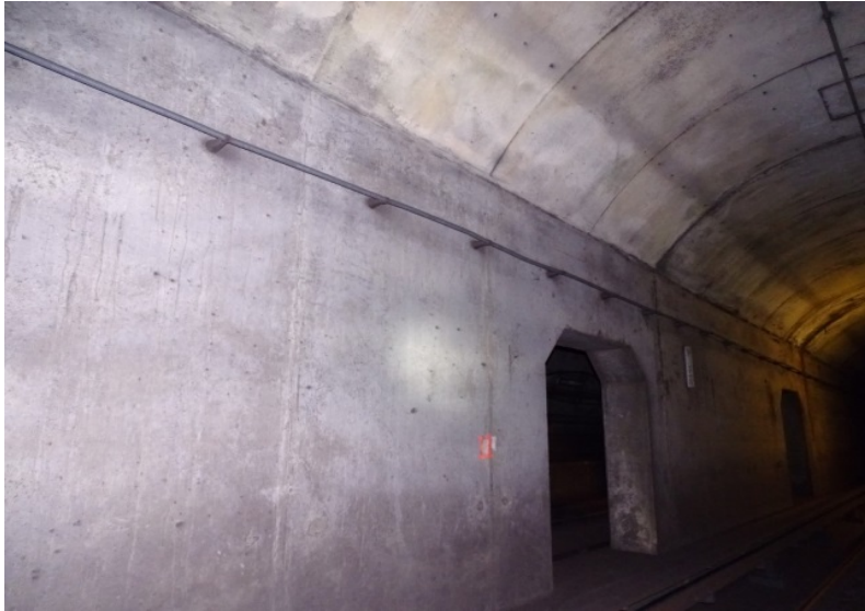
Photograph No. 477 Station 76+80, east wall.
