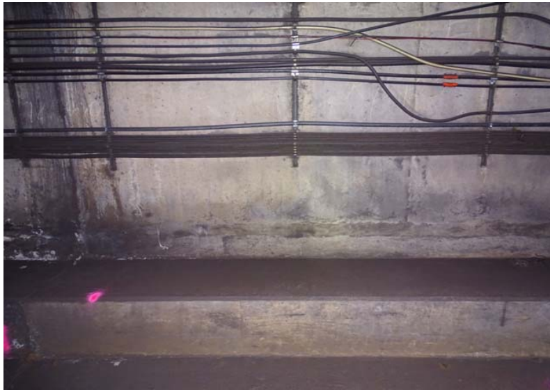
Photograph No. 229 Station 73+20, lower portion of west wall.
