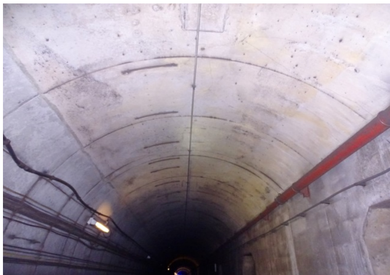
Photograph No. 223 Station 75+40, ceiling.
