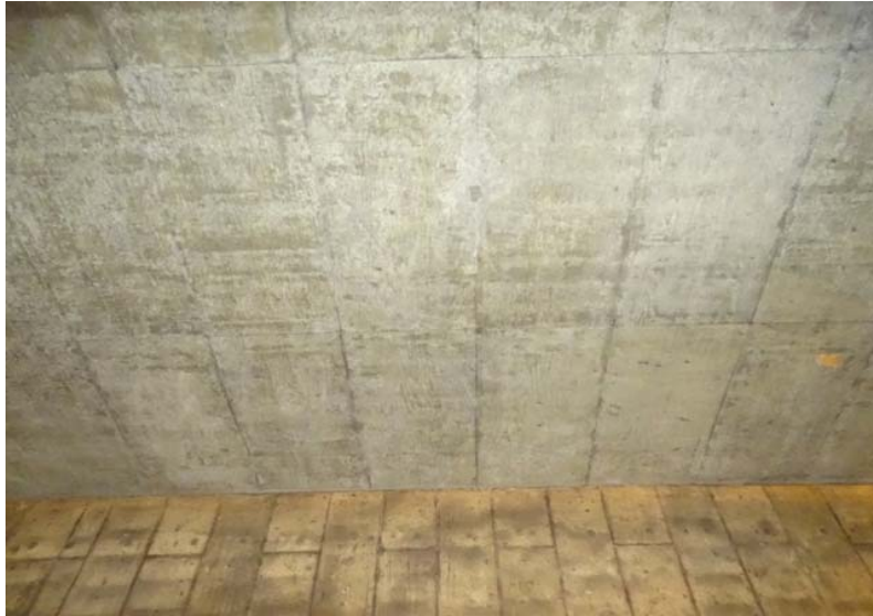
Photograph No. 105 Main room, ceiling, section 2.
