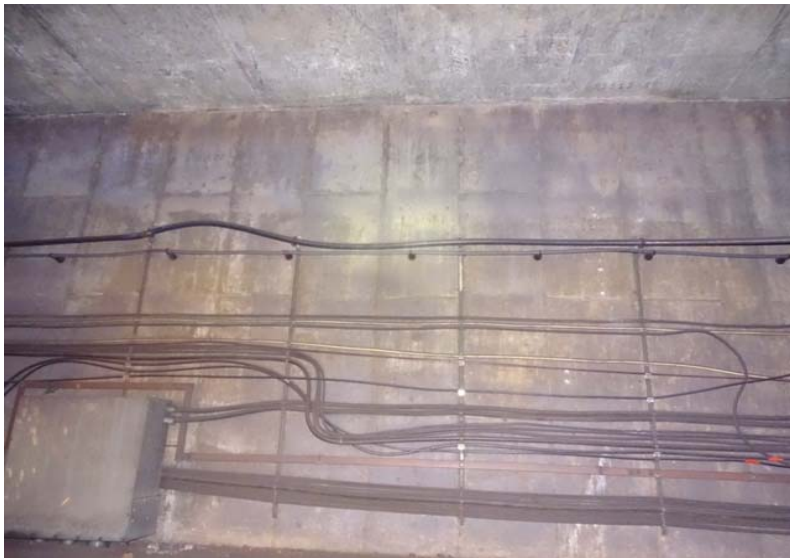
Photograph No. 47 Station 70+50, upper portion of west wall.
