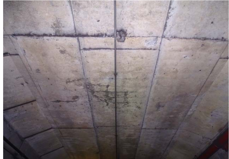
Photograph No. 94 Station 72+20, ceiling.
