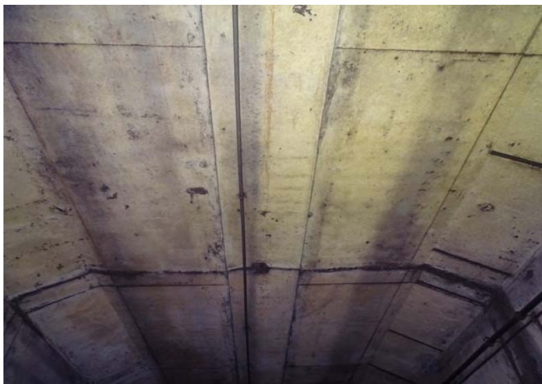
Photograph No. 227 Station 73+20, ceiling.
