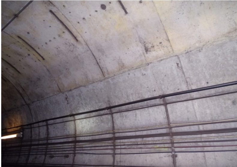
Photograph No. 381 Station 75+40, upper portion of west wall.
