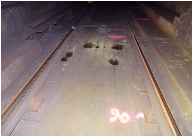
Photograph No. 67 Station 70+90, track bed.
