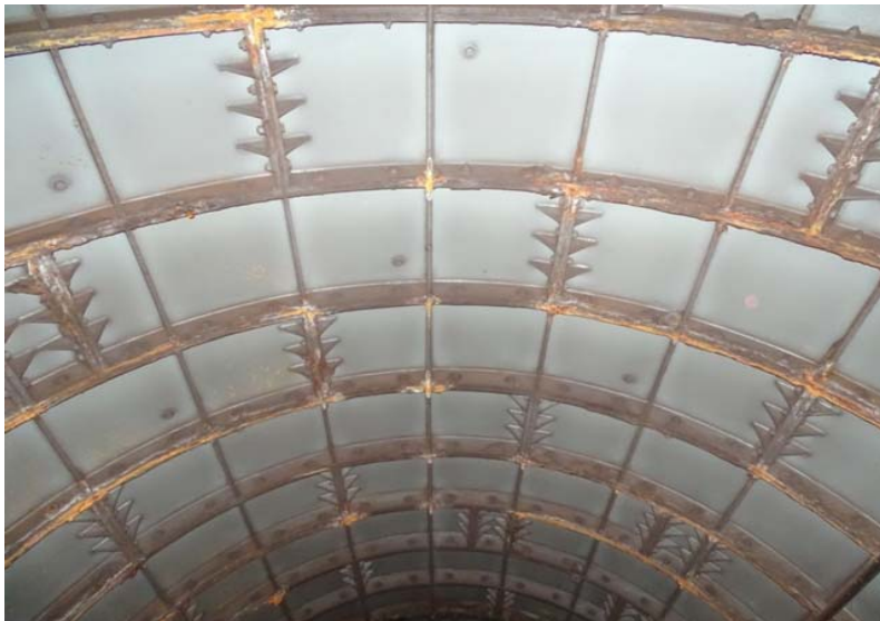
Photograph No. 27 Station 70+20, ceiling.
