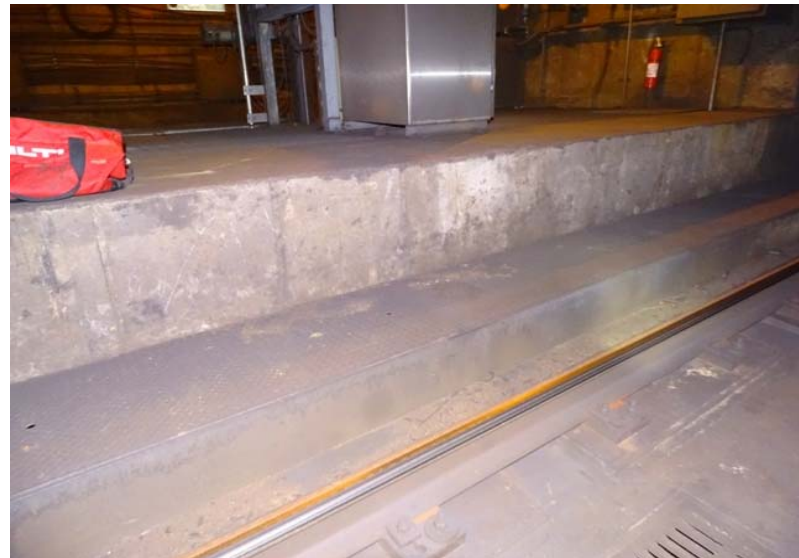
Photograph No. 56 Station 70+70, east wall.
