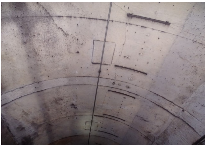
Photograph No. 447 Station 76+30, ceiling.
