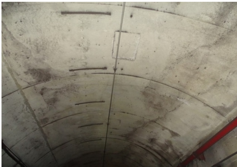
Photograph No. 365 Station 78+80, ceiling.
