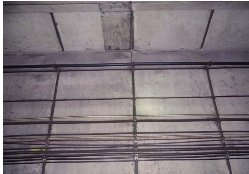
Photograph No. 212 Station 73+00, upper portion of west wall.
