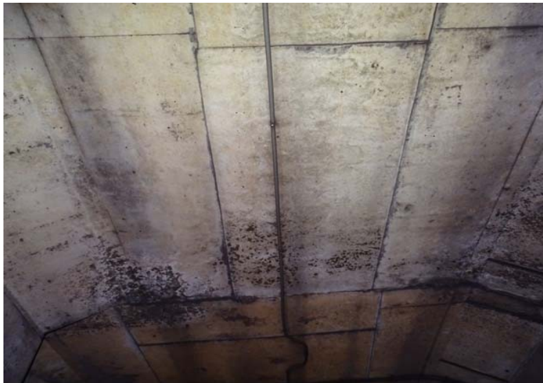
Photograph No. 121 Station 71+70, ceiling.
