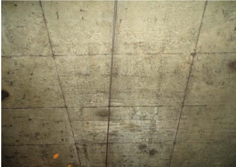
Photograph No. 45 Station 70+50, ceiling.
