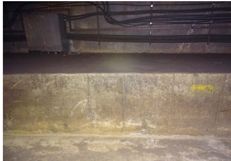
Photograph No. 48 Station 70+50, lower portion of west wall.
