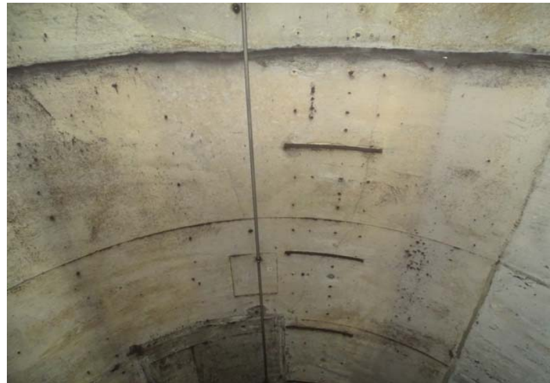
Photograph No. 312 Station 74+50, ceiling.
