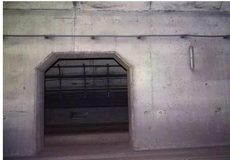
Photograph No. 340 Station 74+90, east wall.
