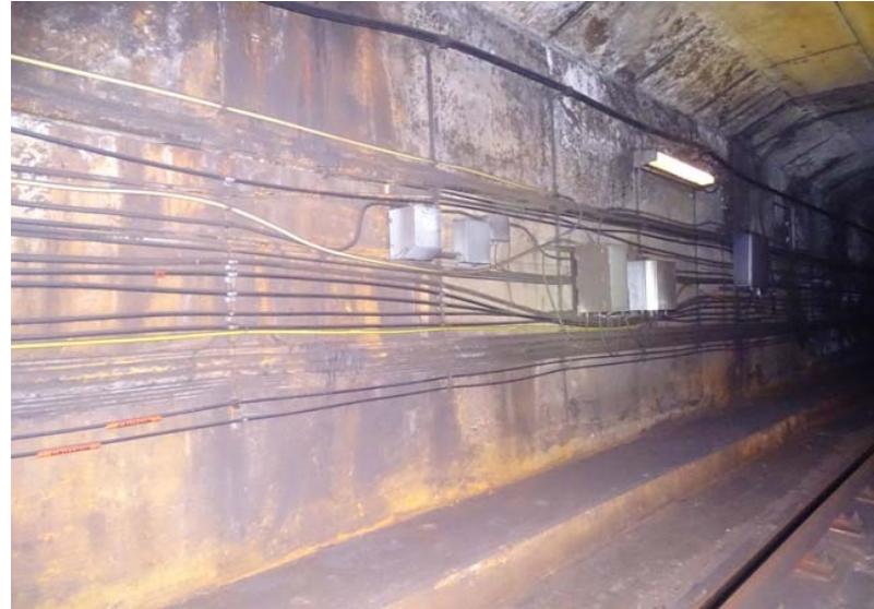
Photograph No. 38 Station 70+80, east wall.
