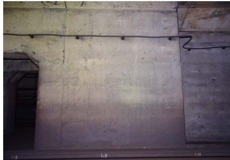
Photograph No. 120 Station 71+70, east wall.
