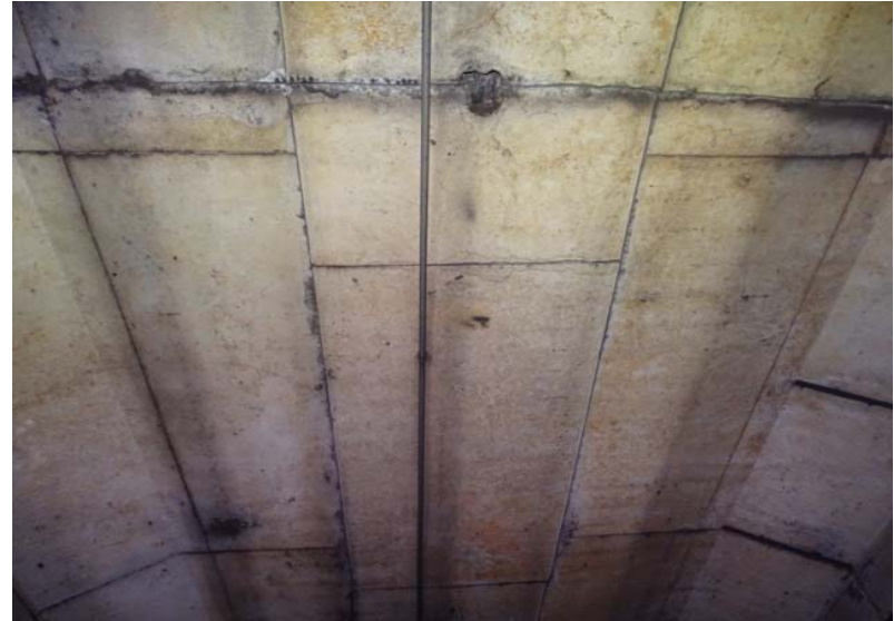
Photograph No. 94 Station 71+30, ceiling.
