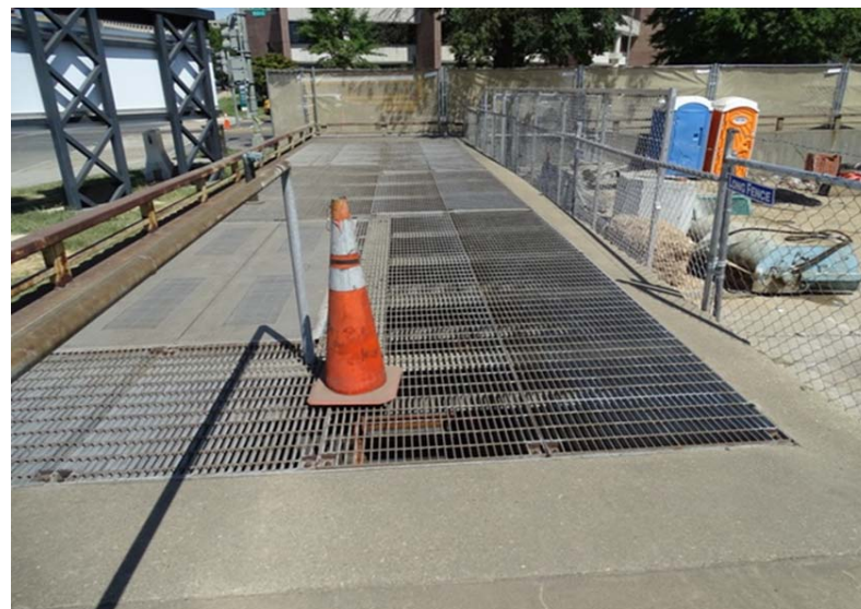
Photograph No. 192 Vent shaft exterior, looking northeast at deck.
