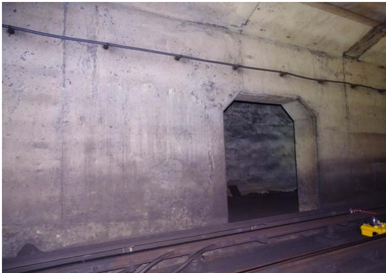
Photograph No. 79 Station 71+10, east wall.
