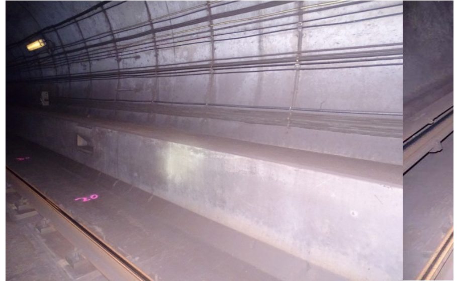
Photograph No. 434 Station 76+10, lower portion of west wall.
