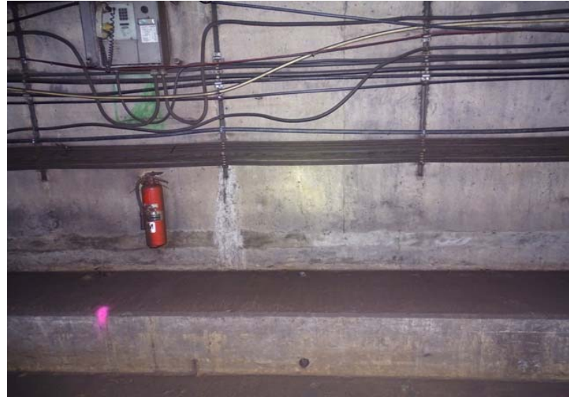
Photograph No. 222 Station 73+10, lower portion of west wall.
