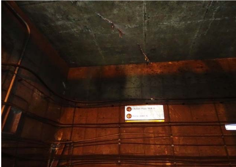
Photograph No. 65 Station 70+80, upper portion of west wall.
