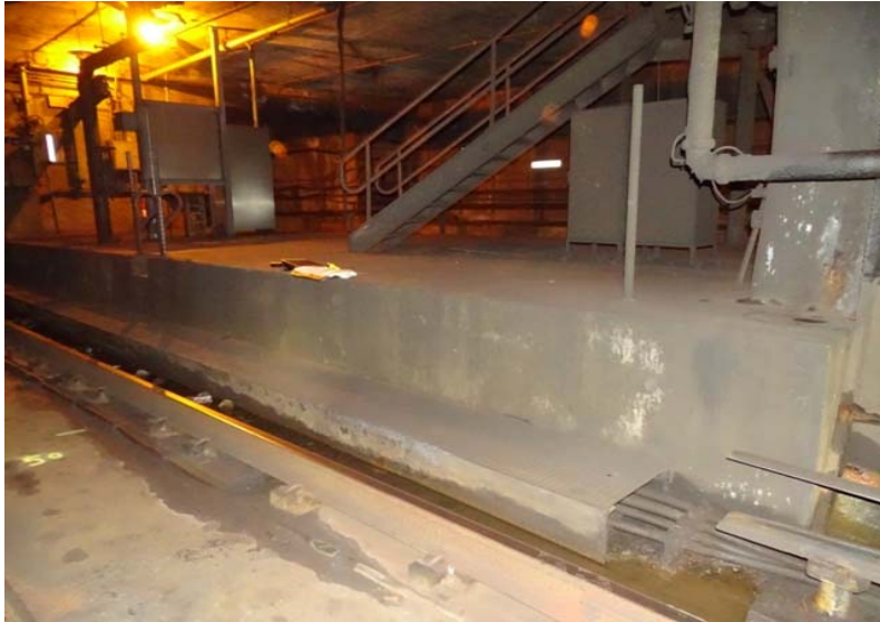
Photograph No. 33 Station 70+40, west wall.
