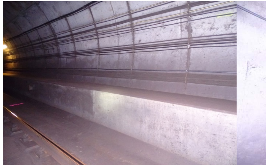
Photograph No. 480 Station 76+80, lower portion of west wall.
