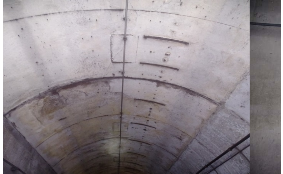
Photograph No. 374 Station 75+30, ceiling.
