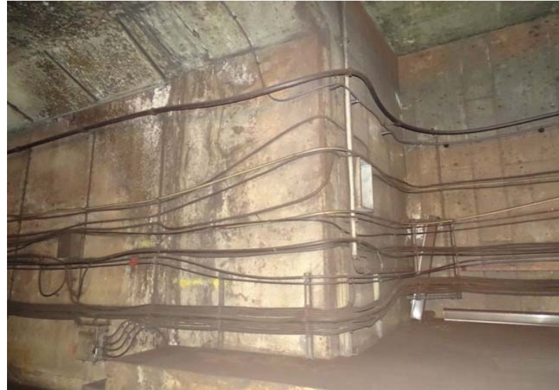
Photograph No. 70 Station 70+90, upper portion of west wall.
