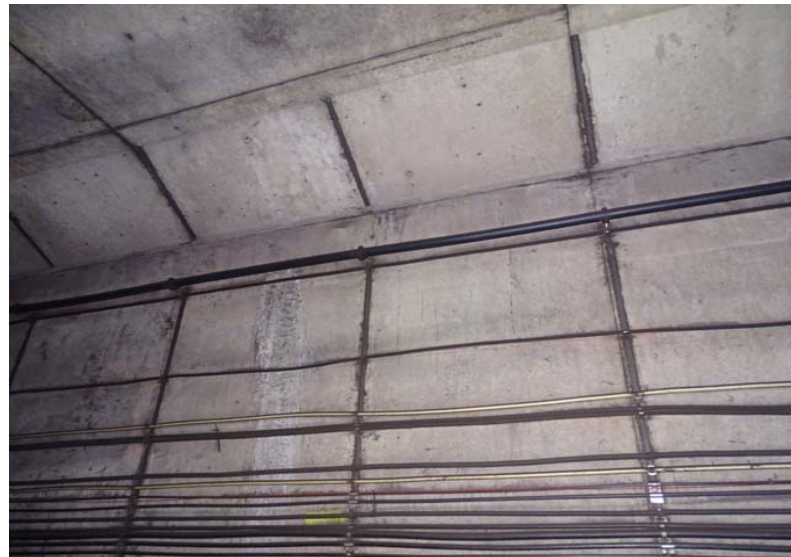
Photograph No. 266 Station 73+80, upper portion of west wall.
