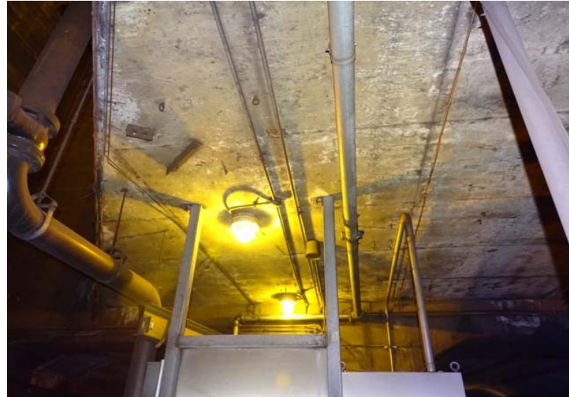
Photograph No. 38 Platform, ceiling, looking south.
