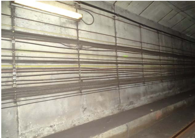
Photograph No. 101 Station 72+40, east wall.
