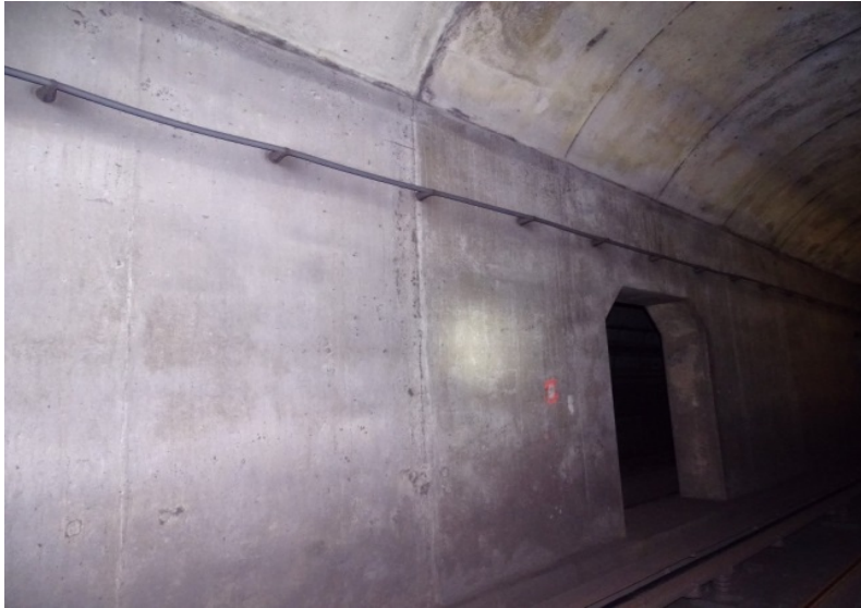
Photograph No. 373 Station 75+30, east wall.
