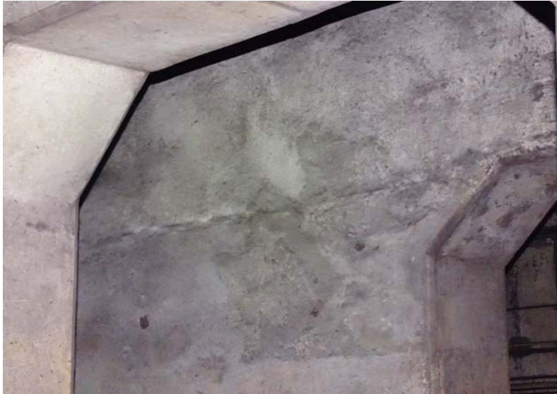
Photograph No. 29 Storage area, section 3, upper south portion.
