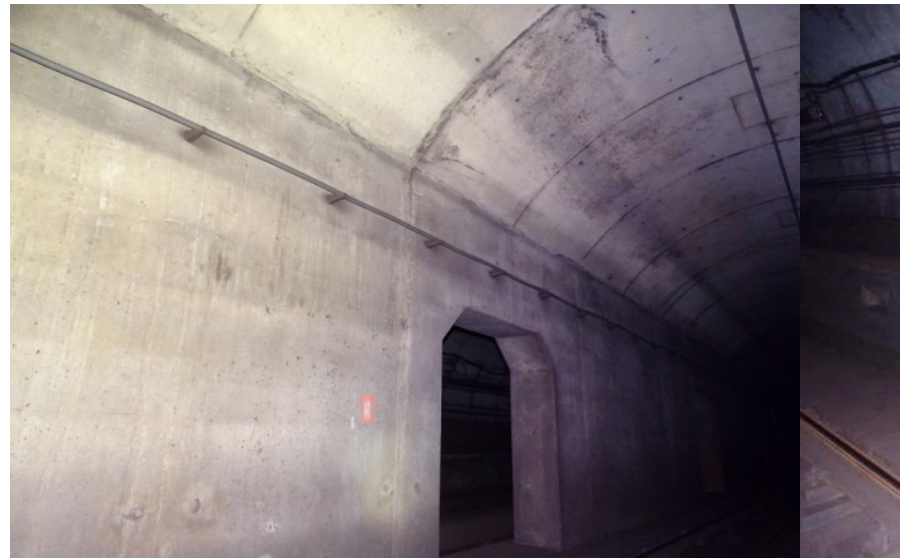
Photograph No. 508 Station 77+30, east wall.
