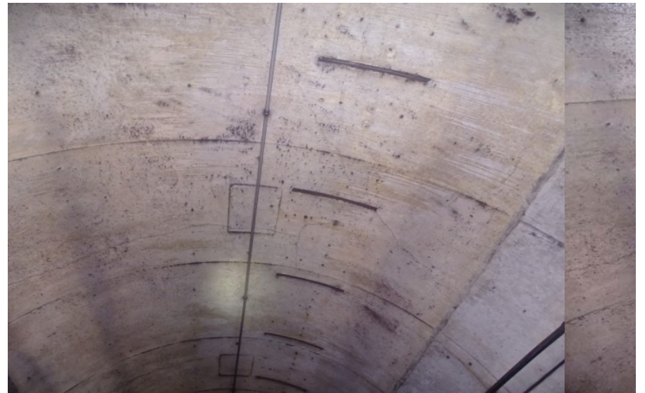
Photograph No. 408 Station 75+80, ceiling.
