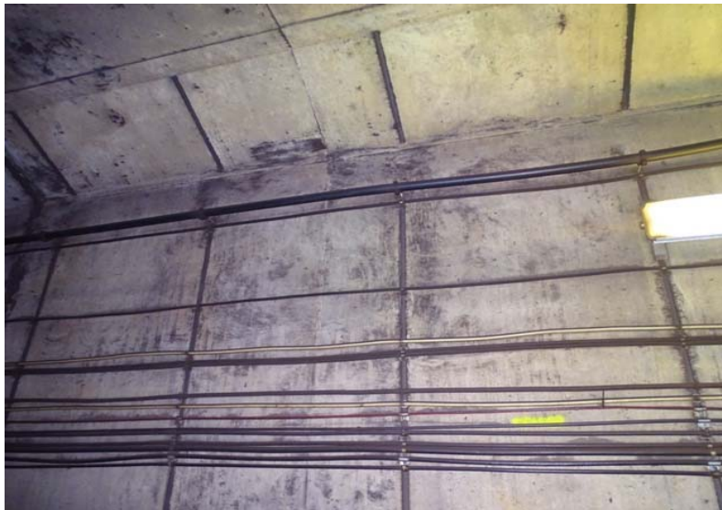
Photograph No. 255 Station 73+60, upper portion of west wall.
