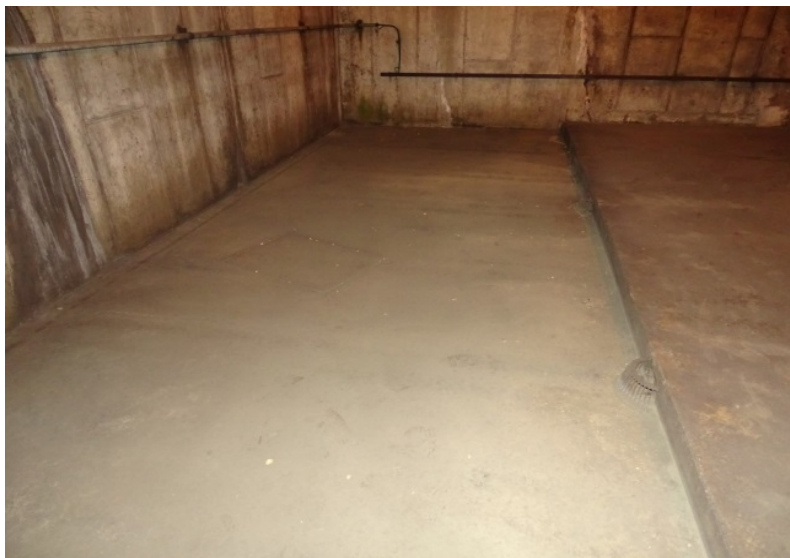
Photograph No. 173 Upper fan room floor, north section, west end.
