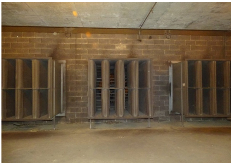
Photograph No. 149 Upper fan room, east wall, south-center section, lower portion.
