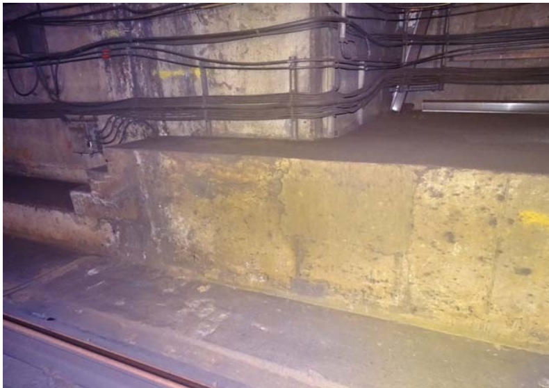
Photograph No. 71 Station 70+90, lower portion of west wall.
