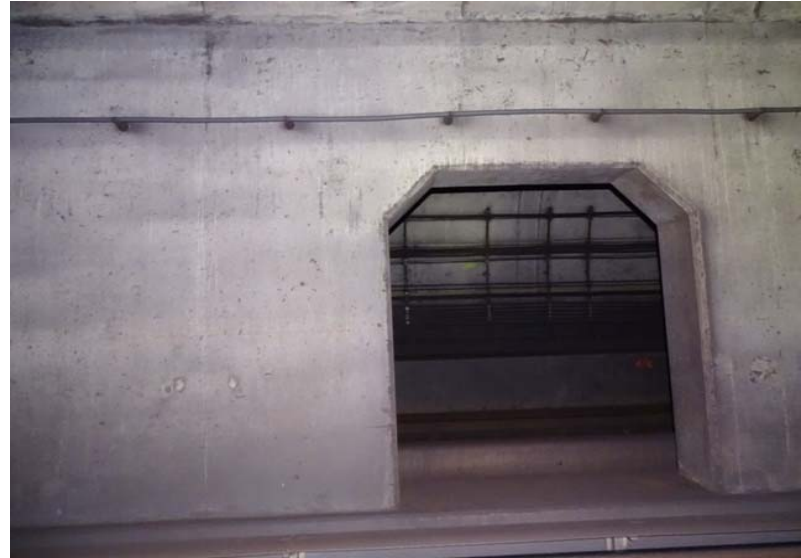
Photograph No. 318 Station 74+60, east wall.
