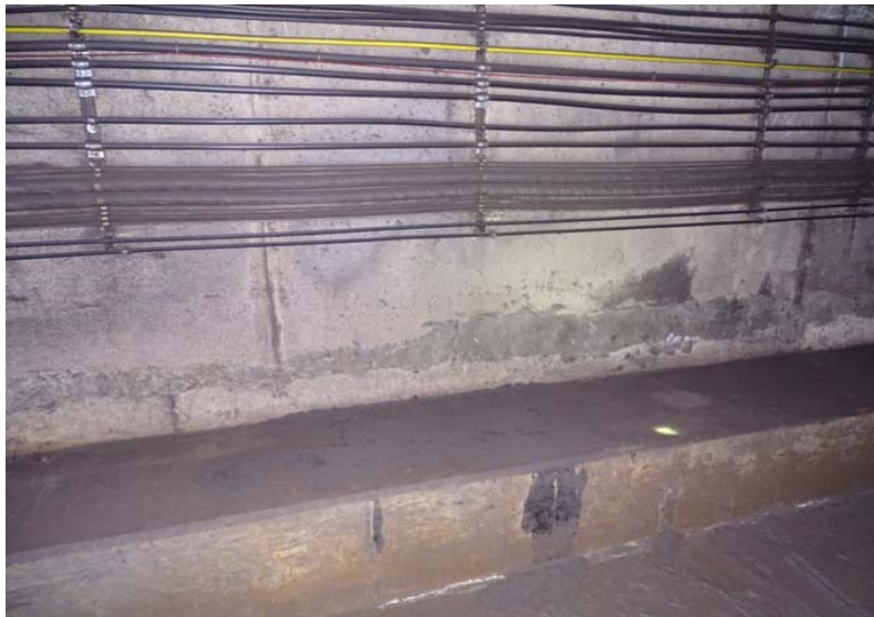
Photograph No. 131 Station 73+00 - previous concrete repair.
