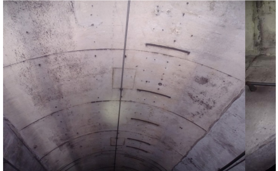
Photograph No. 514 Station 77+40, ceiling.
