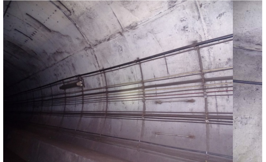
Photograph No. 554 Station 78+20, upper portion of west wall.
