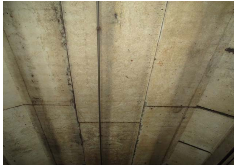
Photograph No. 102 Station 71+40, ceiling.
