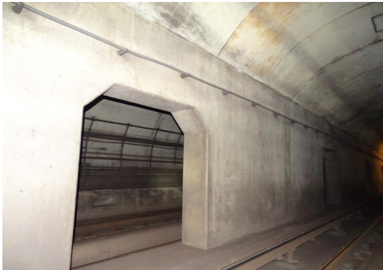
Photograph No. 451 Station 76+40, east wall.
