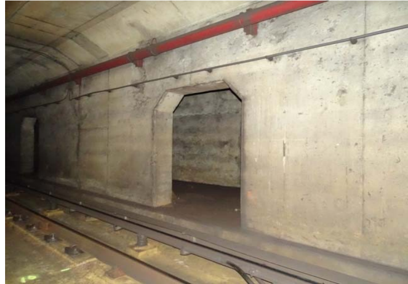
Photograph No. 46 Station 70+80, west wall.
