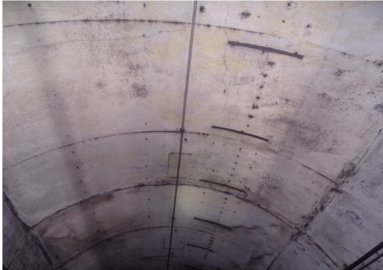
Photograph No. 553 Station 78+20, ceiling.
