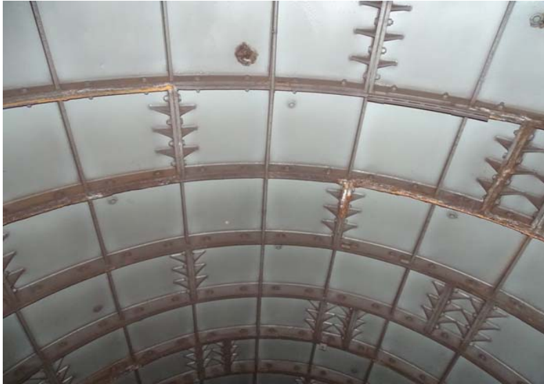
Photograph No. 17 Station 70+00, ceiling.
