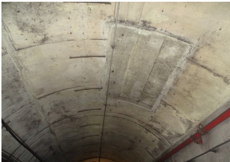
Photograph No. 337 Station 78+00, ceiling.
