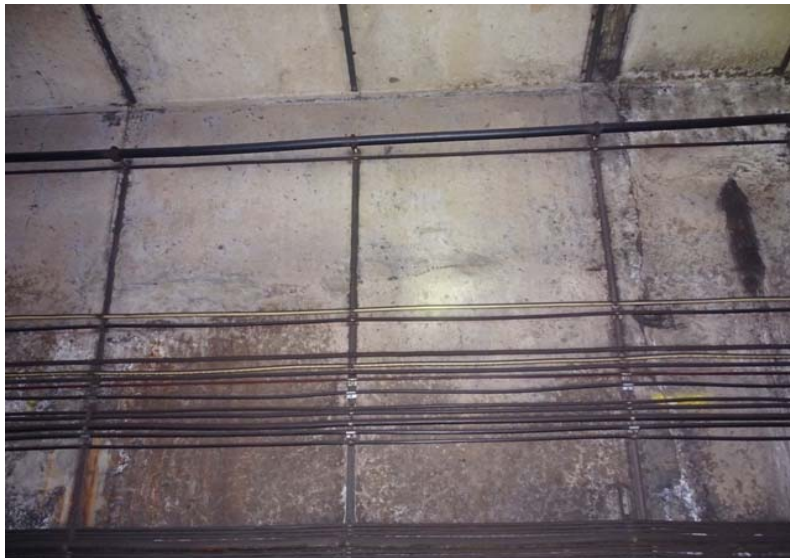
Photograph No. 95 Station 71+30, upper portion of west wall.
