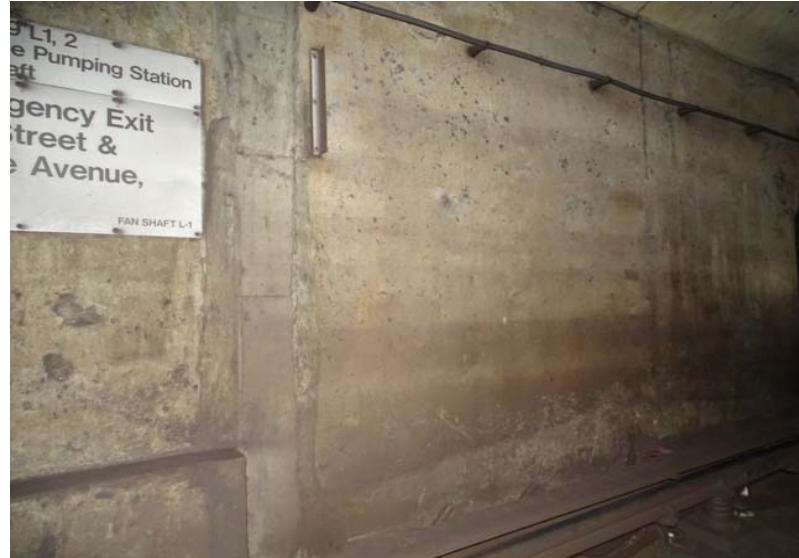
Photograph No. 74 Station 71+00, east wall.
