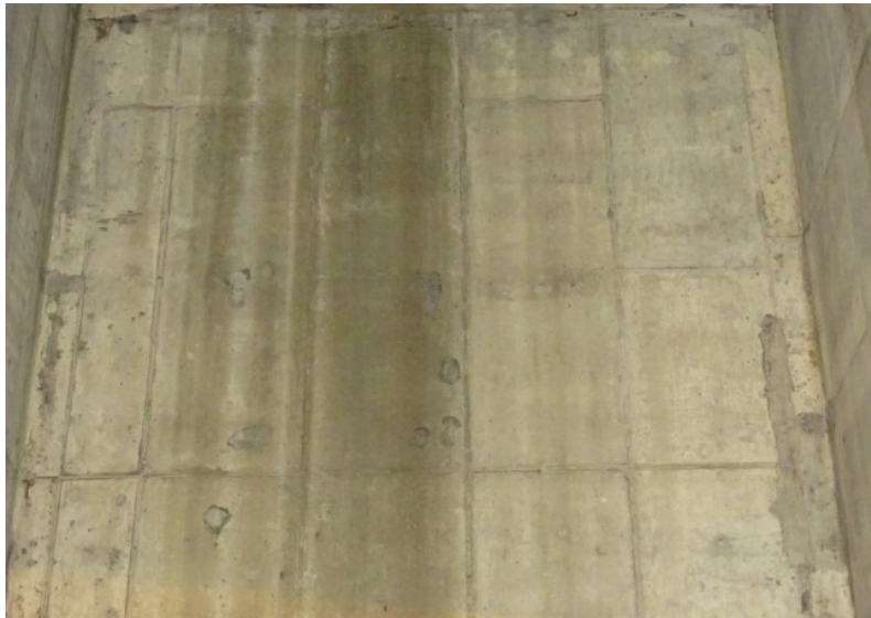
Photograph No. 133 Upper fan room, north wall, middle portion.
