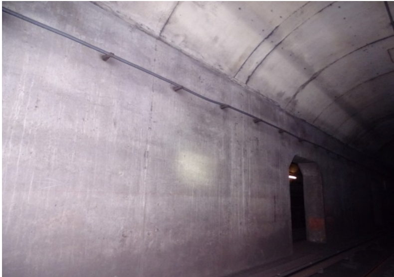
Photograph No. 519 Station 77+50, east wall.
