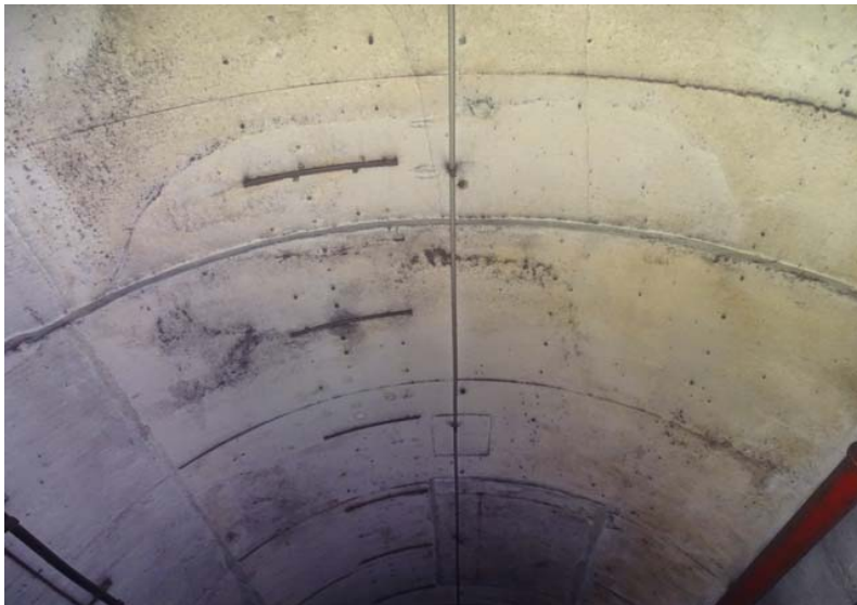
Photograph No. 183 Station 74+40, ceiling.
