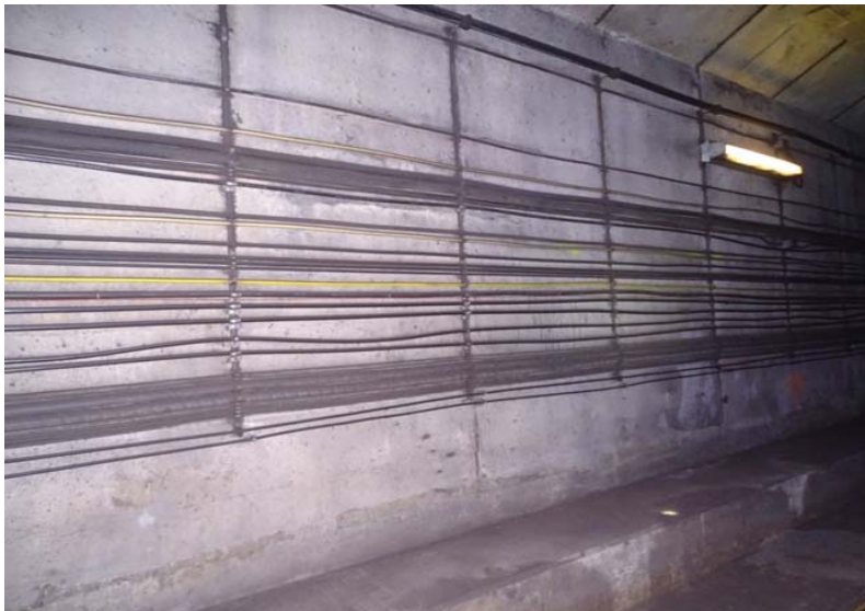
Photograph No. 163 Station 73+80, east wall.
