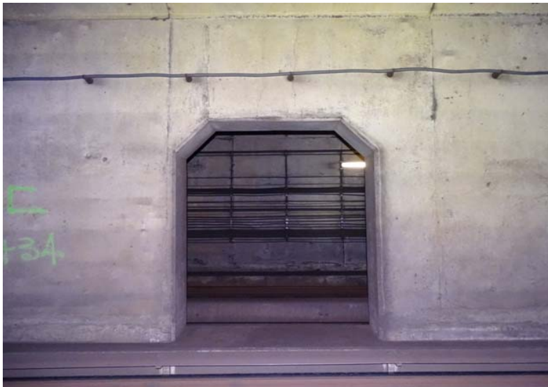
Photograph No. 171 Station 72+40, east wall.
