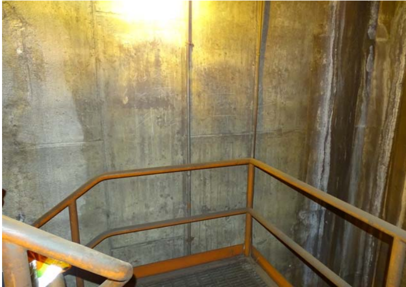
Photograph No. 77 Main room, northwest corner.
