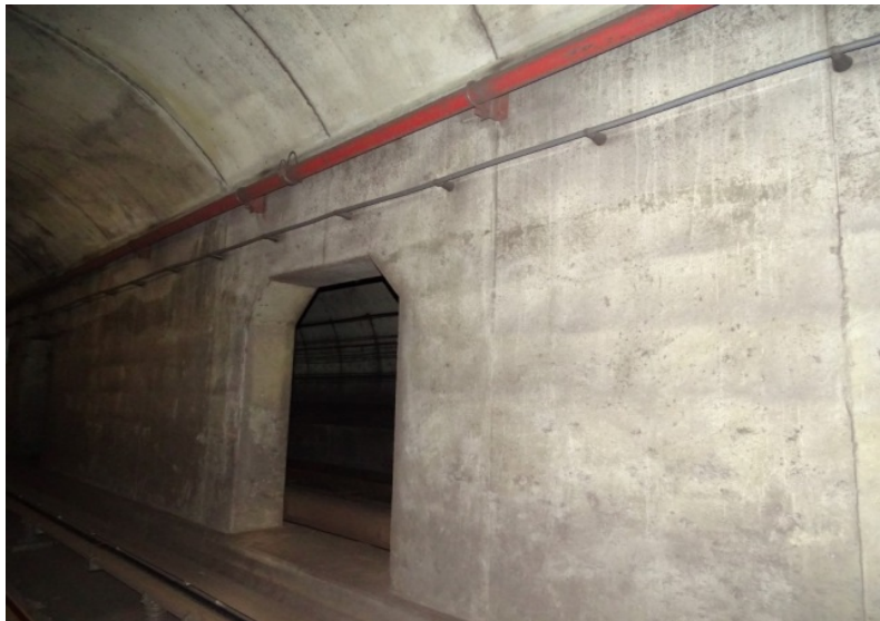
Photograph No. 359 Station 78+60, west wall.
