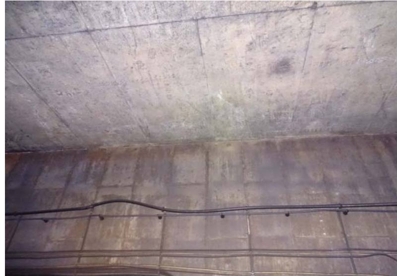
Photograph No. 46 Station 70+50, ceiling, west portion.
