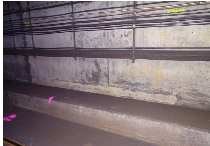
Photograph No. 256 Station 73+60, lower portion of west wall.
