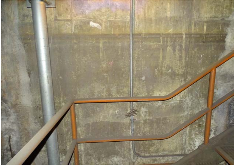
Photograph No. 81 Main room, west wall at the stair.
