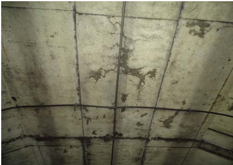
Photograph No. 199 Station 72+80, ceiling.
