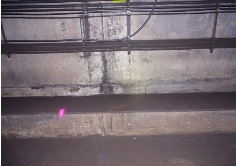
Photograph No. 201 Station 72+80, lower portion of west wall.
