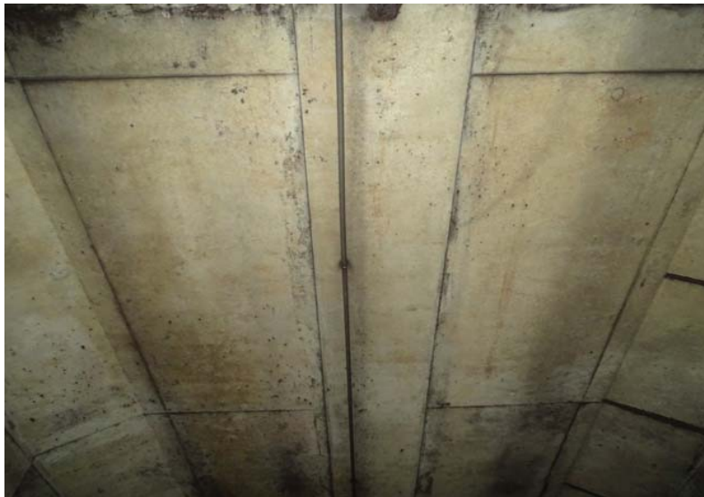
Photograph No. 235 Station 73+30, ceiling.
