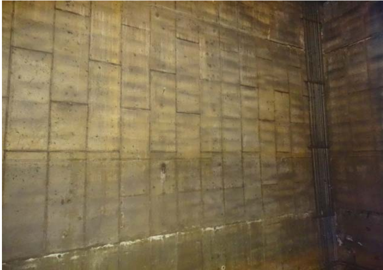
Photograph No. 69 Main room, east wall, upper south portion.
