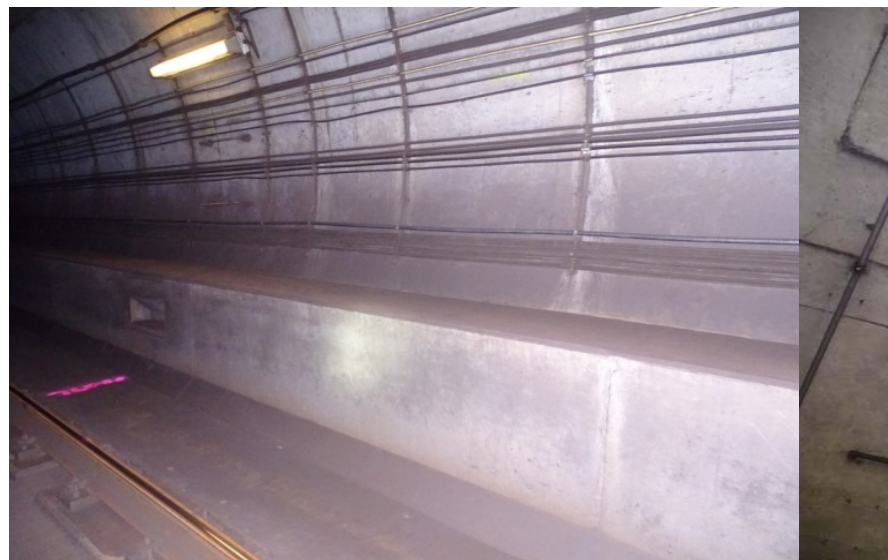
Photograph No. 416 Station 75+90, lower portion of west wall.
