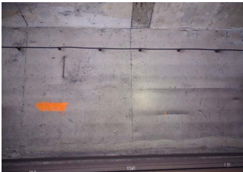
Photograph No. 139 Station 72+00, east wall.
