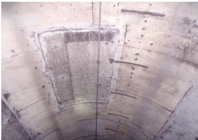
Photograph No. 547 Station 78+00, ceiling.
