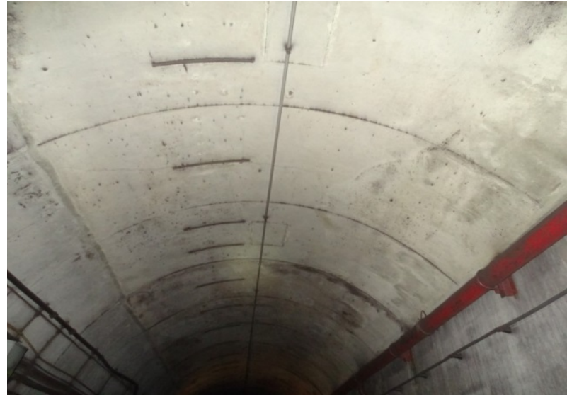
Photograph No. 214 Station 75+20, ceiling.
