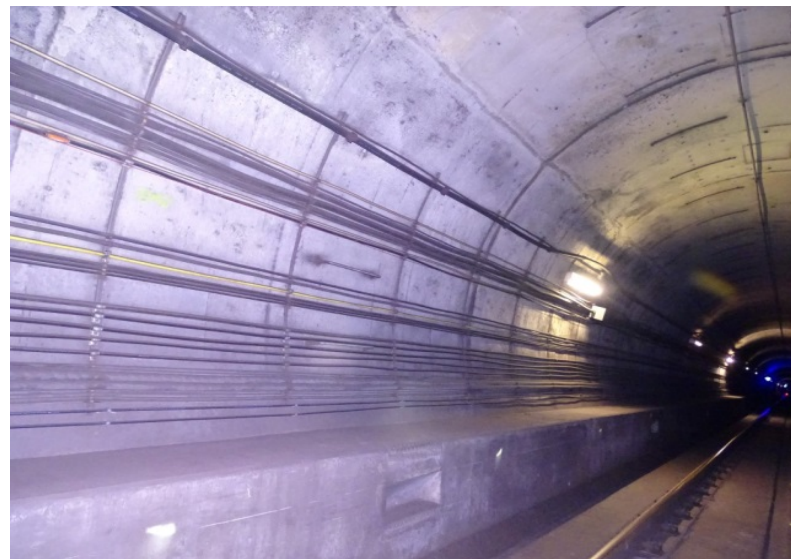
Photograph No. 342 Station 78+20, east wall.
