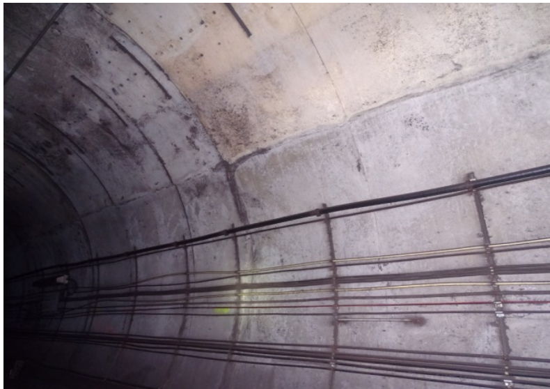
Photograph No. 535 Station 77+70, upper portion of west wall.
