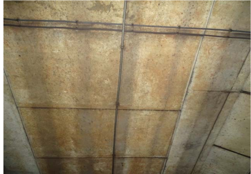
Photograph No. 134 Station 71+90, ceiling.
