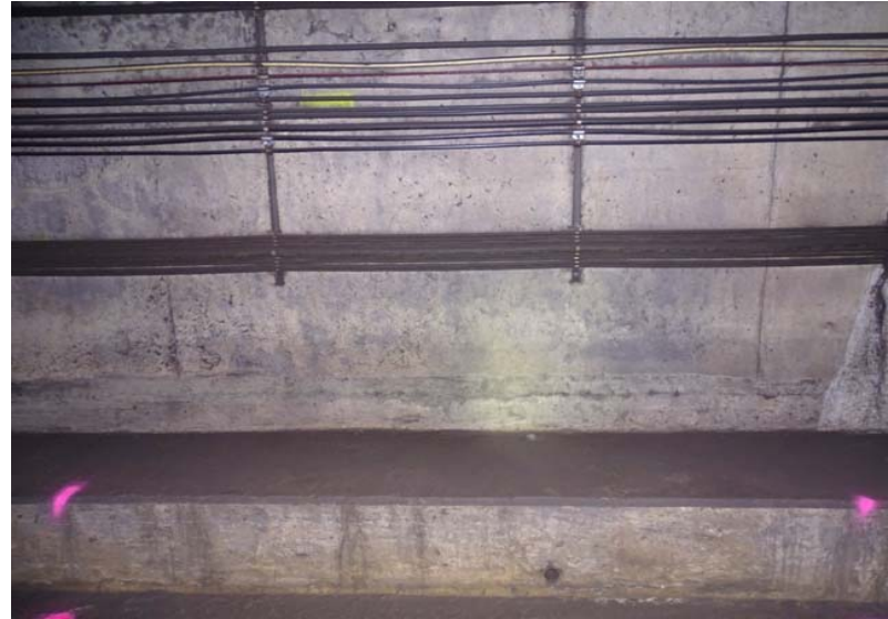
Photograph No. 194 Station 72+70, lower portion of west wall.
