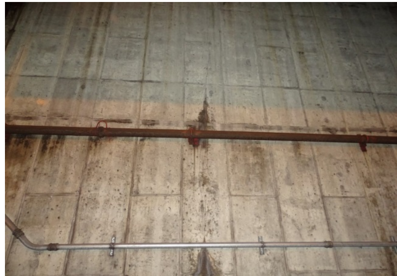
Photograph No. 168 Upper fan room, west wall, middle-south section, middle portion.
