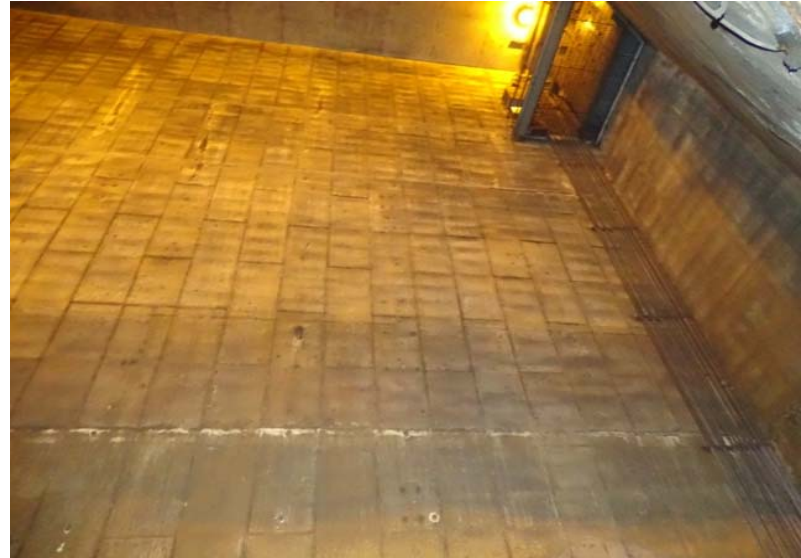
Photograph No. 62 Main room, looking up at east wall.
