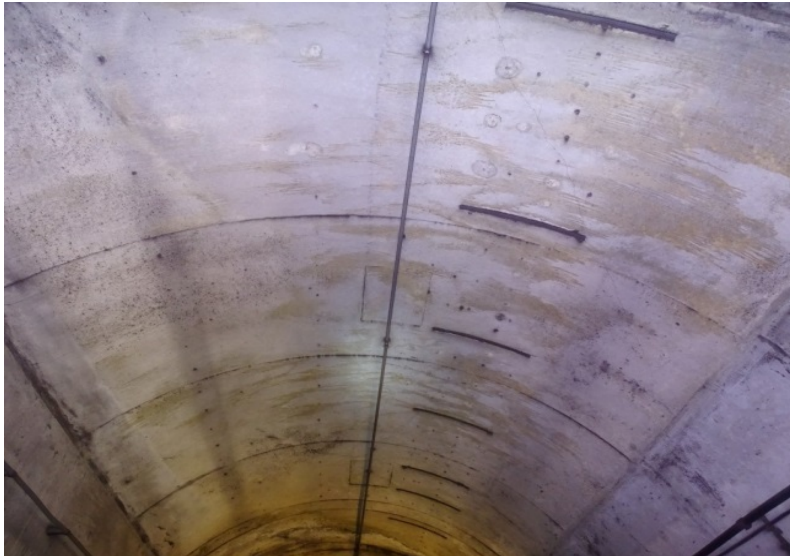
Photograph No. 491 Station 77+00, ceiling.
