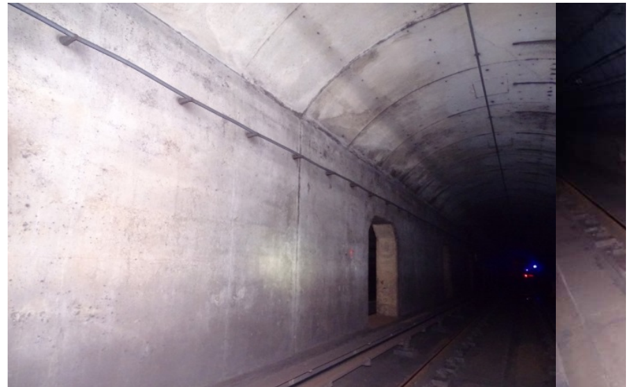
Photograph No. 552 Station 78+20, east wall.
