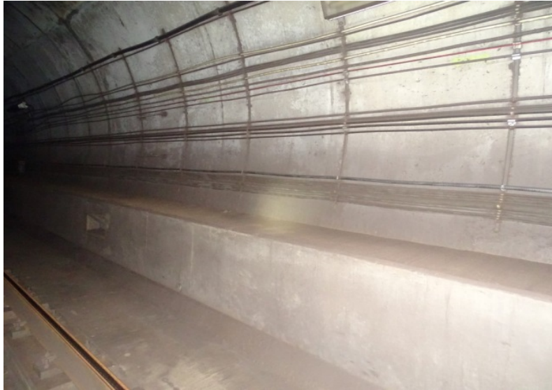
Photograph No. 529 Station 77+60, lower portion of west wall.
