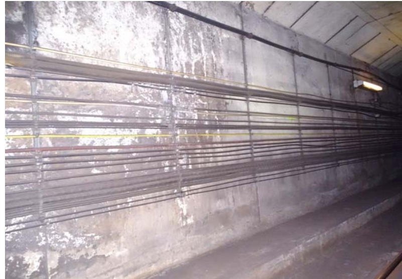
Photograph No. 56 Station 71+40, east wall.
