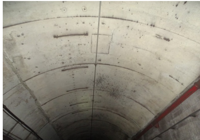
Photograph No. 256 Station 76+20, ceiling.
