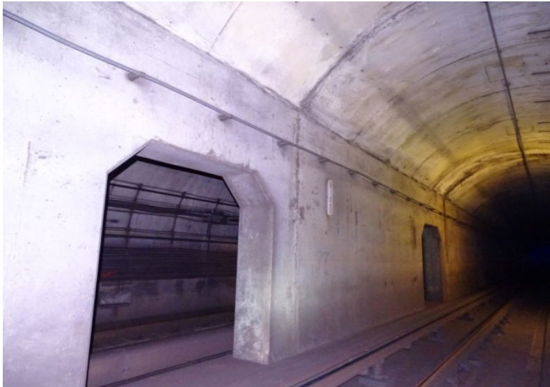
Photograph No. 483 Station 76+90, east wall.
