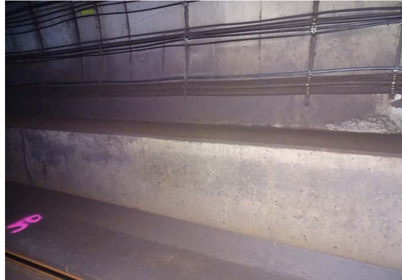
Photograph No. 306 Station 74+40, lower portion of west wall.
