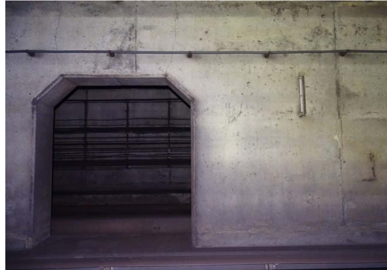
Photograph No. 270 Station 73+90, east wall.
