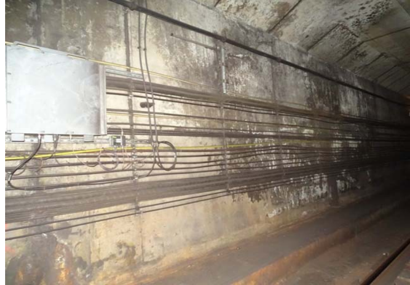
Photograph No. 50 Station 71+20, east wall.
