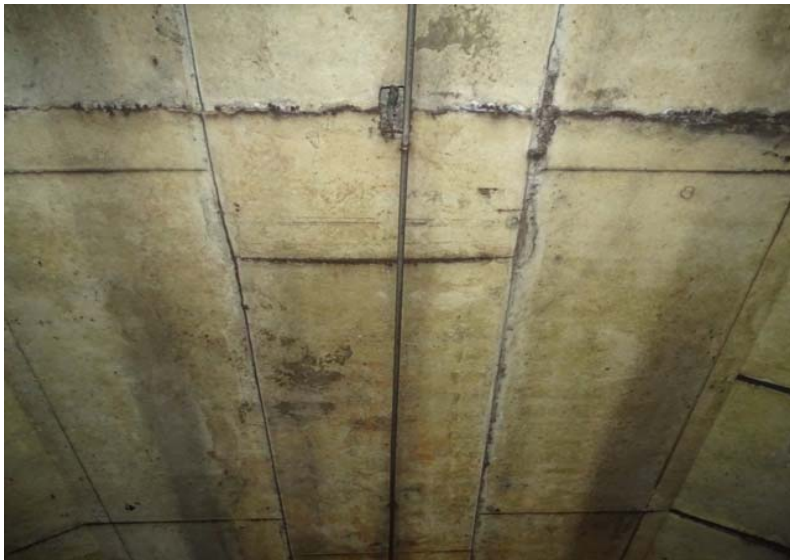
Photograph No. 167 Station 72+30, ceiling.
