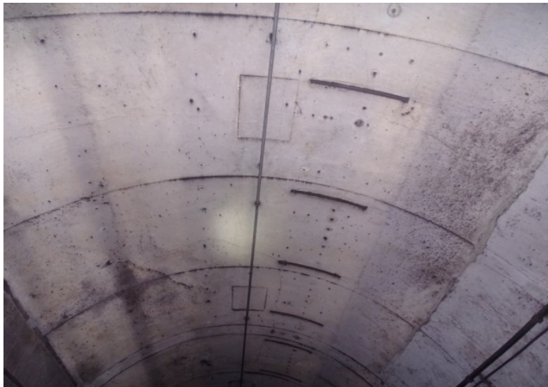
Photograph No. 439 Station 76+20, ceiling.
