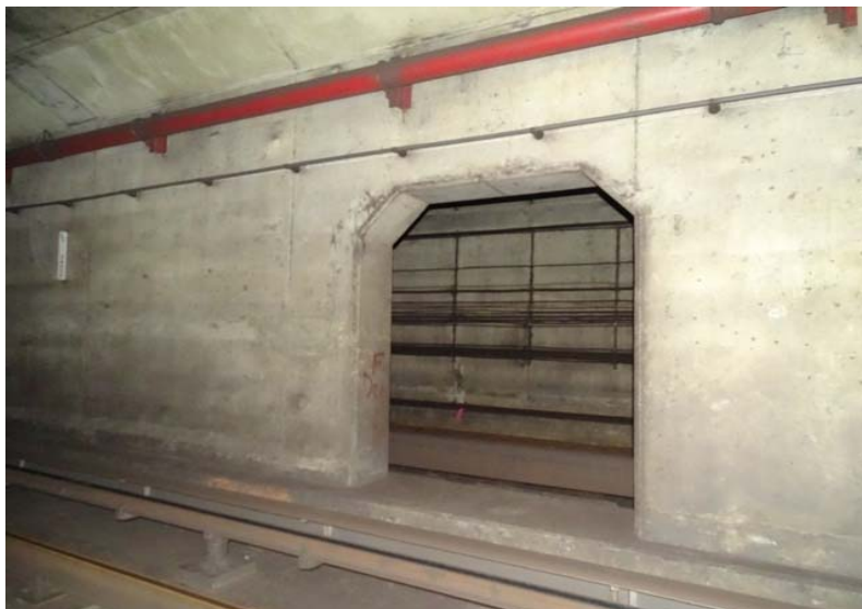
Photograph No. 125 Station 72+80, west wall.
