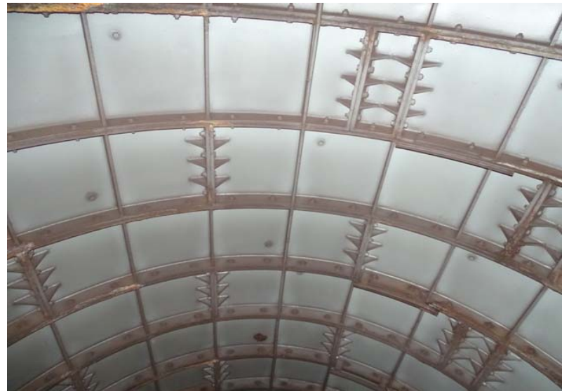
Photograph No. 12 Station 69+90, ceiling.
