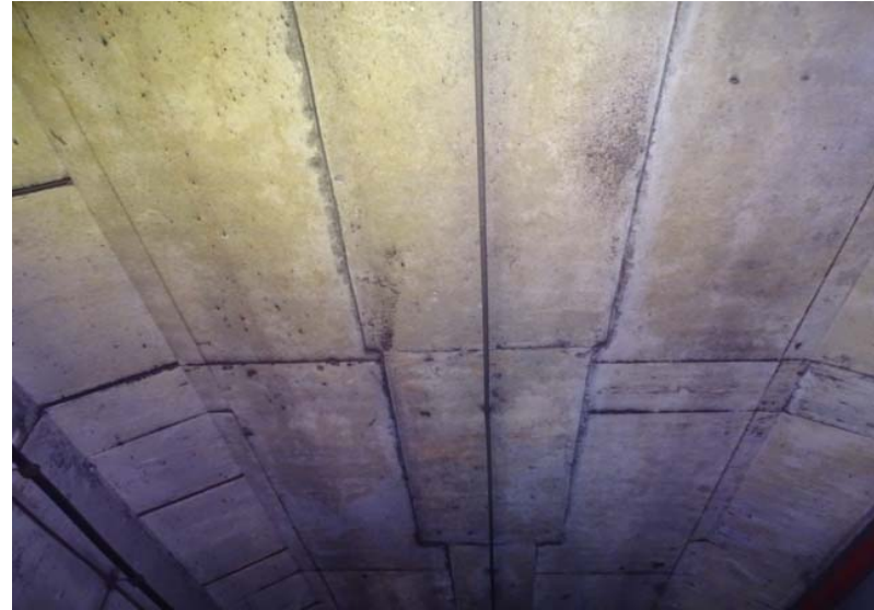
Photograph No. 106 Station 72+40, ceiling.
