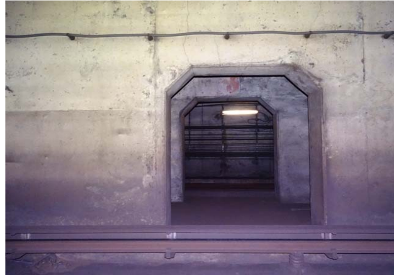
Photograph No. 114 Station 71+60, east wall.
