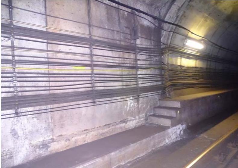
Photograph No. 173 Station 74+20, east wall.
