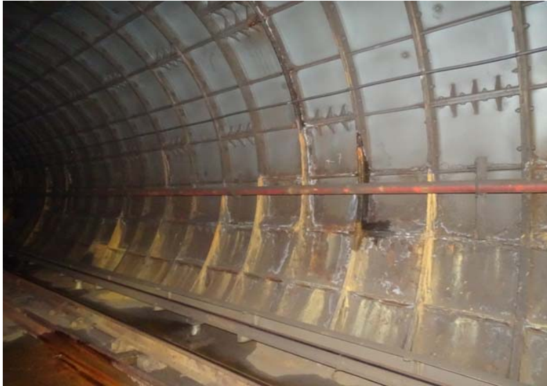
Photograph No. 5 Station 69+60, west wall.
