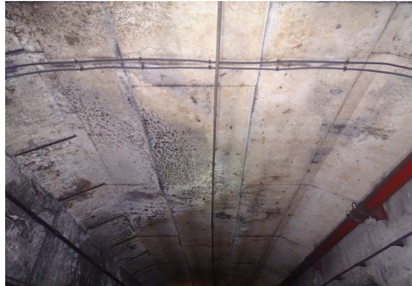
Photograph No. 52 Station 71+20, ceiling.
