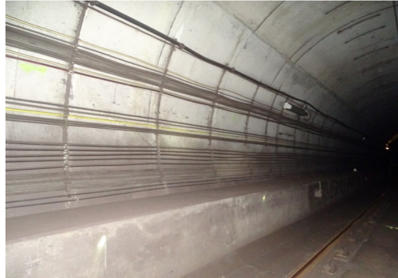
Photograph No. 238 Station 75+80, east wall.
