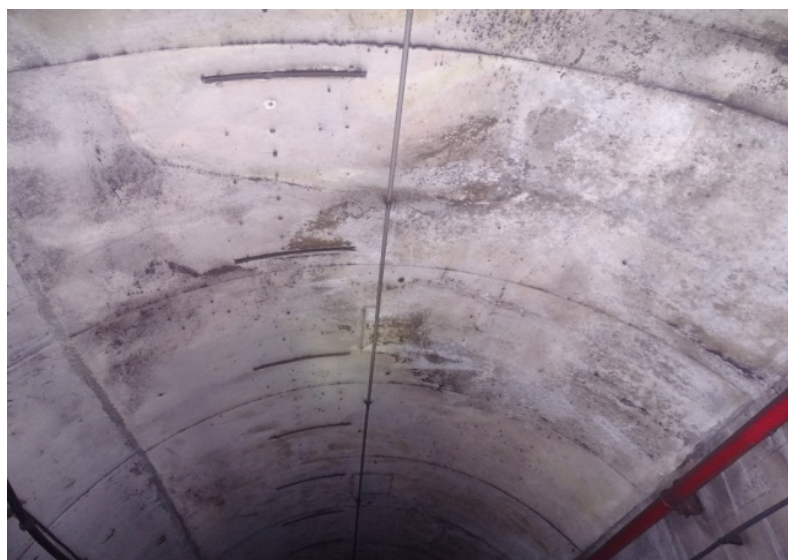
Photograph No. 308 Station 77+20, ceiling.
