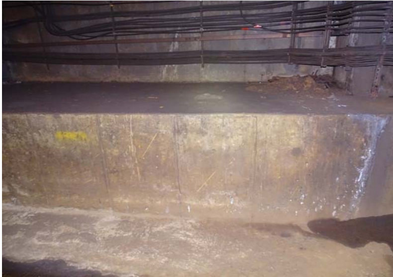
Photograph No. 41 Station 70+40, west catwalk.
