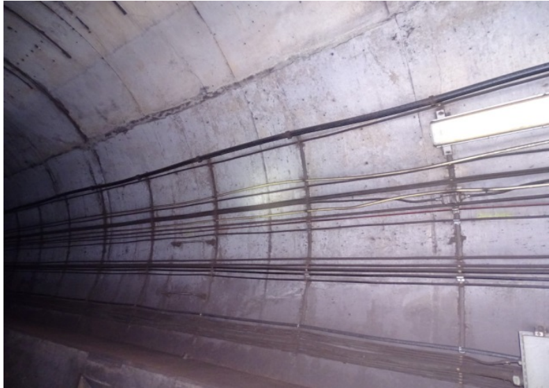
Photograph No. 453 Station 76+40, upper portion of west wall.
