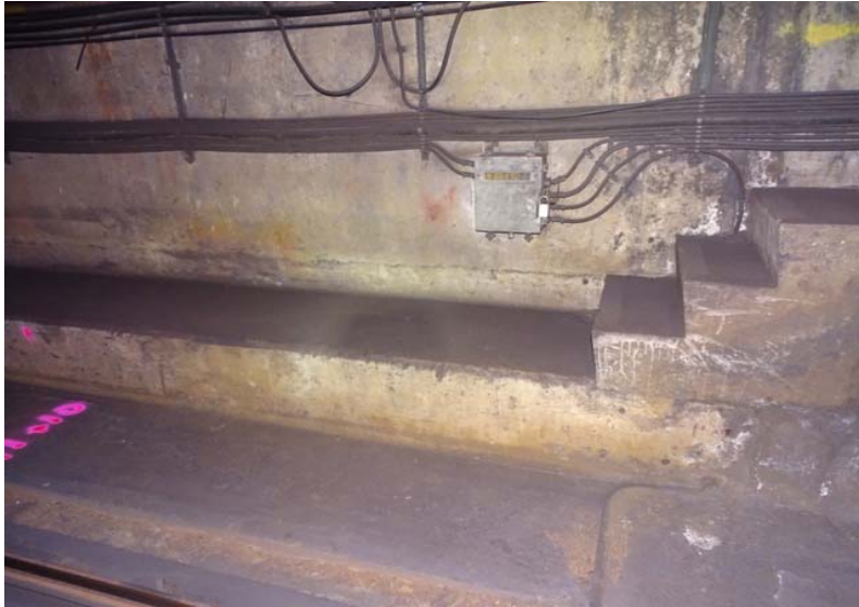
Photograph No. 77 Station 71+00, lower portion of west wall.
