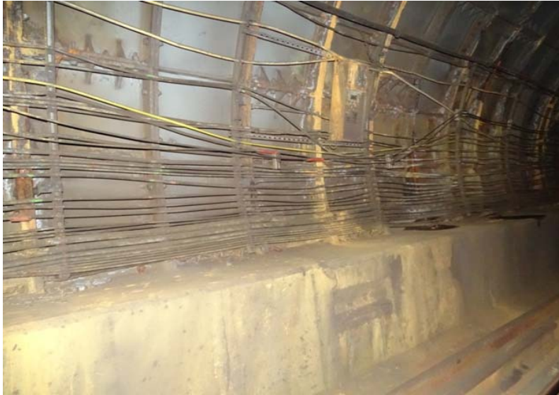
Photograph No. 17 Station 70+00, east wall.
