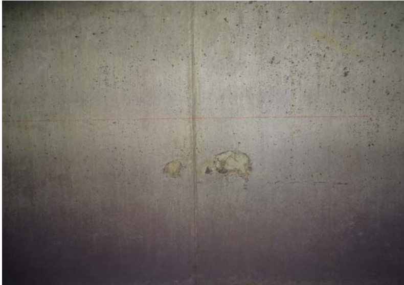
Photograph No. 333 Station 74+80 - previous concrete repair on east wall.
