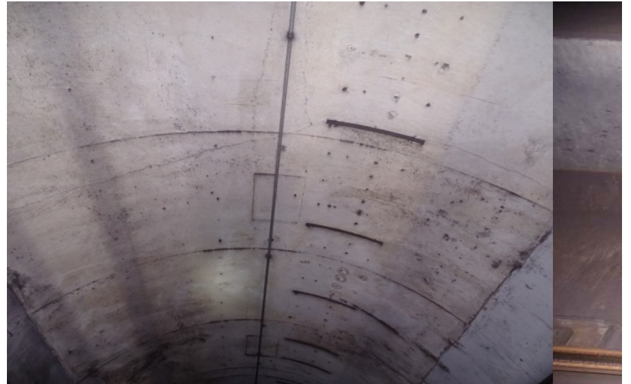
Photograph No. 464 Station 76+60, ceiling.
