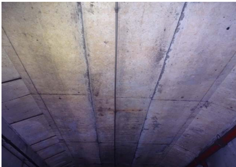
Photograph No. 87 Station 72+00, ceiling.
