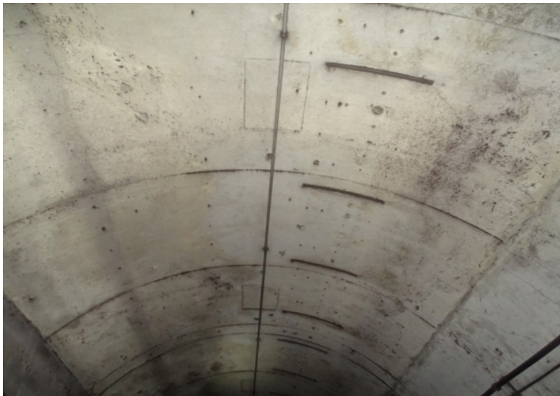
Photograph No. 351 Station 75+00, ceiling.
