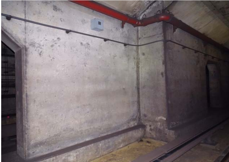
Photograph No. 69 Station 71+60, west wall, looking north.
