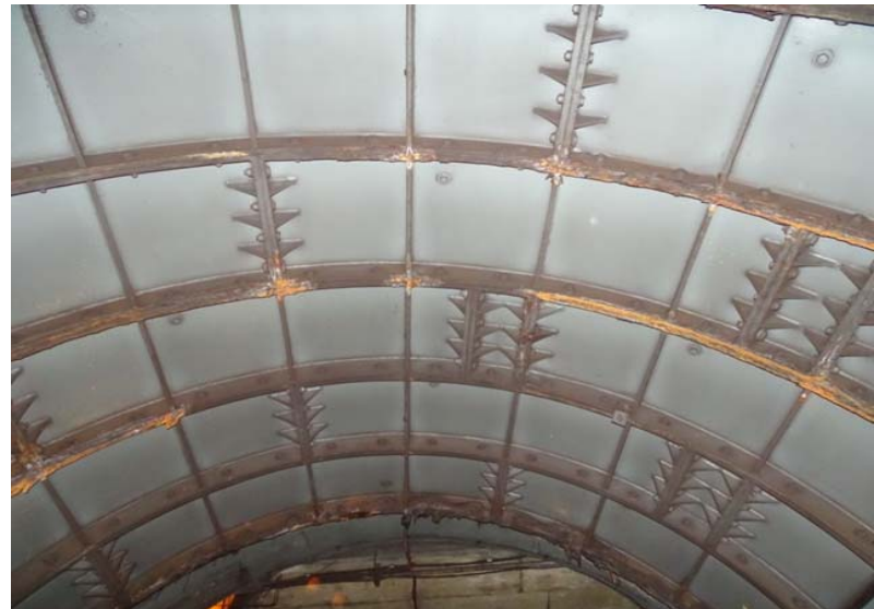
Photograph No. 32 Station 70+30, ceiling.
