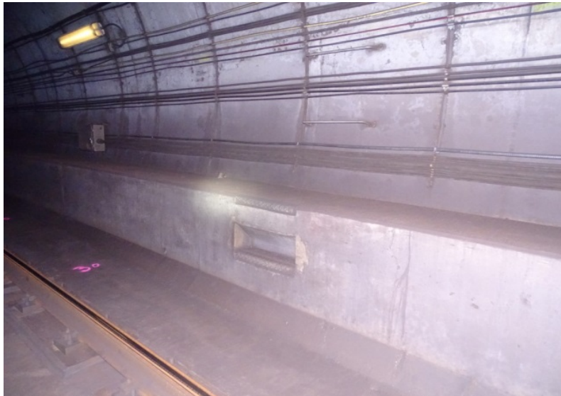
Photograph No. 441 Station 76+20, lower portion of west wall.
