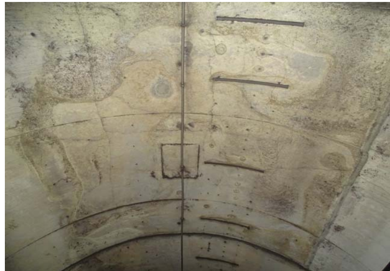
Photograph No. 304 Station 74+40, ceiling.
