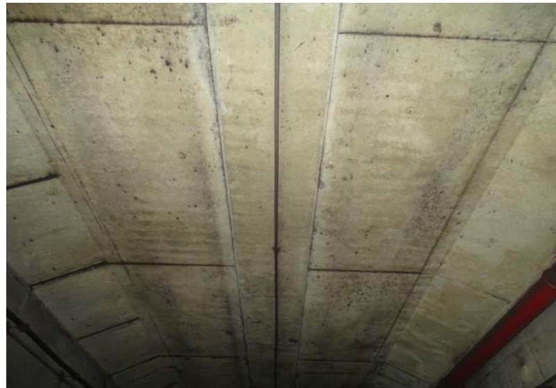
Photograph No. 124 Station 72+80, ceiling.
