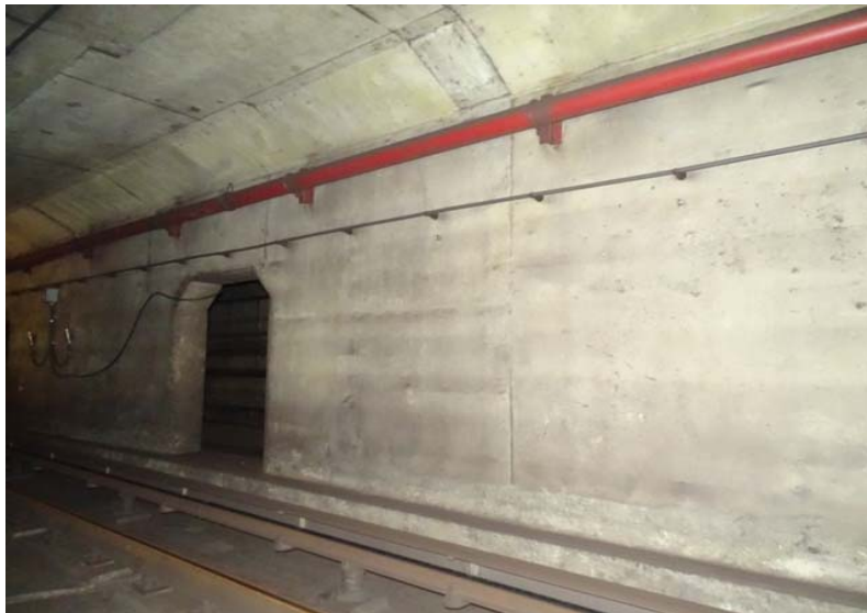
Photograph No. 107 Station 72+40, west wall.
