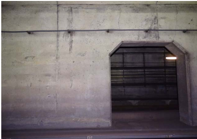
Photograph No. 263 Station 73+80, east wall.
