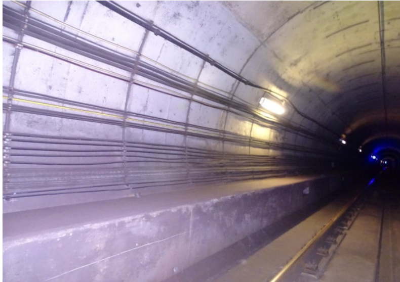
Photograph No. 373 Station 79+00, east wall.
