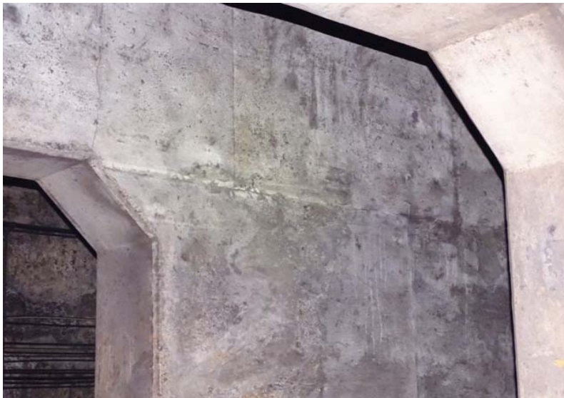
Photograph No. 23 Storage area, section 3, upper north portion.
