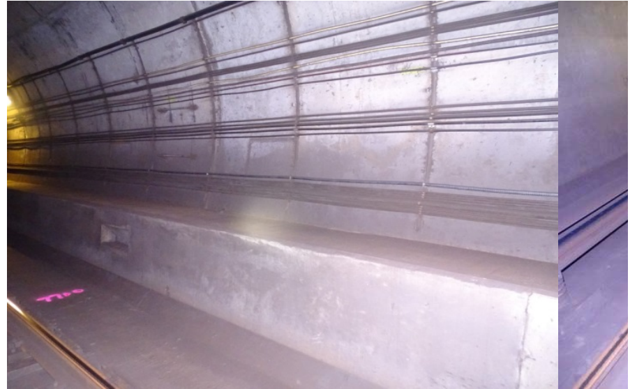
Photograph No. 486 Station 76+90, lower portion of west wall.
