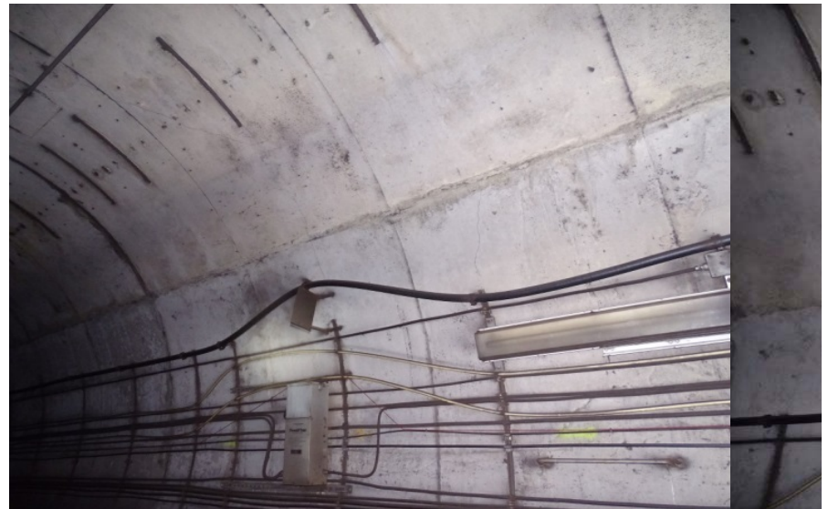
Photograph No. 368 Station 75+20, upper portion of west wall.
