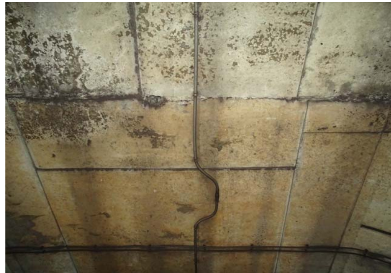
Photograph No. 128 Station 71+80, ceiling.
