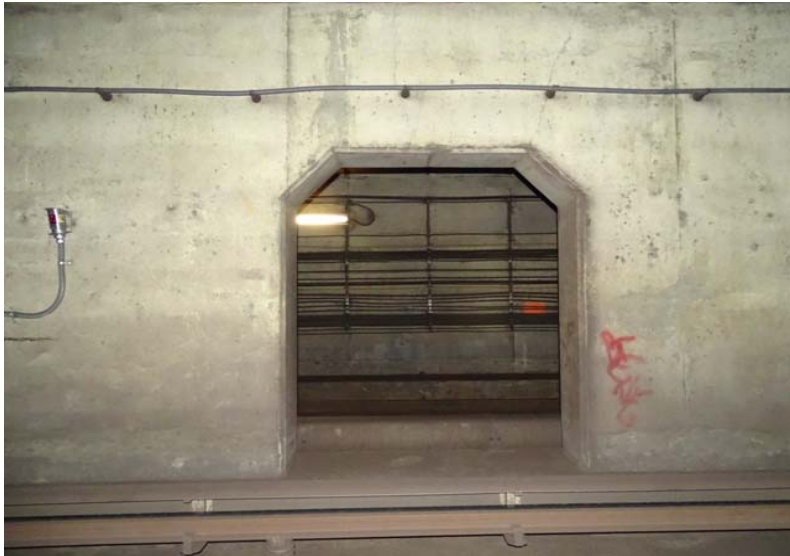
Photograph No. 203 Station 72+90, east wall.
