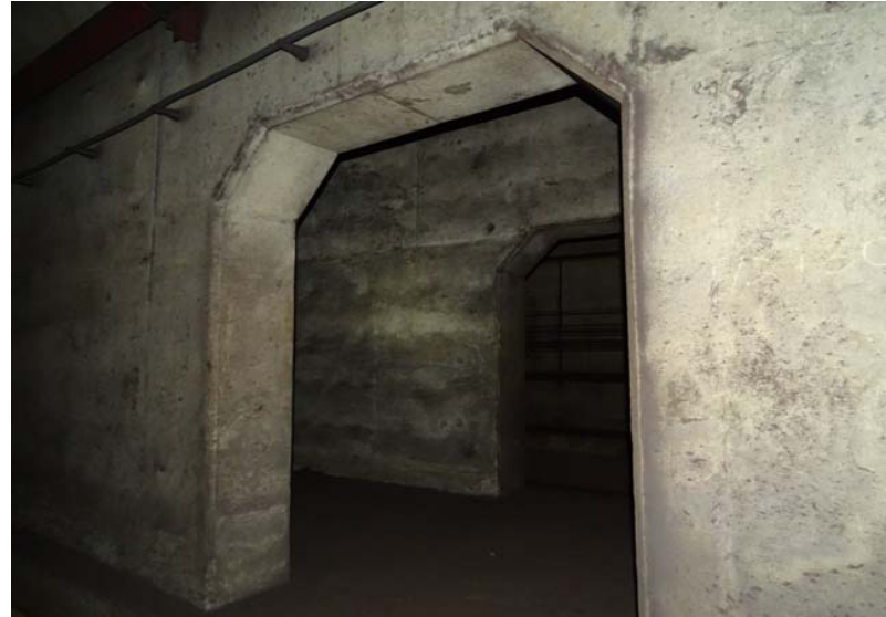
Photograph No. 18 Storage area, section 2, looking south.
