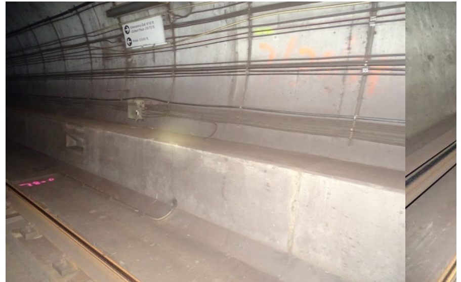
Photograph No. 542 Station 77+80, lower portion of west wall.
