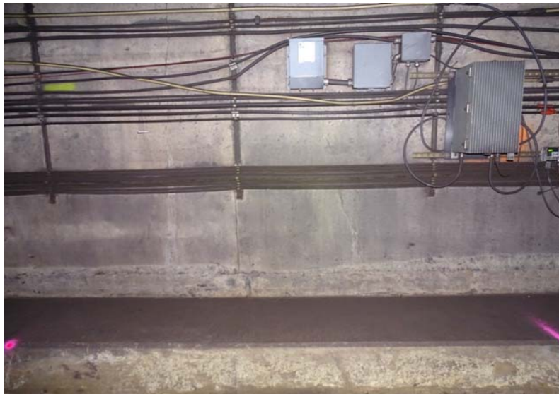
Photograph No. 143 Station 72+00, lower portion of west wall.
