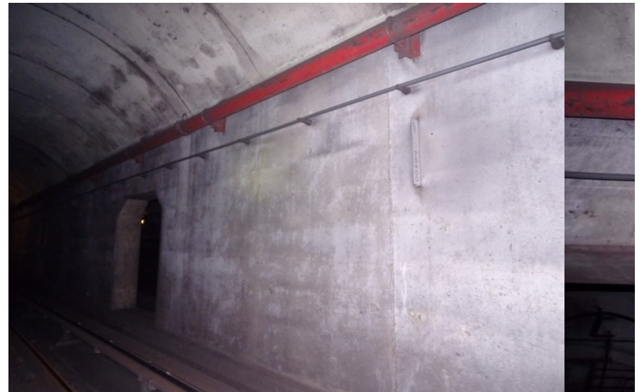
Photograph No. 208 Station 75+00, west wall.
