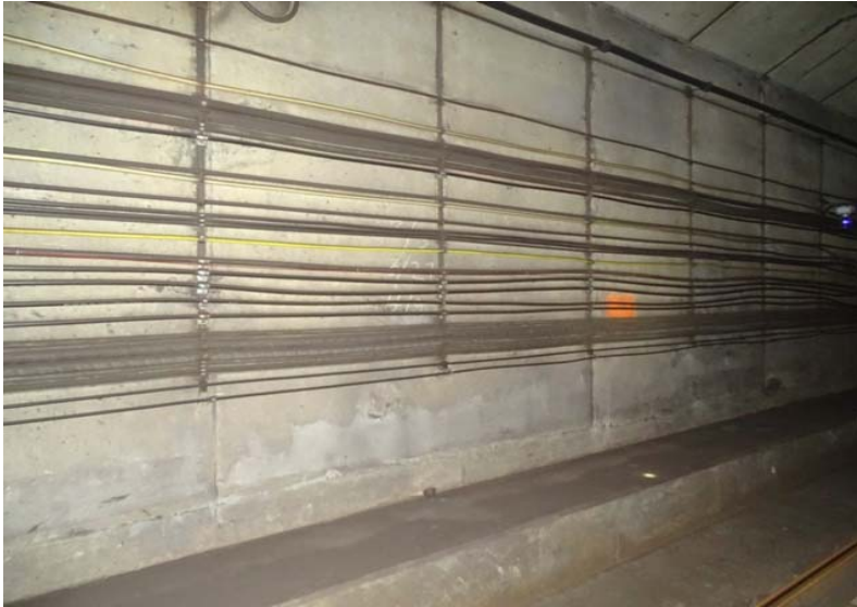
Photograph No. 121 Station 72+80, east wall.
