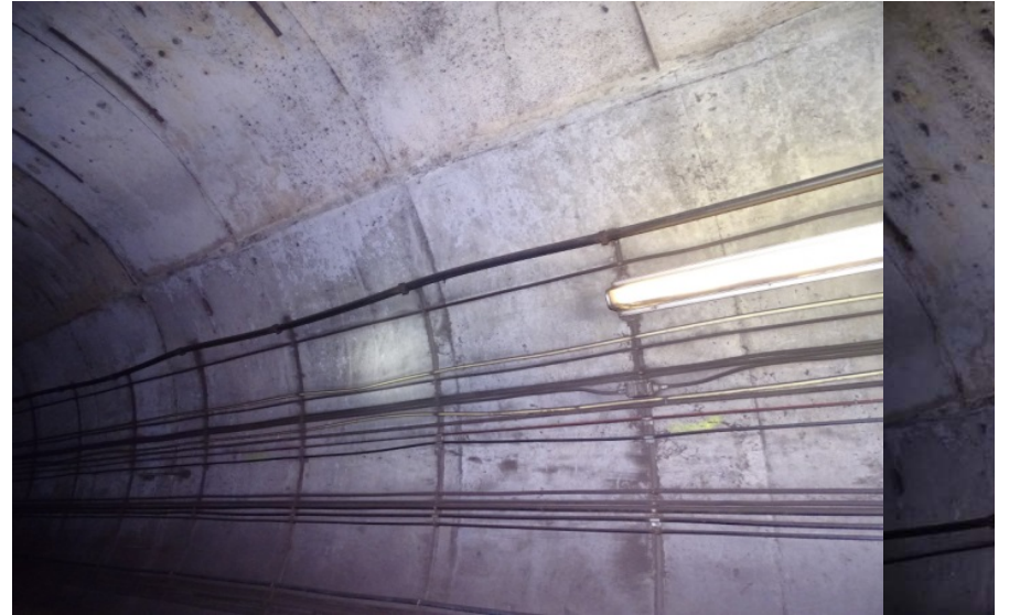
Photograph No. 394 Station 75+60, upper portion of west wall.
