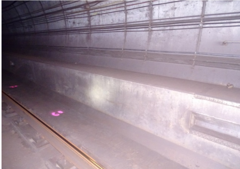
Photograph No. 389 Station 75+50, lower portion of west wall.
