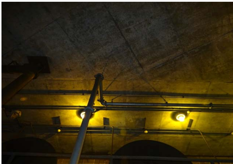
Photograph No. 109 Main room, ceiling, section 5.
