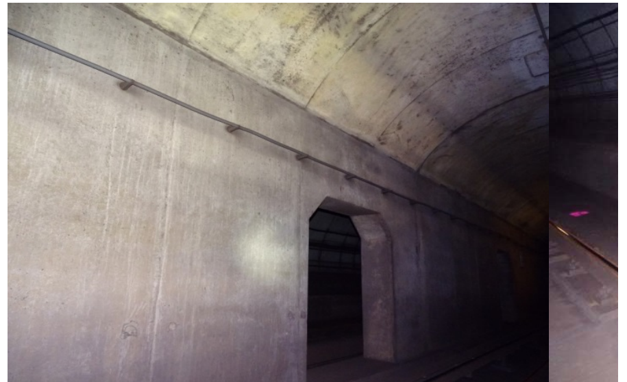
Photograph No. 392 Station 75+60, east wall.
