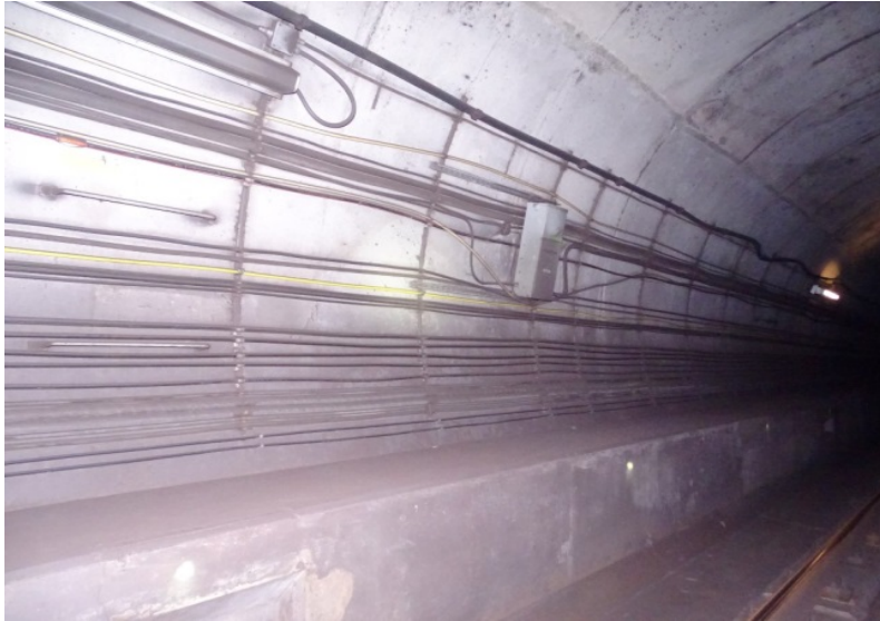
Photograph No. 213 Station 75+20, east wall.
