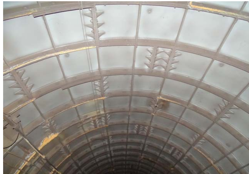
Photograph No. 12 Station 69+80, ceiling.
