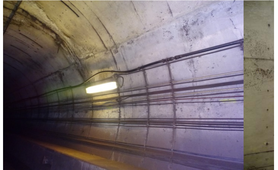
Photograph No. 498 Station 77+10, upper portion of west wall.
