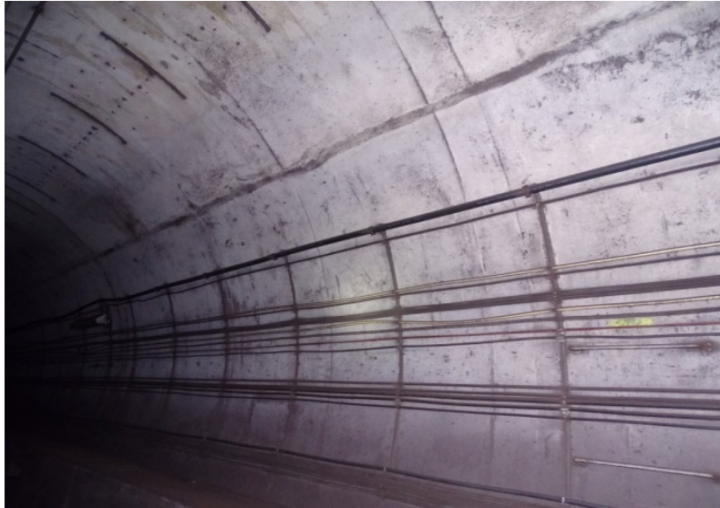
Photograph No. 561 Station 78+40, upper portion of west wall.
