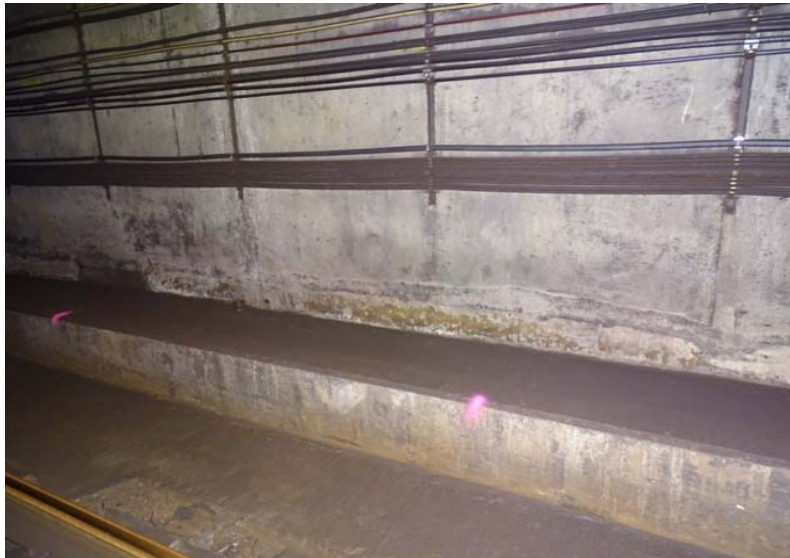
Photograph No. 249 Station 73+50, lower portion of west wall.
