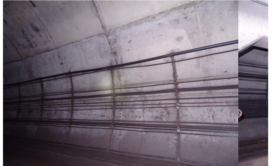
Photograph No. 510 Station 77+30, upper portion of west wall.
