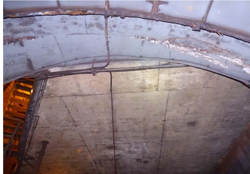
Photograph No. 38 Station 70+40, ceiling.
