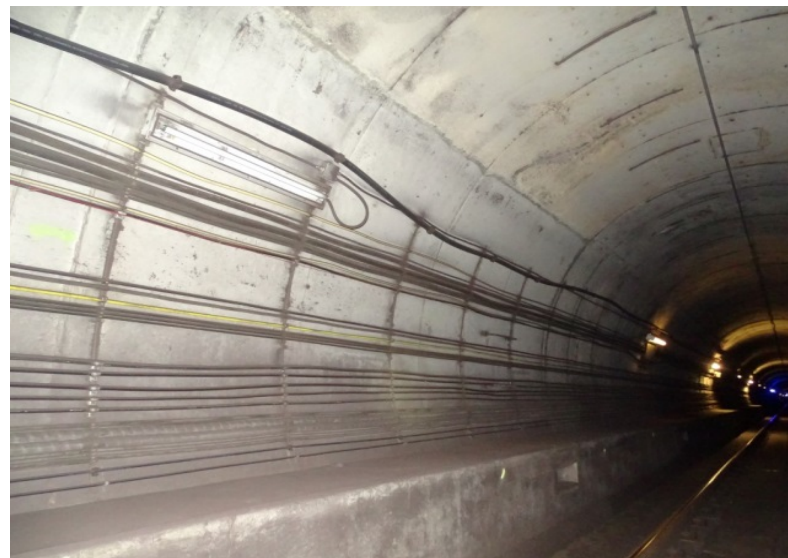
Photograph No. 322 Station 77+60, east wall.
