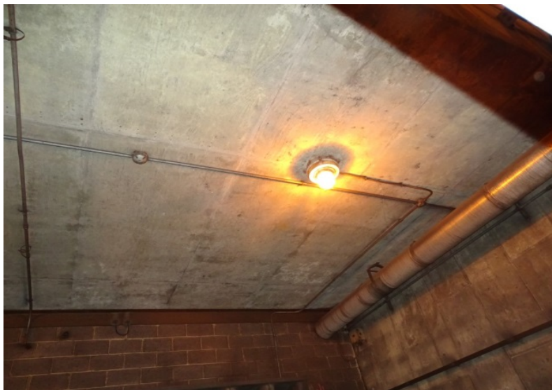
Photograph No. 153 Upper fan room, east wall, south end, middle-lower portion.
