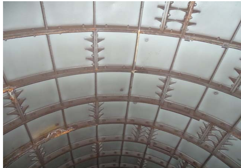
Photograph No. 8 Station 69+80, ceiling.
