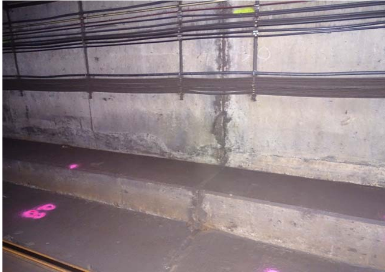
Photograph No. 261 Station 73+70, lower portion of west wall.
