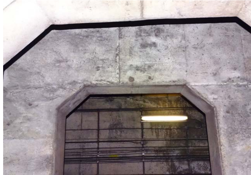
Photograph No. 26 Storage area, section 3, upper middle portion.
