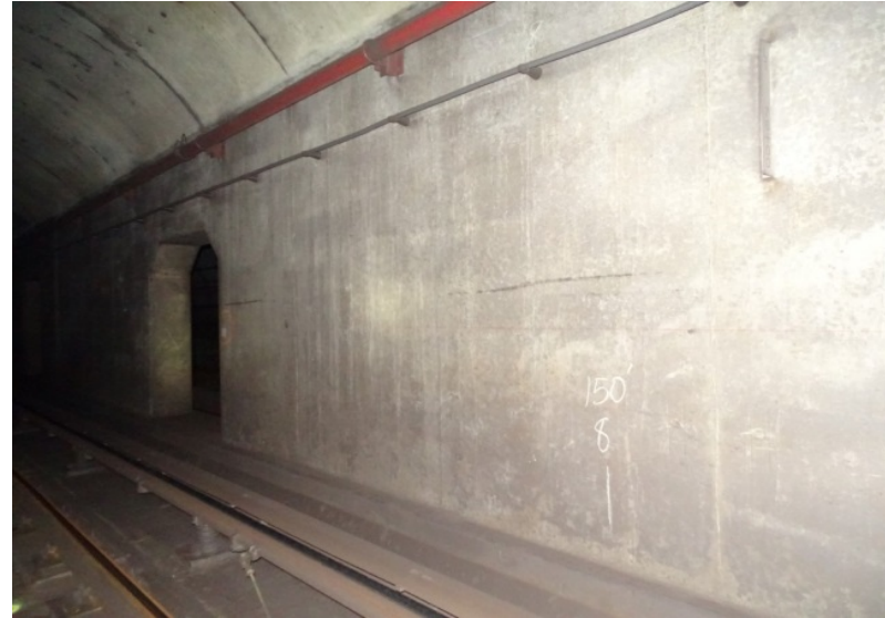
Photograph No. 250 Station 76+00, west wall.
