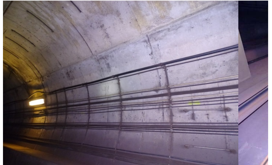
Photograph No. 492 Station 77+00, upper portion of west wall.
