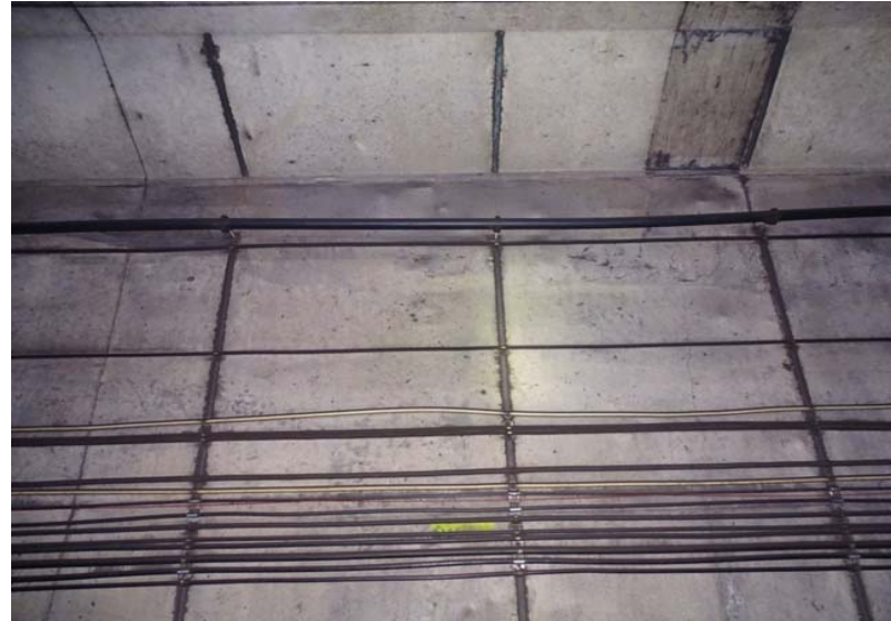
Photograph No. 186 Station 72+60, upper portion of west wall.
