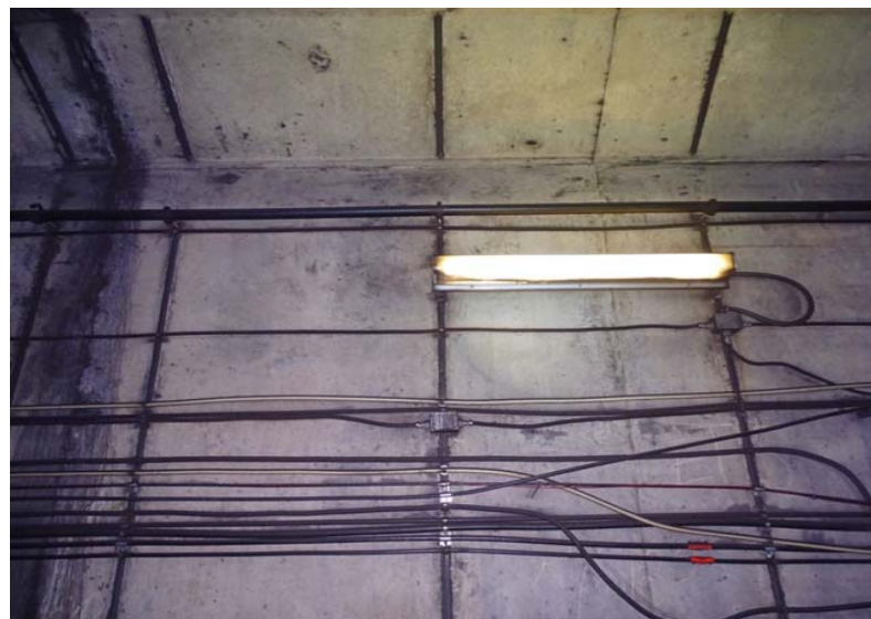
Photograph No. 228 Station 73+20, upper portion of west wall.
