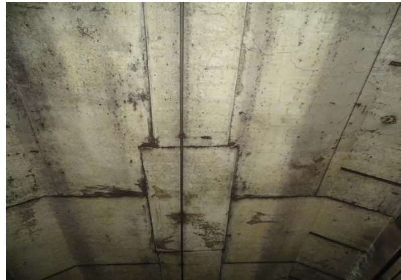
Photograph No. 290 Station 74+20, ceiling.
