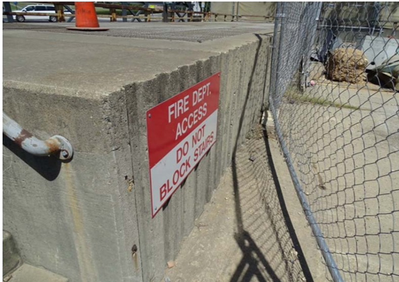
Photograph No. 185 Vent shaft exterior, close up of southeast side.
