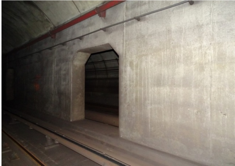
Photograph No. 233 Station 75+60, west wall.
