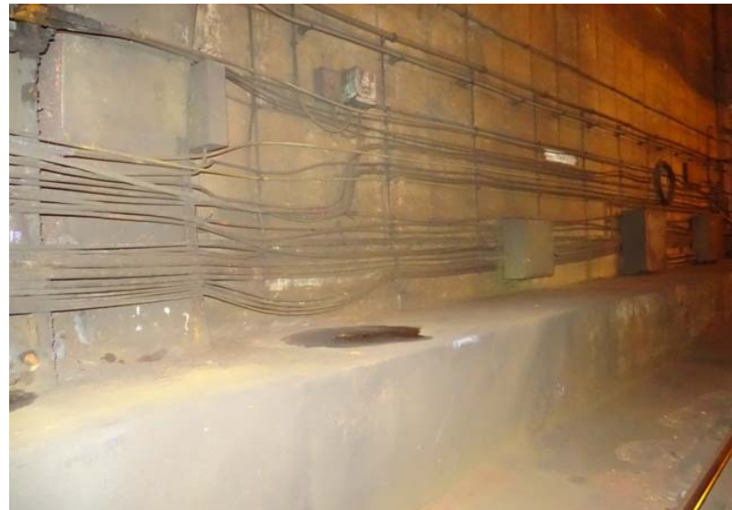
Photograph No. 32 Station 70+40, east wall.
