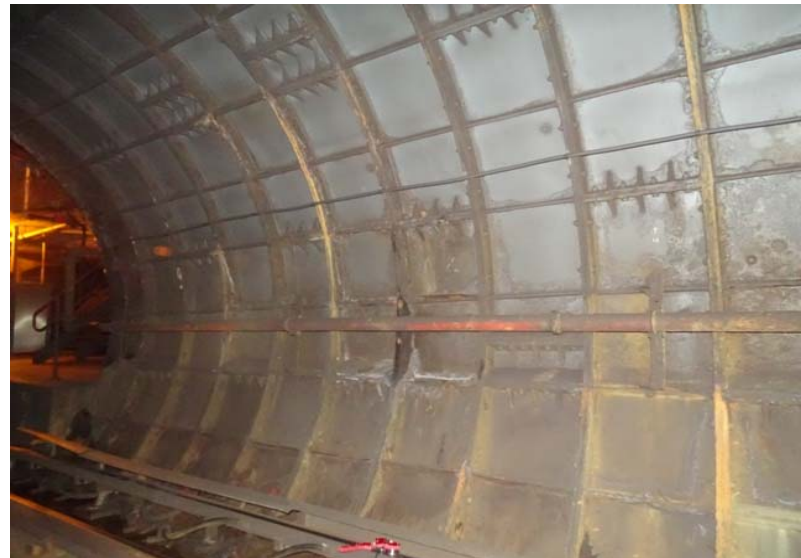
Photograph No. 28 Station 70+20, west wall.
