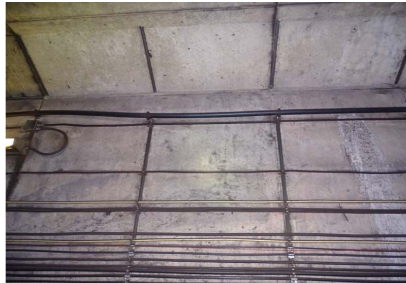
Photograph No. 272 Station 73+90, upper portion of west wall.
