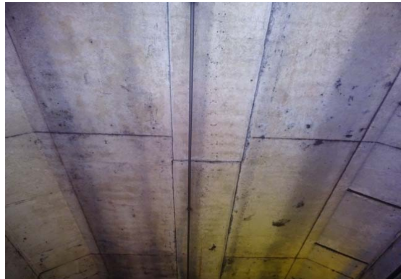
Photograph No. 220 Station 73+10, ceiling.
