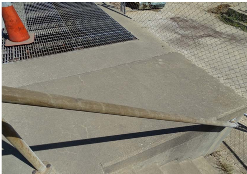
Photograph No. 191 Vent shaft exterior, south corner of deck.
