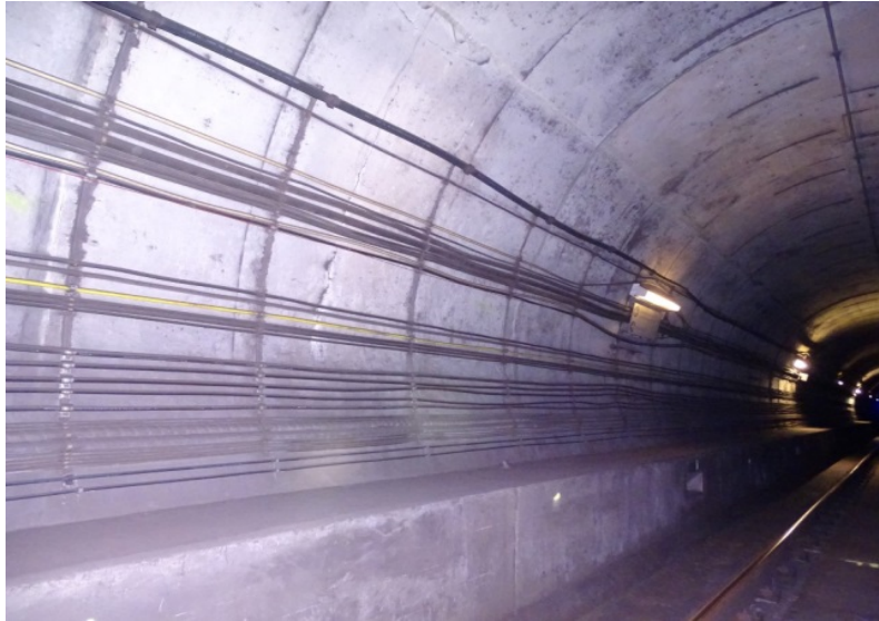
Photograph No. 329 Station 77+80, east wall.
