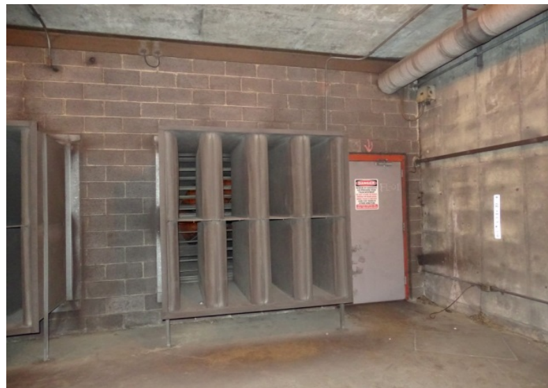
Photograph No. 154 Upper fan room, east wall, south end, lower portion.
