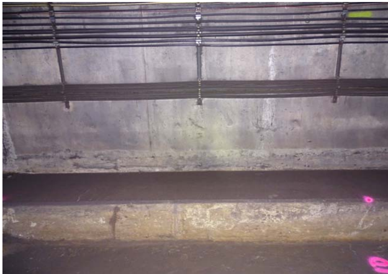
Photograph No. 153 Station 72+10, lower portion of west wall.
