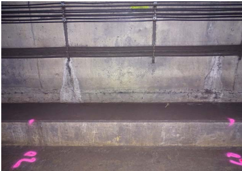
Photograph No. 187 Station 72+60, lower portion of west wall.
