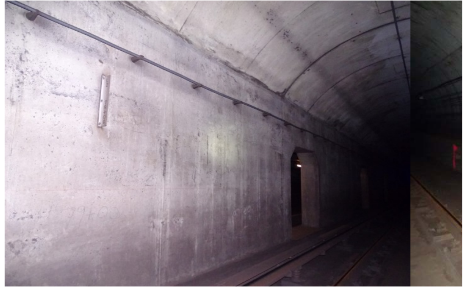
Photograph No. 570 Station 79+00, east wall.
