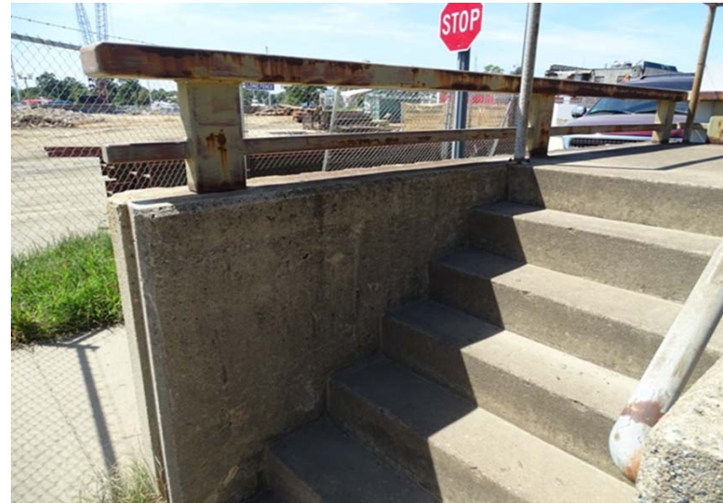
Photograph No. 186 Vent shaft exterior, steps at the south corner.
