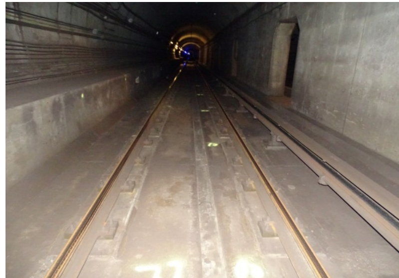
Photograph No. 296 Station 77+00, track bed.
