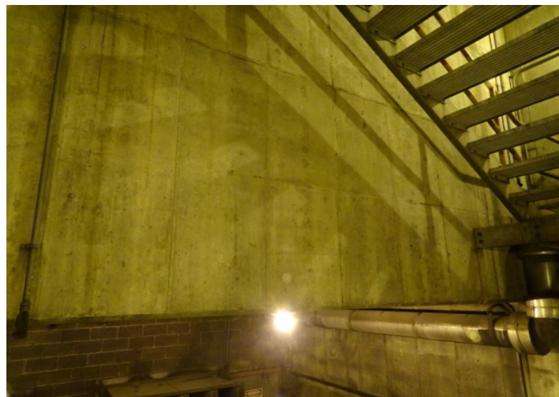
Photograph No. 152 Upper fan room, east wall, south end, middle portion.
