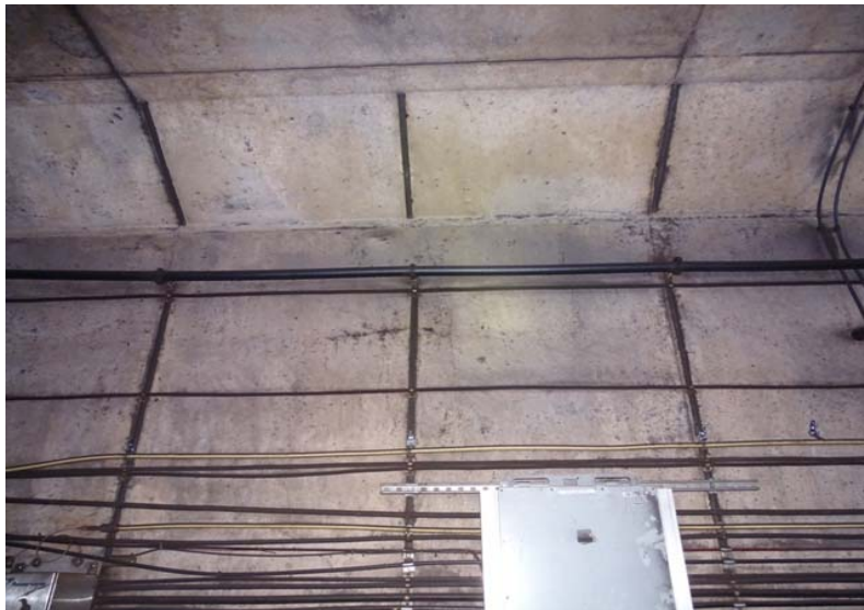
Photograph No. 135 Station 71+90, upper portion of west wall.
