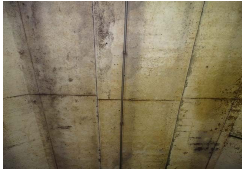
Photograph No. 116 Station 71+60, ceiling.
