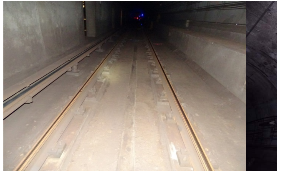
Photograph No. 532 Station 77+70, track bed.
