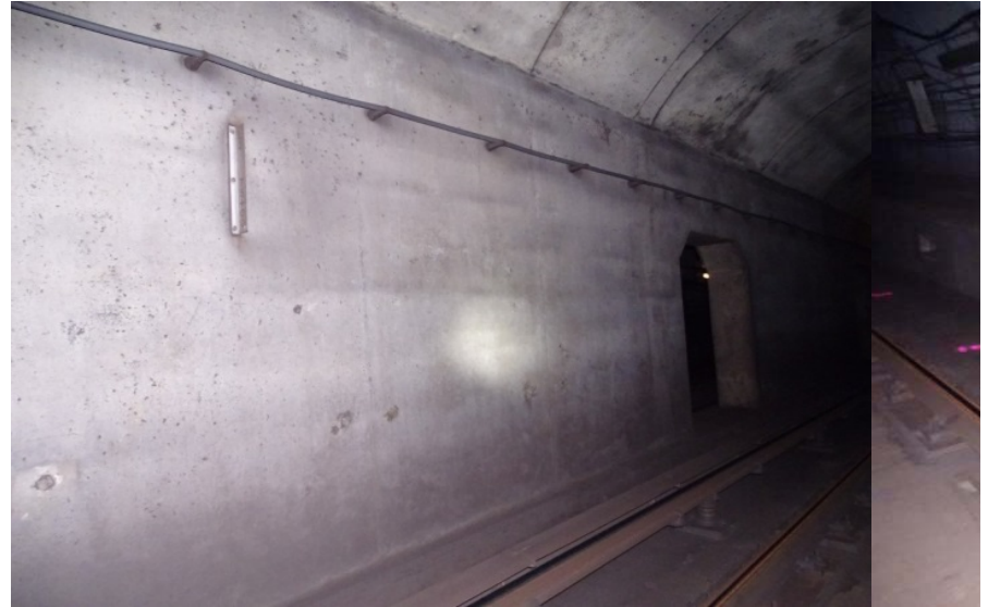
Photograph No. 350 Station 75+00, east wall.
