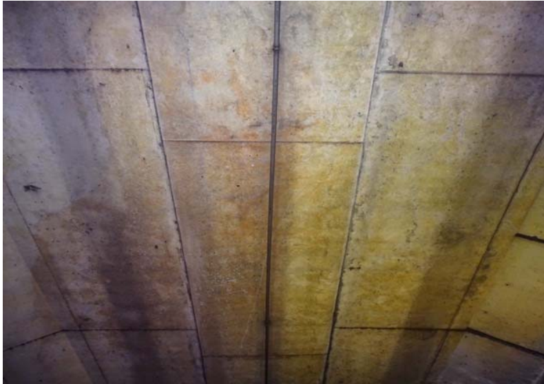
Photograph No. 173 Station 72+40, ceiling.
