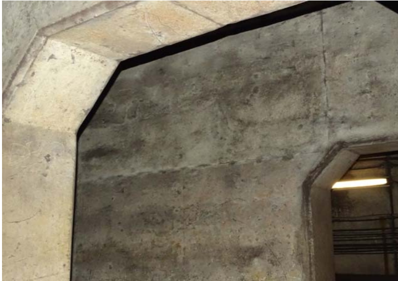
Photograph No. 9 Storage area, section 1, upper south portion.
