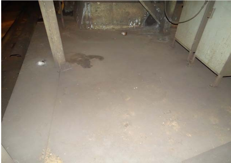
Photograph No. 53 Platform, floor, northwest portion.
