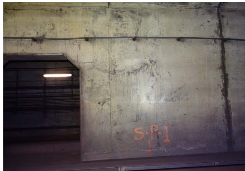
Photograph No. 252 Station 73+60, east wall.
