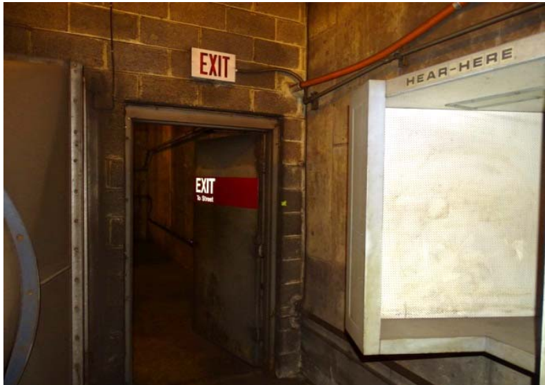
Photograph No. 129 Main room, upper level, west wall, north end.
