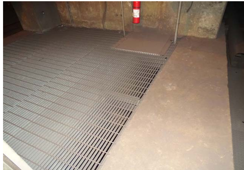
Photograph No. 40 Platform, floor, southwest portion.
