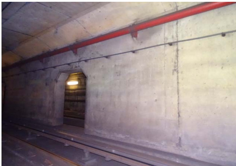
Photograph No. 141 Station 73+20, west wall.
