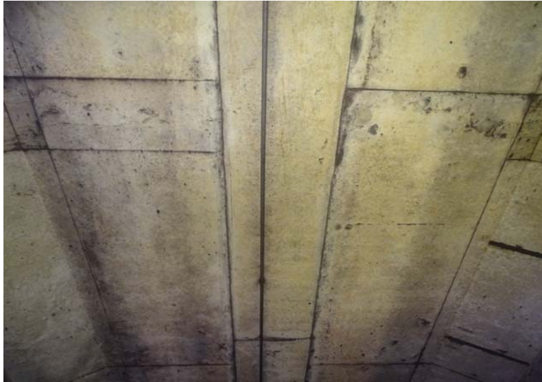
Photograph No. 277 Station 74+00, ceiling.
