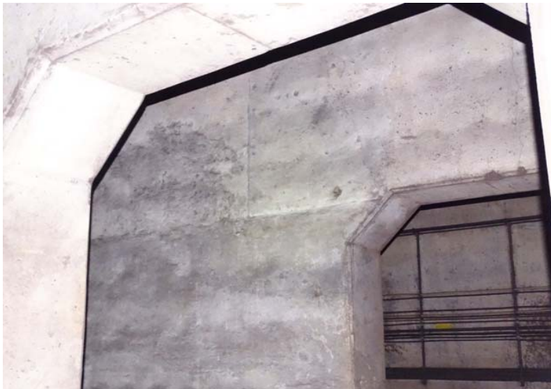
Photograph No. 19 Storage area, section 2, upper south portion.
