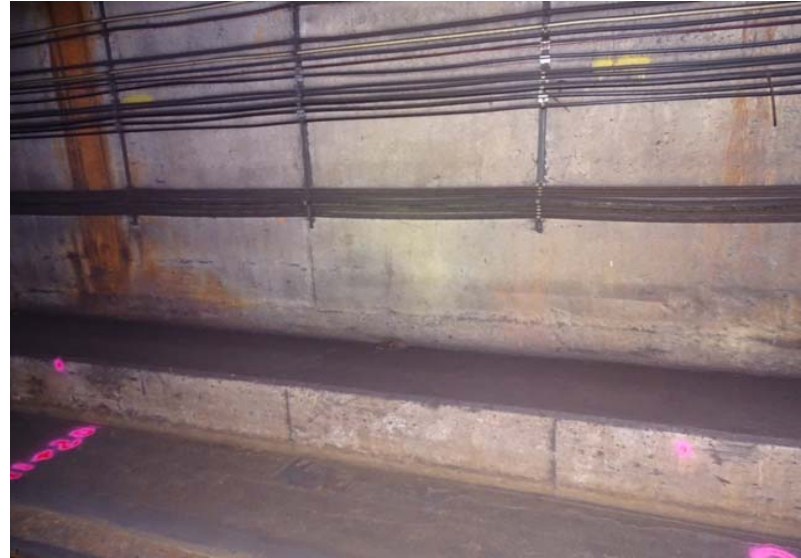
Photograph No. 82 Station 71+10, lower portion of west wall.
