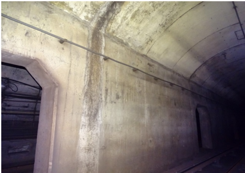
Photograph No. 503 Station 77+20, east wall.
