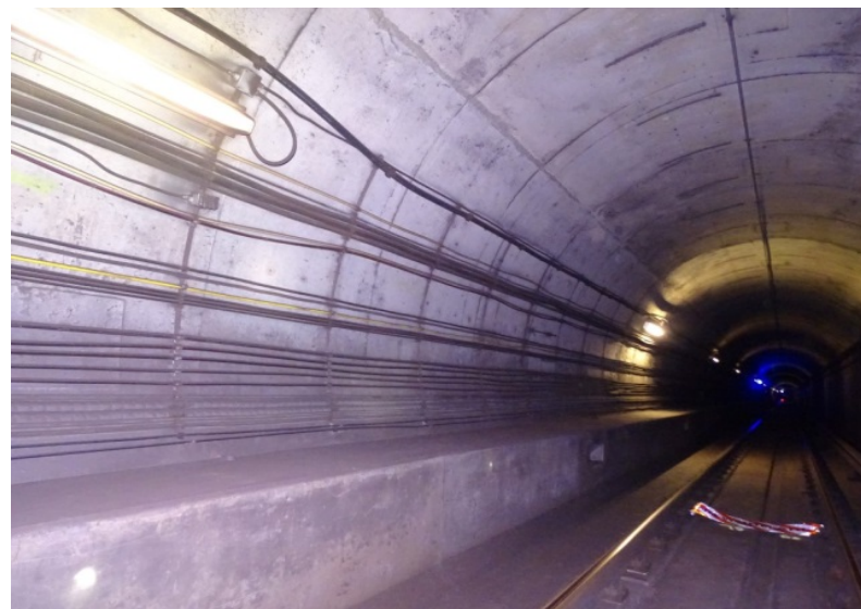
Photograph No. 364 Station 78+80, east wall.
