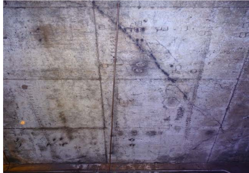
Photograph No. 62 Station 70+80, ceiling.
