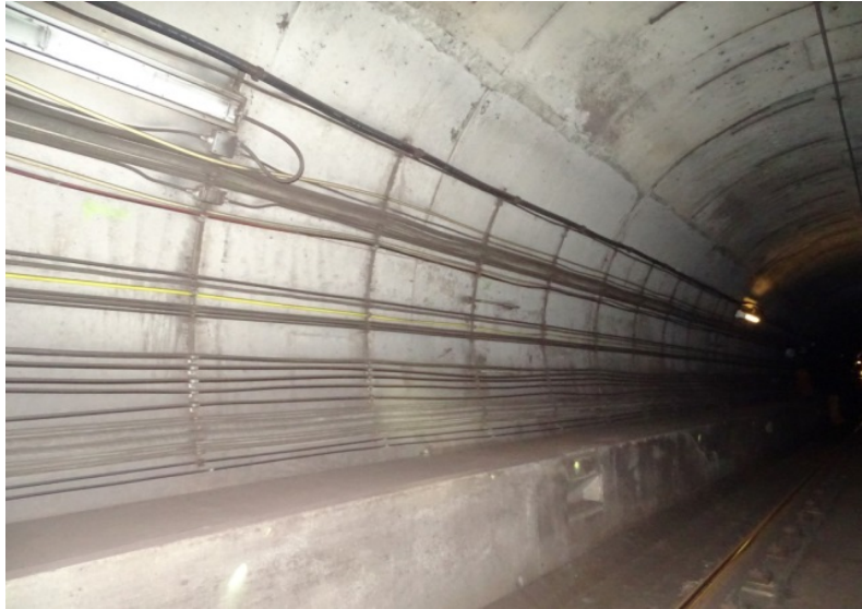
Photograph No. 265 Station 76+40, east wall.
