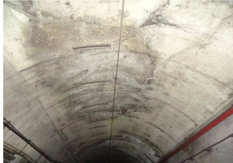
Photograph No. 298 Station 77+00, ceiling.
