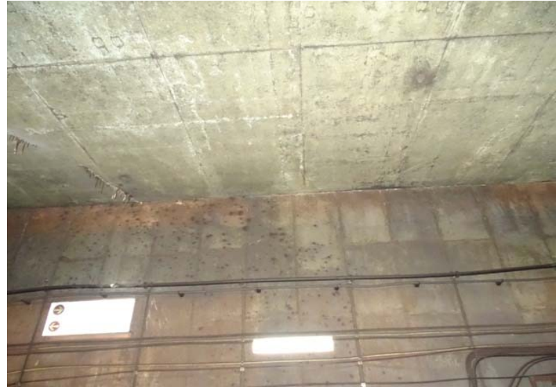
Photograph No. 58 Station 70+70, upper portion of west wall.
