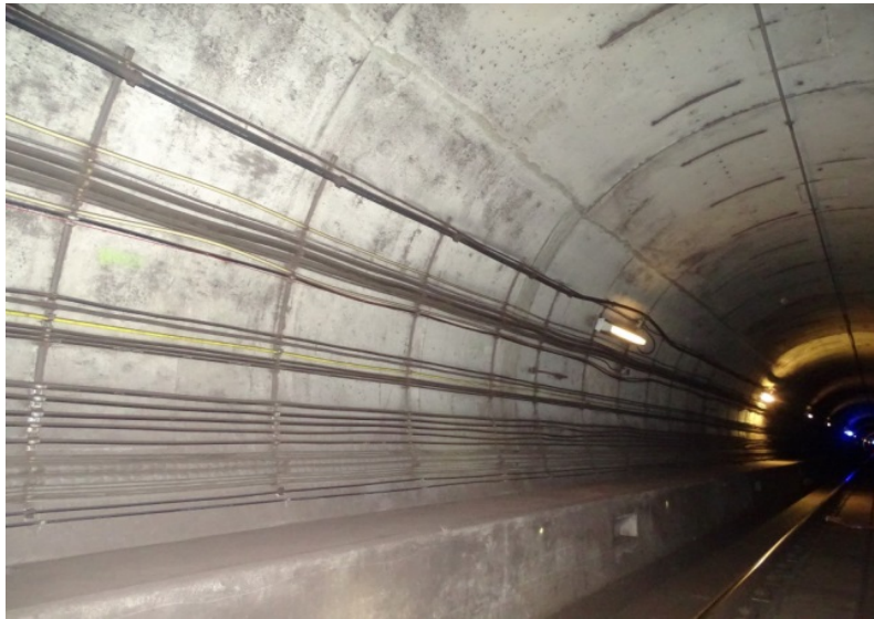
Photograph No. 357 Station 78+60, east wall.
