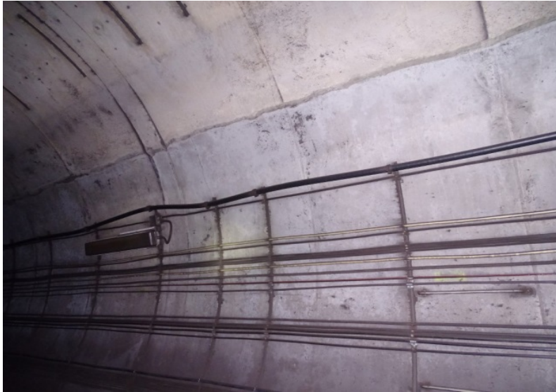
Photograph No. 521 Station 77+50, upper portion of west wall.
