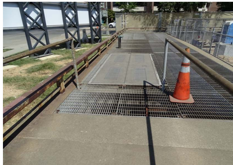
Photograph No. 190 Vent shaft exterior, looking northeast at deck.
