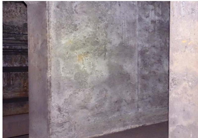
Photograph No. 24 Storage area, section 3, lower north portion.
