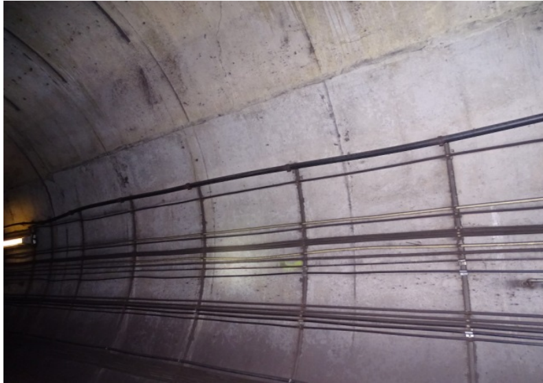
Photograph No. 409 Station 75+80, upper portion of west wall.
