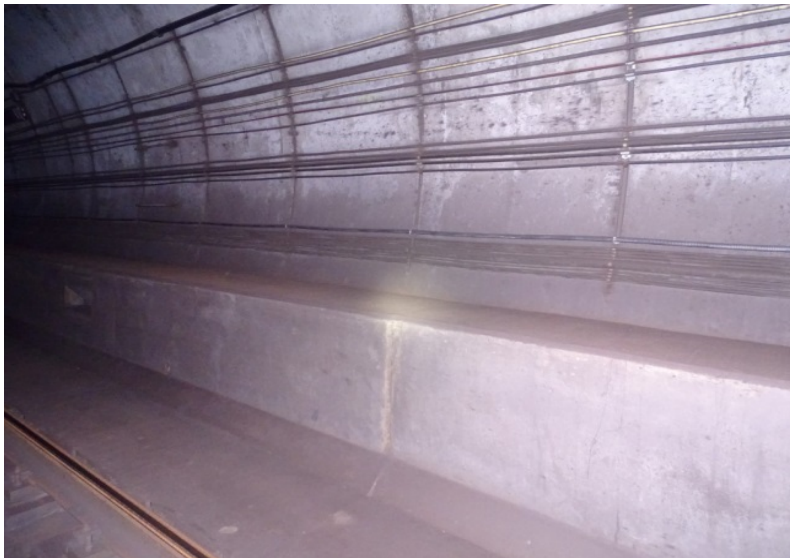
Photograph No. 511 Station 77+30, lower portion of west wall.
