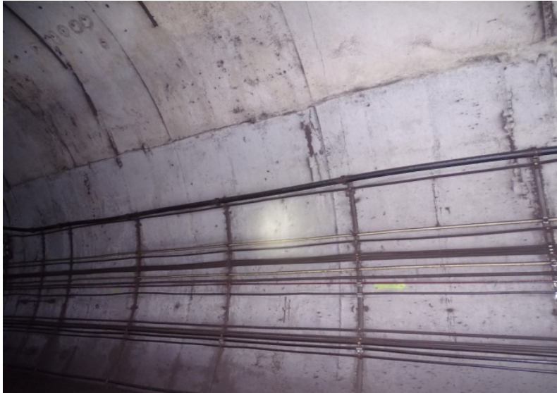
Photograph No. 465 Station 76+60, upper portion of west wall.
