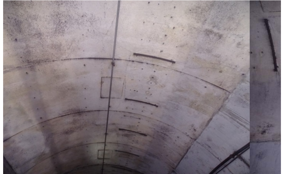
Photograph No. 478 Station 76+80, ceiling.
