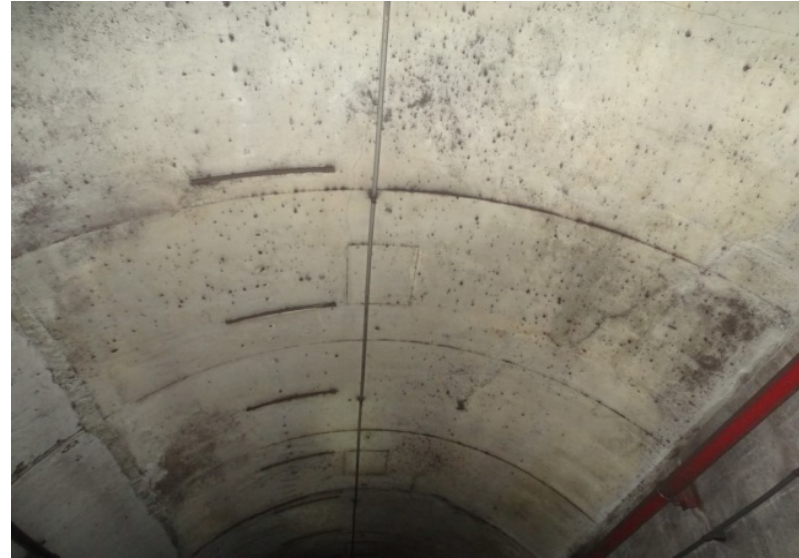
Photograph No. 266 Station 76+40, ceiling.
