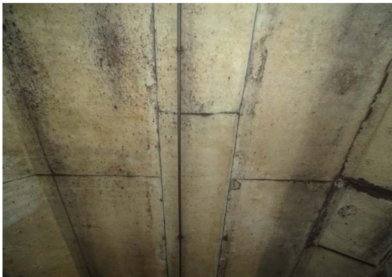
Photograph No. 241 Station 73+40, ceiling.
