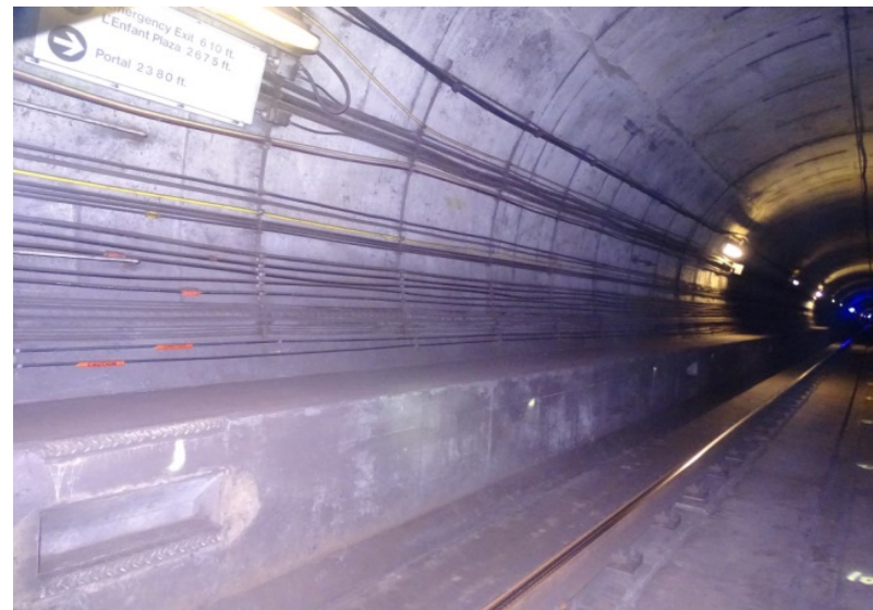
Photograph No. 336 Station 78+00, east wall.
