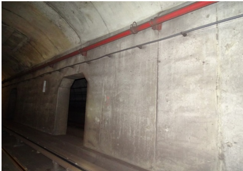
Photograph No. 331 Station 77+80, west wall.
