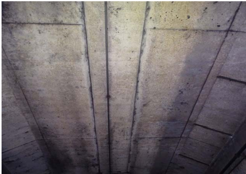
Photograph No. 283 Station 74+10, ceiling.
