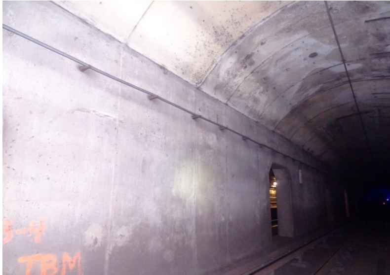
Photograph No. 533 Station 77+70, east wall.
