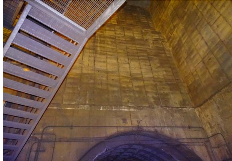
Photograph No. 58 Main room, looking up at north wall.
