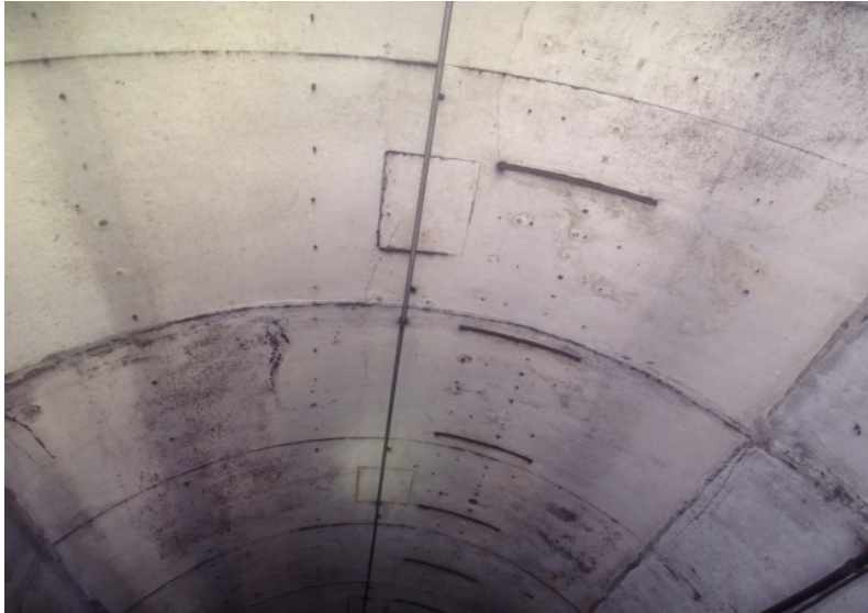
Photograph No. 509 Station 77+30, ceiling.
