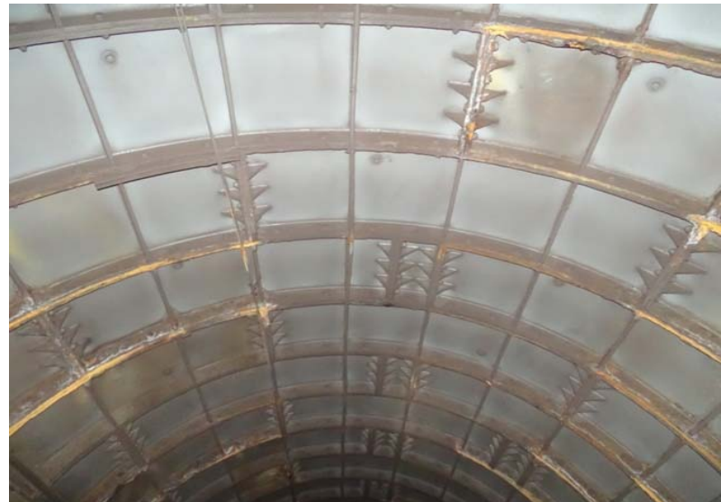
Photograph No. 20 Station 70+00, ceiling.
