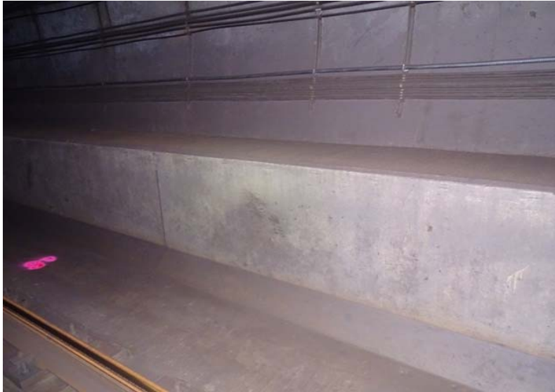
Photograph No. 329 Station 74+70, lower portion of west wall.
