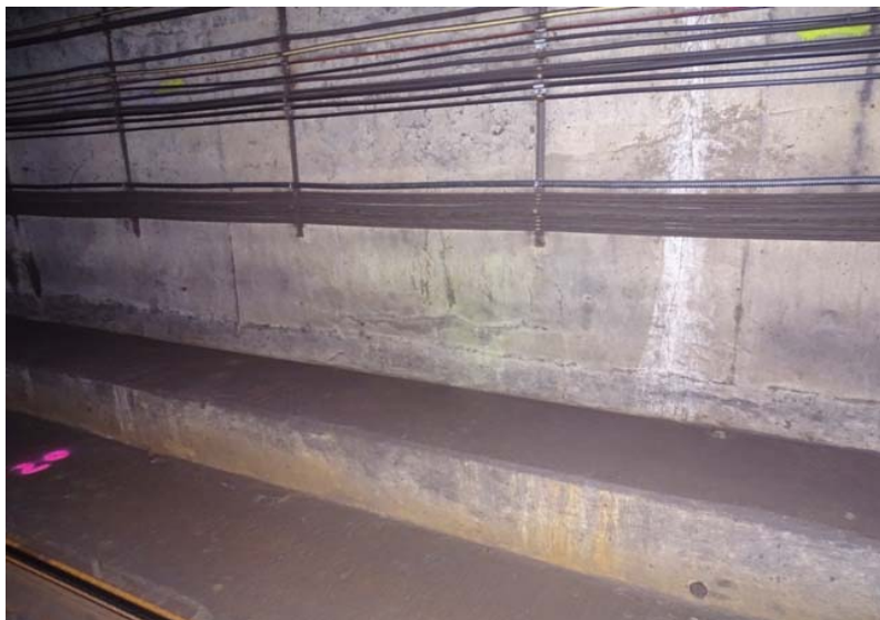
Photograph No. 285 Station 74+10, lower portion of west wall.
