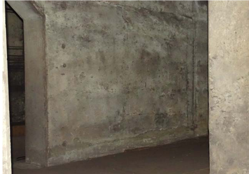
Photograph No. 14 Storage area, section 2, lower north portion.
