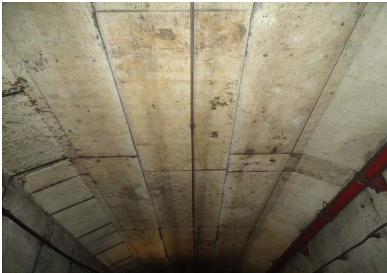
Photograph No. 59 Station 71+40, ceiling.
