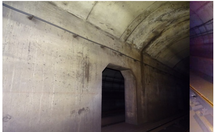
Photograph No. 496 Station 77+10, east wall.
