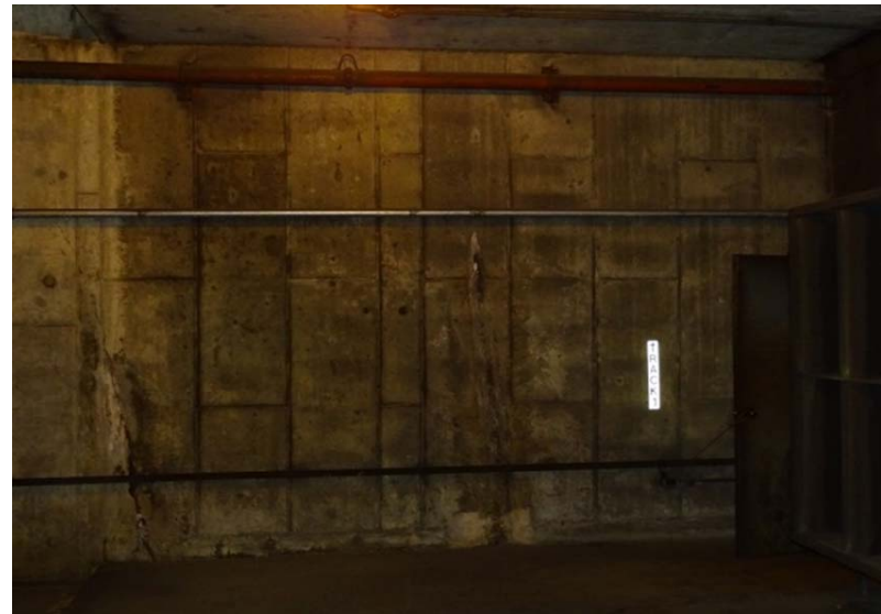
Photograph No. 136 Upper fan room, north wall, lower-east portion.
