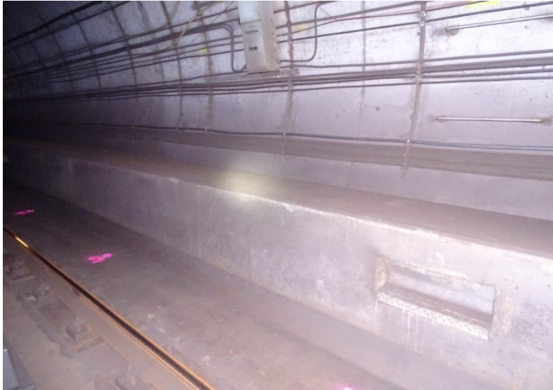
Photograph No. 369 Station 75+20, lower portion of west wall.
