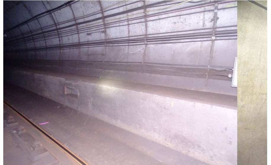
Photograph No. 454 Station 76+40, lower portion of west wall.
