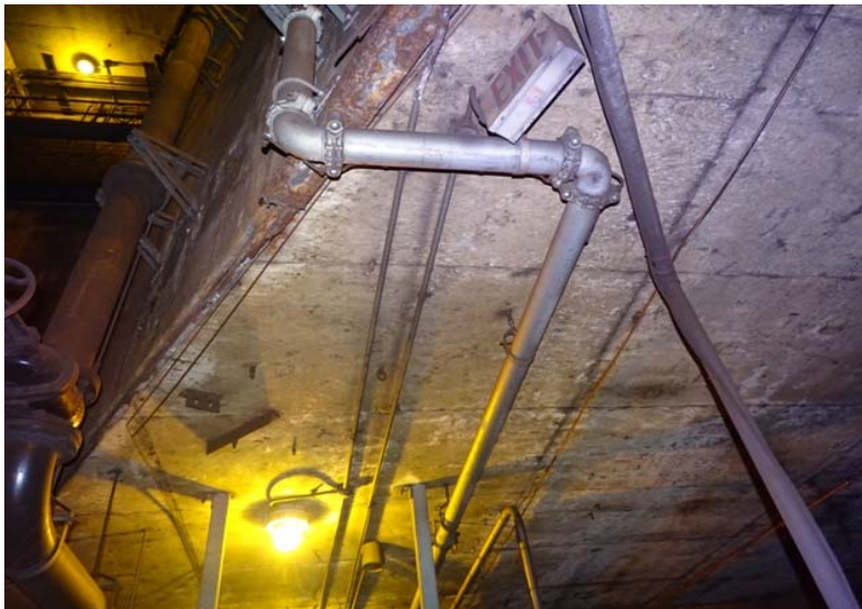
Photograph No. 43 Platform, ceiling, looking south.
