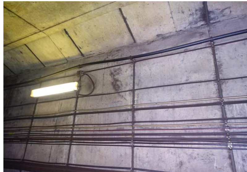
Photograph No. 248 Station 73+50, upper portion of west wall.
