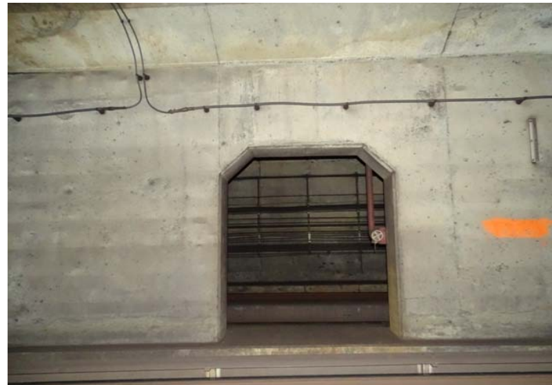
Photograph No. 132 Station 71+90, east wall.
