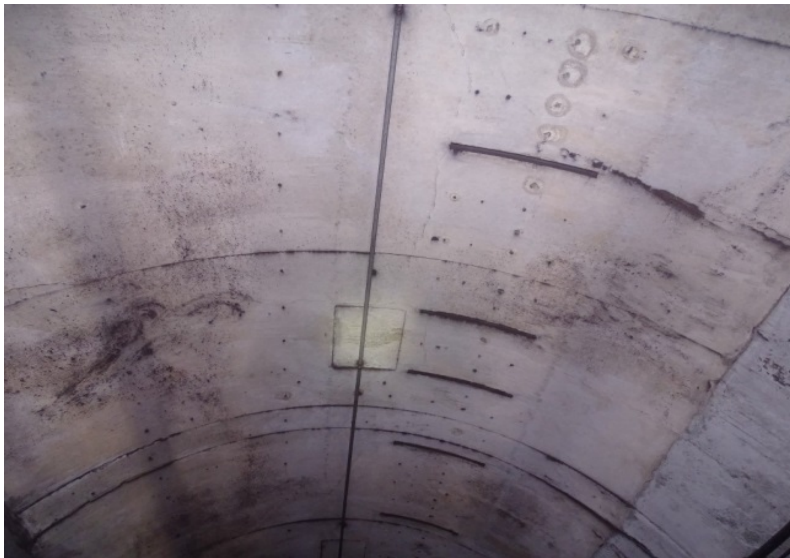
Photograph No. 471 Station 76+70, ceiling.
