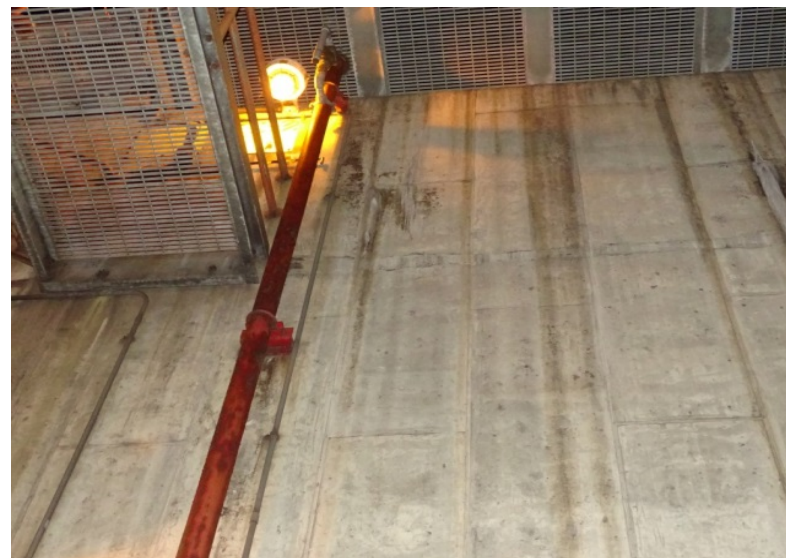
Photograph No. 164 Upper fan room, west wall, middle-north section, upper portion.
