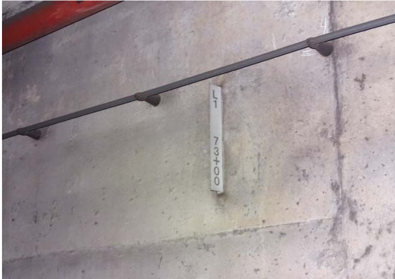
Photograph No. 81 Station 72+00 - marker for L1 73+00.
