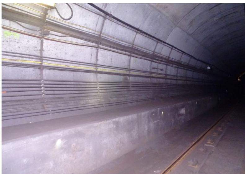
Photograph No. 231 Station 75+60, east wall.
