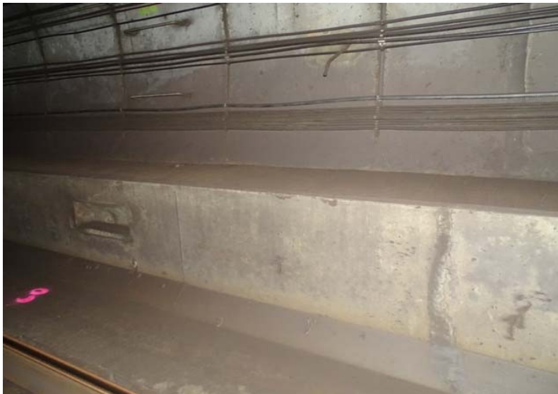
Photograph No. 315 Station 74+50, lower portion of west wall.
