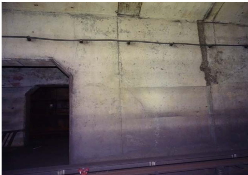
Photograph No. 85 Station 71+20, east wall.
