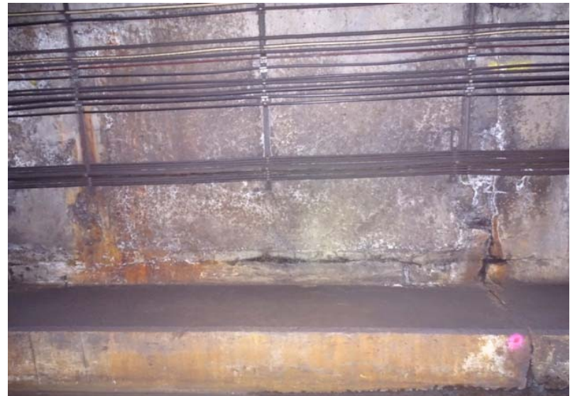
Photograph No. 96 Station 71+30, lower portion of west wall.
