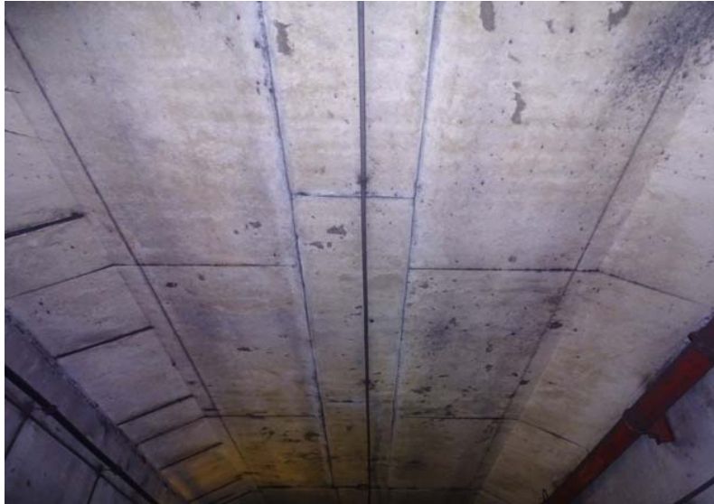
Photograph No. 133 Station 73+00, ceiling.
