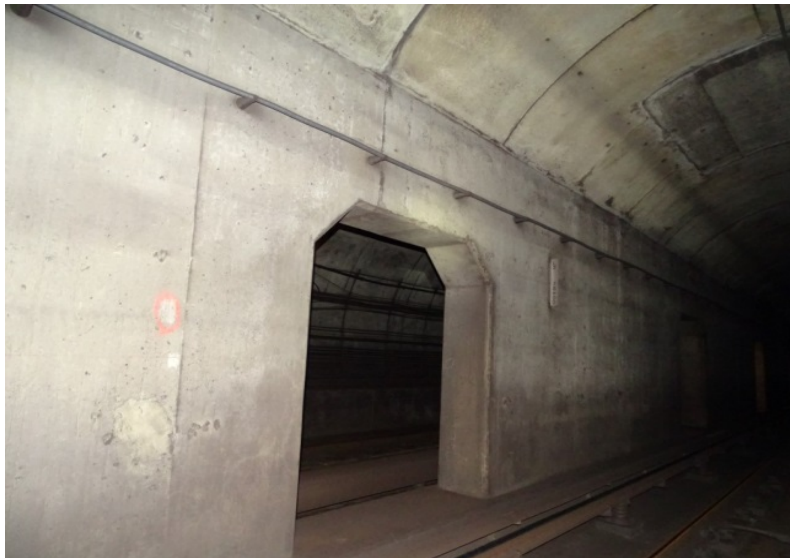
Photograph No. 539 Station 77+80, east wall.
