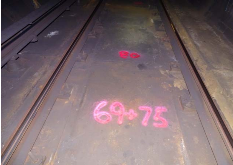
Photograph No. 1 Station 69+70, track bed.
