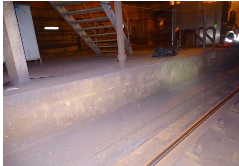
Photograph No. 44 Station 70+50, east wall.
