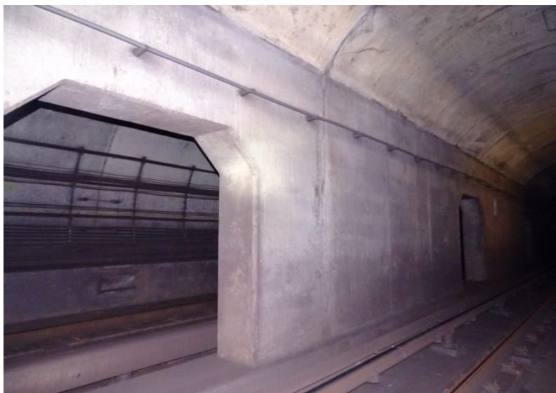
Photograph No. 399 Station 75+70, east wall.
