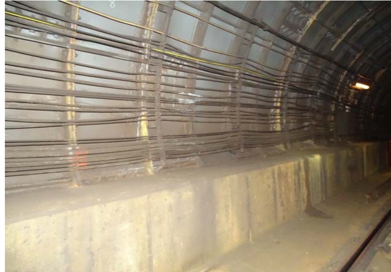
Photograph No. 2 Station 69+60, east wall.
