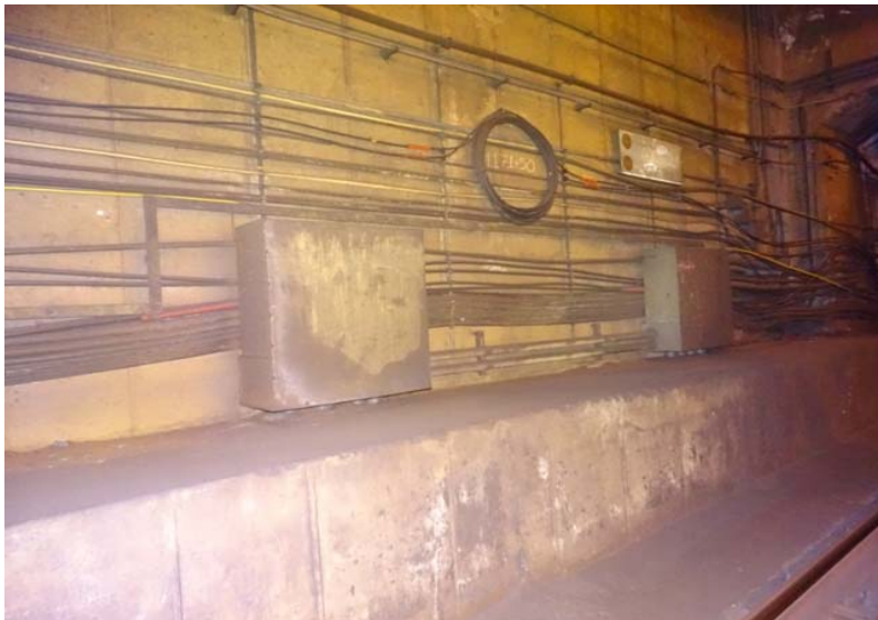
Photograph No. 35 Station 70+60, east wall.
