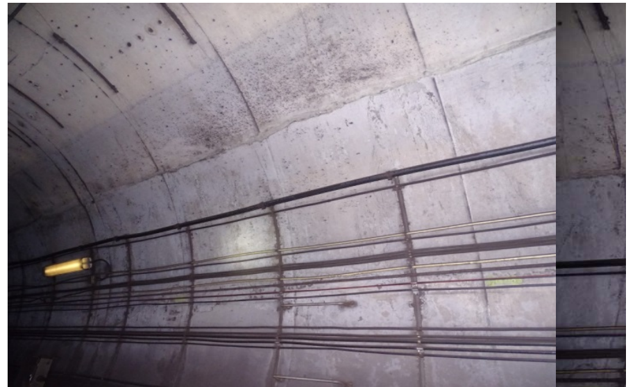
Photograph No. 440 Station 76+20, upper portion of west wall.
