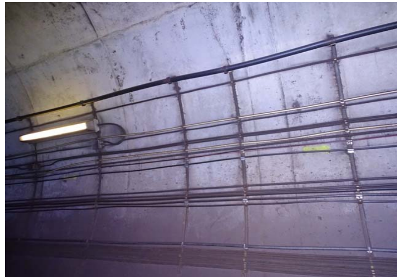
Photograph No. 328 Station 74+70, upper portion of west wall.
