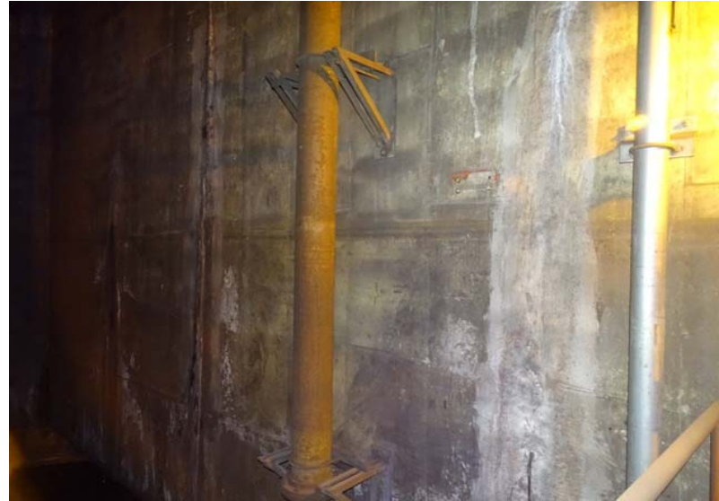
Photograph No. 74 Main room, west wall.
