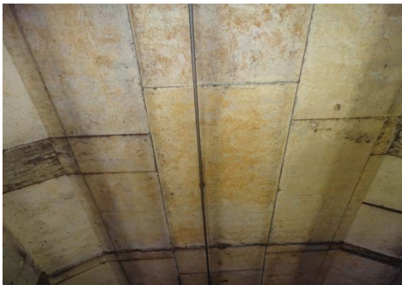
Photograph No. 87 Station 71+20, ceiling.
