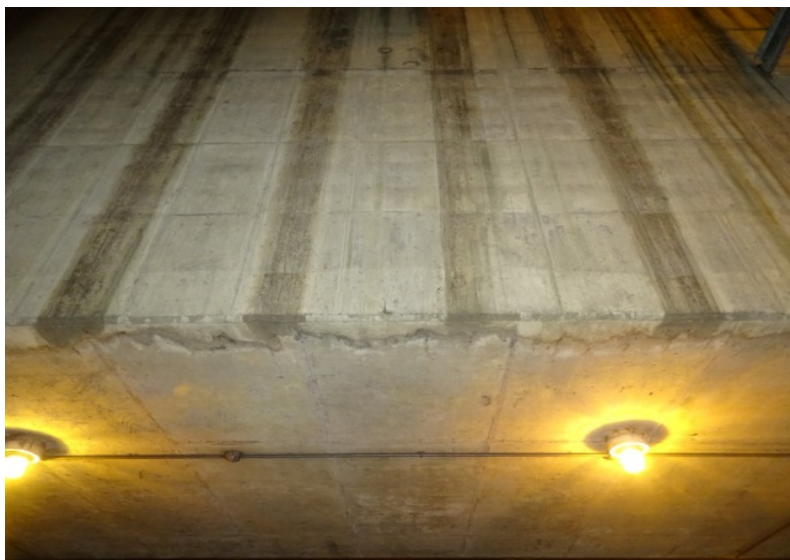
Photograph No. 143 Upper fan room, east wall, north-center section, middle-upper portion.
