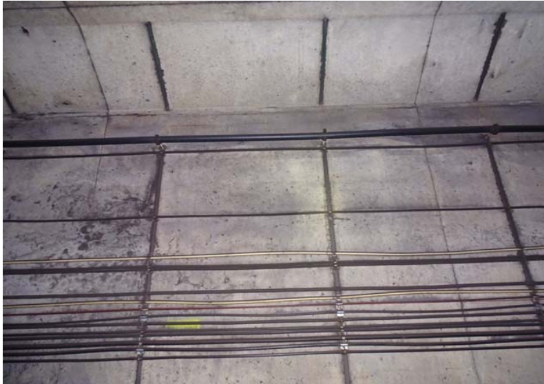
Photograph No. 193 Station 72+70, upper portion of west wall.
