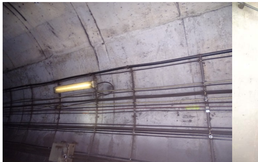
Photograph No. 448 Station 76+30, upper portion of west wall.
