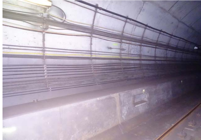
Photograph No. 198 Station 74+80, east wall.
