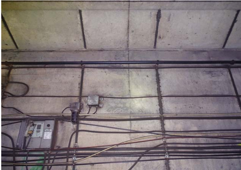
Photograph No. 221 Station 73+10, upper portion of west wall.
