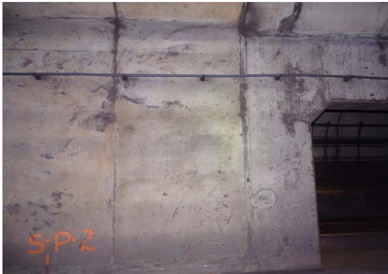
Photograph No. 295 Station 74+30, east wall.
