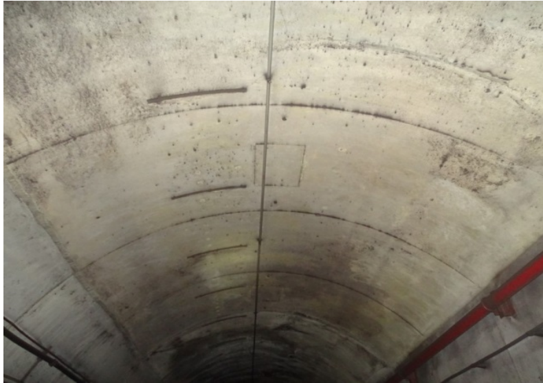
Photograph No. 289 Station 76+80, ceiling.
