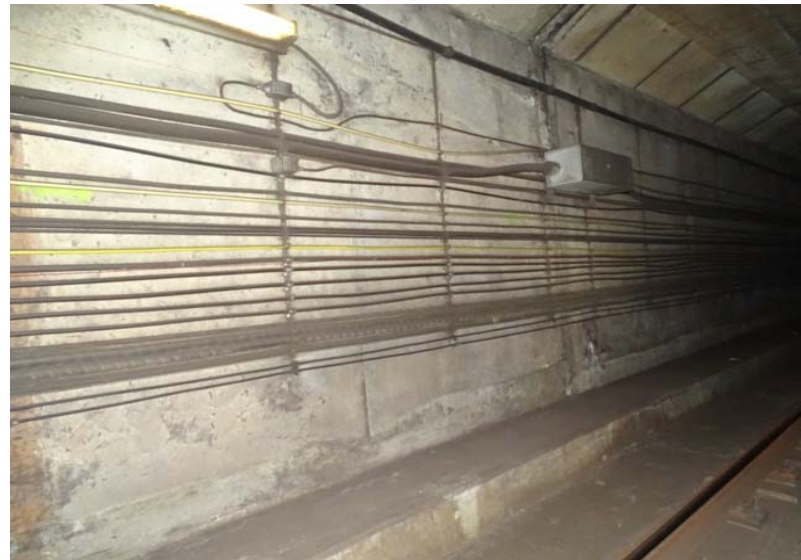
Photograph No. 64 Station 71+60, east wall.
