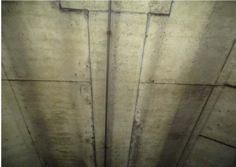
Photograph No. 205 Station 72+90, ceiling.
