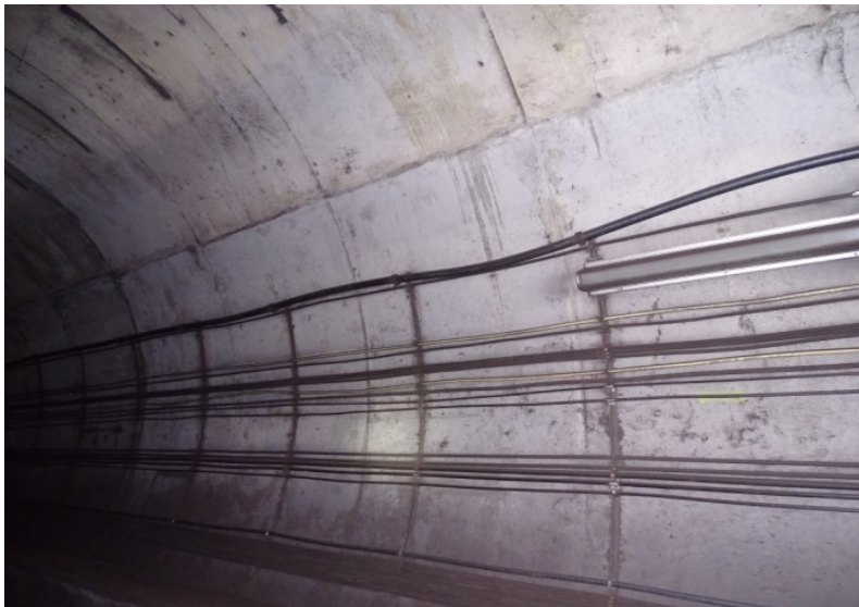
Photograph No. 479 Station 76+80, upper portion of west wall.
