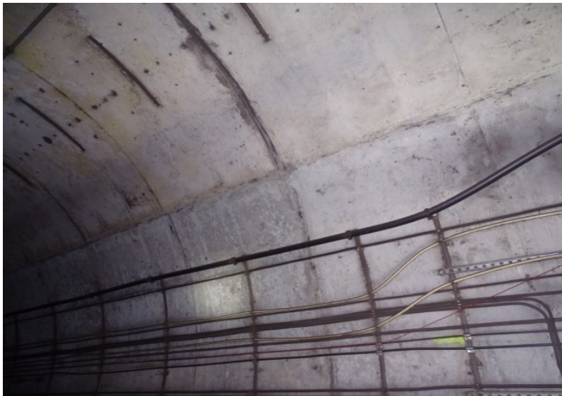
Photograph No. 375 Station 75+30, upper portion of west wall.
