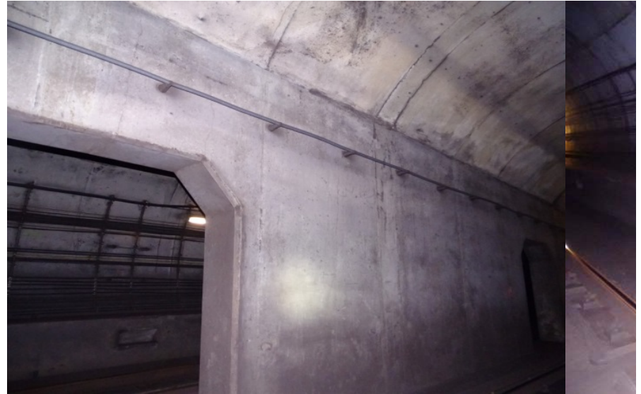
Photograph No. 470 Station 76+70, east wall.
