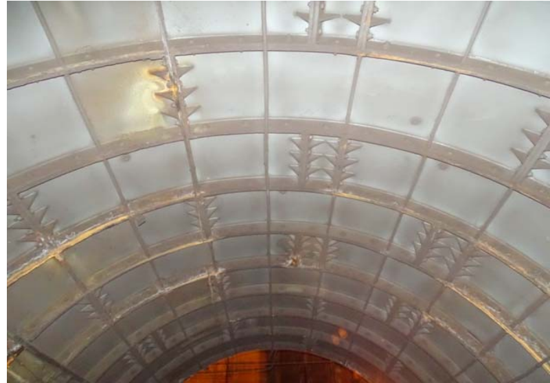
Photograph No. 26 Station 70+20, ceiling.
