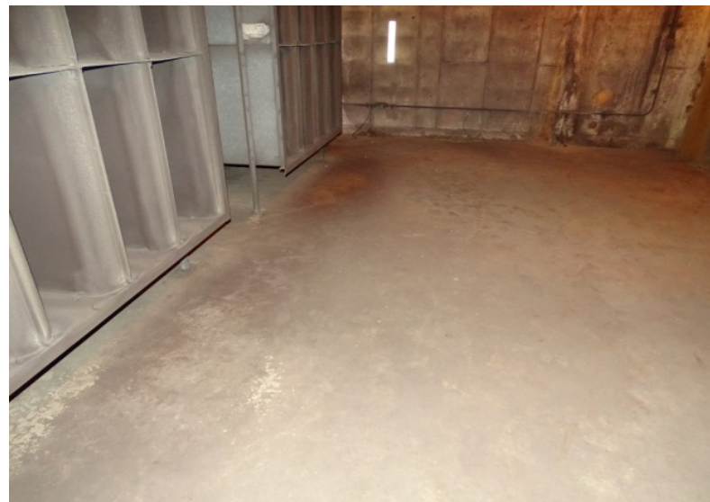
Photograph No. 178 Upper fan room floor, south section, east end.
