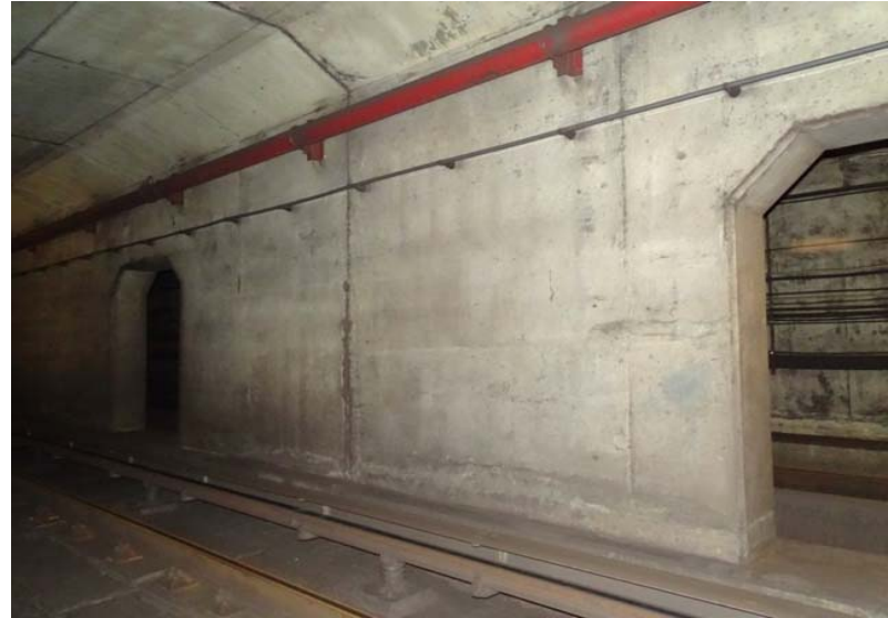
Photograph No. 158 Station 73+60, west wall.
