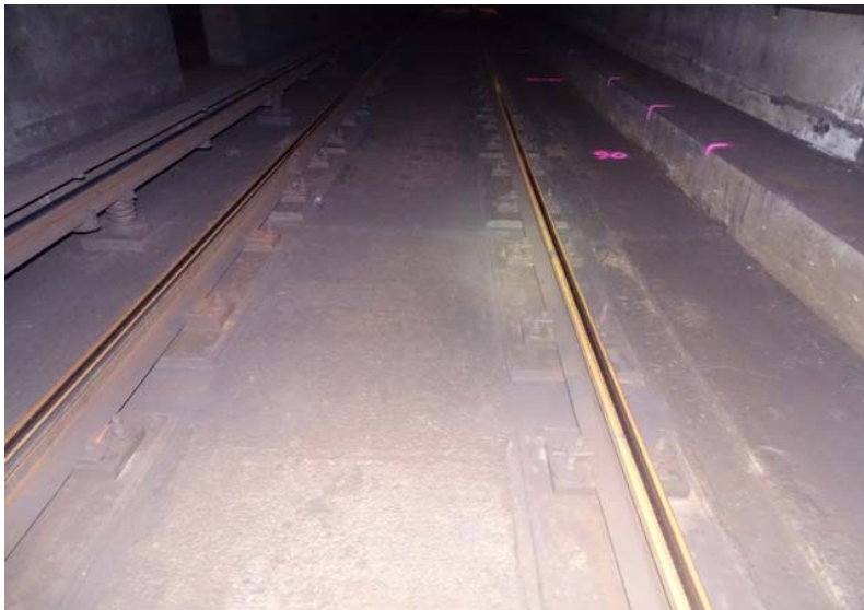
Photograph No. 195 Station 72+80, track bed.
