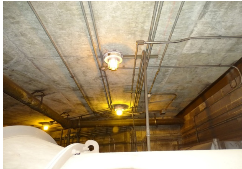
Photograph No. 130 Main room, upper level, southwest portion of ceiling.
