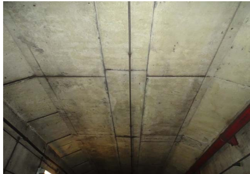
Photograph No. 164 Station 73+80, ceiling.
