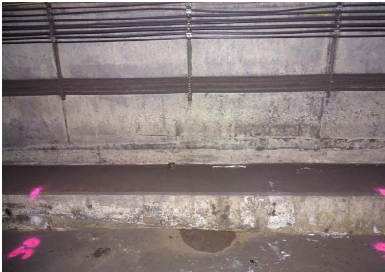
Photograph No. 175 Station 72+40, lower portion of west wall.
