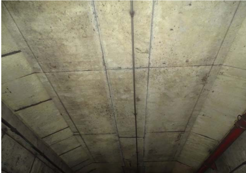
Photograph No. 169 Station 74+00, ceiling.
