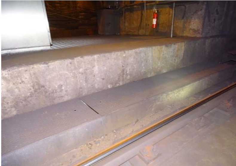
Photograph No. 61 Station 70+80, east wall.
