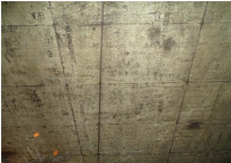
Photograph No. 51 Station 70+60, ceiling.
