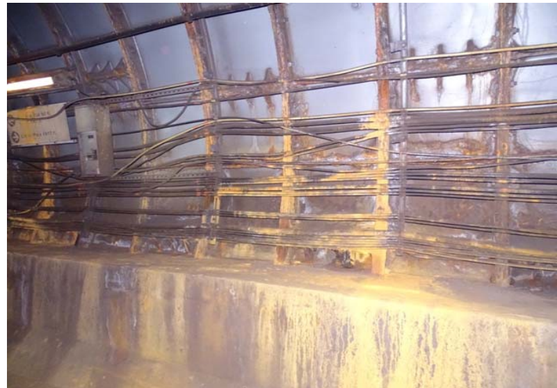
Photograph No. 28 Station 70+20, west wall.
