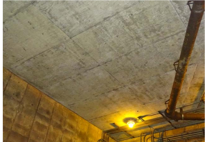
Photograph No. 106 Main room, ceiling, section 3, south end.
