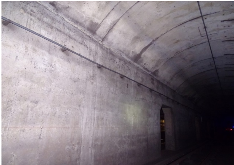
Photograph No. 559 Station 78+40, east wall.
