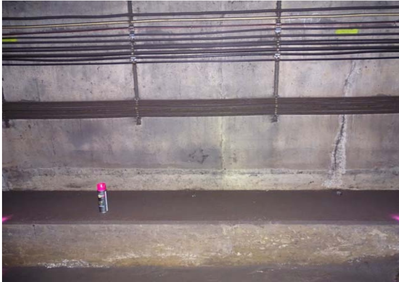
Photograph No. 161 Station 72+20, lower portion of west wall.
