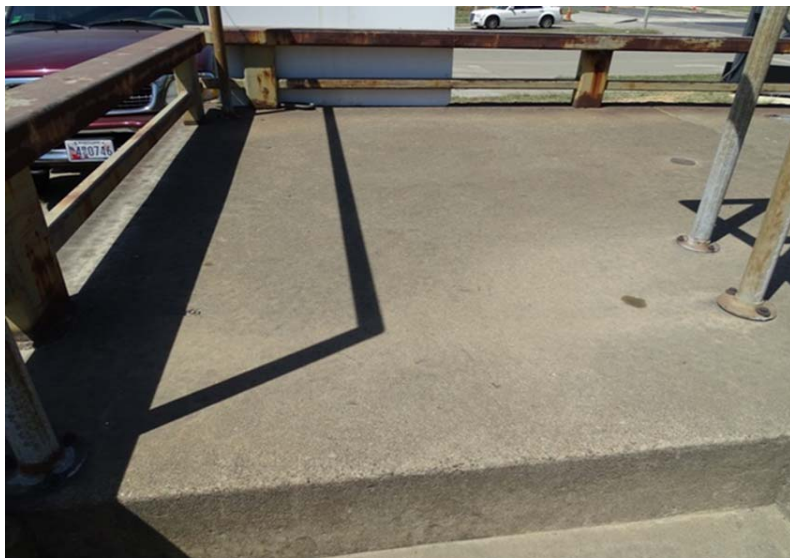
Photograph No. 189 Vent shaft exterior, south end of deck.
