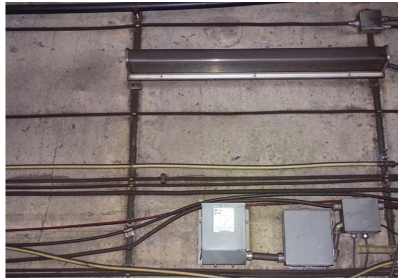
Photograph No. 144 Station 72+00 - cracks on west wall.
