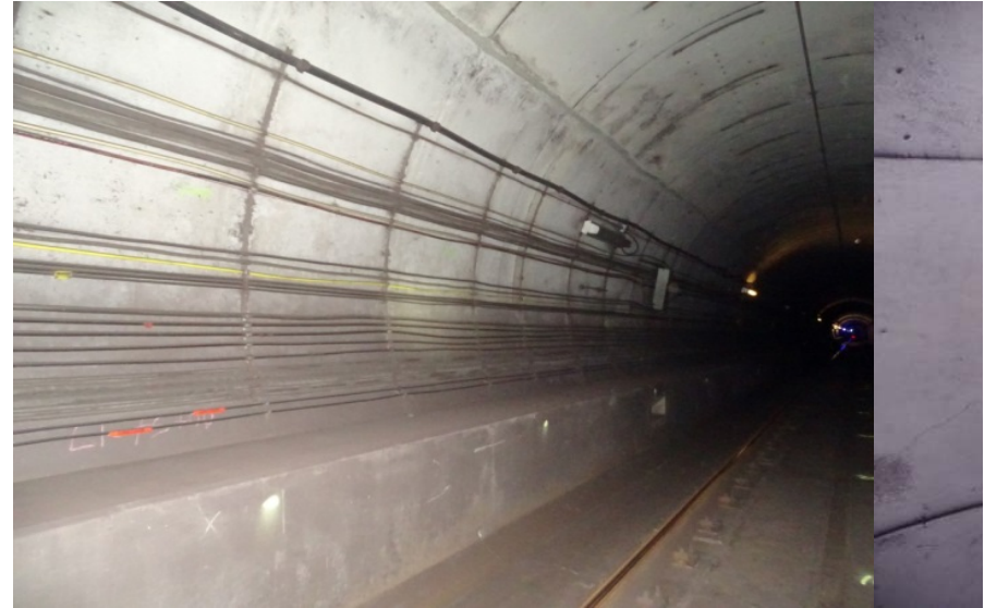
Photograph No. 206 Station 75+00, east wall.
