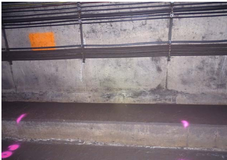
Photograph No. 273 Station 73+90, lower portion of west wall.
