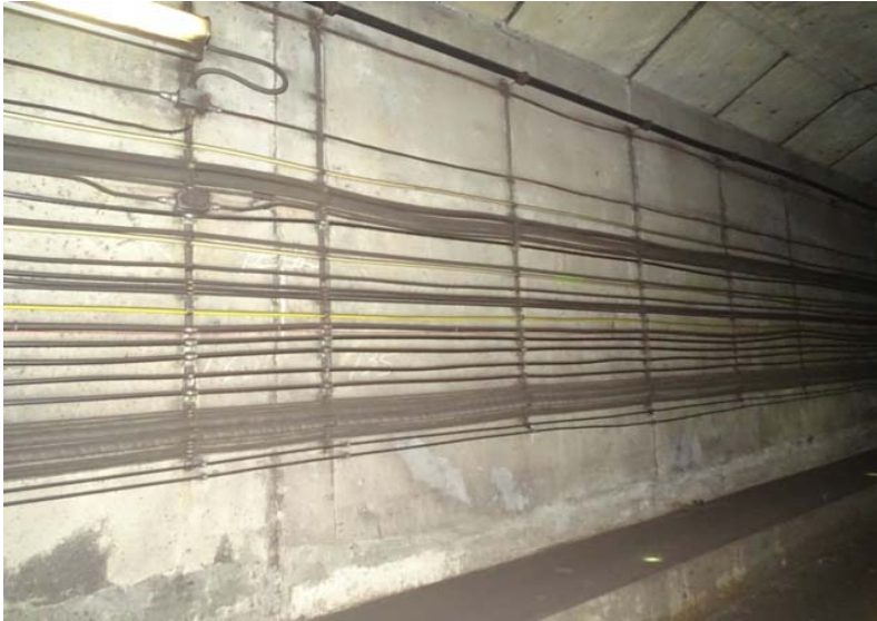
Photograph No. 137 Station 73+20, east wall.
