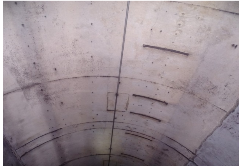
Photograph No. 520 Station 77+50, ceiling.
