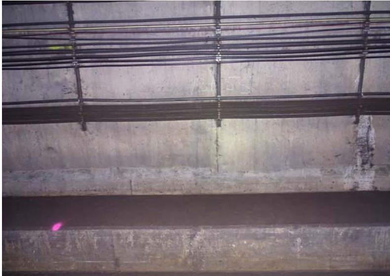
Photograph No. 213 Station 73+00, lower portion of west wall.
