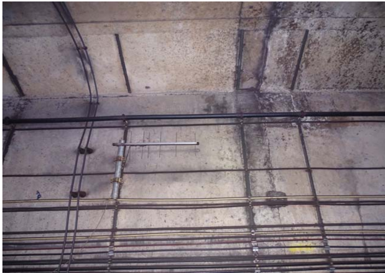
Photograph No. 129 Station 71+80, upper portion of west wall.
