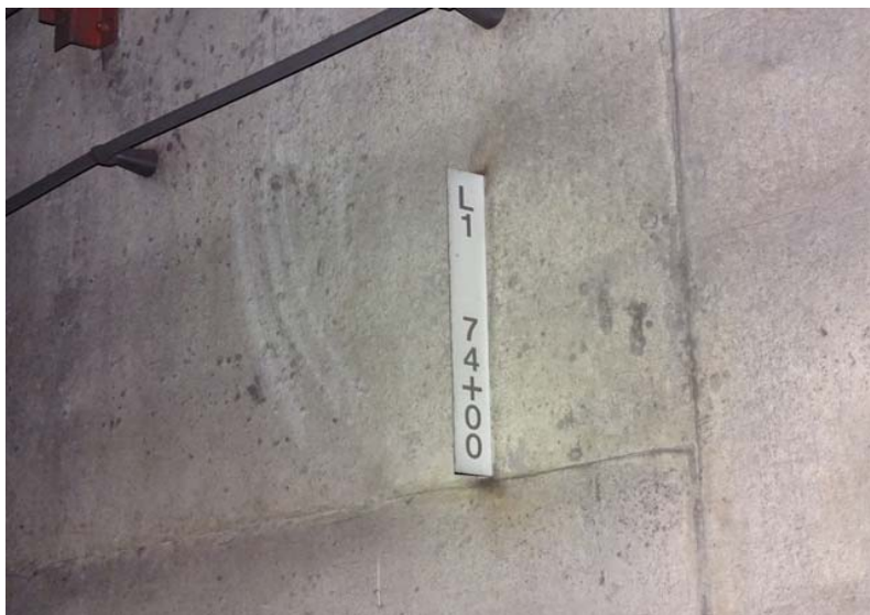
Photograph No. 127 Station 73+00 - marker for L1 74+00.
