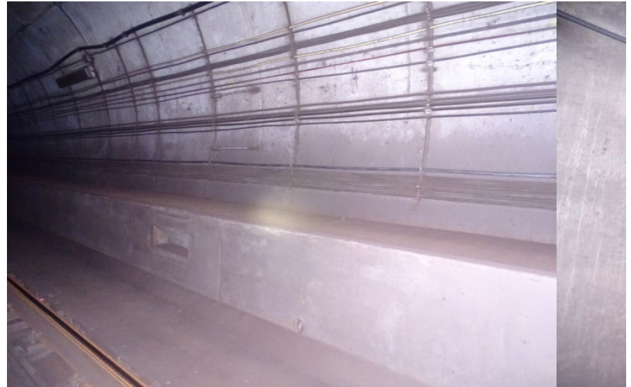
Photograph No. 516 Station 77+40, lower portion of west wall.
