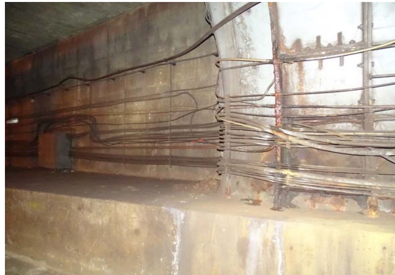
Photograph No. 40 Station 70+40, west wall.
