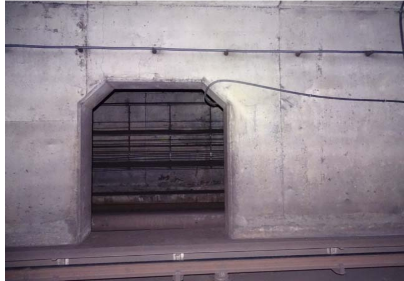
Photograph No. 190 Station 72+70, east wall.
