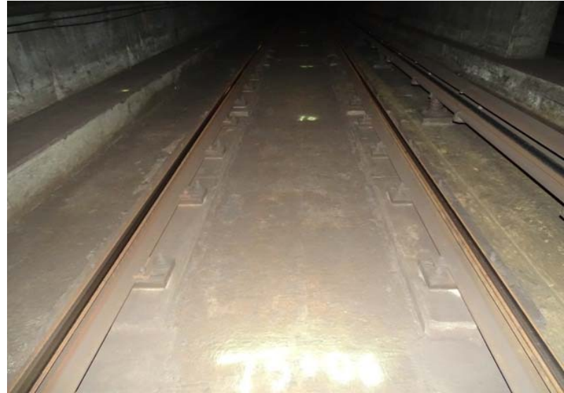
Photograph No. 82 Station 72+00, track bed.
