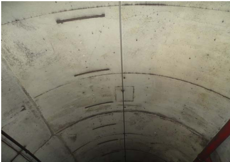
Photograph No. 199 Station 74+80, ceiling.
