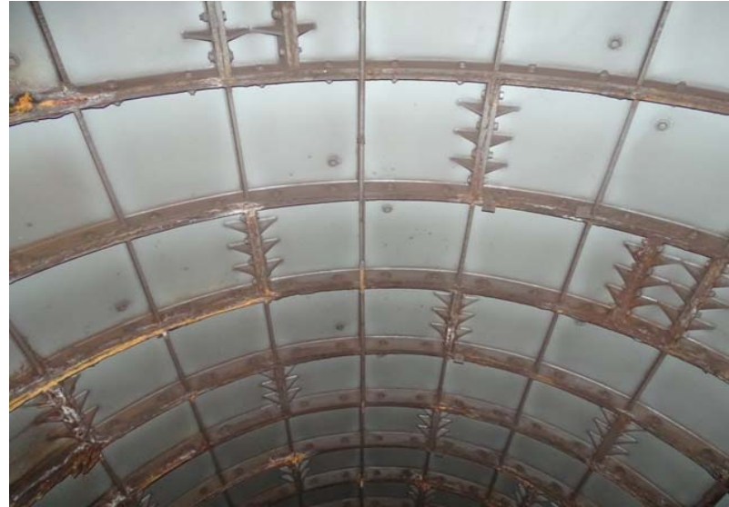
Photograph No. 22 Station 70+10, ceiling.
