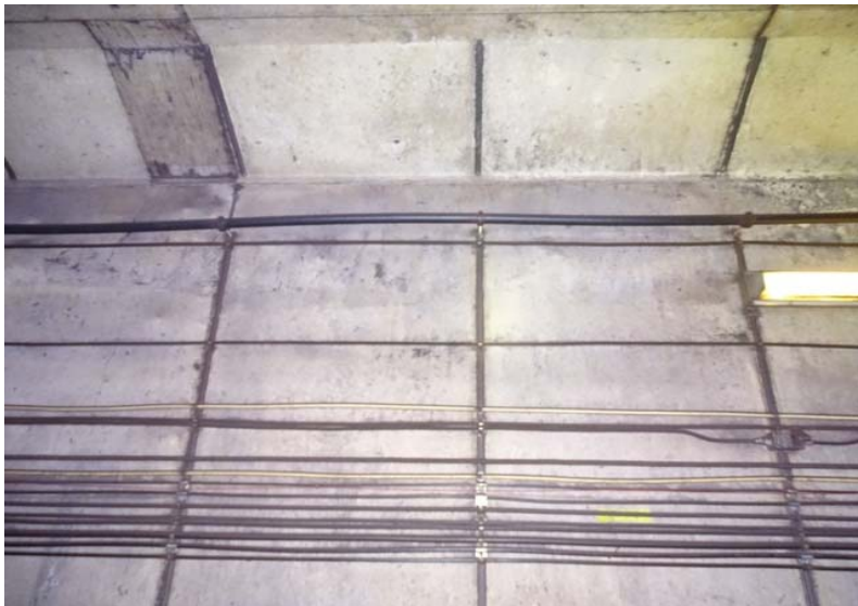
Photograph No. 179 Station 72+50, upper portion of west wall.
