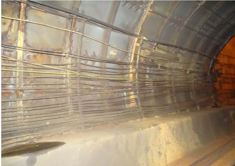
Photograph No. 25 Station 70+20, east wall.
