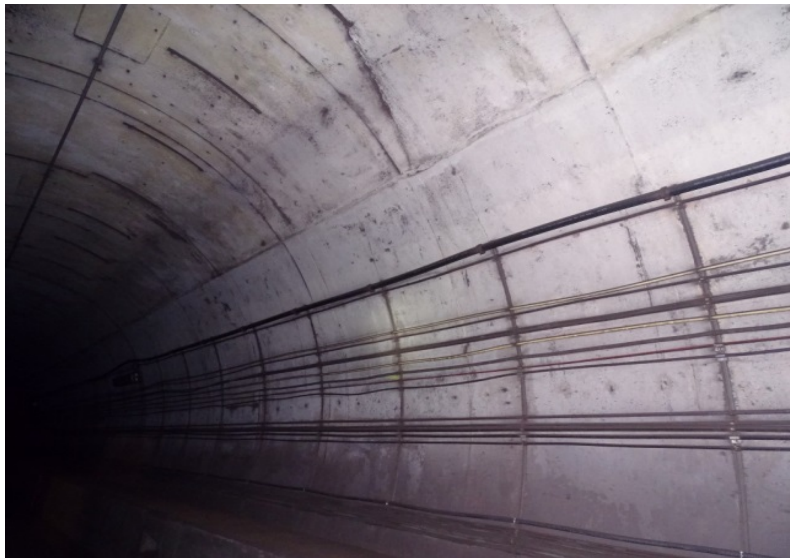
Photograph No. 567 Station 78+50, upper portion of west wall.
