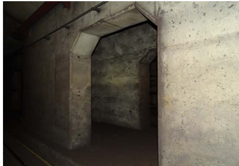
Photograph No. 28 Storage area, section 3, looking south.
