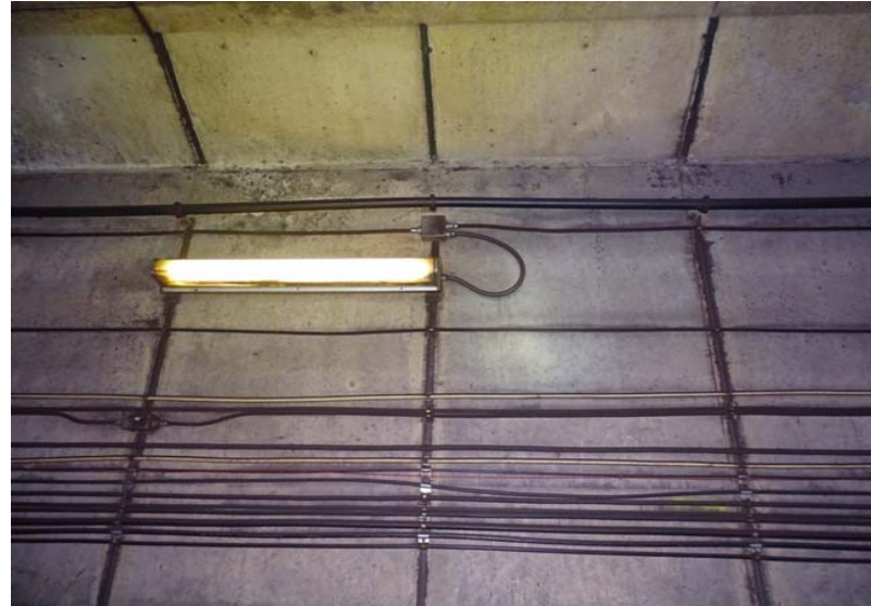
Photograph No. 174 Station 72+40, upper portion of west wall.
