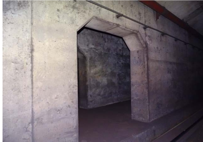
Photograph No. 22 Storage area, section 3, looking north toward arch 3.
