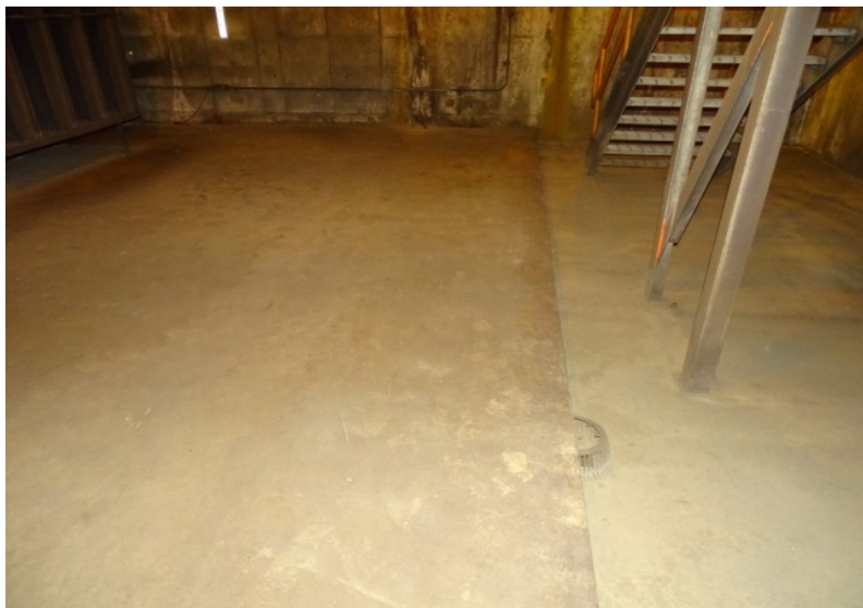
Photograph No. 177 Upper fan room floor, south section, center portion.
