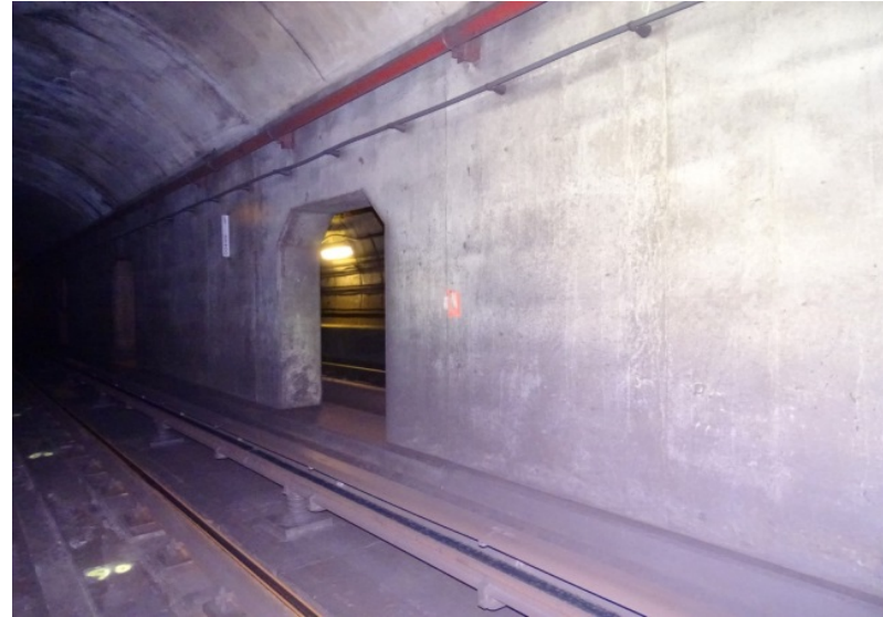
Photograph No. 290 Station 76+80, west wall.
