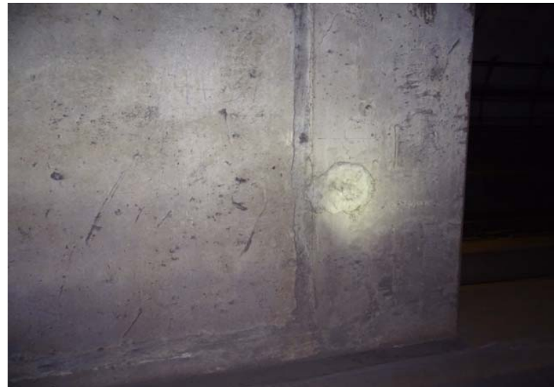
Photograph No. 296 Station 74+30 - previous concrete repair on east wall.
