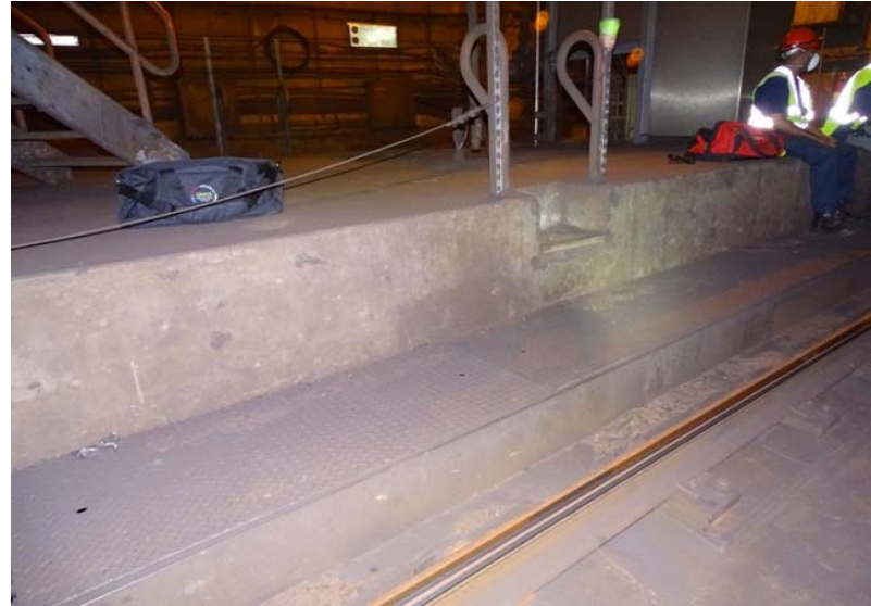
Photograph No. 50 Station 70+60, east wall.
