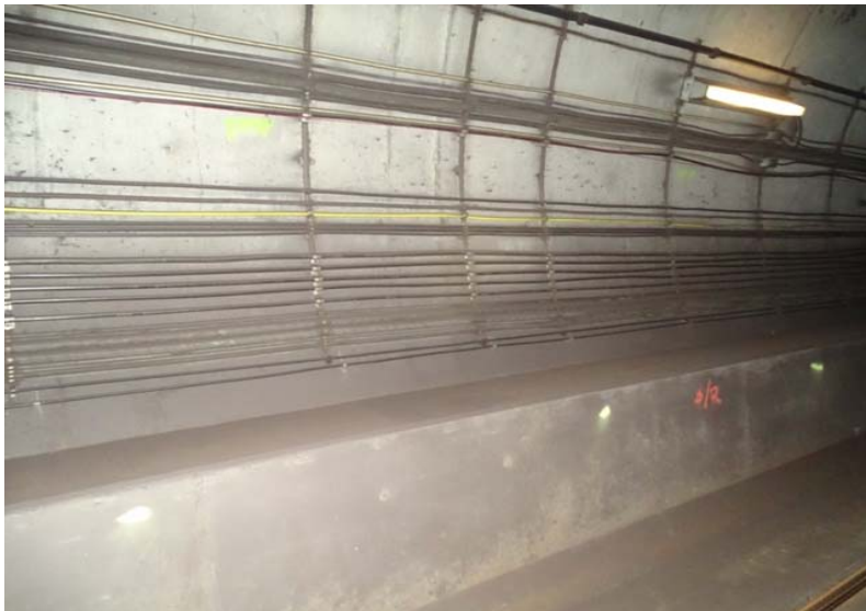
Photograph No. 191 Station 74+60, east wall.
