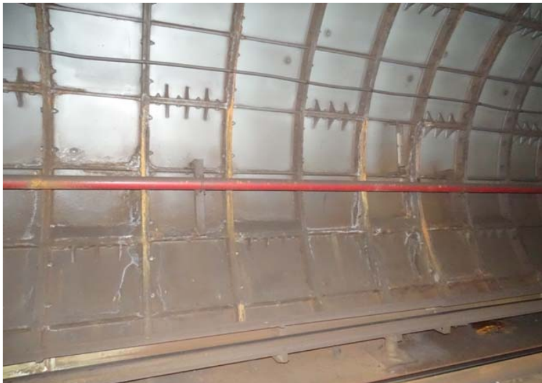
Photograph No. 11 Station 69+90, east wall.
