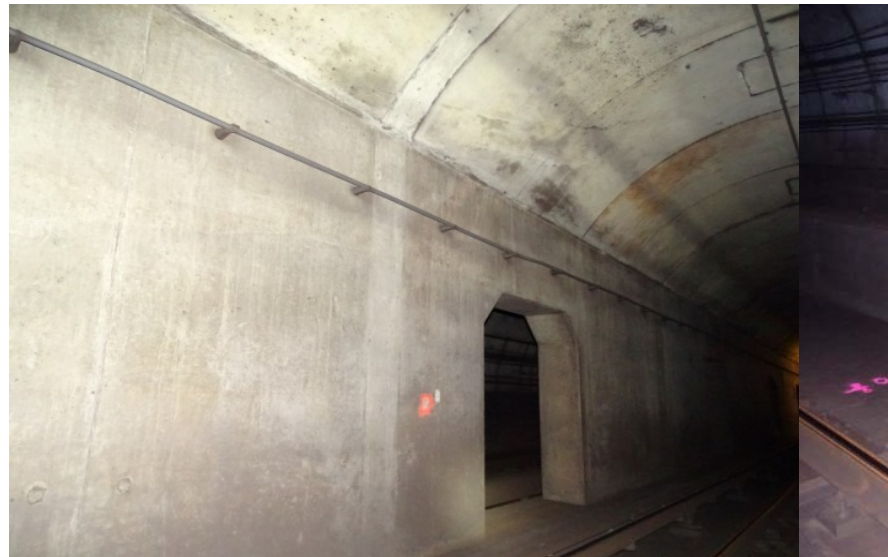
Photograph No. 446 Station 76+30, east wall.
