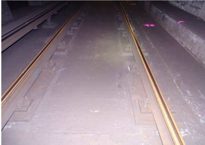
Photograph No. 233 Station 73+30, track bed.
