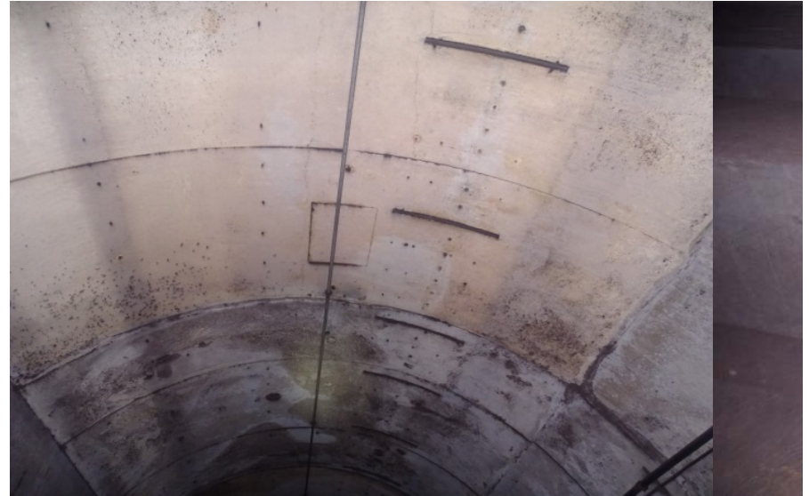
Photograph No. 534 Station 77+70, ceiling.
