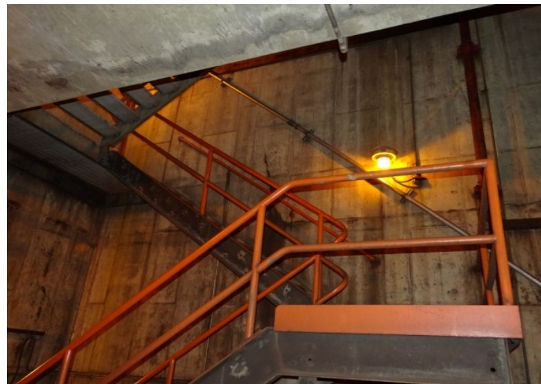
Photograph No. 162 Upper fan room, west wall, south section, middle portion.
