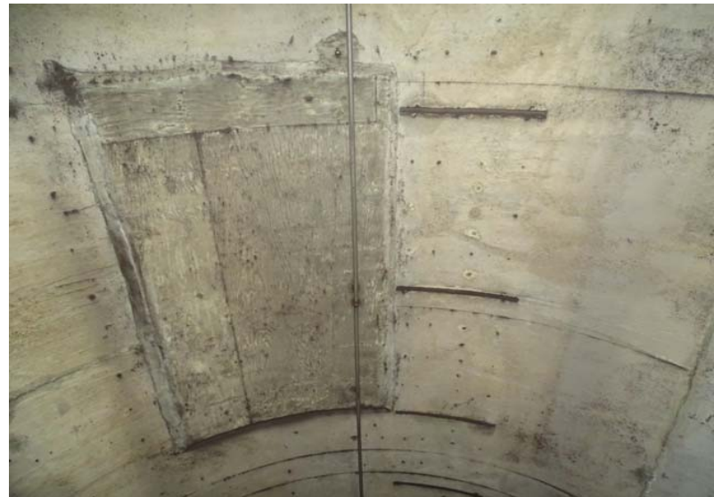
Photograph No. 320 Station 74+60, ceiling.
