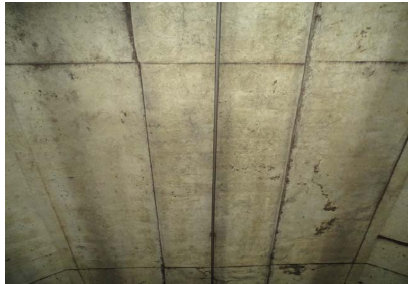
Photograph No. 192 Station 72+70, ceiling.
