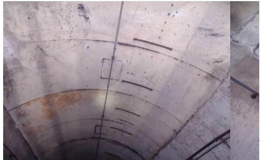
Photograph No. 452 Station 76+40, ceiling.
