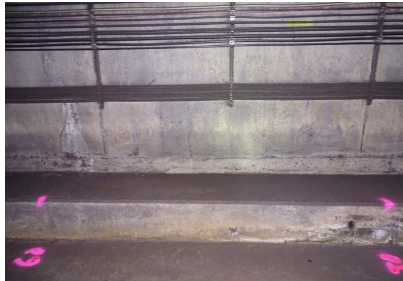
Photograph No. 180 Station 72+50, lower portion of west wall.
