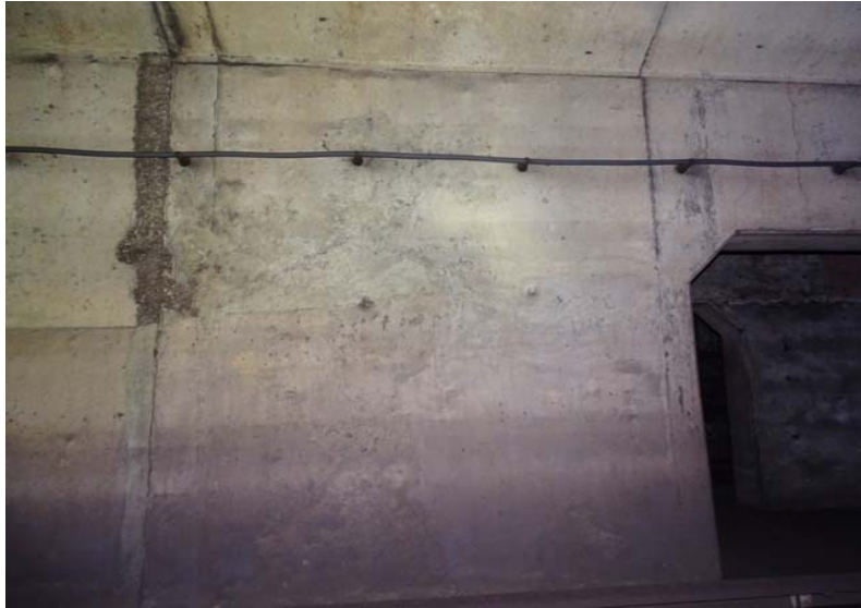
Photograph No. 93 Station 71+30, east wall.
