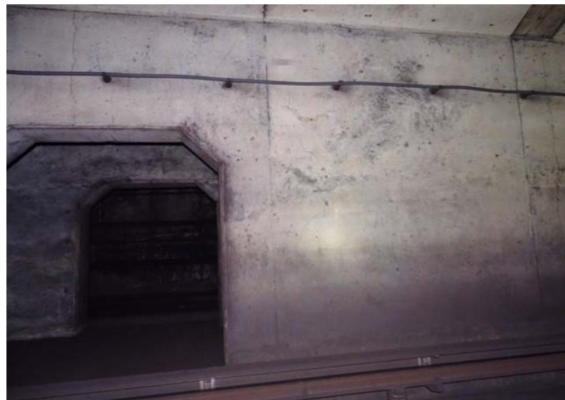
Photograph No. 100 Station 71+40, east wall.
