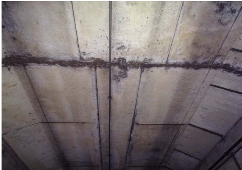
Photograph No. 259 Station 73+70, ceiling.
