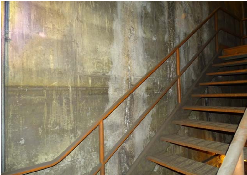
Photograph No. 83 Main room, west wall at the stair.
