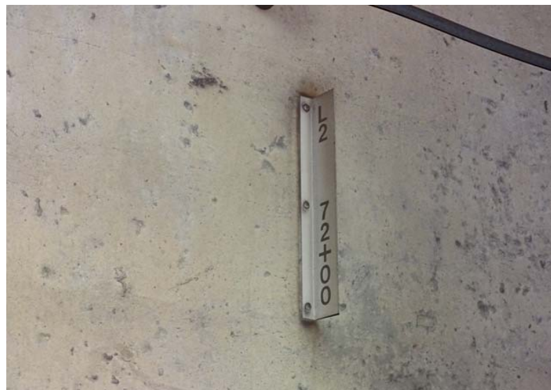
Photograph No. 140 Station 72+00 - marker for L2 72+00.
