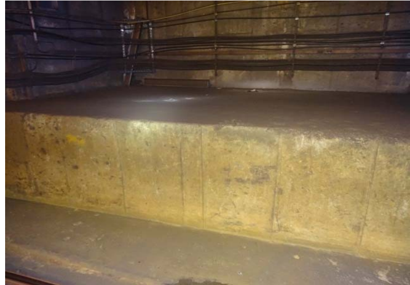
Photograph No. 66 Station 70+80, lower portion of west wall.
