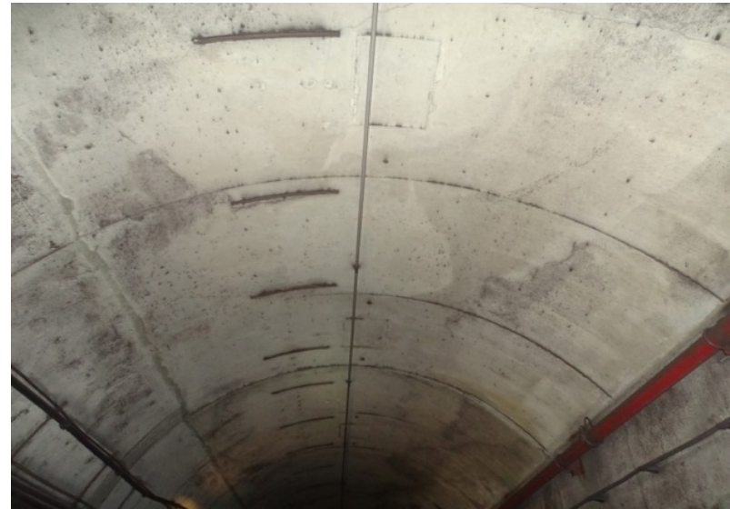
Photograph No. 358 Station 78+60, ceiling.
