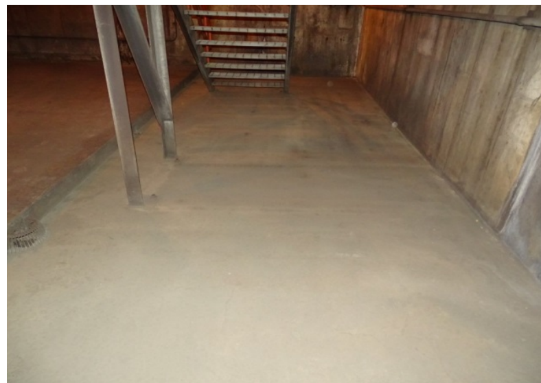
Photograph No. 176 Upper fan room floor, south section, west end.
