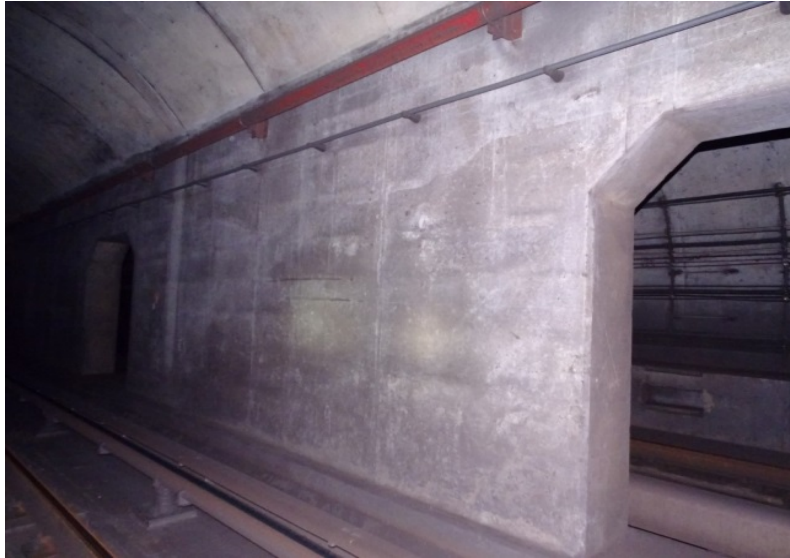
Photograph No. 257 Station 76+20, west wall.
