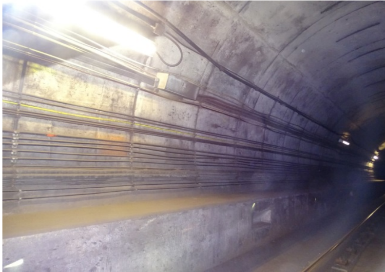
Photograph No. 349 Station 78+40, east wall.
