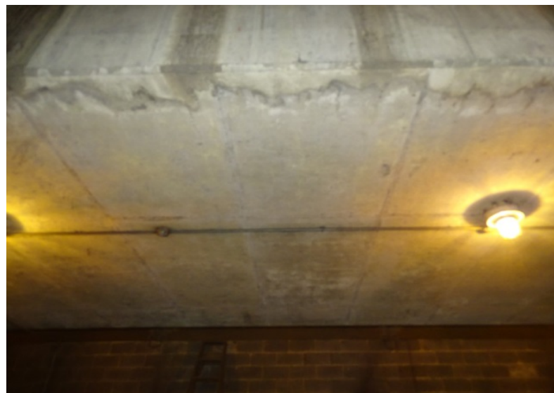
Photograph No. 144 Upper fan room, east wall, north-center section, middle-lower portion.
