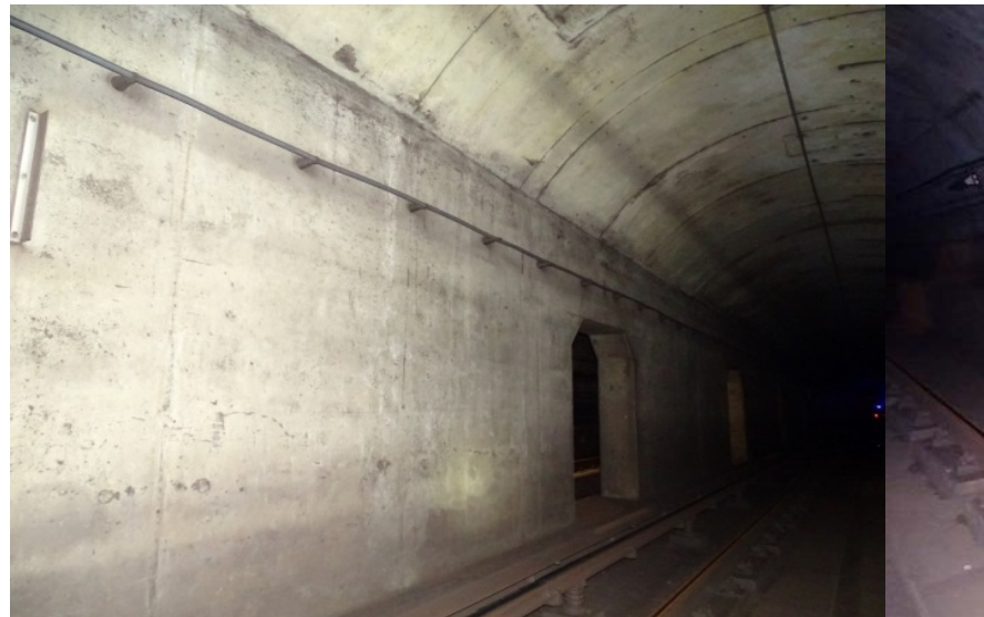
Photograph No. 546 Station 78+00, east wall.
