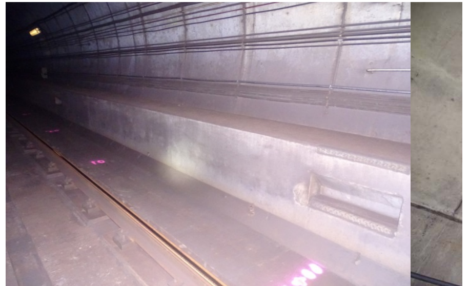
Photograph No. 424 Station 76+00, lower portion of west wall.
