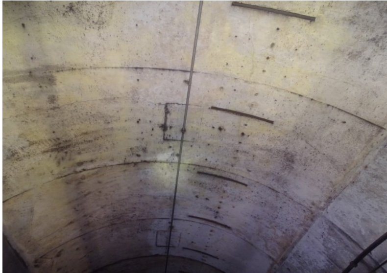
Photograph No. 393 Station 75+60, ceiling.
