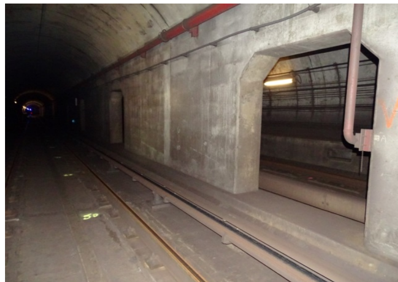
Photograph No. 224 Station 75+40, west wall.
