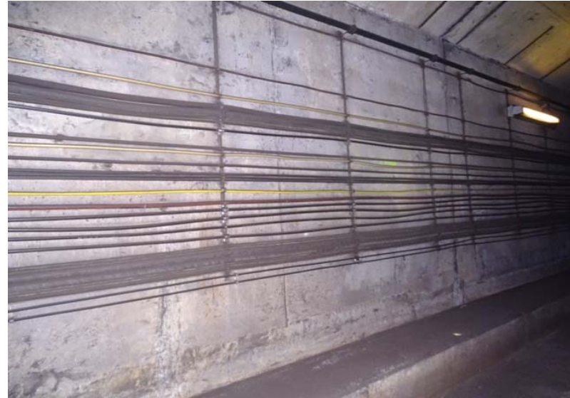
Photograph No. 110 Station 72+60, east wall.
