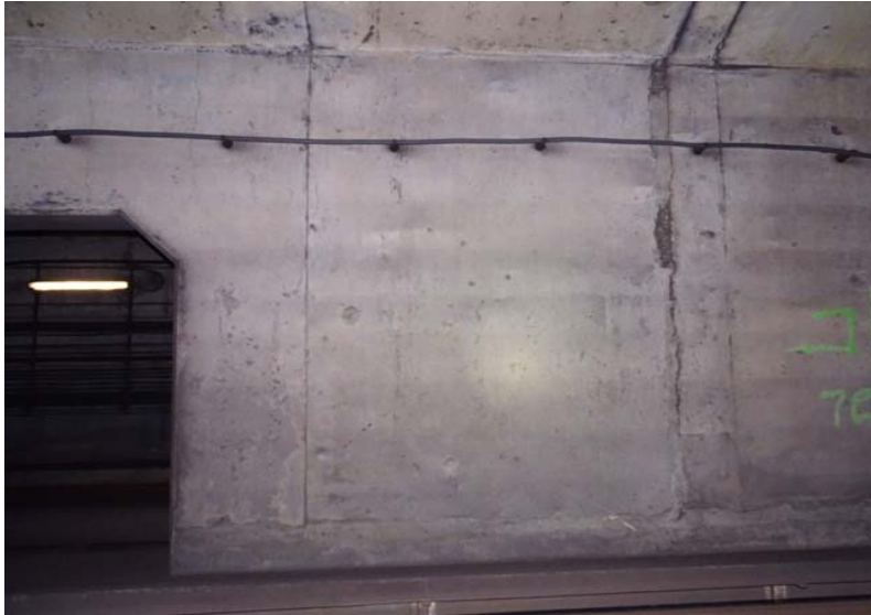
Photograph No. 157 Station 72+20, east wall.
