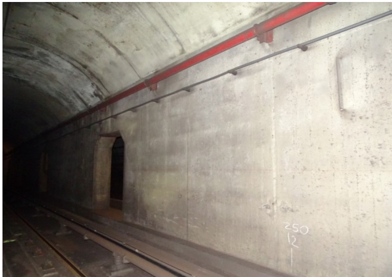
Photograph No. 299 Station 77+00, west wall.
