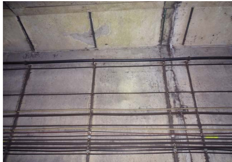
Photograph No. 168 Station 72+30, upper portion of west wall.
