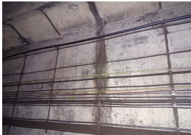
Photograph No. 242 Station 73+40, upper portion of west wall.
