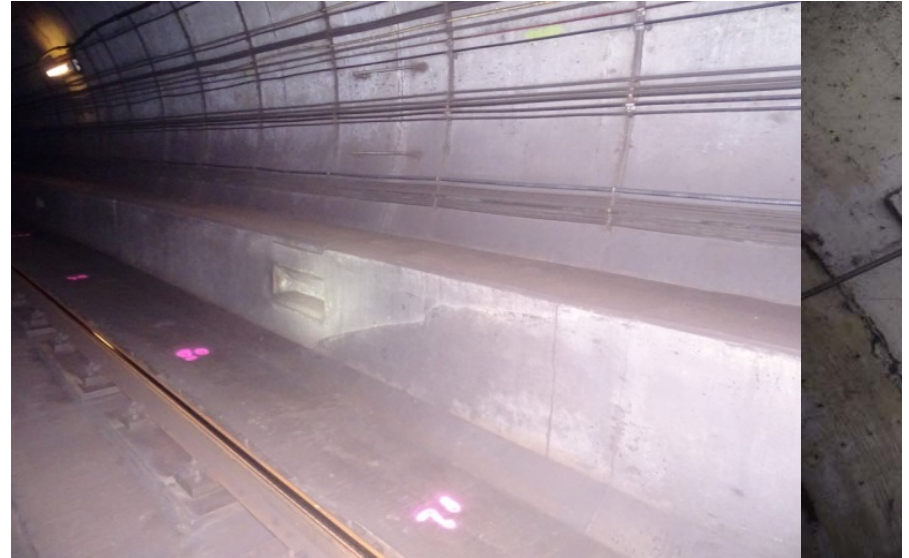
Photograph No. 402 Station 75+70, lower portion of west wall.
