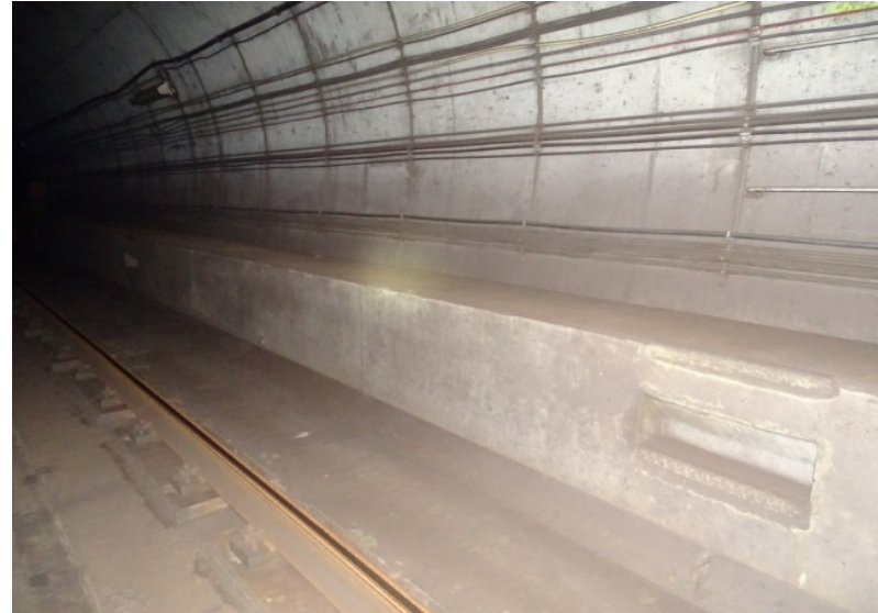
Photograph No. 562 Station 78+40, lower portion of west wall.
