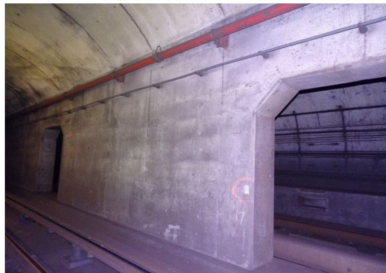
Photograph No. 344 Station 78+20, west wall.
