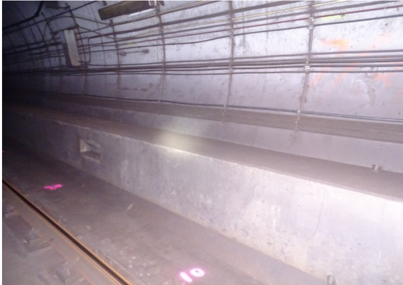
Photograph No. 361 Station 75+10, lower portion of west wall.
