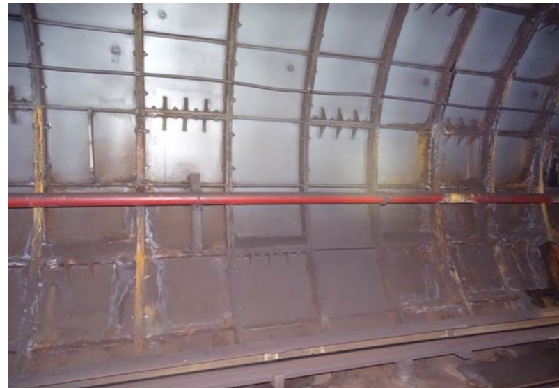
Photograph No. 16 Station 70+00, east wall.
