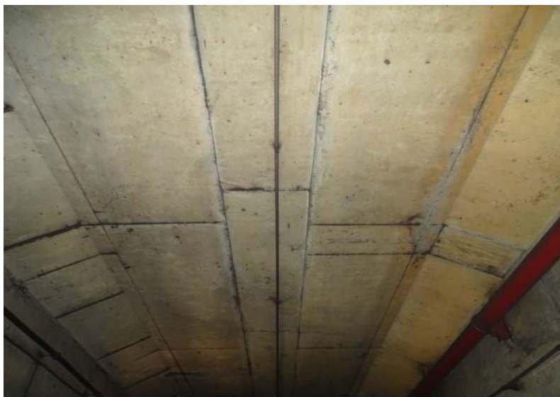
Photograph No. 147 Station 73+40, ceiling.
