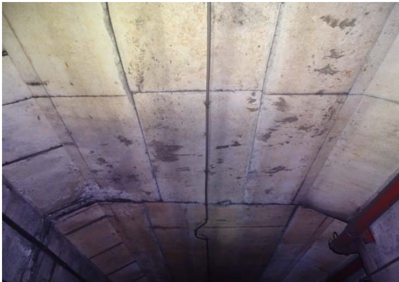
Photograph No. 67 Station 71+60, ceiling.
