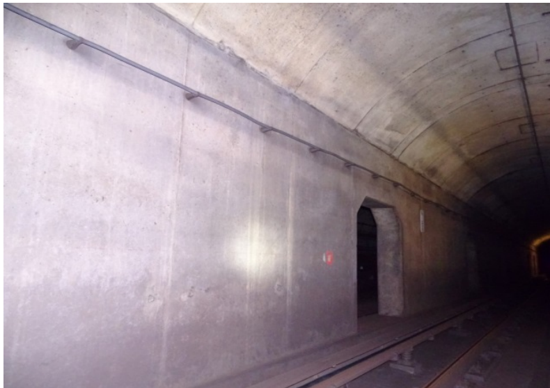
Photograph No. 407 Station 75+80, east wall.
