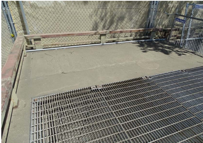
Photograph No. 193 Vent shaft exterior, north end of deck.
