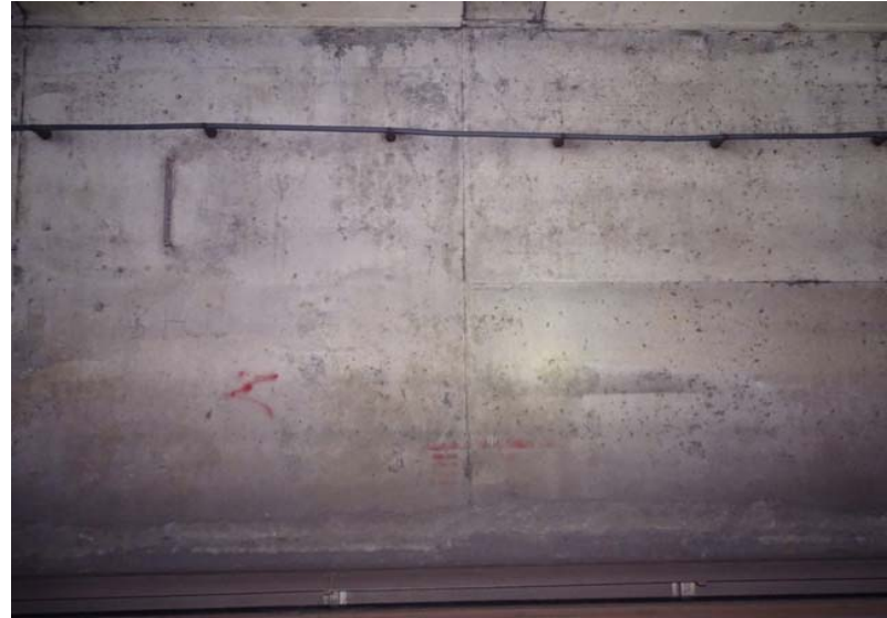
Photograph No. 210 Station 73+00, east wall.
