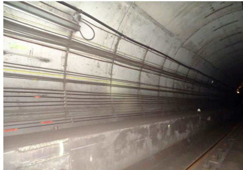
Photograph No. 248 Station 76+00, east wall.
