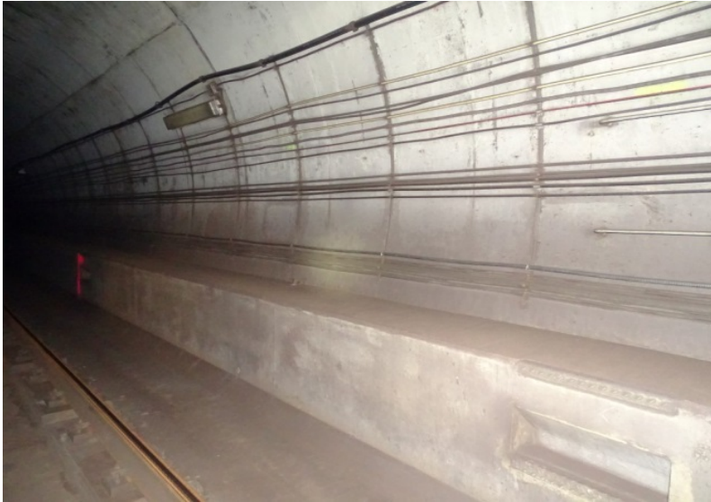
Photograph No. 573 Station 79+00, lower portion of west wall.
