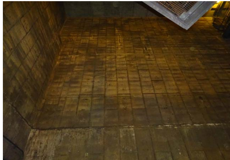
Photograph No. 60 Main room, looking up at east wall.
