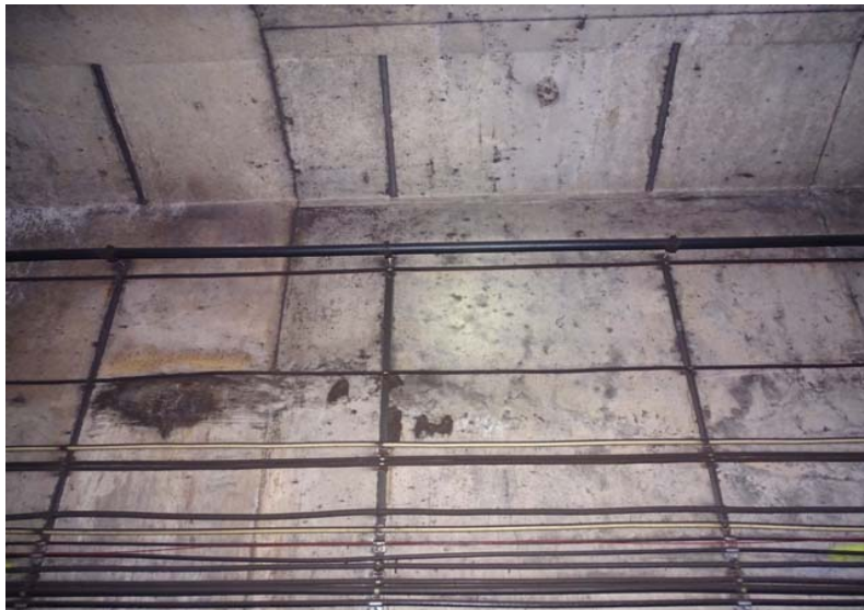
Photograph No. 291 Station 74+20, upper portion of west wall.
