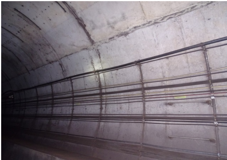
Photograph No. 459 Station 76+50, upper portion of west wall.
