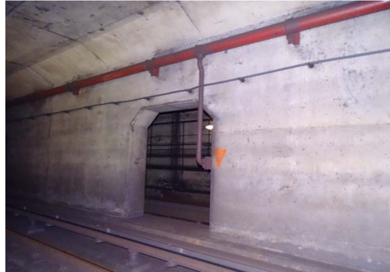
Photograph No. 134 Station 73+00, west wall.
