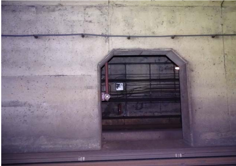
Photograph No. 217 Station 73+10, east wall.
