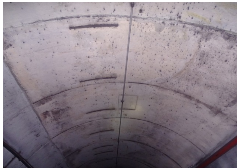
Photograph No. 316 Station 77+40, ceiling.
