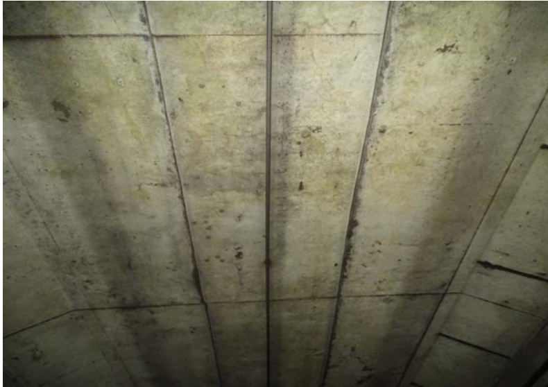
Photograph No. 185 Station 72+60, ceiling.
