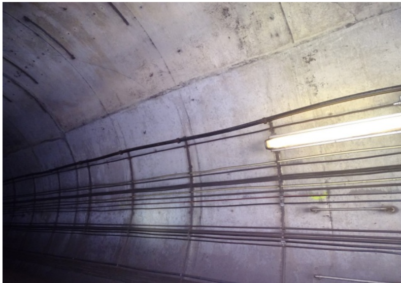
Photograph No. 423 Station 76+00, upper portion of west wall.
