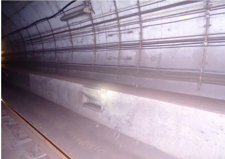
Photograph No. 473 Station 76+70, lower portion of west wall.
