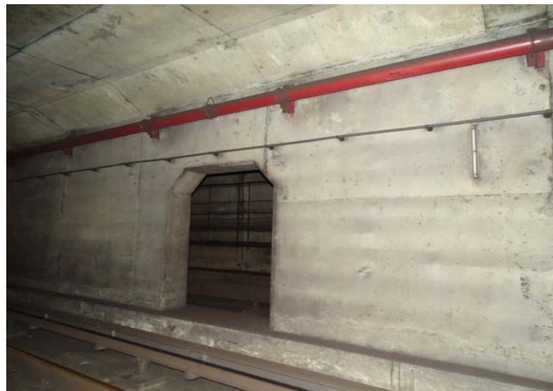
Photograph No. 88 Station 72+00, west wall.
