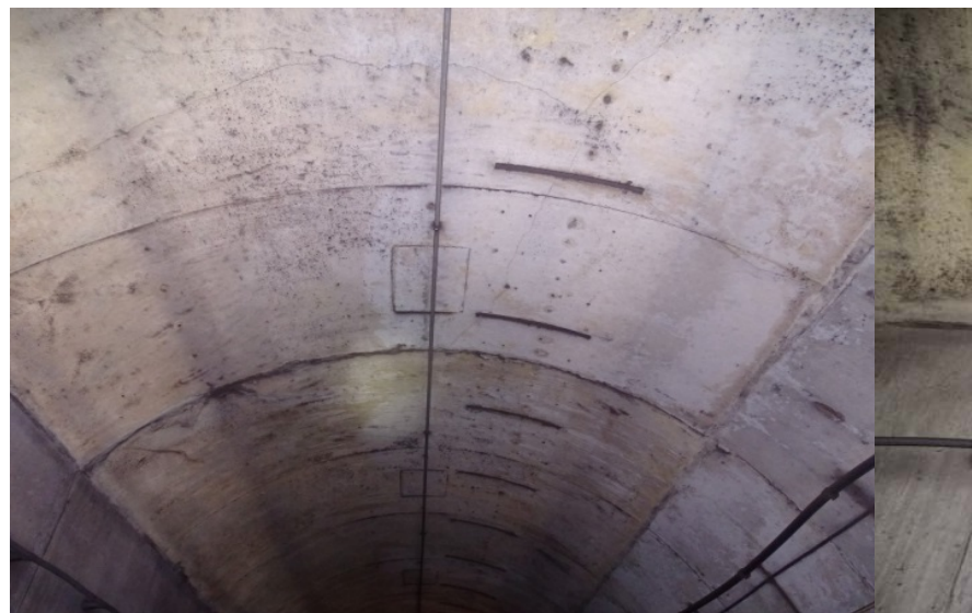
Photograph No. 400 Station 75+70, ceiling.
