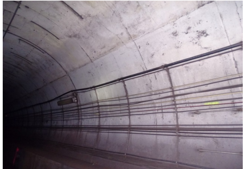
Photograph No. 572 Station 79+00, upper portion of west wall.
