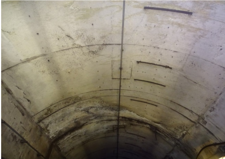
Photograph No. 497 Station 77+10, ceiling.
