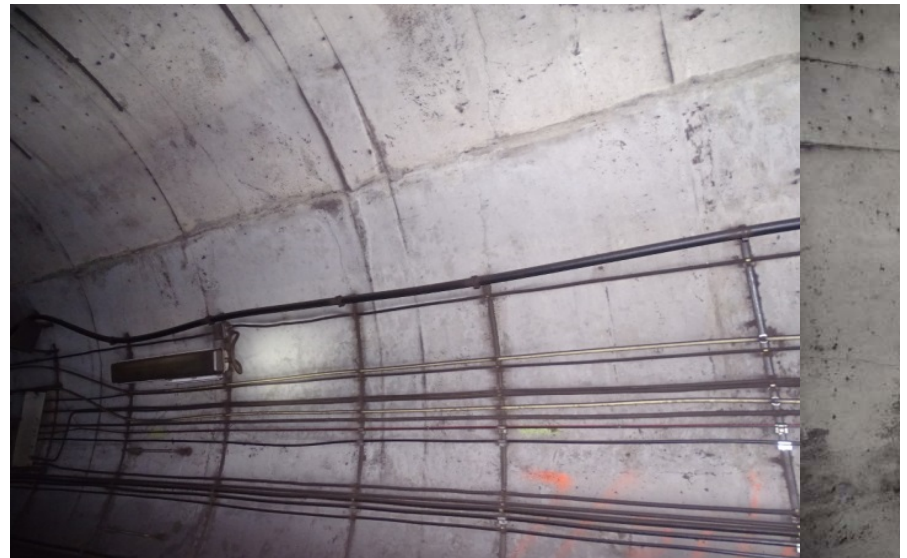
Photograph No. 360 Station 75+10, upper portion of west wall.
