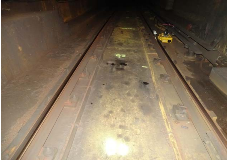
Photograph No. 37 Station 70+80, track bed.
