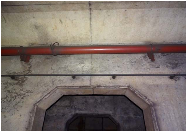
Photograph No. 47 Station 70+80 - construction joint above west arch.
