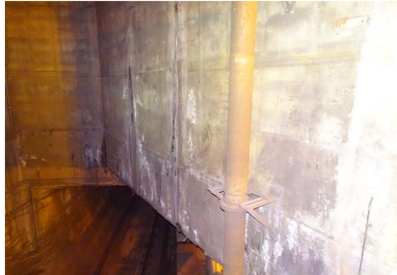
Photograph No. 72 Main room, west wall.
