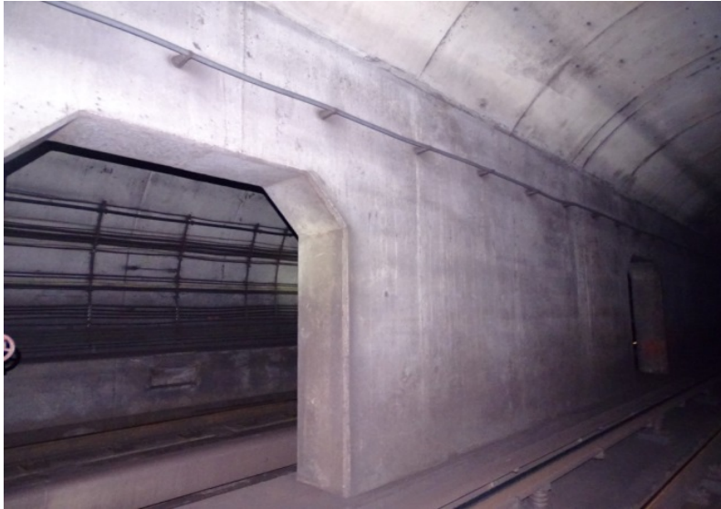
Photograph No. 513 Station 77+40, east wall.
