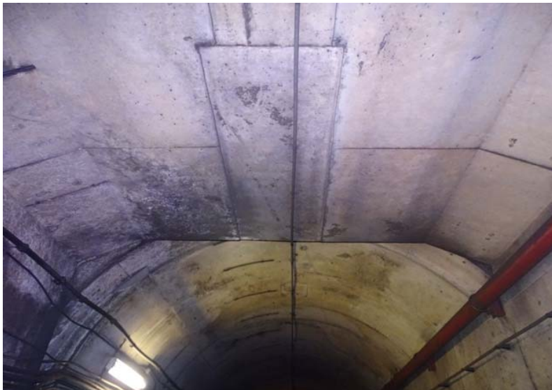
Photograph No. 175 Station 74+20, ceiling.
