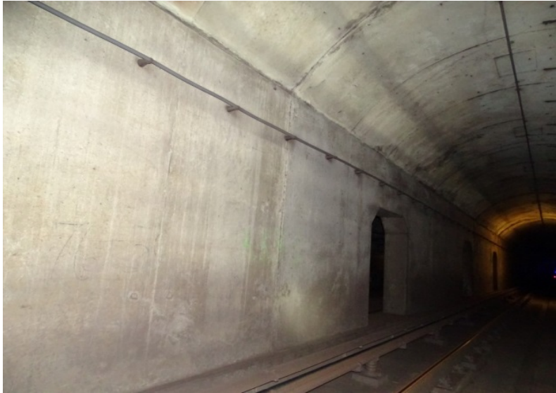
Photograph No. 457 Station 76+50, east wall.
