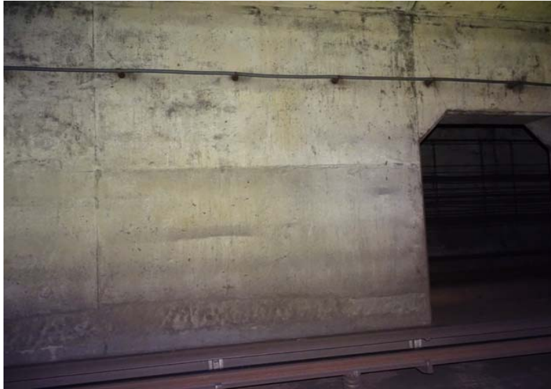
Photograph No. 245 Station 73+50, east wall.
