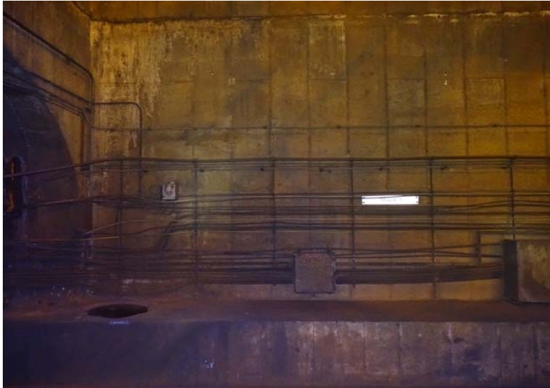
Photograph No. 61 Main room, lower north portion of east wall.
