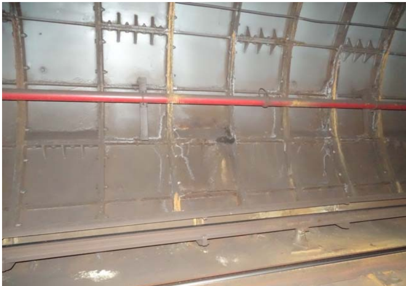
Photograph No. 7 Station 69+80, east wall.
