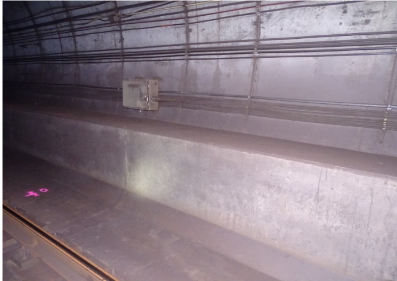
Photograph No. 449 Station 76+30, lower portion of west wall.
