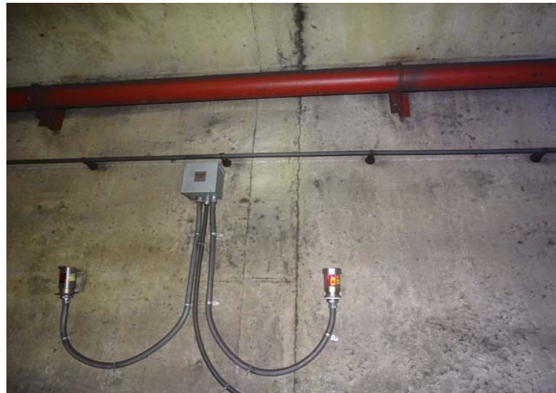
Photograph No. 118 Station 72+60 - crack on the west wall.
