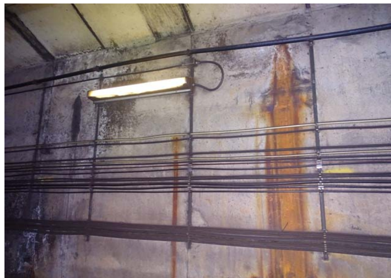
Photograph No. 88 Station 71+20, upper portion of west wall.
