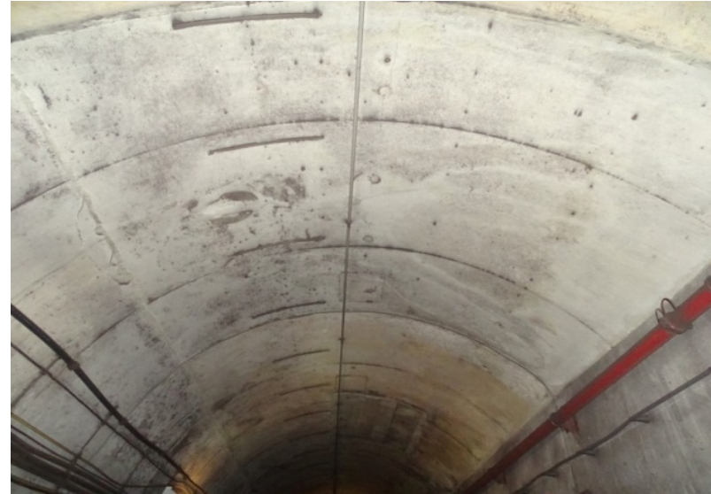
Photograph No. 330 Station 77+80, ceiling.
