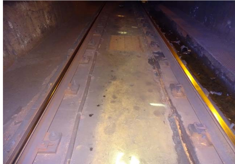
Photograph No. 34 Station 70+60, track bed.
