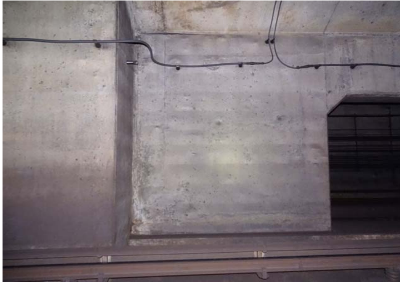
Photograph No. 125 Station 71+80, east wall.
