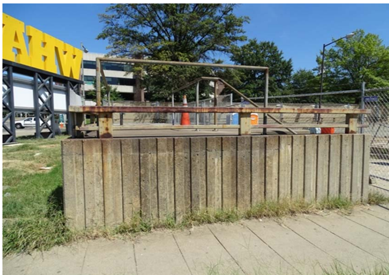
Photograph No. 179 Exterior of main vent shaft, south wall.
