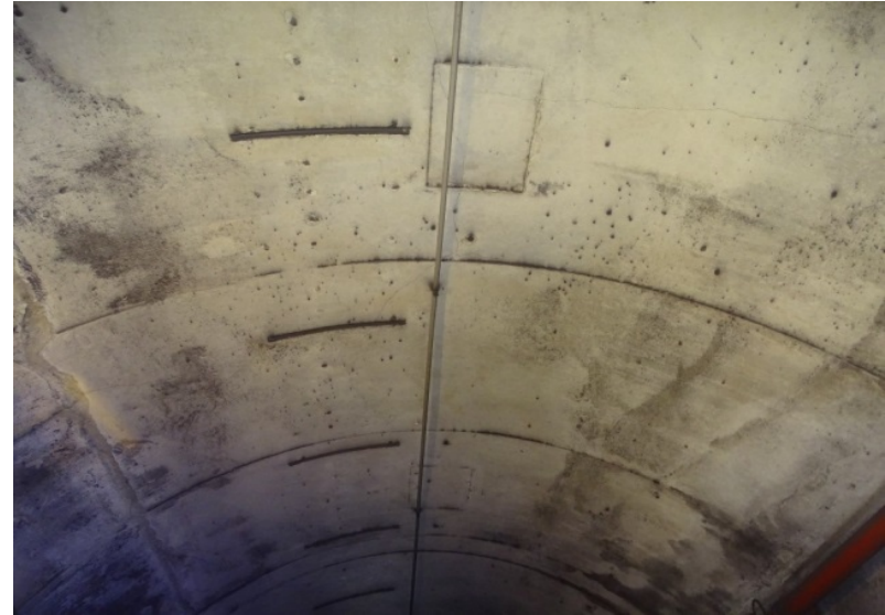
Photograph No. 350 Station 78+40, ceiling.
