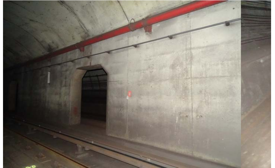
Photograph No. 202 Station 74+80, west wall.
