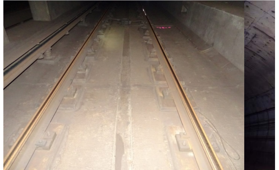
Photograph No. 538 Station 77+80, track bed.
