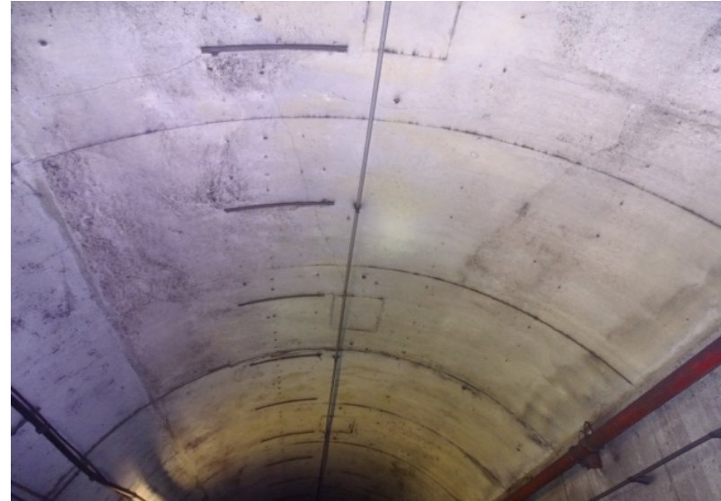
Photograph No. 374 Station 79+00, ceiling.
