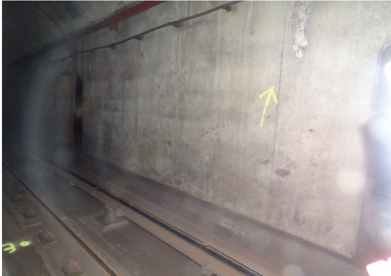
Photograph No. 309 Station 77+20, west wall.
