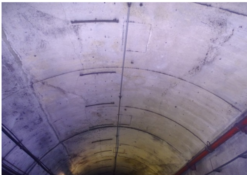
Photograph No. 343 Station 78+20, ceiling.
