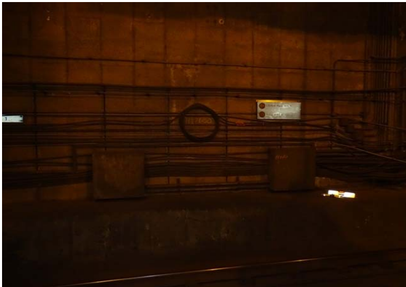
Photograph No. 63 Main room, lower south portion of east wall.
