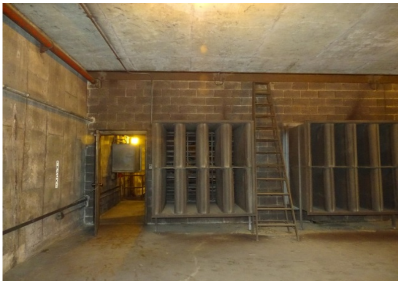
Photograph No. 141 Upper fan room, east wall, north end, lower portion.
