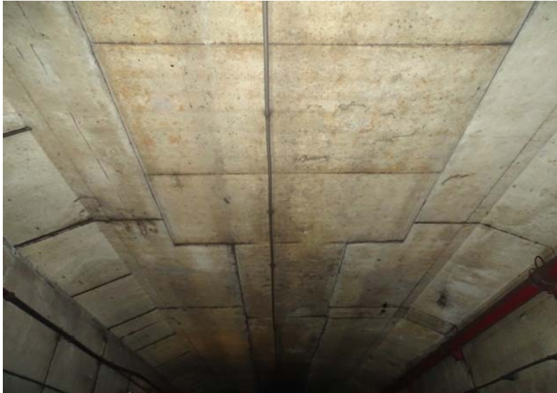
Photograph No. 77 Station 71+80, ceiling.
