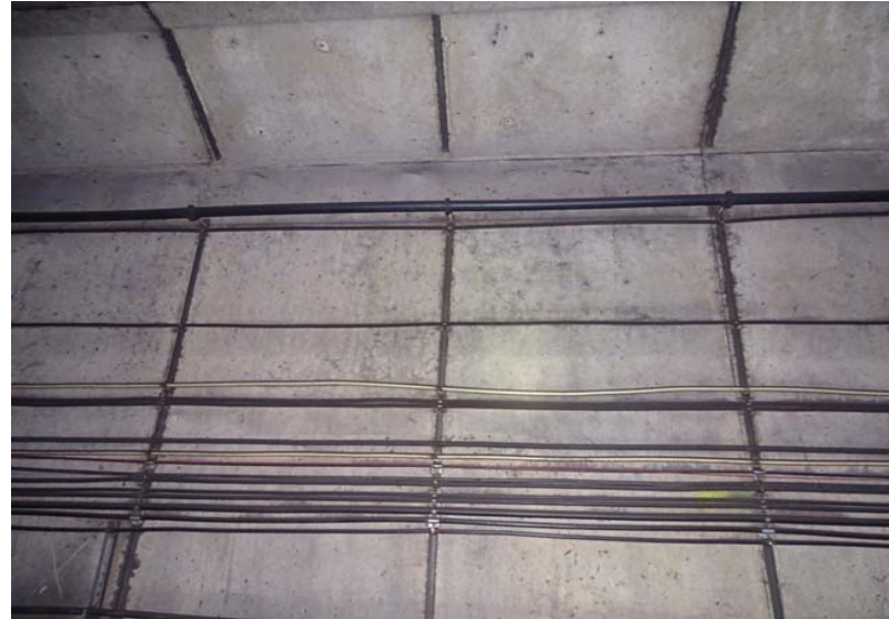
Photograph No. 206 Station 72+90, upper portion of west wall.
