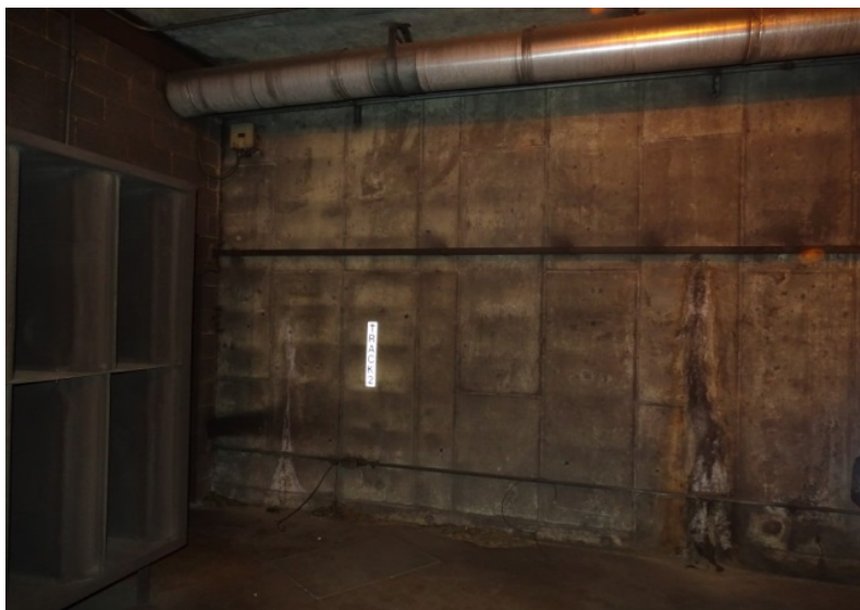
Photograph No. 155 Upper fan room, south wall, lower-east portion.
