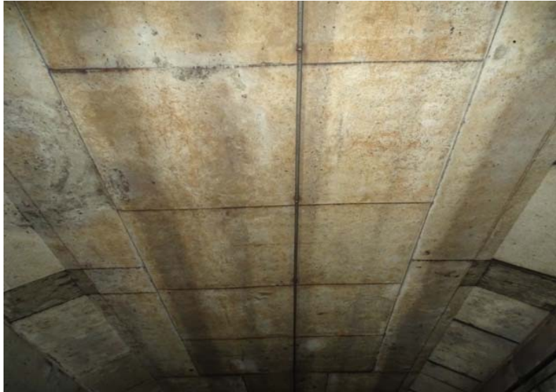
Photograph No. 141 Station 72+00, ceiling.
