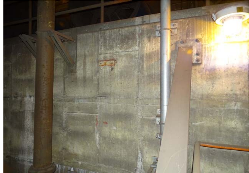
Photograph No. 98 Main room, upper portion, west wall at the stair.
