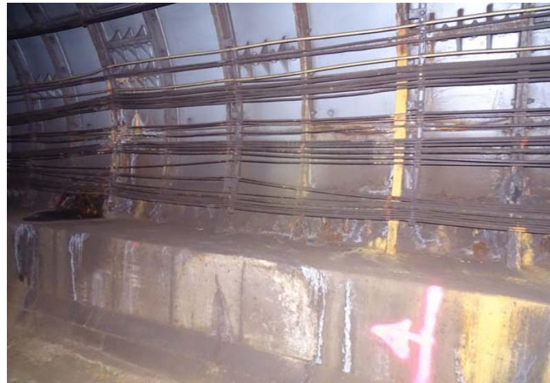
Photograph No. 4 Station 69+70, west wall.
