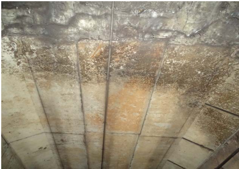
Photograph No. 75 Station 71+00, ceiling.
