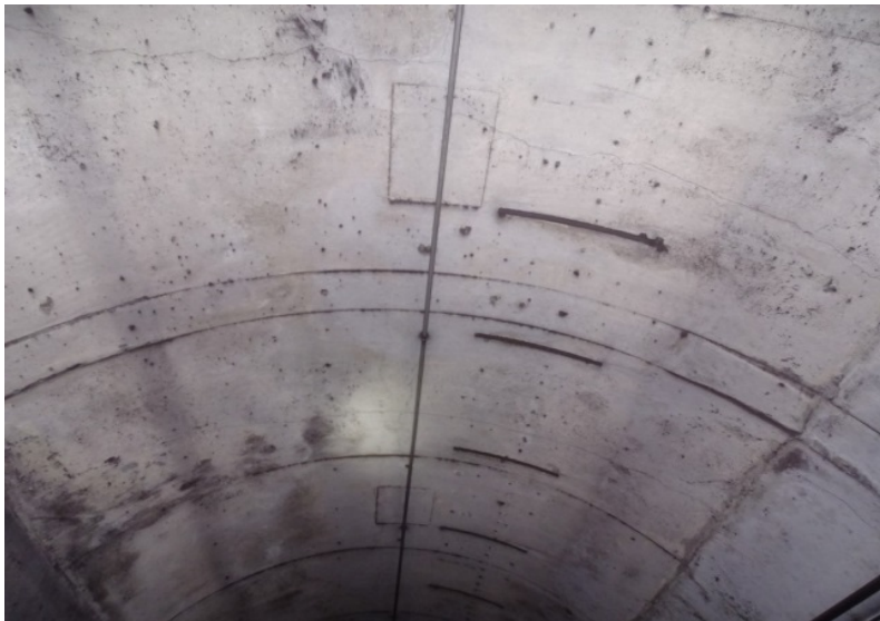
Photograph No. 359 Station 75+10, ceiling.
