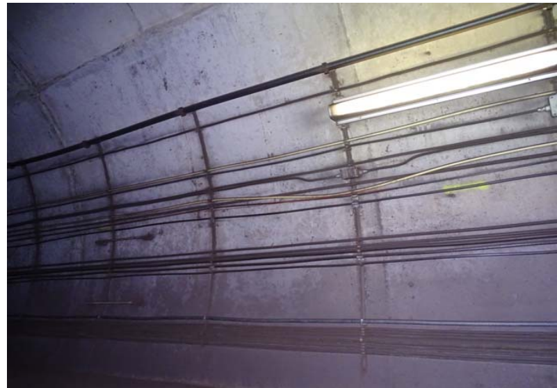
Photograph No. 336 Station 74+80, upper portion of west wall.
