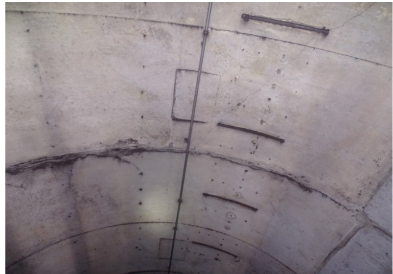
Photograph No. 432 Station 76+10, ceiling.
