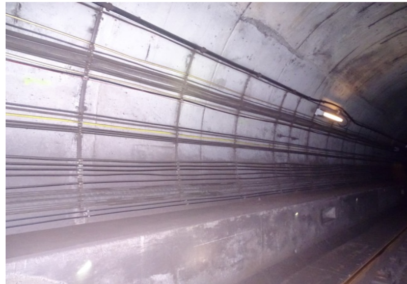
Photograph No. 276 Station 76+60, east wall.
