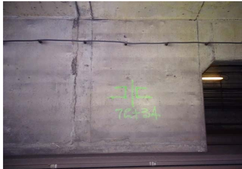
Photograph No. 164 Station 72+30, east wall.
