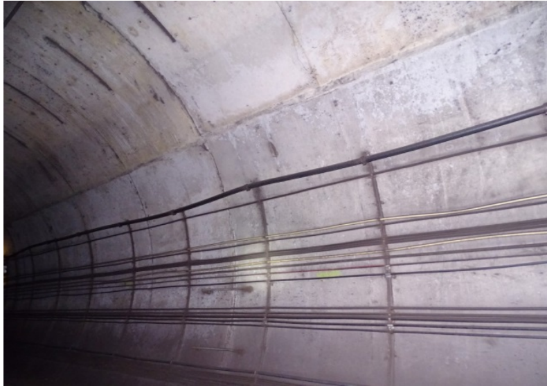
Photograph No. 401 Station 75+70, upper portion of west wall.
