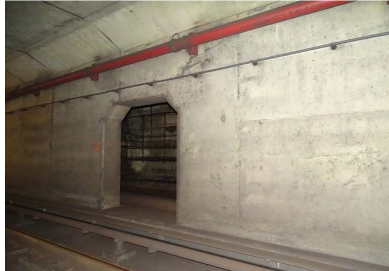
Photograph No. 170 Station 74+00, west wall.
