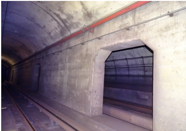
Photograph No. 351 Station 78+40, west wall.
