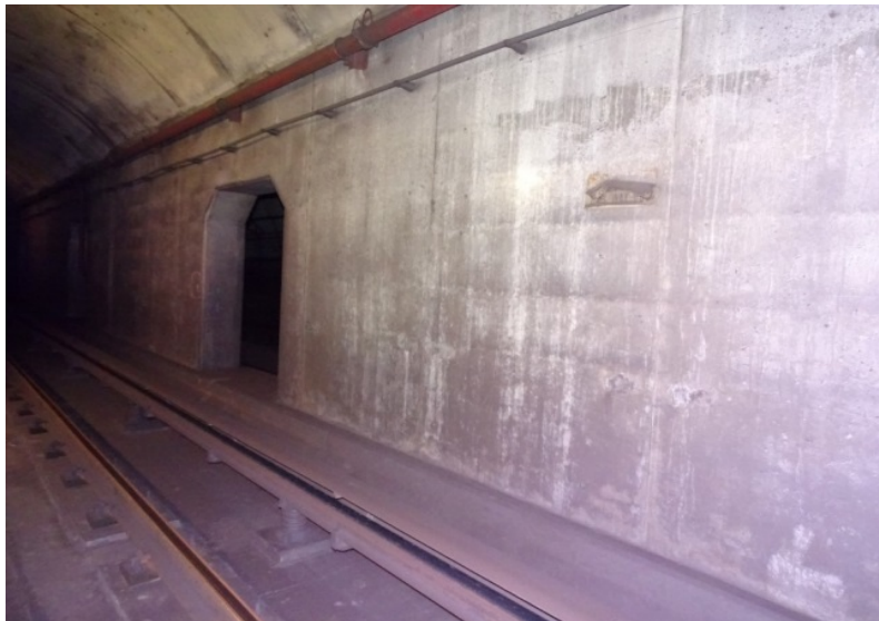
Photograph No. 375 Station 79+00, west wall.
