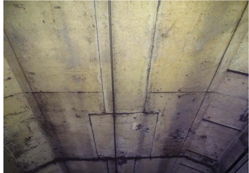
Photograph No. 254 Station 73+60, ceiling.
