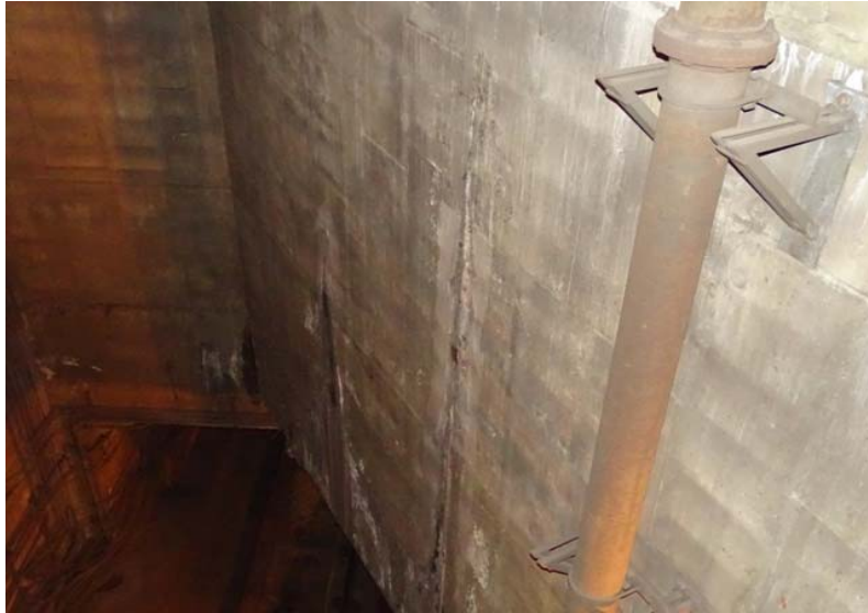
Photograph No. 97 Main room, upper portion, looking down at west wall.
