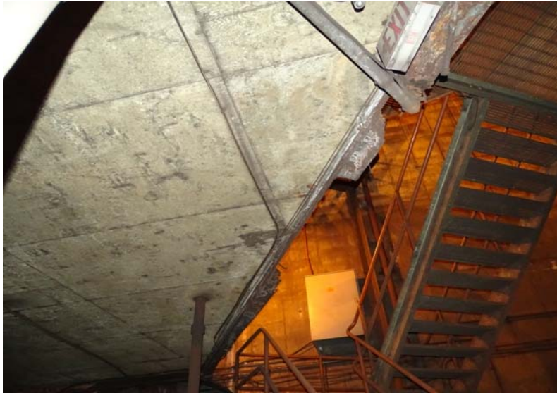
Photograph No. 49 Platform, ceiling, looking north.
