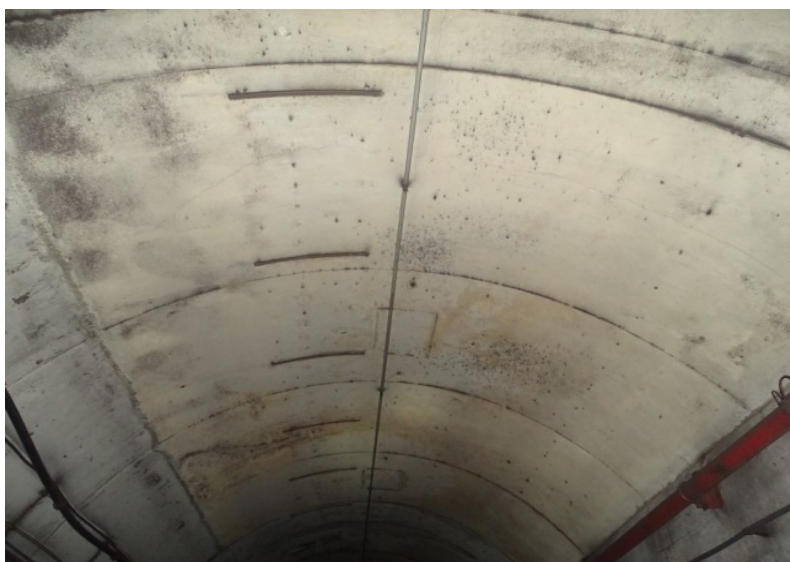
Photograph No. 323 Station 77+60, ceiling.
