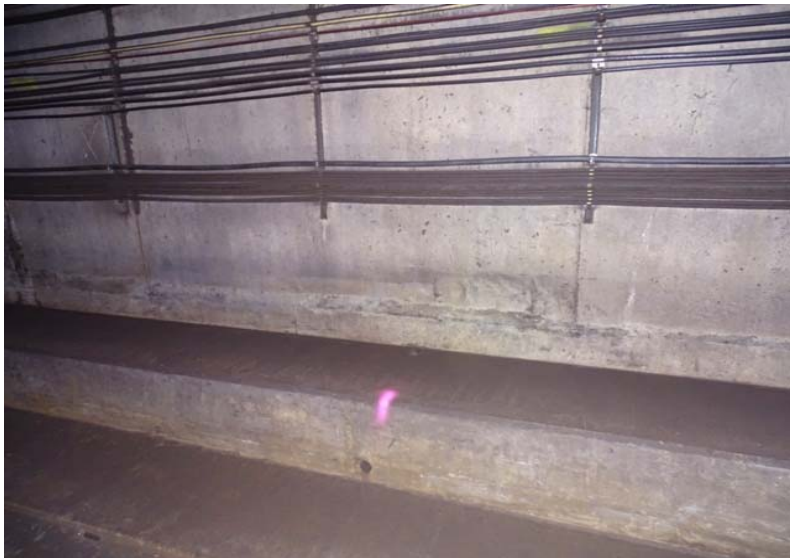
Photograph No. 207 Station 72+90, lower portion of west wall.
