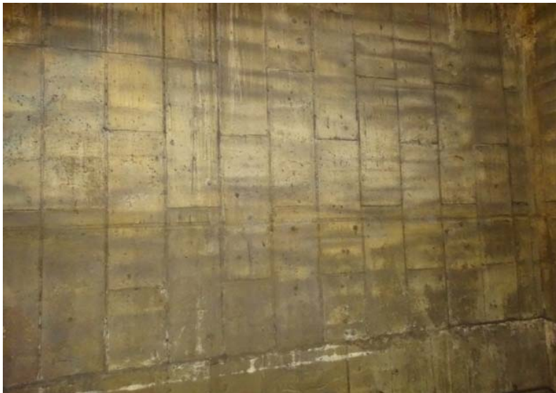
Photograph No. 67 Main room, east wall, middle south portion.
