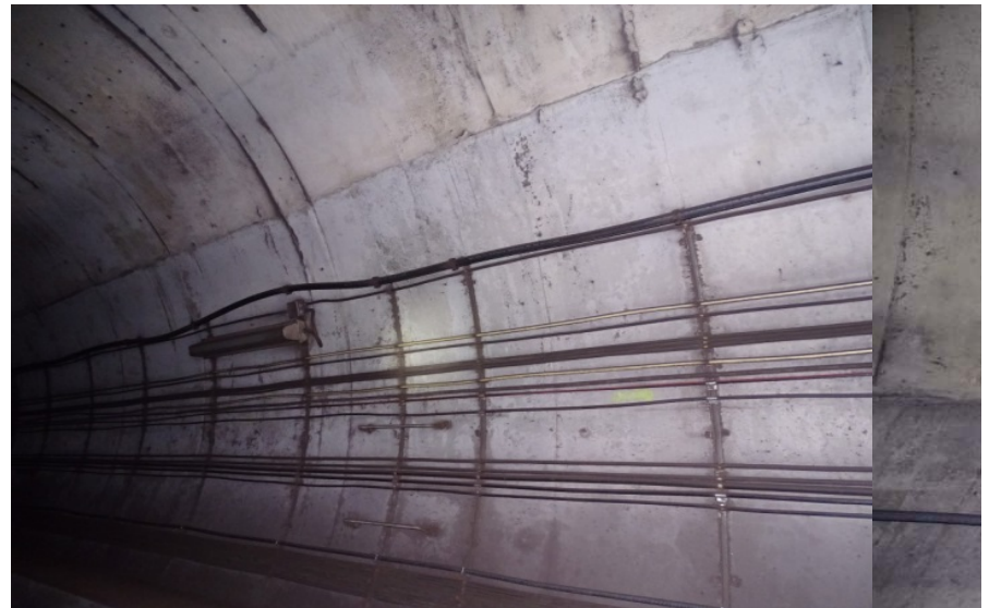
Photograph No. 472 Station 76+70, upper portion of west wall.
