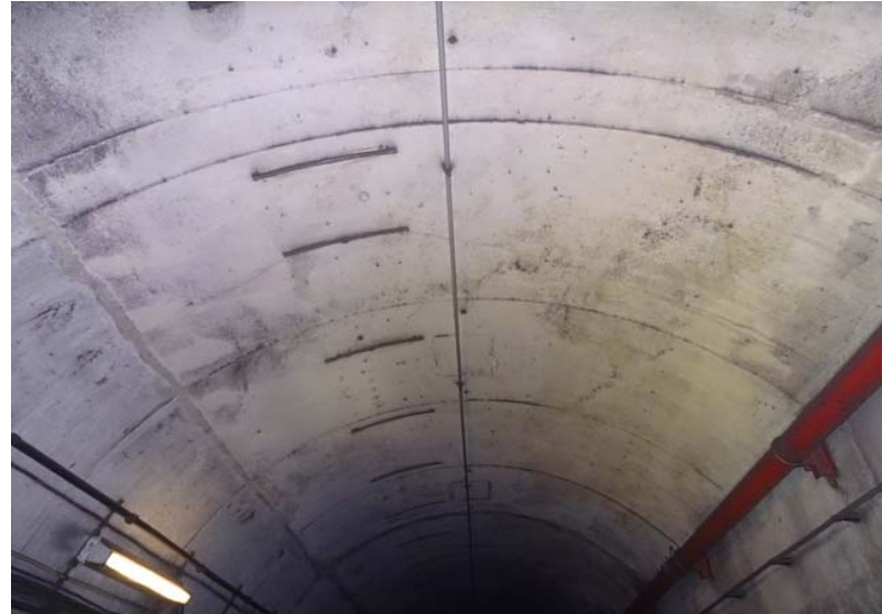
Photograph No. 194 Station 74+60, ceiling.
