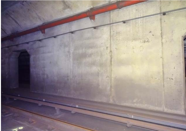
Photograph No. 185 Station 74+40, west wall.
