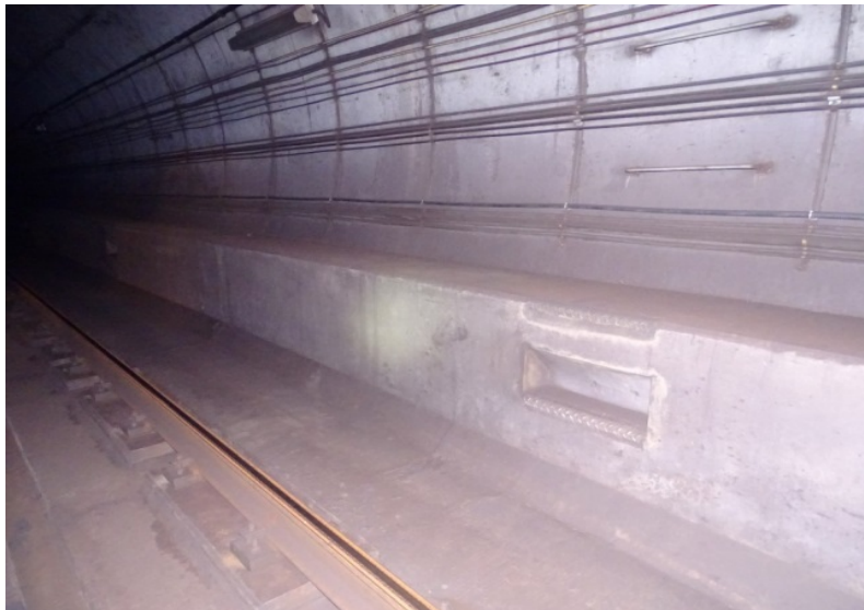
Photograph No. 555 Station 78+20, lower portion of west wall.
