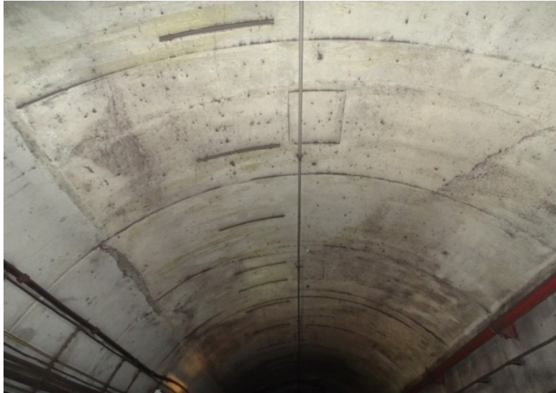
Photograph No. 277 Station 76+60, ceiling.
