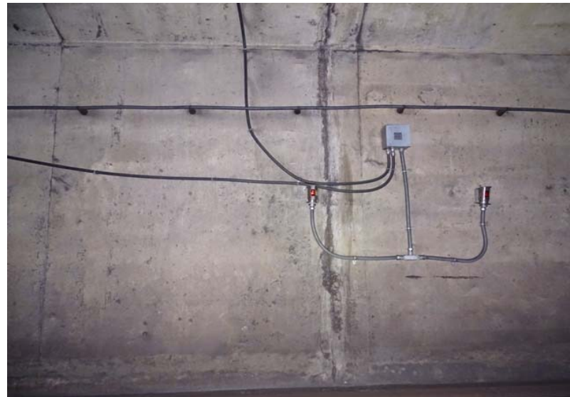
Photograph No. 196 Station 72+80, east wall.
