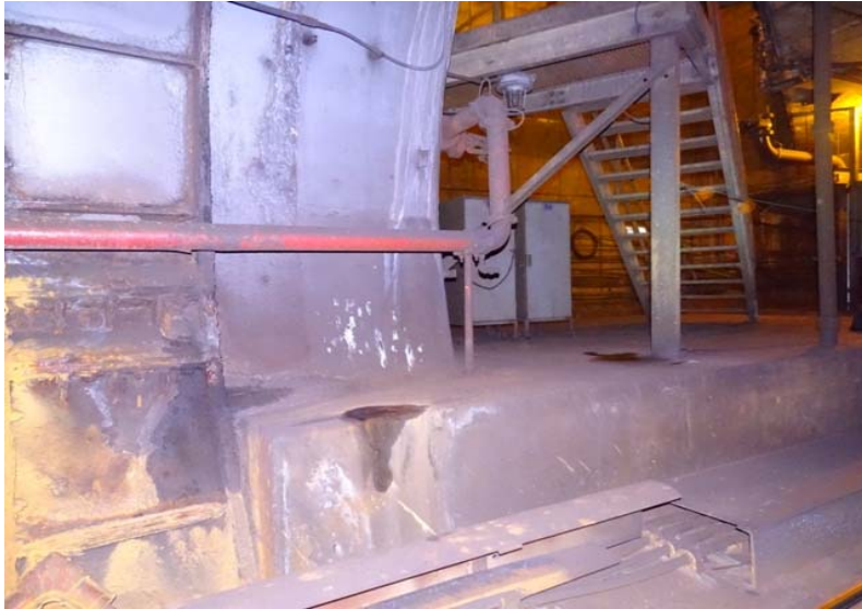
Photograph No. 37 Station 70+40, east wall.
