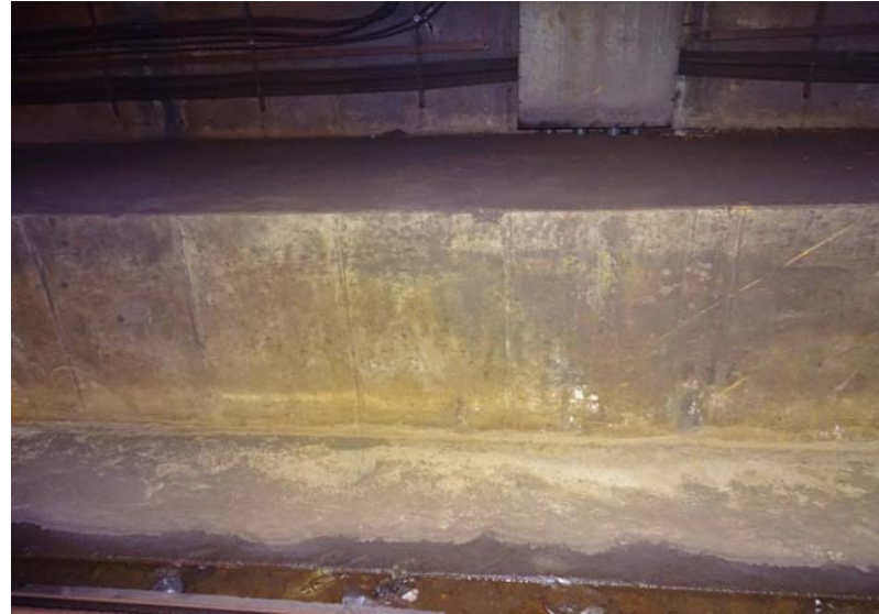
Photograph No.54 Station 70+60, lower portion of west wall.
