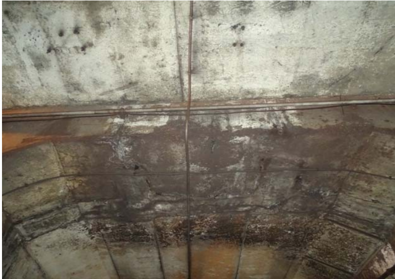
Photograph No. 69 Station 70+90, ceiling.
