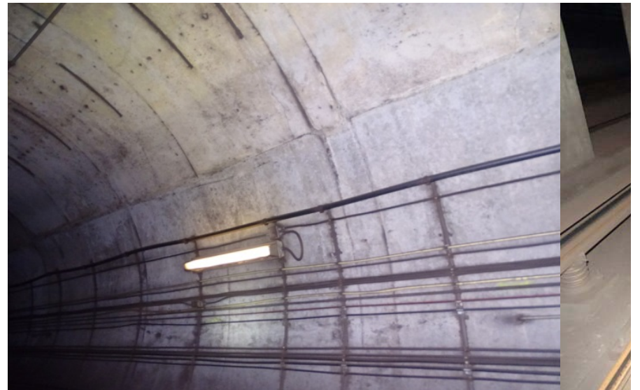
Photograph No. 388 Station 75+50, upper portion of west wall.
