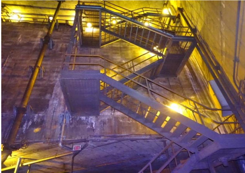
Photograph No. 37 Main room, stair at the southwest wall.
