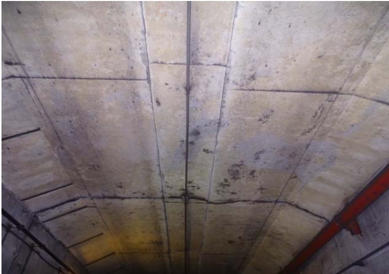
Photograph No. 115 Station 72+60, ceiling.
