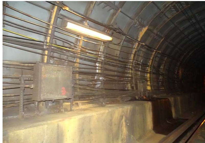
Photograph No. 8 Station 69+80, east wall.
