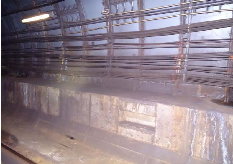
Photograph No. 13 Station 69+90, west wall.
