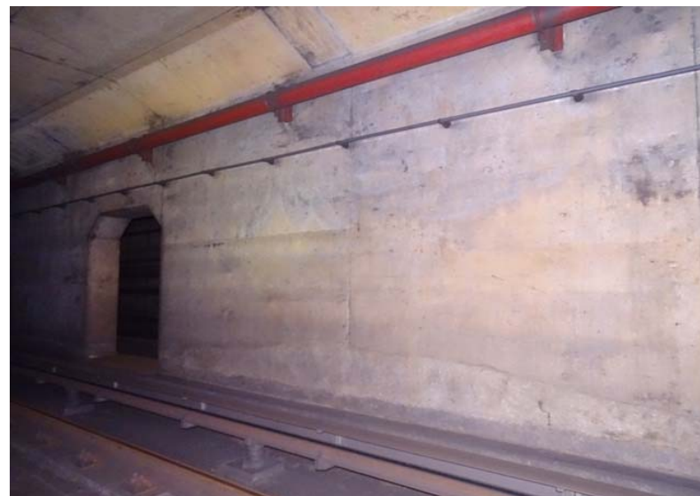
Photograph No. 148 Station 73+40, west wall.
