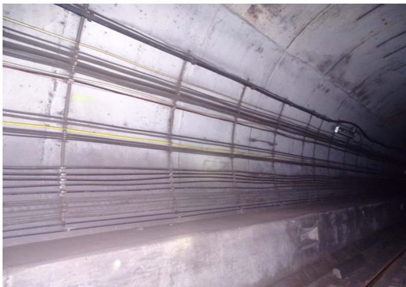
Photograph No. 315 Station 77+40, east wall.
