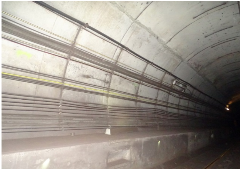
Photograph No. 255 Station 76+20, east wall.
