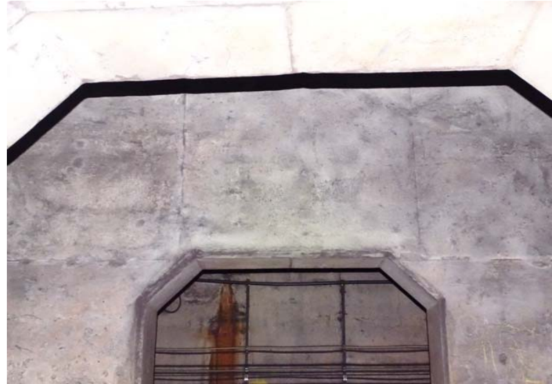
Photograph No. 6 Storage area, section 1, upper middle portion.
