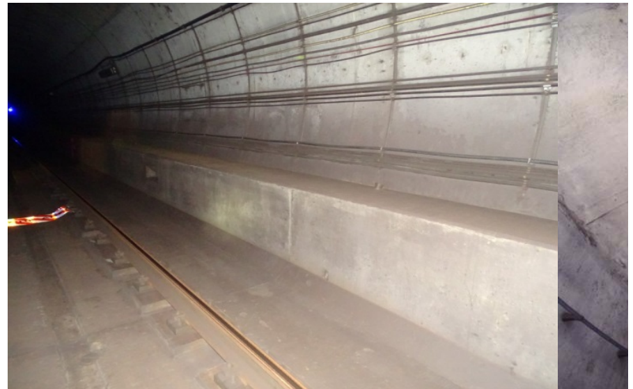
Photograph No. 568 Station 78+50, lower portion of west wall.
