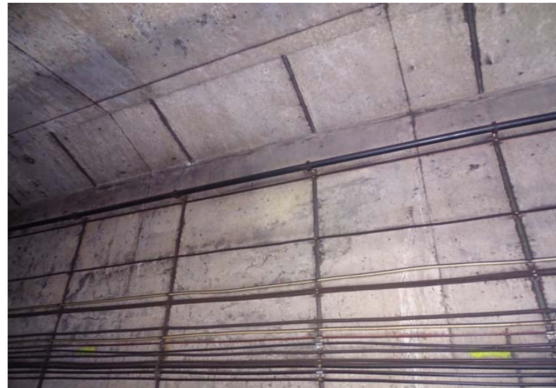
Photograph No. 284 Station 74+10, upper portion of west wall.
