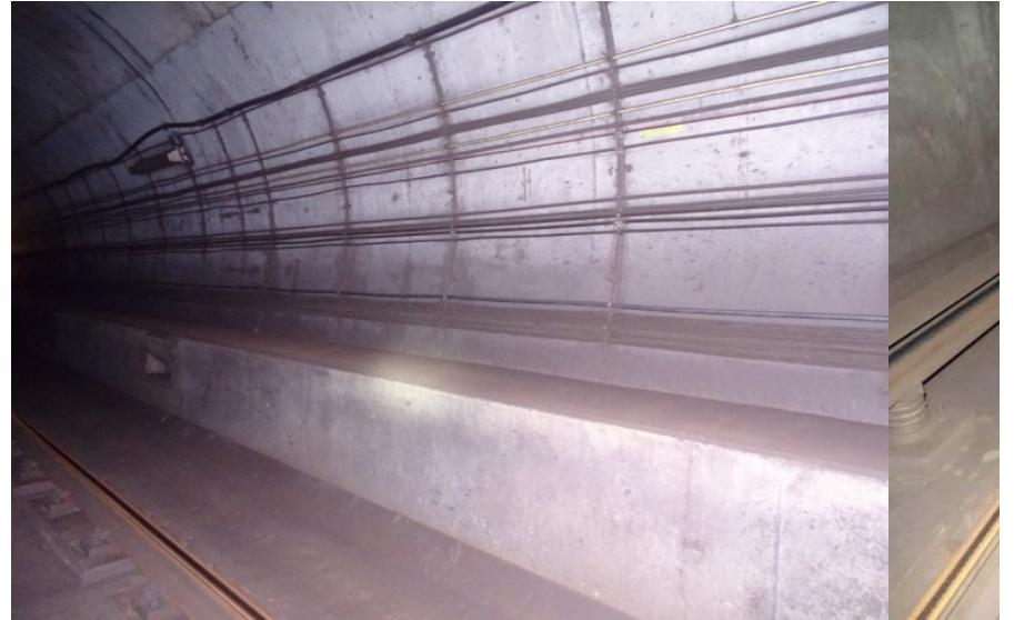
Photograph No. 466 Station 76+60, lower portion of west wall.
