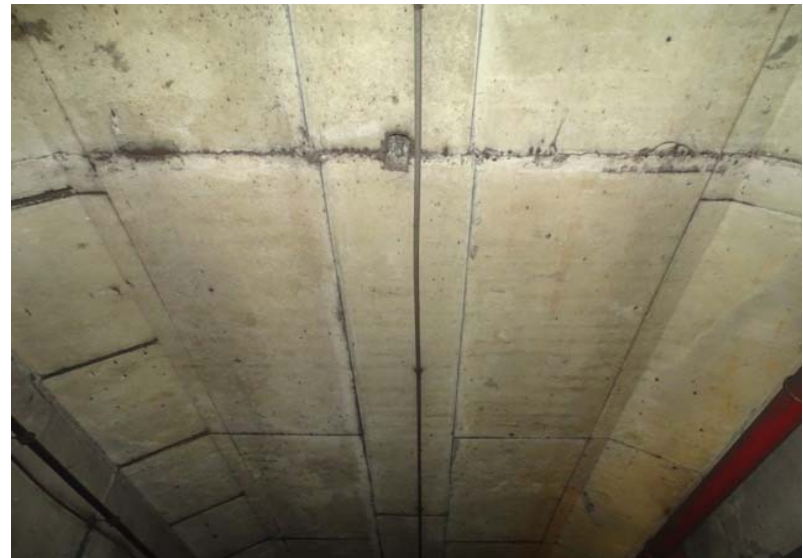
Photograph No. 140 Station 73+20, ceiling.
