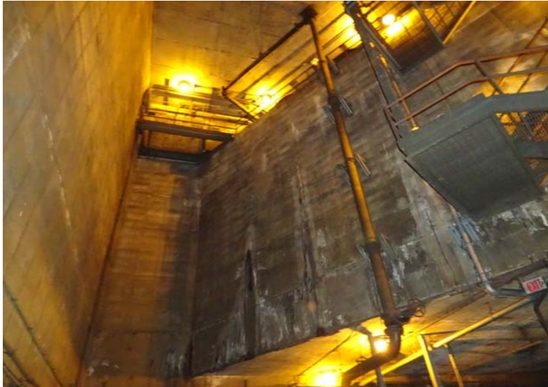
Photograph No. 33 Main room at entrance to tracks from vent shaft.
