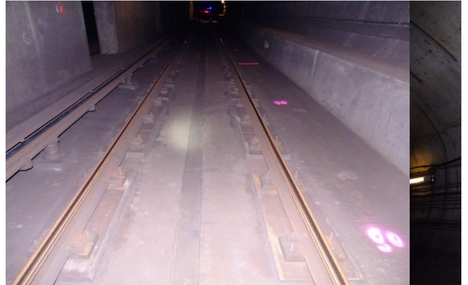
Photograph No. 406 Station 75+80, track bed.
