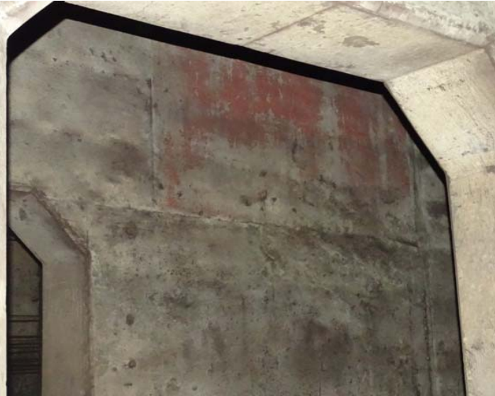
Photograph No. 13 Storage area, section 2, upper north portion.
