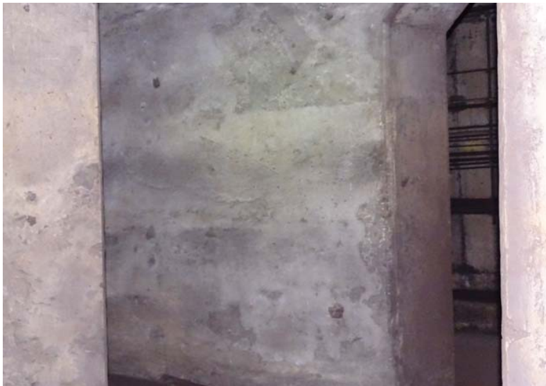
Photograph No. 31 Storage area, section 3. Close up of previous concrete repair.
