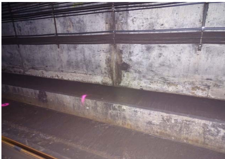
Photograph No. 243 Station 73+40, lower portion of west wall.
