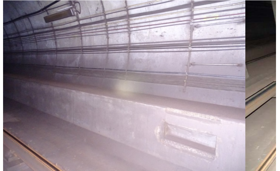
Photograph No. 522 Station 77+50, lower portion of west wall.
