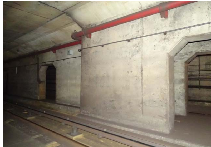
Photograph No. 68 Station 71+60, west wall.
