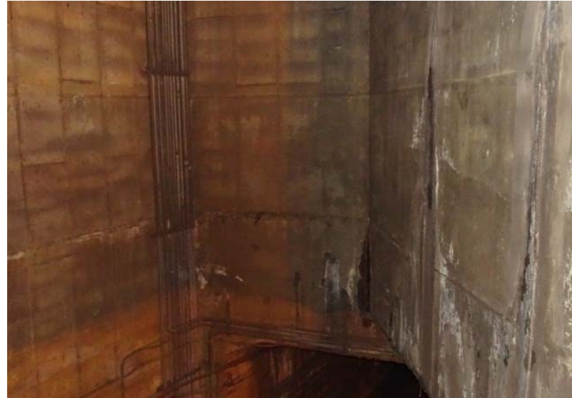
Photograph No. 70 Main room, lower south wall.
