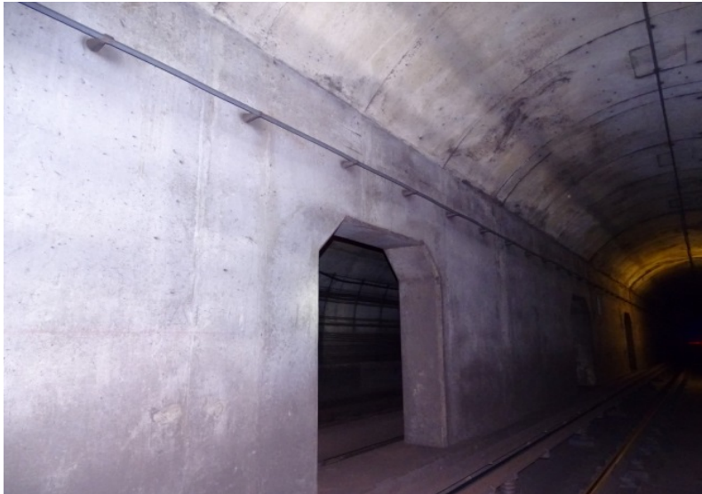
Photograph No. 463 Station 76+60, east wall.
