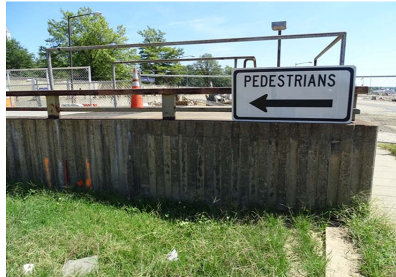
Photograph No. 194 Vent shaft exterior, northwest side, section 1.
