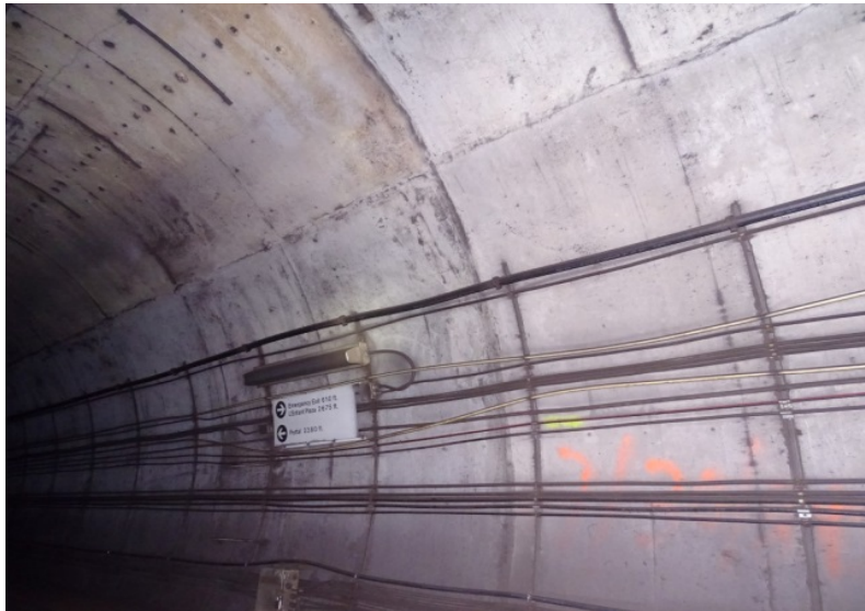
Photograph No. 541 Station 77+80, upper portion of west wall.
