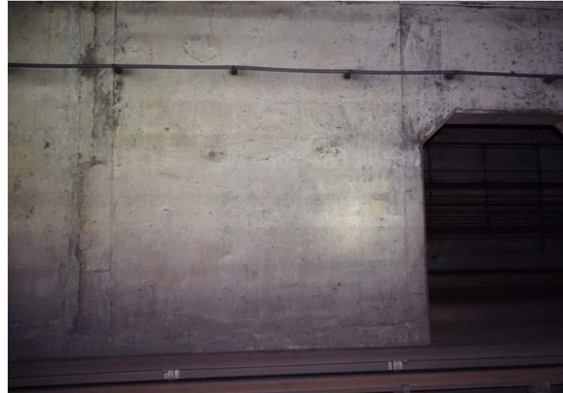
Photograph No. 234 Station 73+30, east wall.
