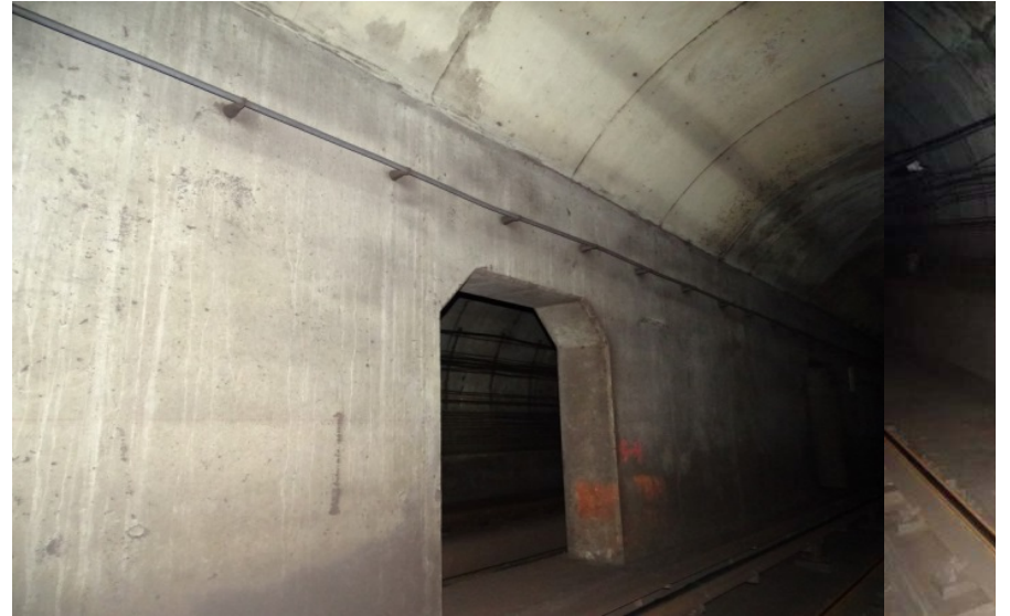
Photograph No. 526 Station 77+60, east wall.
