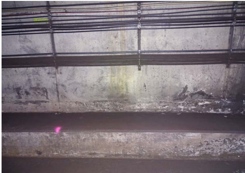
Photograph No. 237 Station 73+30, lower portion of west wall.
