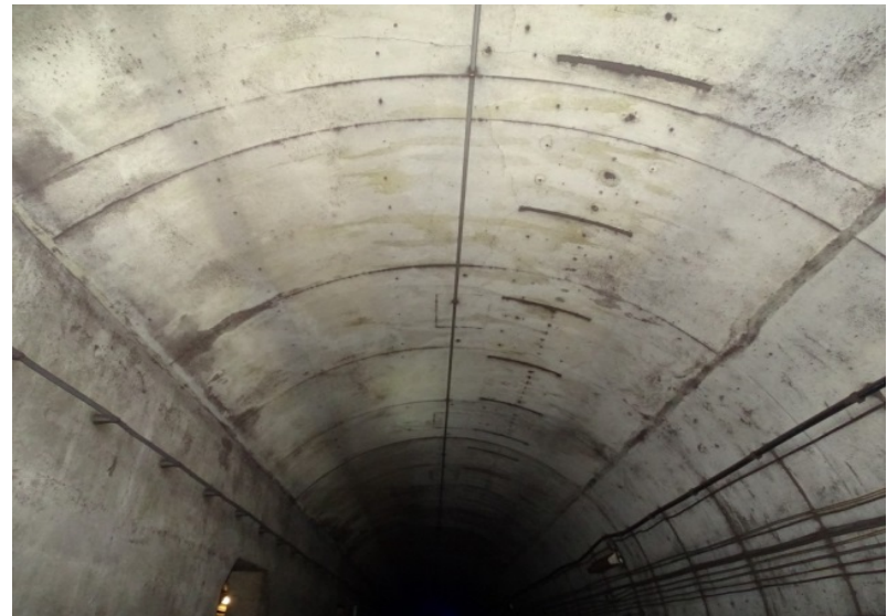
Photograph No. 560 Station 78+40, ceiling.
