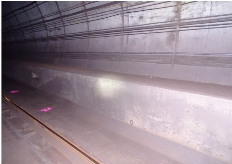
Photograph No. 395 Station 75+60, lower portion of west wall.
