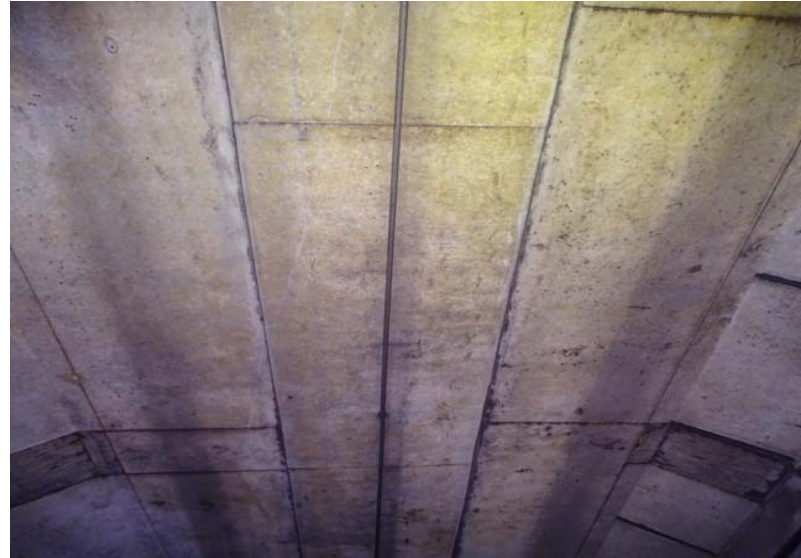
Photograph No. 178 Station 72+50, ceiling.
