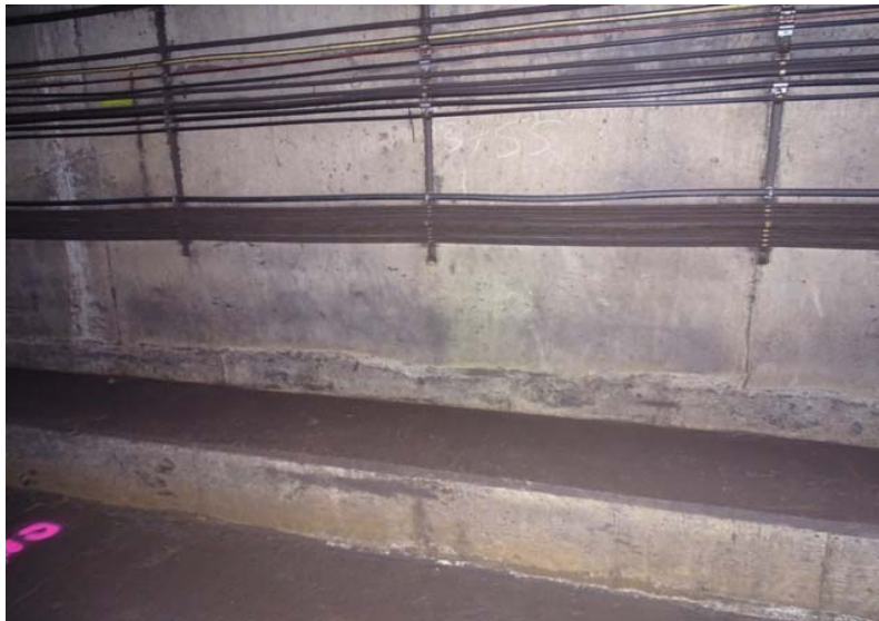
Photograph No. 279 Station 74+00, lower portion of west wall.
