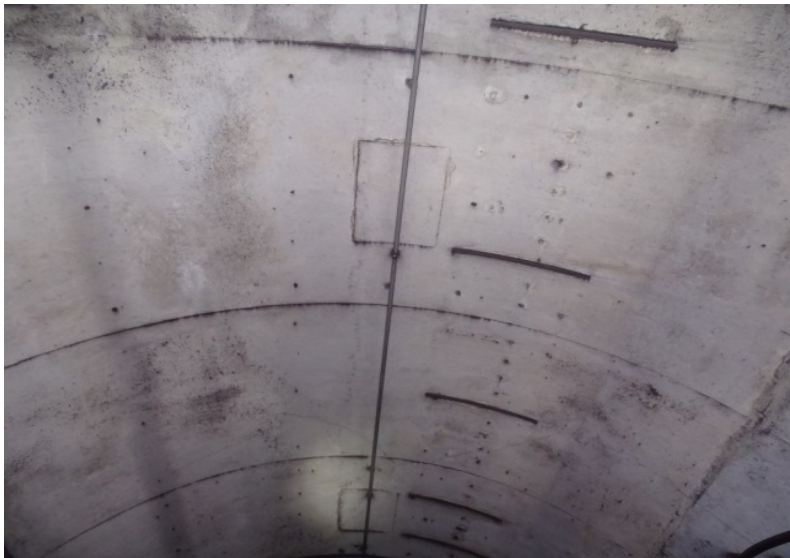
Photograph No. 367 Station 75+20, ceiling.
