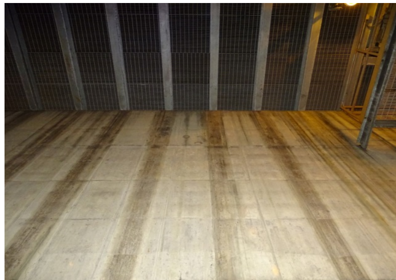
Photograph No. 142 Upper fan room, east wall, north-center section, upper portion.
