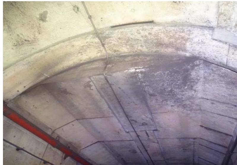
Photograph No. 176 Station 74+20, ceiling, looking north.
