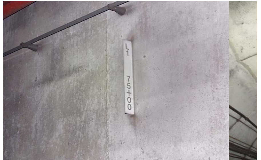
Photograph No. 204 Station 75+00 - marker for L1 75+00.
