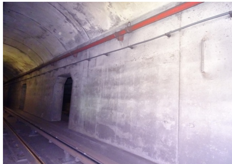
Photograph No. 338 Station 78+00, west wall.
