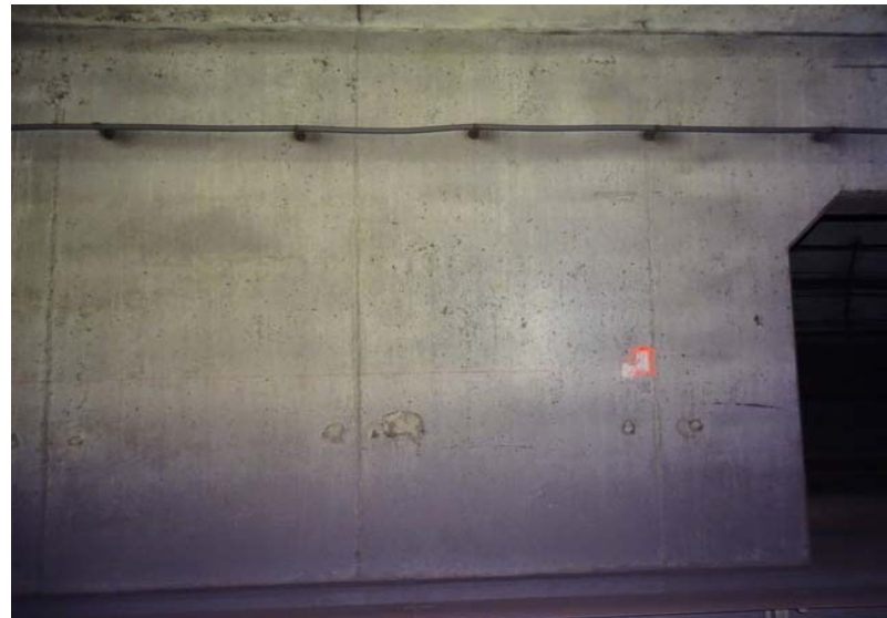
Photograph No. 332 Station 74+80, east wall.
