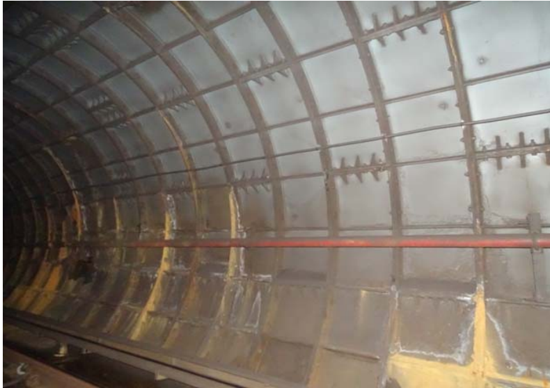
Photograph No. 13 Station 69+80, west wall.
