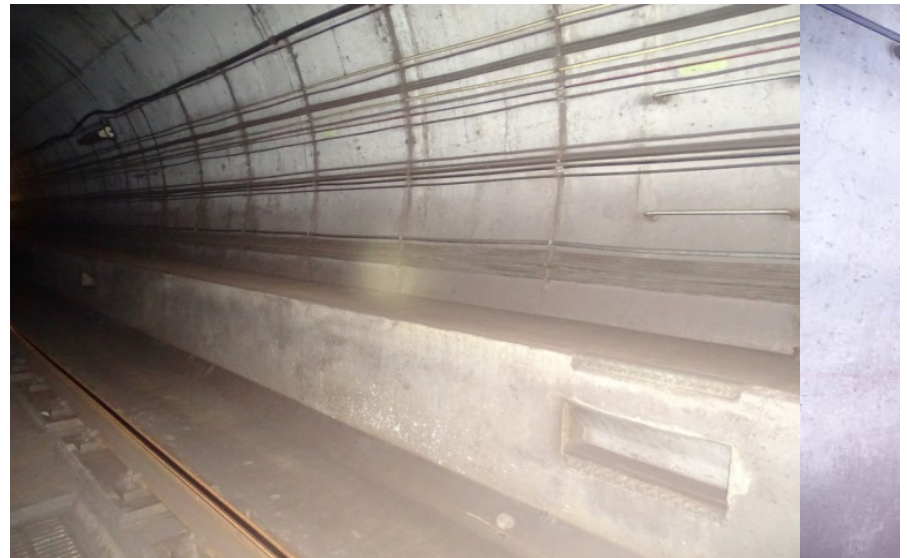
Photograph No. 460 Station 76+50, lower portion of west wall.
