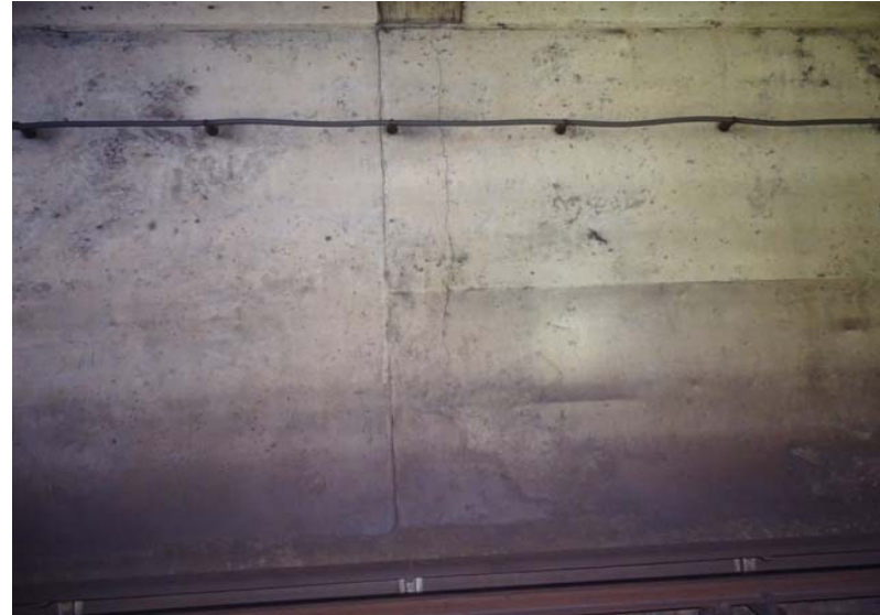
Photograph No. 106 Station 71+50, east wall.
