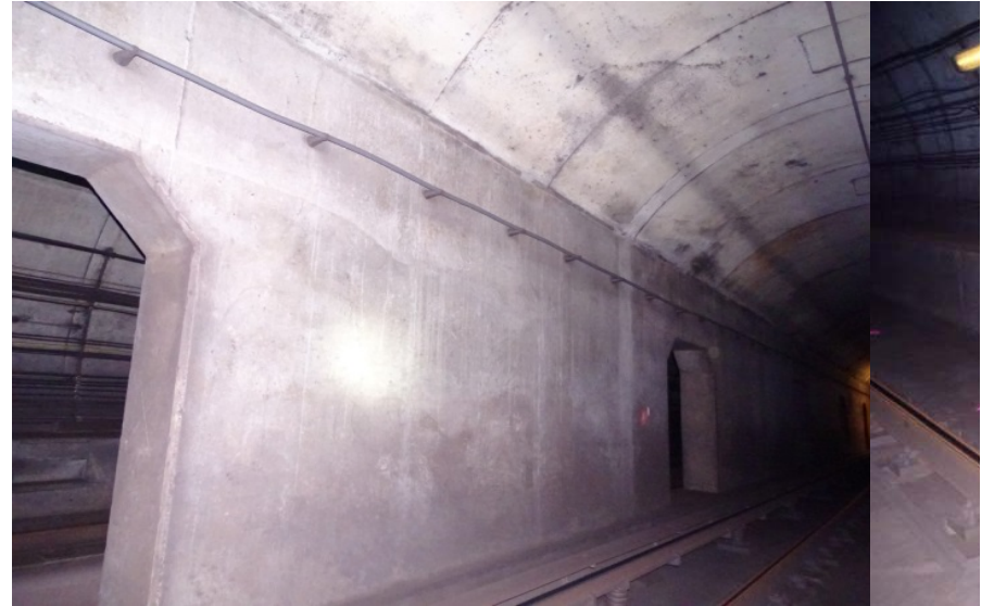
Photograph No. 438 Station 76+20, east wall.
