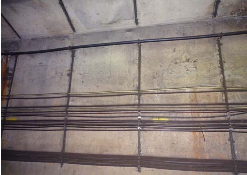
Photograph No. 81 Station 71+10, upper portion of west wall.
