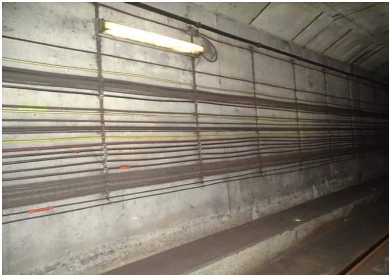
Photograph No. 83 Station 72+00, east wall.
