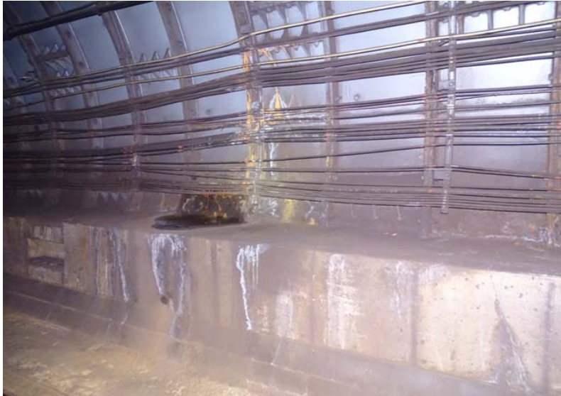
Photograph No. 9 Station 69+80, west wall.
