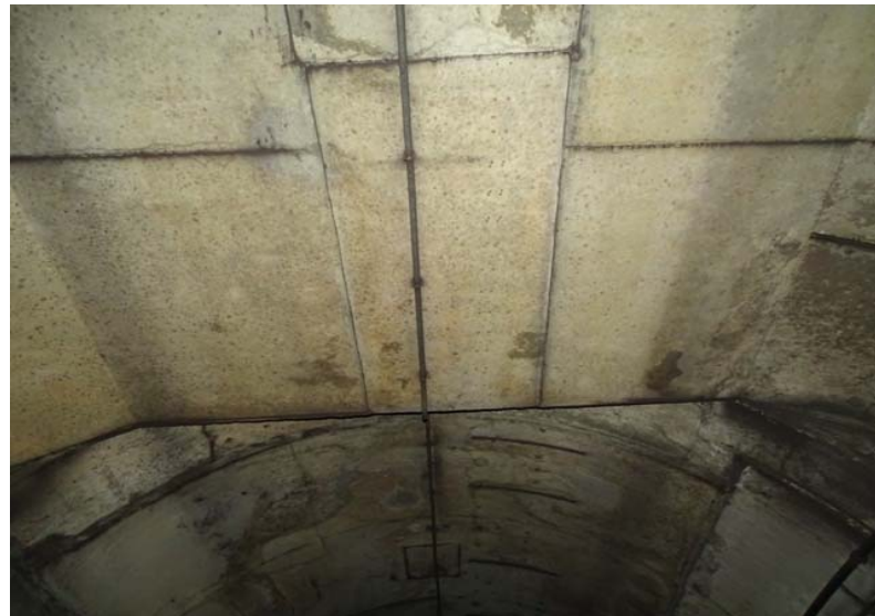
Photograph No. 298 Station 74+30, ceiling.
