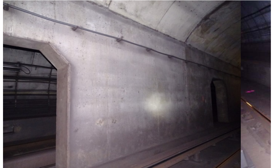
Photograph No. 366 Station 75+20, east wall.
