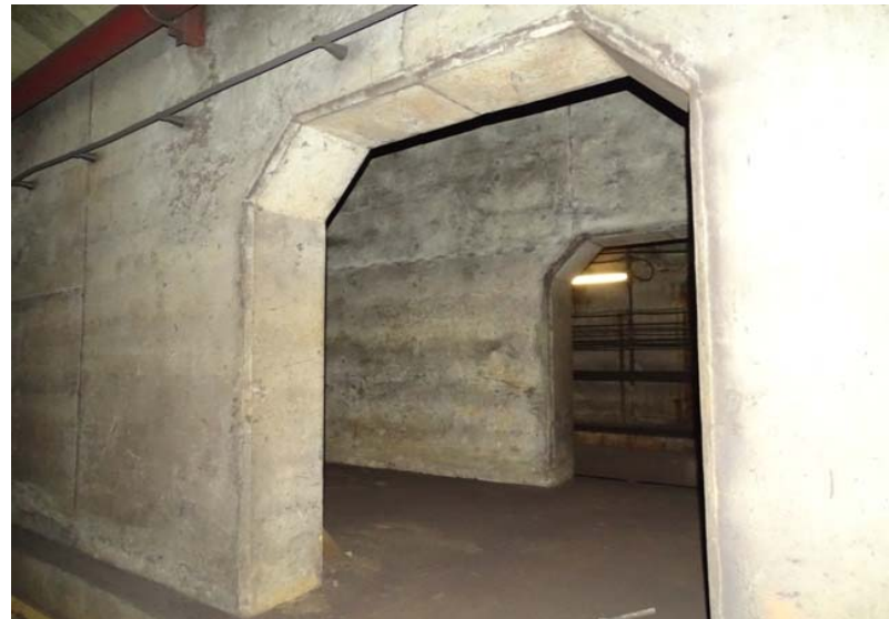
Photograph No. 8 Storage area, section 1, looking south.
