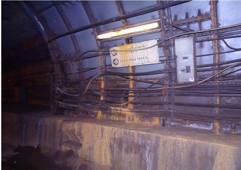
Photograph No. 33 Station 70+30, west wall.
