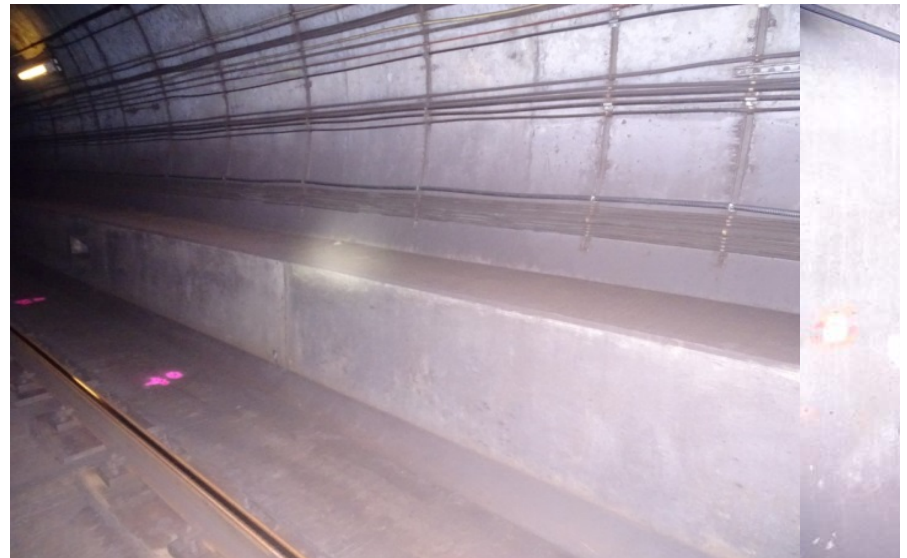
Photograph No. 376 Station 75+30, lower portion of west wall.
