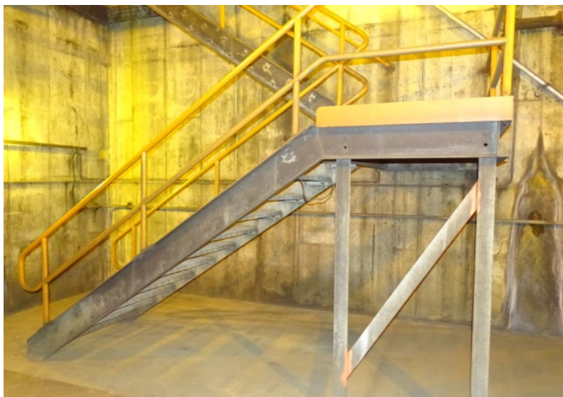
Photograph No. 163 Upper fan room, west wall, south section, lower portion.
