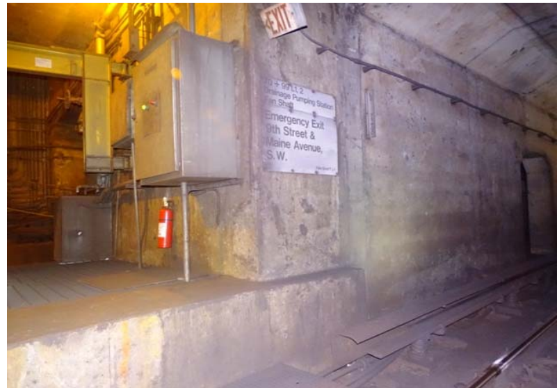
Photograph No. 68 Station 70+90, east wall.
