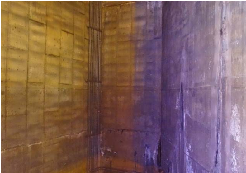
Photograph No. 71 Main room, upper south wall.
