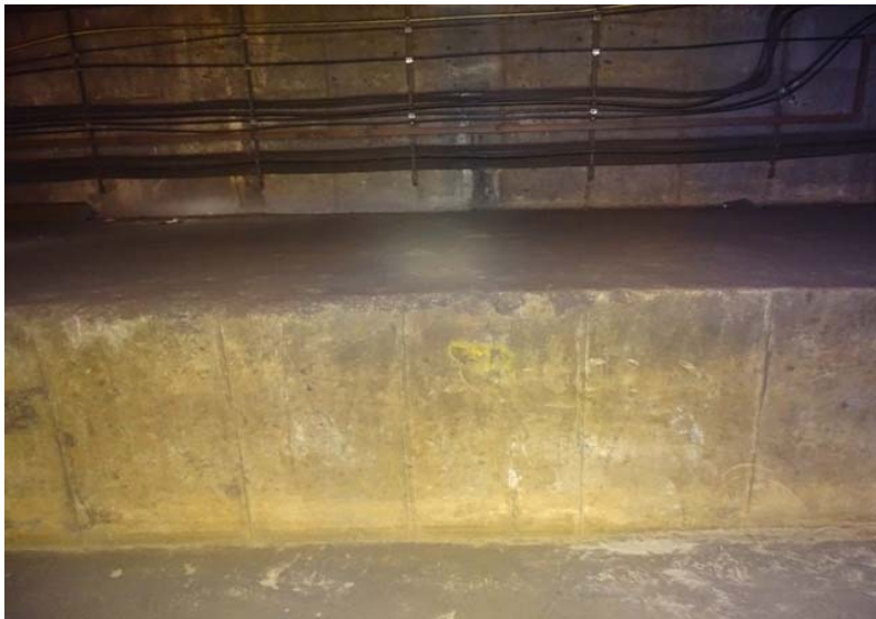
Photograph No. 59 Station 70+70, lower portion of west wall.
