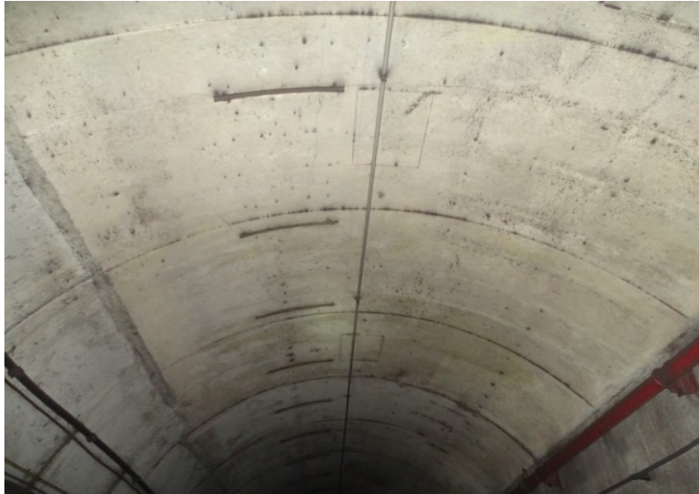
Photograph No. 249 Station 76+00, ceiling.
