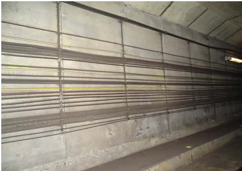
Photograph No. 71 Station 71+80, east wall.
