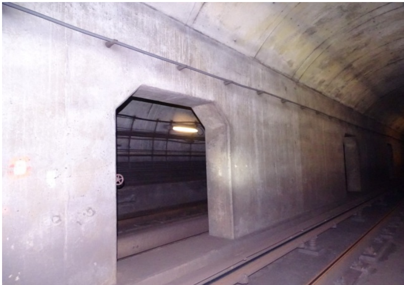
Photograph No. 379 Station 75+40, east wall.
