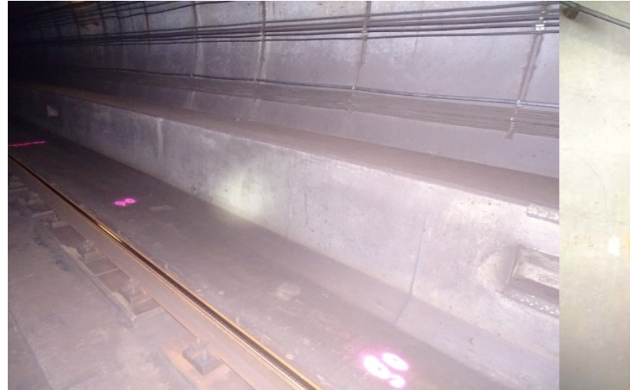
Photograph No. 410 Station 75+80, lower portion of west wall.
