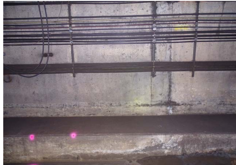
Photograph No. 130 Station 71+80, lower portion of west wall.
