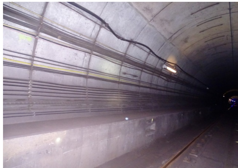
Photograph No. 222 Station 75+40, east wall.
