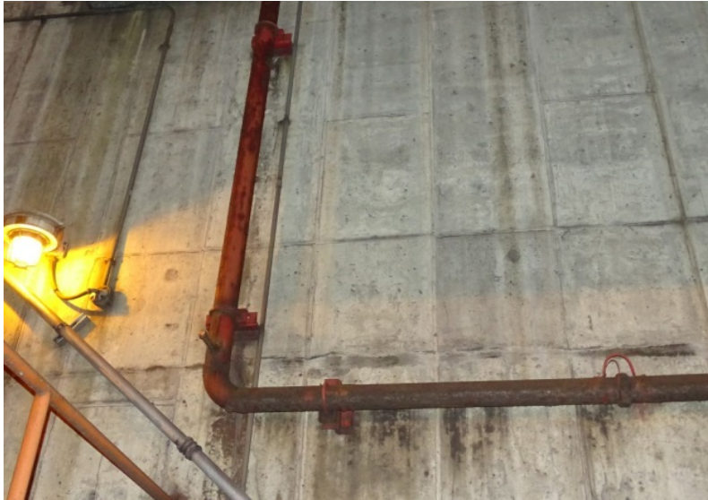
Photograph No. 165 Upper fan room, west wall, middle-north section, middle portion.
