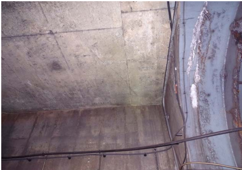
Photograph No. 39 Station 70+40, ceiling, looking west.
