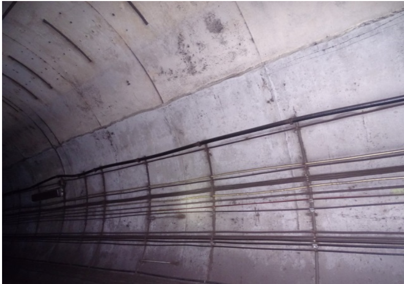
Photograph No. 515 Station 77+40, upper portion of west wall.
