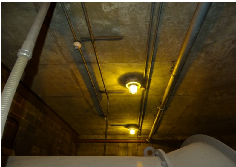
Photograph No. 131 Main room, upper level, northwest portion of ceiling.
