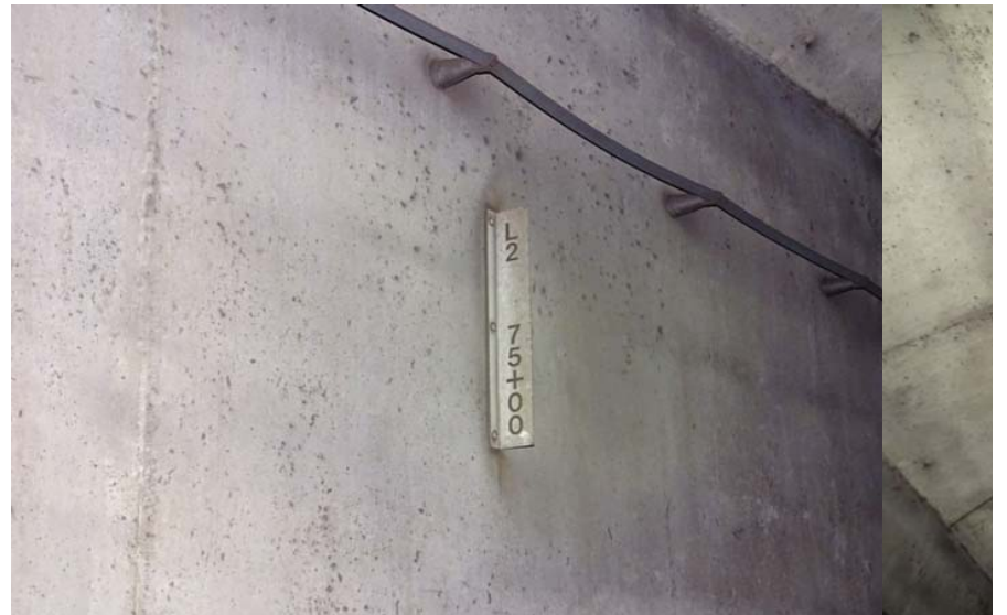
Photograph No. 348 Station 75+00 - marker for L2 75+00.
