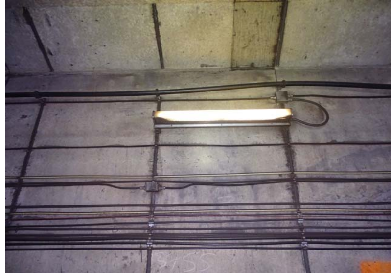
Photograph No. 278 Station 74+00, upper portion of west wall.
