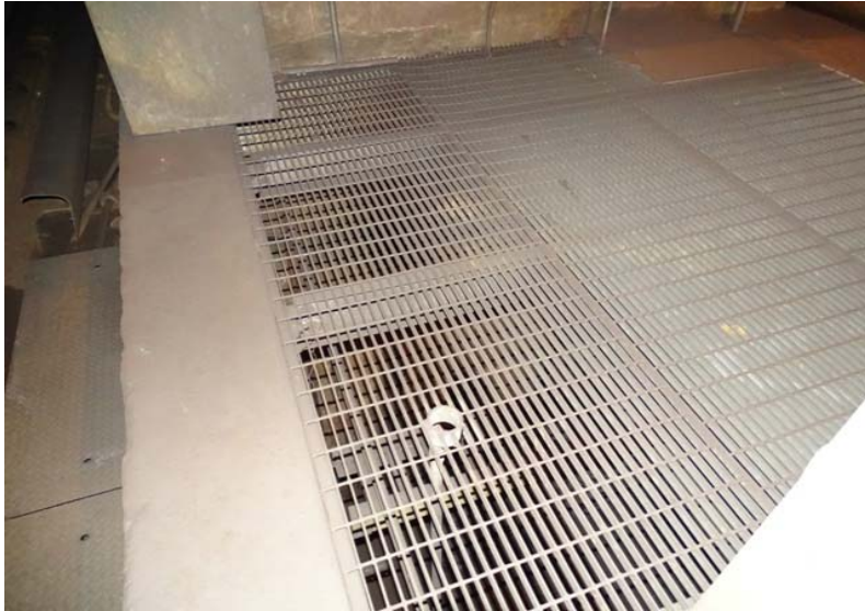
Photograph No. 41 Platform, floor, southeast portion.
