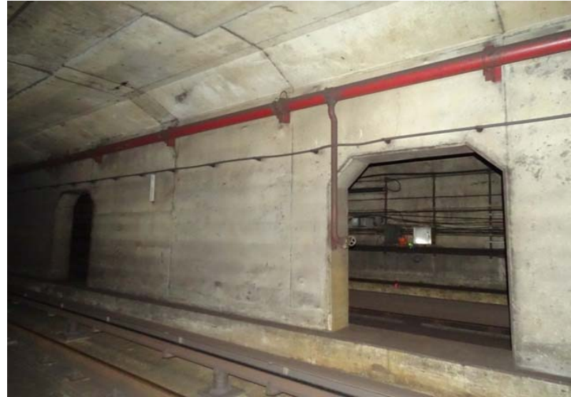
Photograph No. 78 Station 71+80, west wall.
