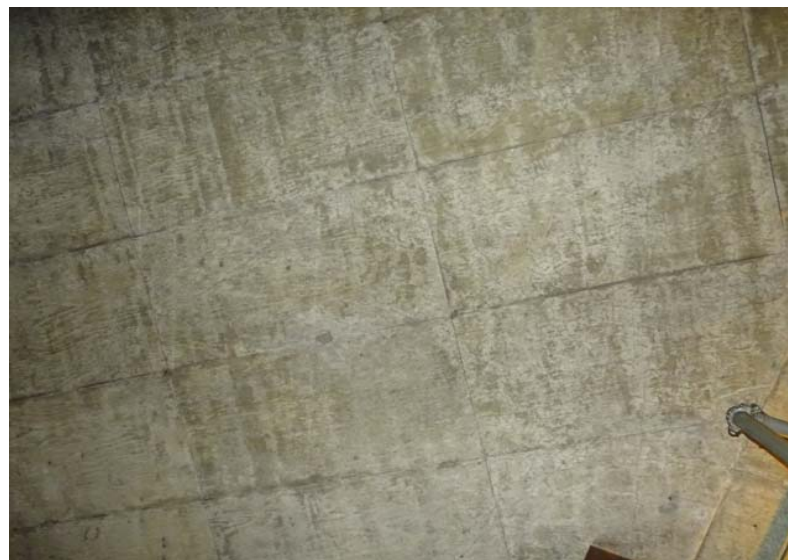
Photograph No. 112 Main room, ceiling, section 8, middle portion.
