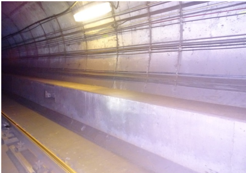
Photograph No. 499 Station 77+10, lower portion of west wall.
