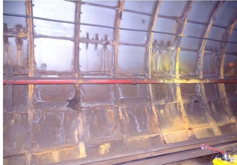
Photograph No. 26 Station 70+20, east wall.
