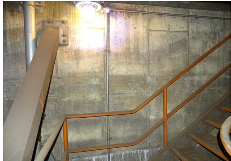
Photograph No. 100 Main room, upper portion, west wall at the stair.
