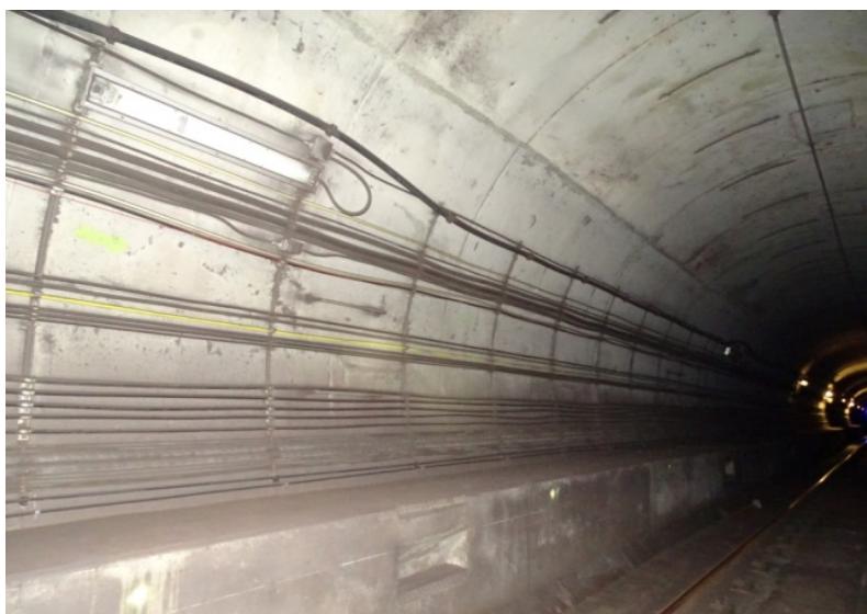
Photograph No. 307 Station 77+20, east wall.
