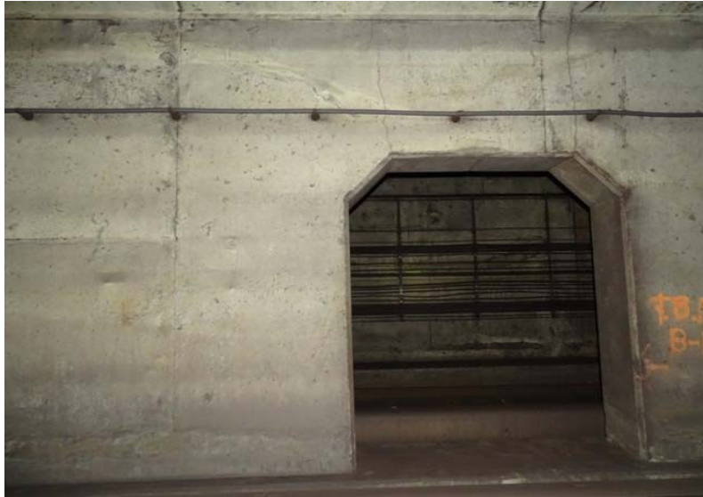
Photograph No. 281 Station 74+10, east wall.
