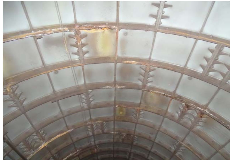
Photograph No. 4 Station 69+60, ceiling.
