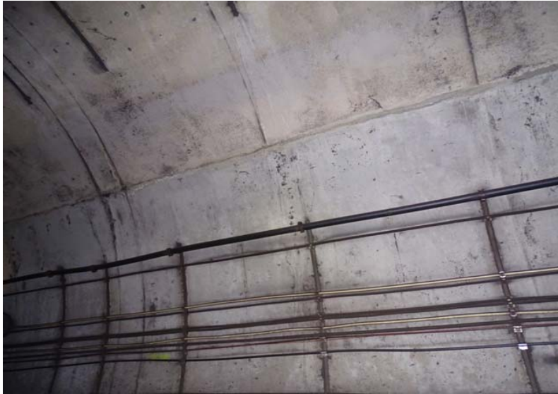
Photograph No. 321 Station 74+60, upper portion of west wall.
