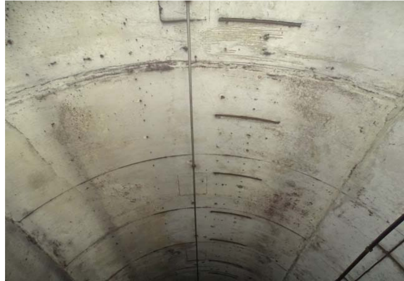
Photograph No. 342 Station 74+90, ceiling.
