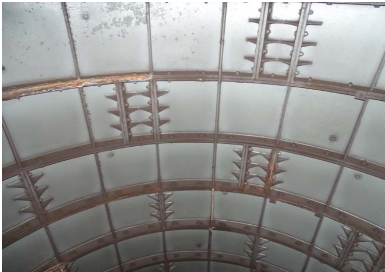
Photograph No. 3 Station 69+70, ceiling.
