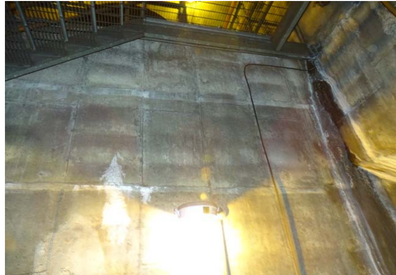
Photograph No. 76 Main room, northwest corner.
