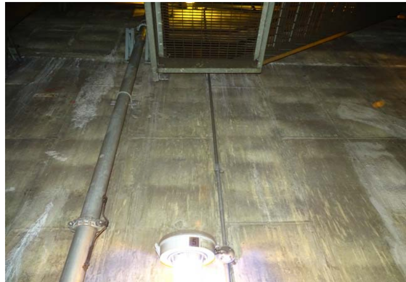
Photograph No. 80 Main room, west wall at the stair.
