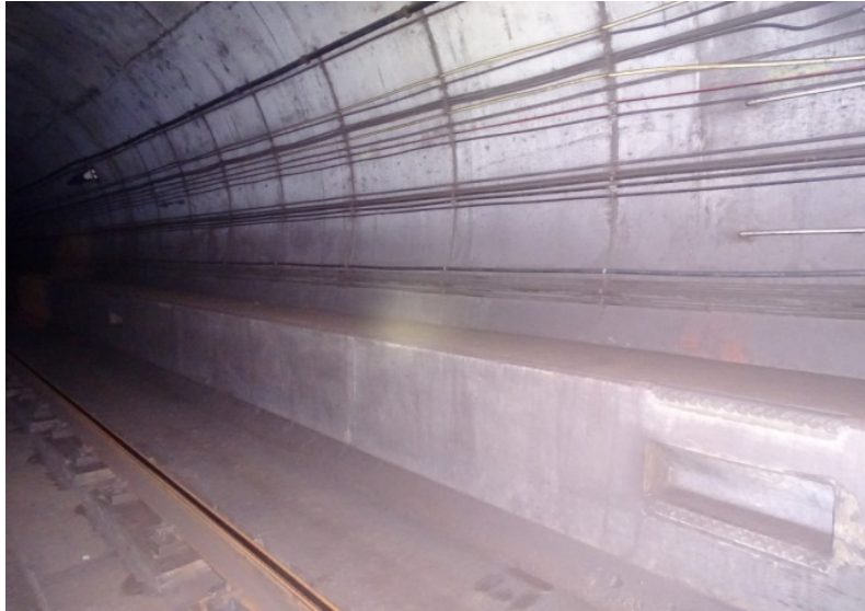
Photograph No. 549 Station 78+00, lower portion of west wall.
