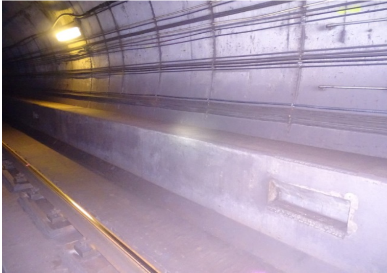
Photograph No. 493 Station 77+00, lower portion of west wall.
