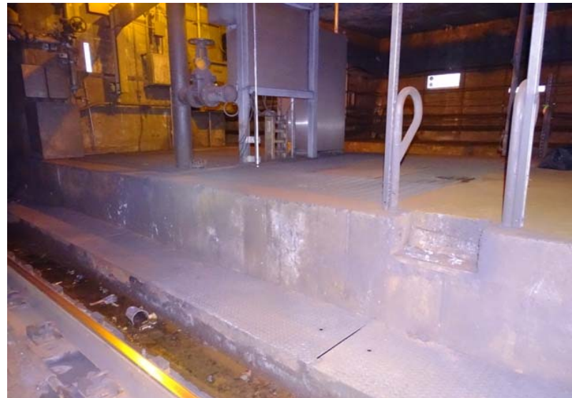
Photograph No. 36 Station 70+60, west wall.
