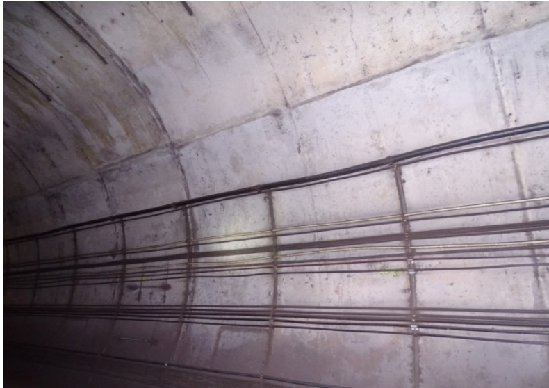
Photograph No. 485 Station 76+90, upper portion of west wall.
