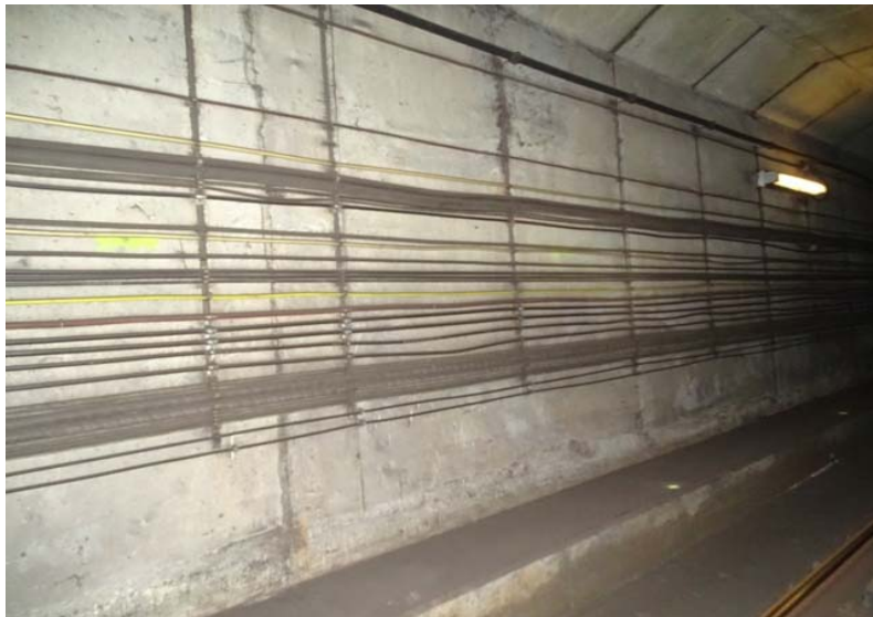
Photograph No. 91 Station 72+20, east wall.
