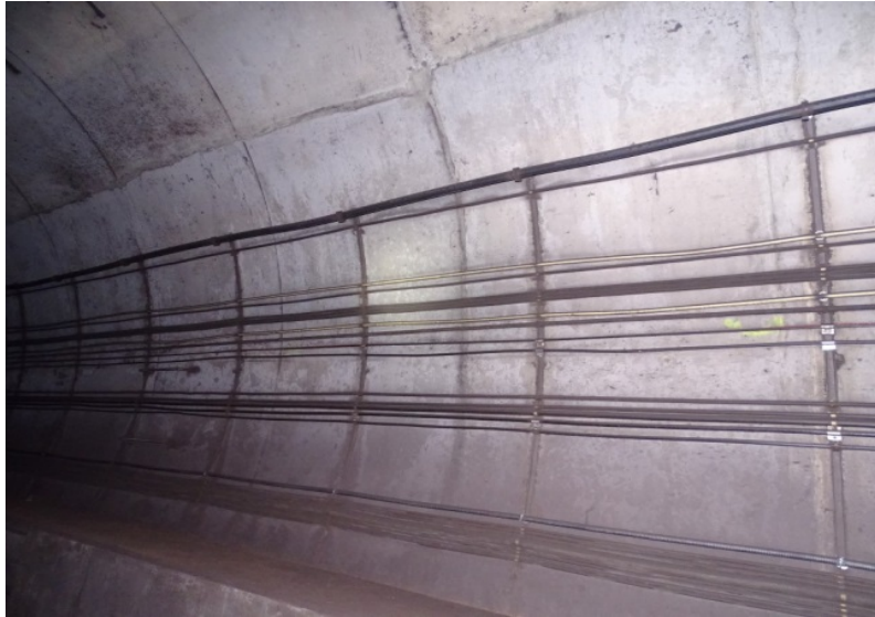
Photograph No. 433 Station 76+10, upper portion of west wall.
