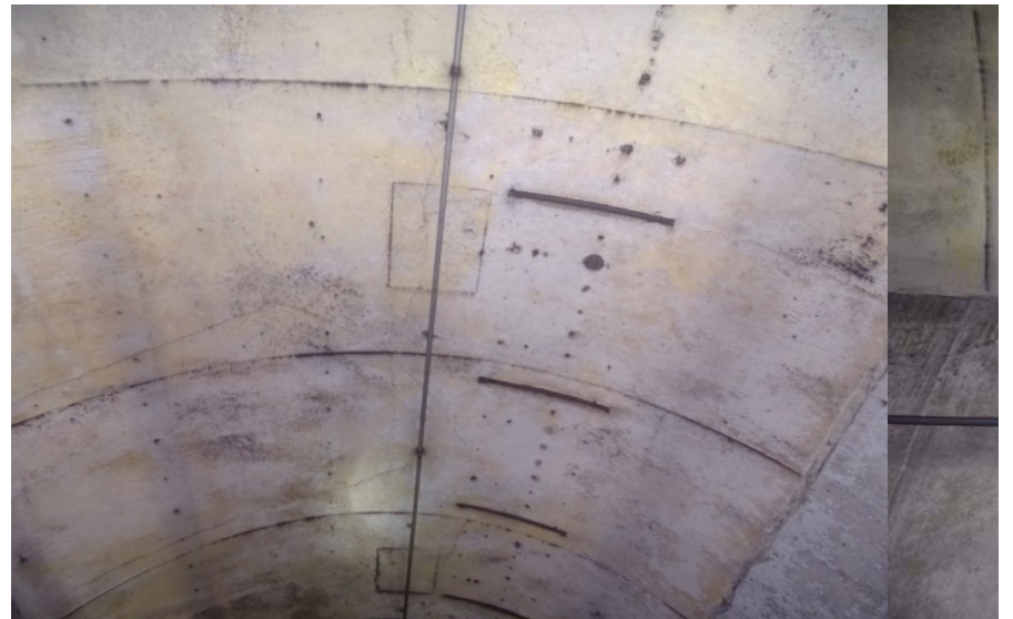
Photograph No. 380 Station 75+40, ceiling.
