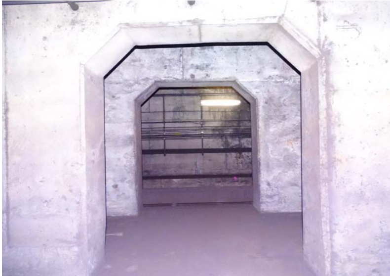
Photograph No. 25 Storage area, section 3, middle portion.
