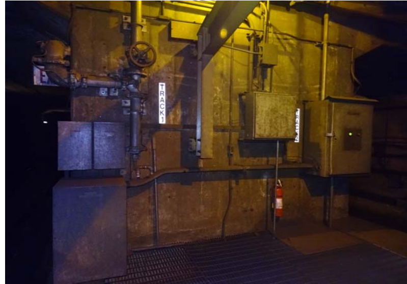
Photograph No. 42 Platform, south wall.
