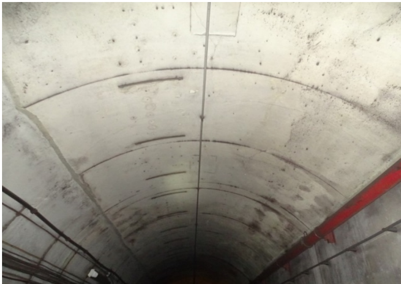
Photograph No. 207 Station 75+00, ceiling.
