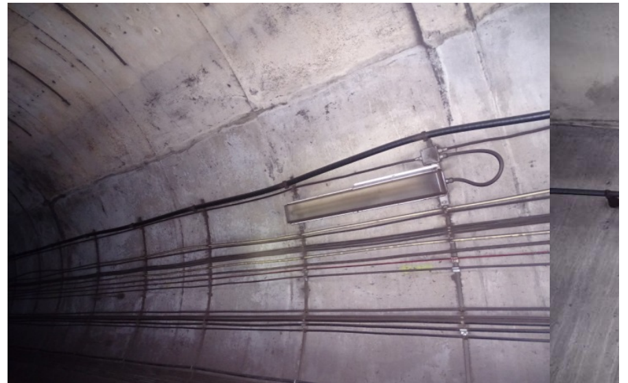
Photograph No. 528 Station 77+60, upper portion of west wall.
