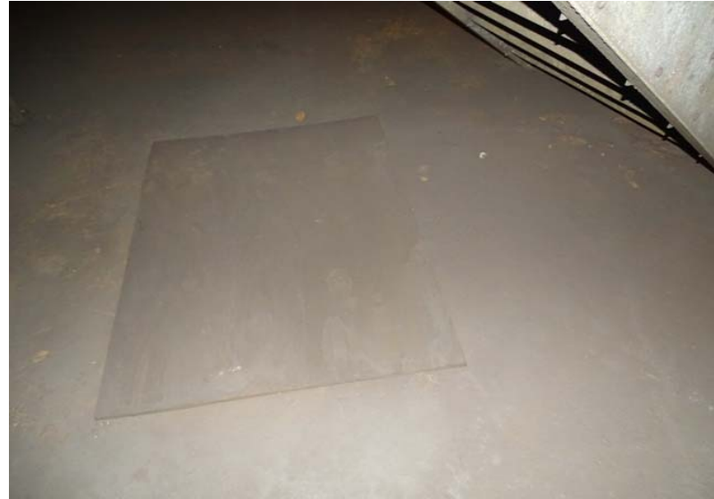
Photograph No. 54 Platform, floor, below stair.
