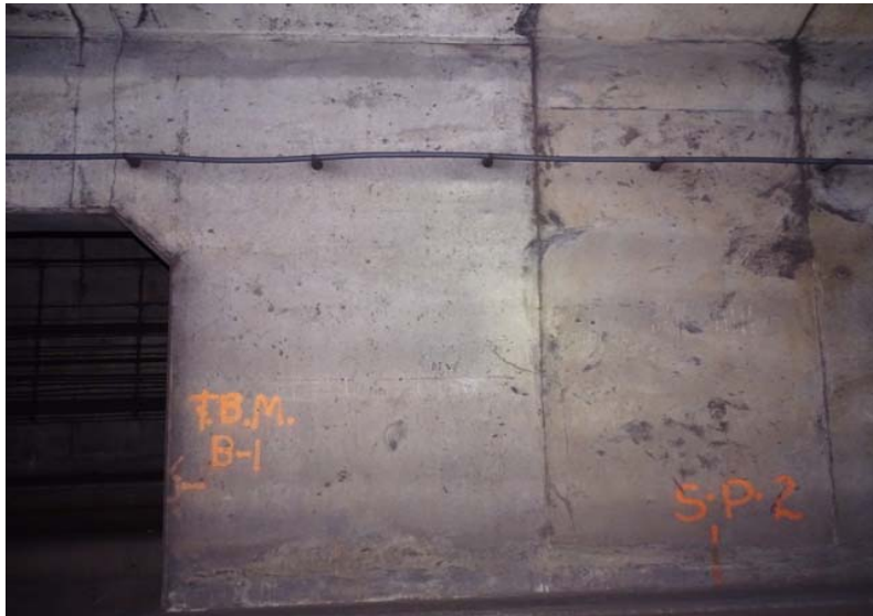
Photograph No. 289 Station 74+20, east wall.
