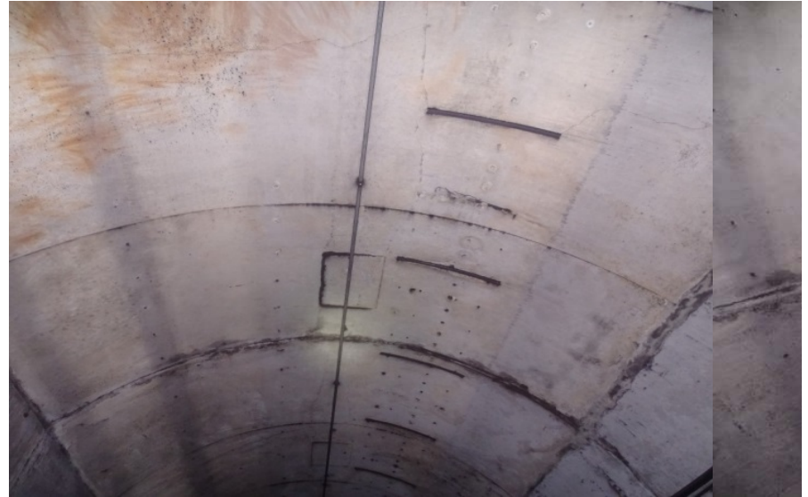
Photograph No. 458 Station 76+50, ceiling.
