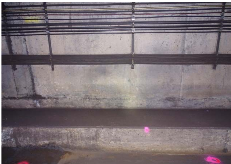
Photograph No. 123 Station 71+70, lower portion of west wall.
