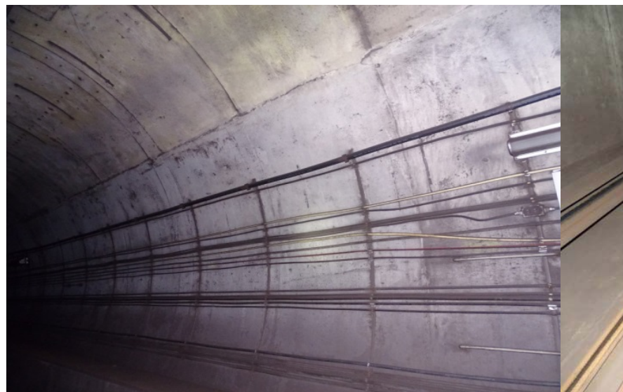
Photograph No. 548 Station 78+00, upper portion of west wall.
