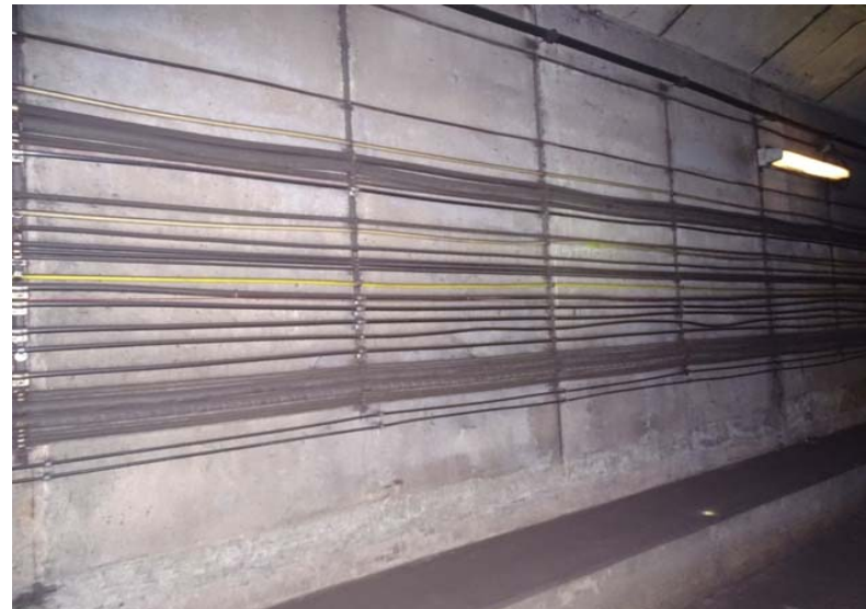
Photograph No. 146 Station 73+40, east wall.
