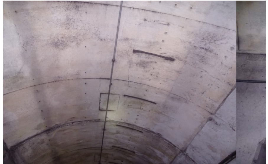
Photograph No. 484 Station 76+90, ceiling.
