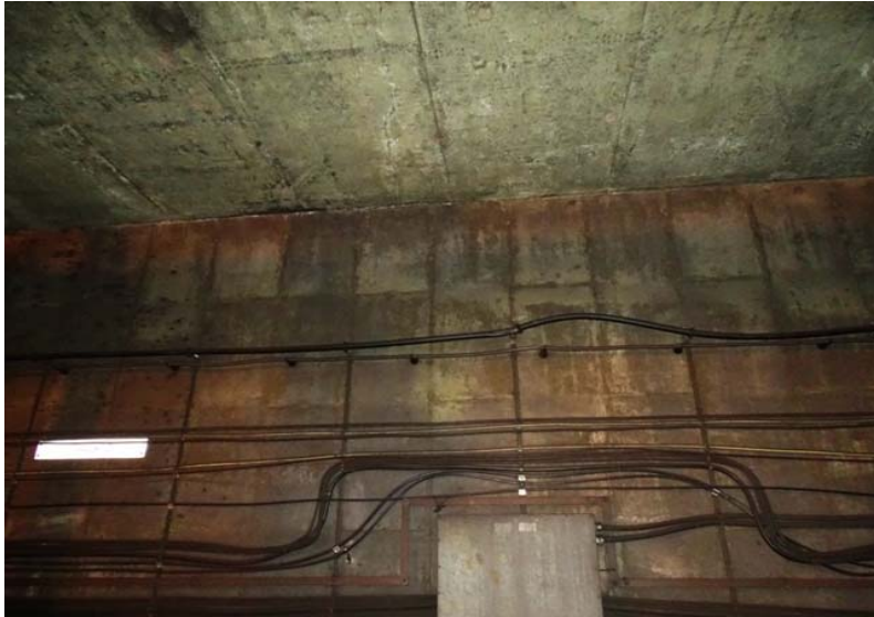
Photograph No. 53 Station 70+60, upper portion of west wall.
