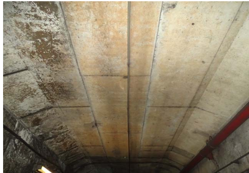
Photograph No. 44 Station 70+80, ceiling.
