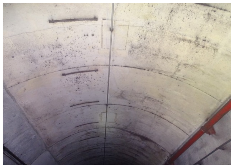
Photograph No. 232 Station 75+60, ceiling.
