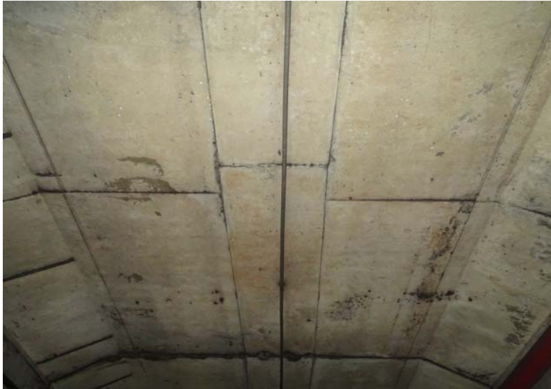
Photograph No. 157 Station 73+60, ceiling.
