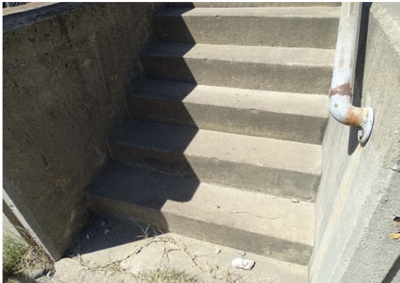
Photograph No. 187 Vent shaft exterior, steps at the south corner.
