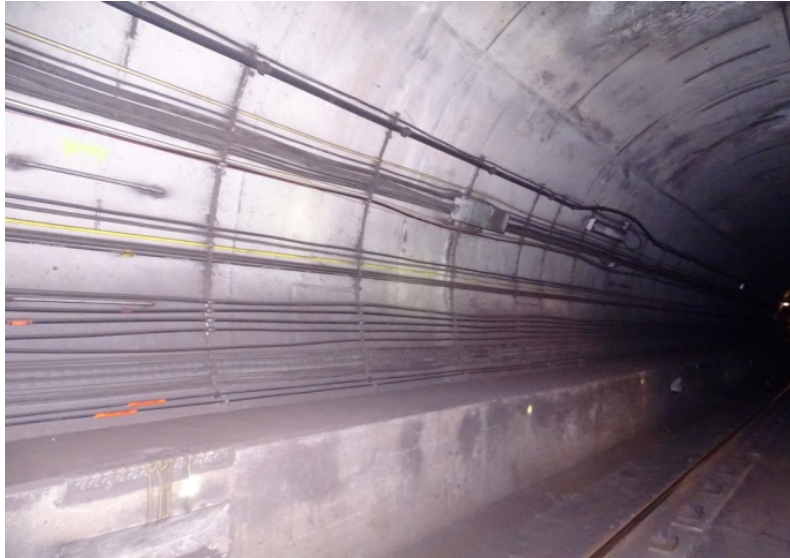
Photograph No. 297 Station 77+00, east wall.
