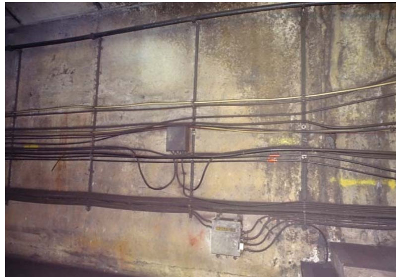
Photograph No. 76 Station 71+00, upper portion of west wall.
