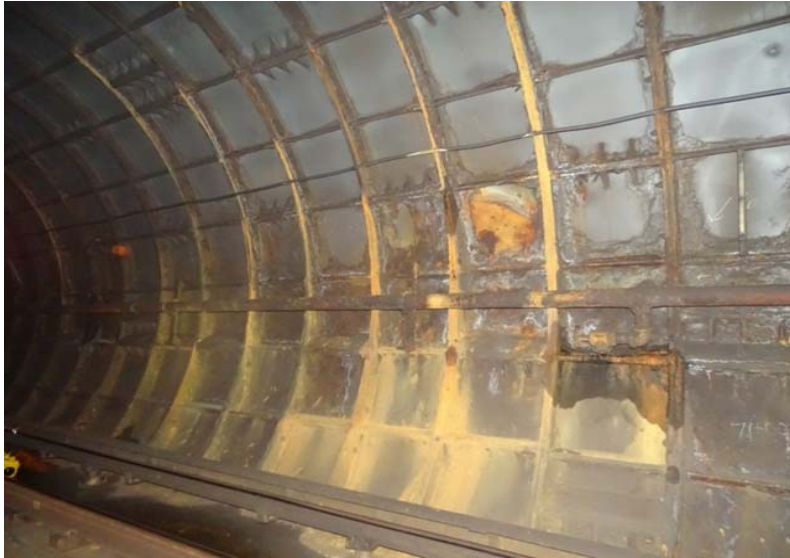
Photograph No. 21 Station 70+00, west wall.
