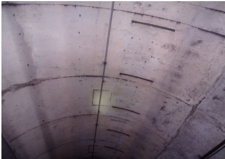
Photograph No. 527 Station 77+60, ceiling.
