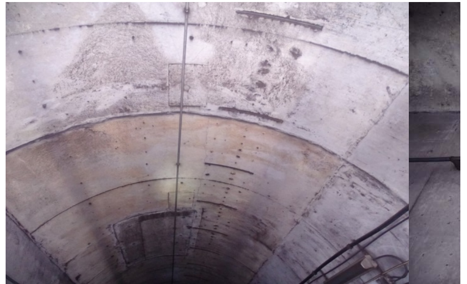
Photograph No. 540 Station 77+80, ceiling.
