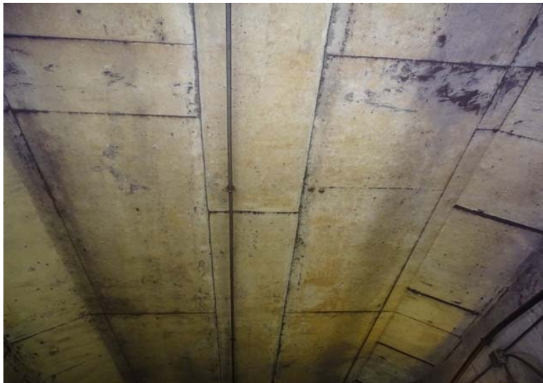
Photograph No. 247 Station 73+50, ceiling.
