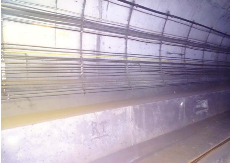
Photograph No. 181 Station 74+40, east wall.
