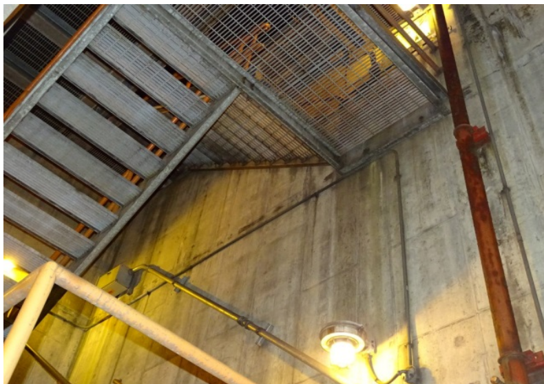
Photograph No. 161 Upper fan room, west wall, south section, upper portion.
