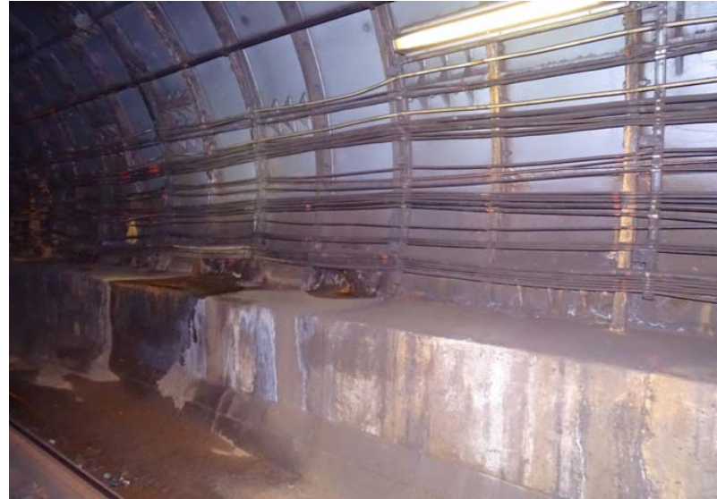
Photograph No. 18 Station 70+00, west wall.
