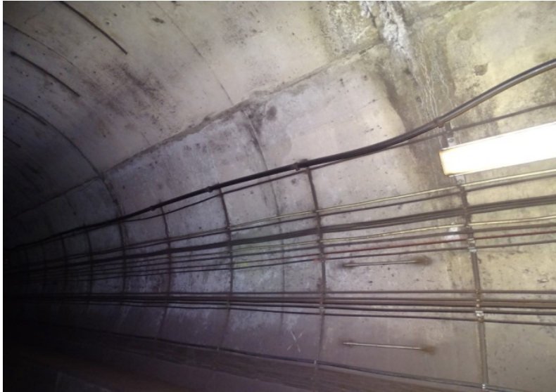
Photograph No. 505 Station 77+20, upper portion of west wall.
