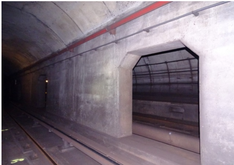
Photograph No. 267 Station 76+40, west wall.
