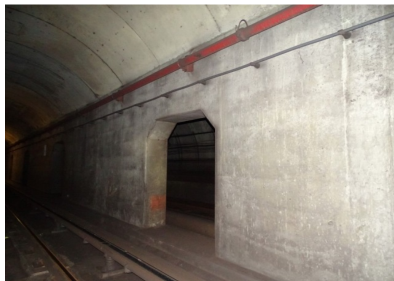
Photograph No. 324 Station 77+60, west wall.
