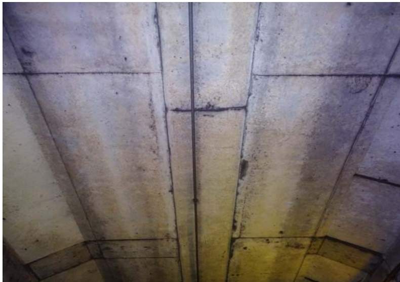
Photograph No. 271 Station 73+90, ceiling.
