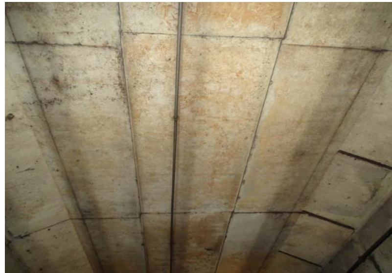
Photograph No. 80 Station 71+10, ceiling.
