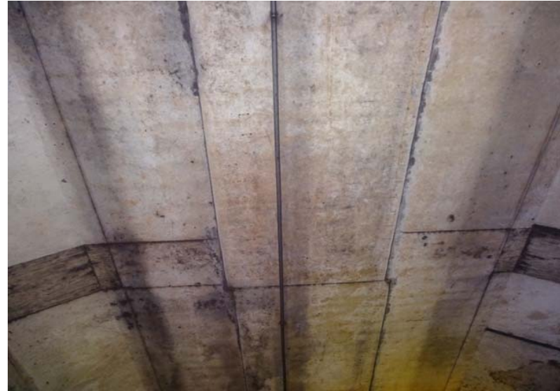
Photograph No. 110 Station 71+50, ceiling.
