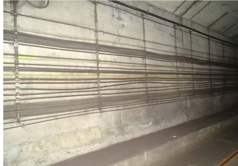
Photograph No. 150 Station 73+60, east wall.
