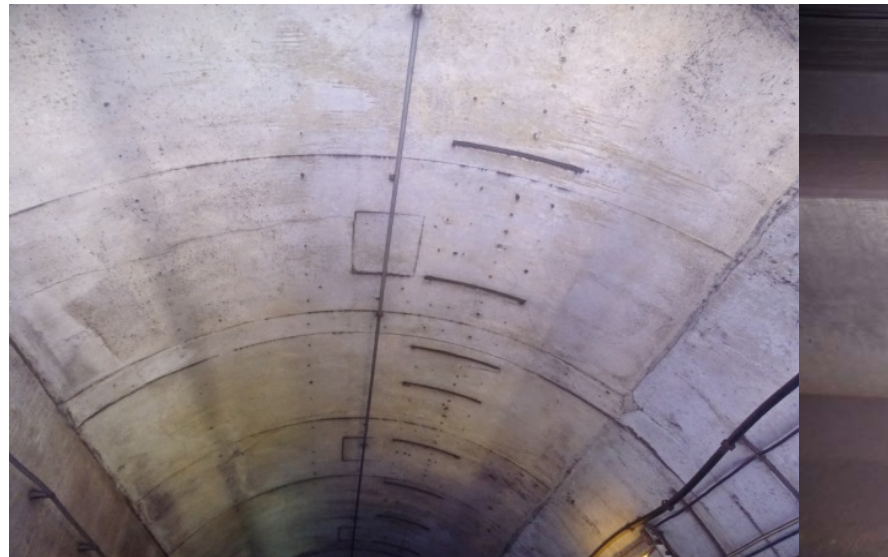
Photograph No. 414 Station 75+90, ceiling.
