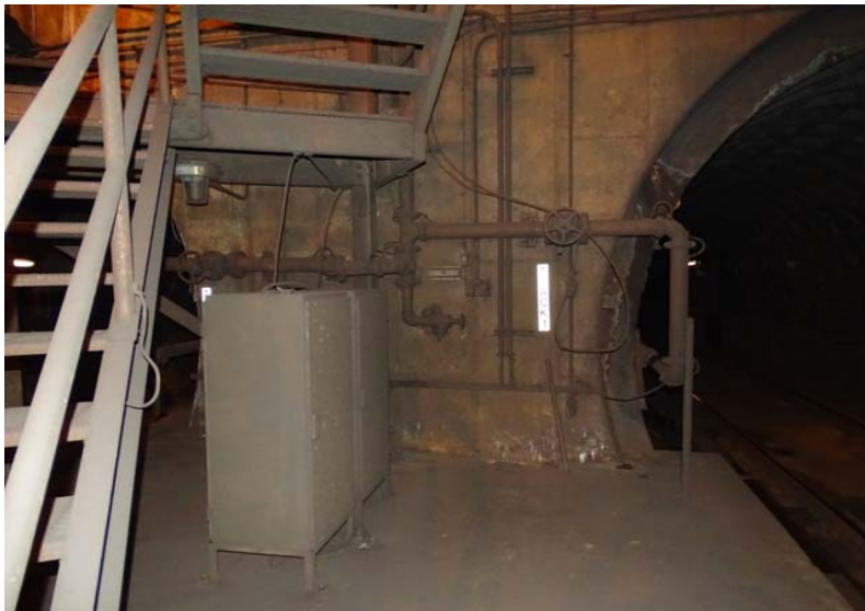
Photograph No. 55 Platform, north wall, east portion.
