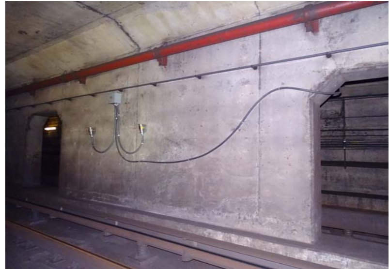
Photograph No. 116 Station 72+60, west wall.
