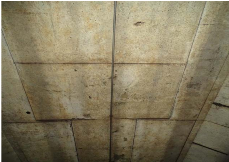
Photograph No. 151 Station 72+10, ceiling.
