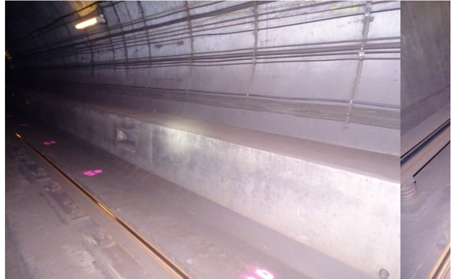
Photograph No. 382 Station 75+40, lower portion of west wall.
