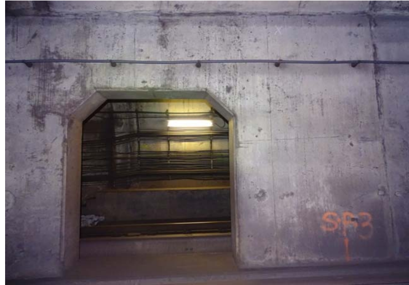
Photograph No. 302 Station 74+40, east wall.
