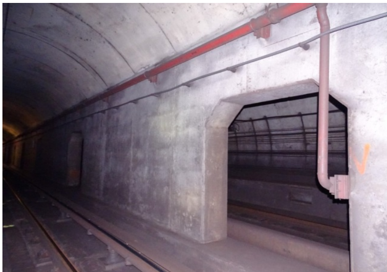
Photograph No. 317 Station 77+40, west wall.
