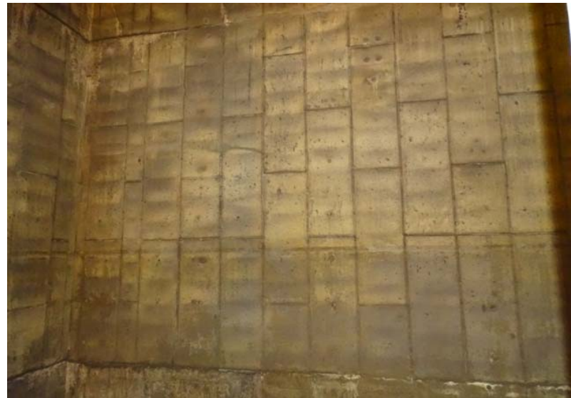
Photograph No. 64 Main room, east wall, middle north portion.
