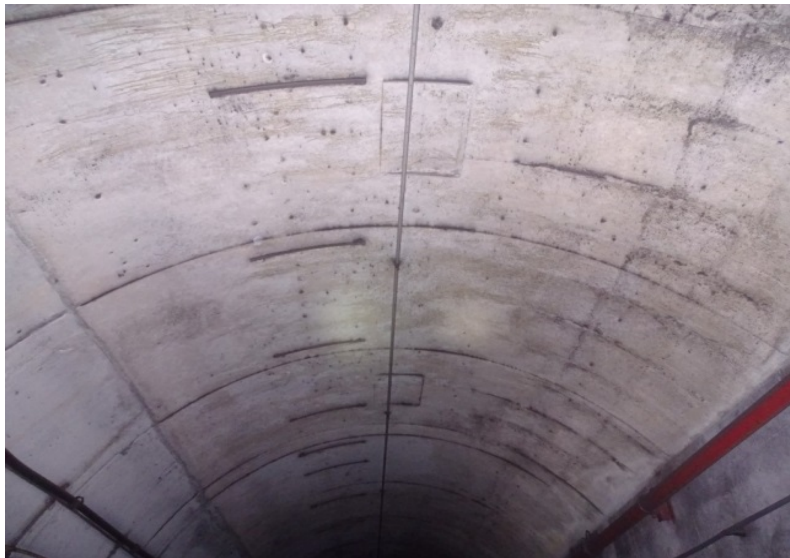
Photograph No. 239 Station 75+80, ceiling.
