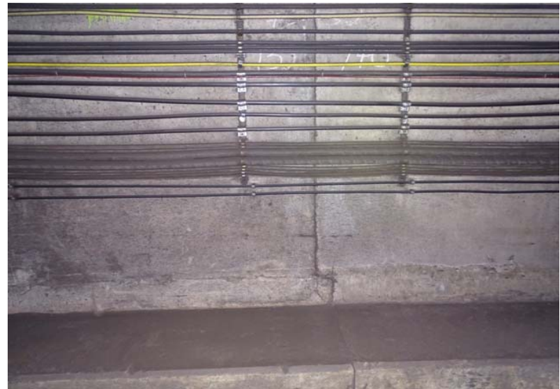
Photograph No. 156 Station 73+60 - construction joint on the east wall.
