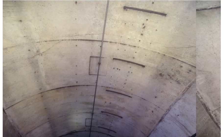
Photograph No. 422 Station 76+00, ceiling.
