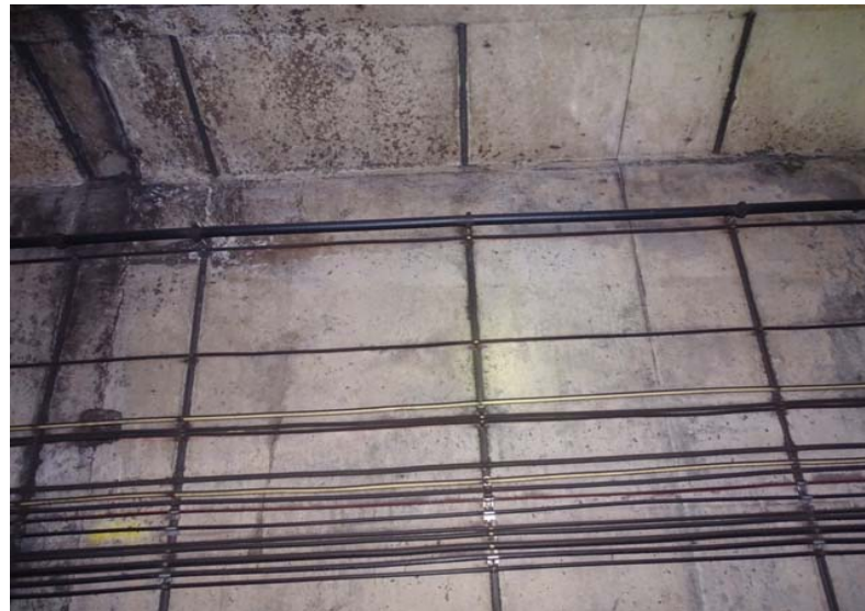
Photograph No. 122 Station 71+70, upper portion of west wall.
