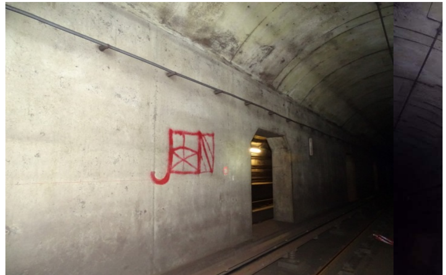
Photograph No. 564 Station 78+50, east wall.
