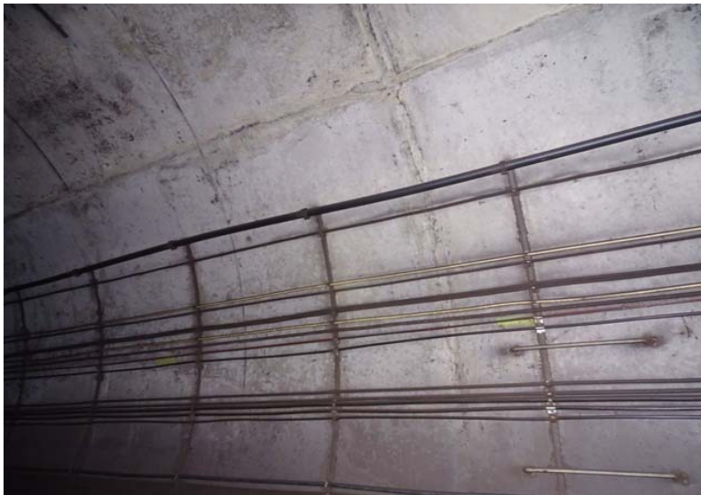
Photograph No. 343 Station 74+90, upper portion of west wall.
