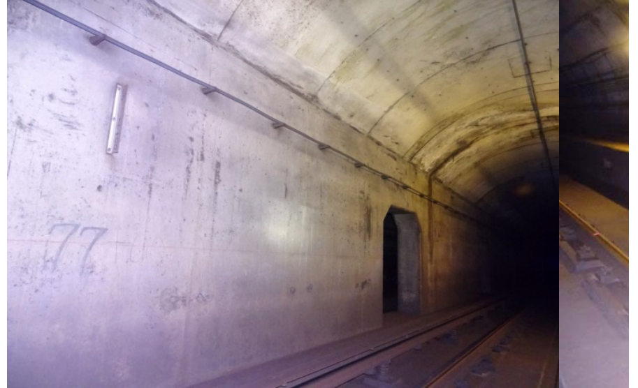
Photograph No. 490 Station 77+00, east wall.
