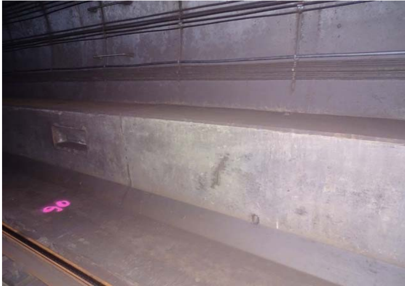
Photograph No. 337 Station 74+80, lower portion of west wall.
