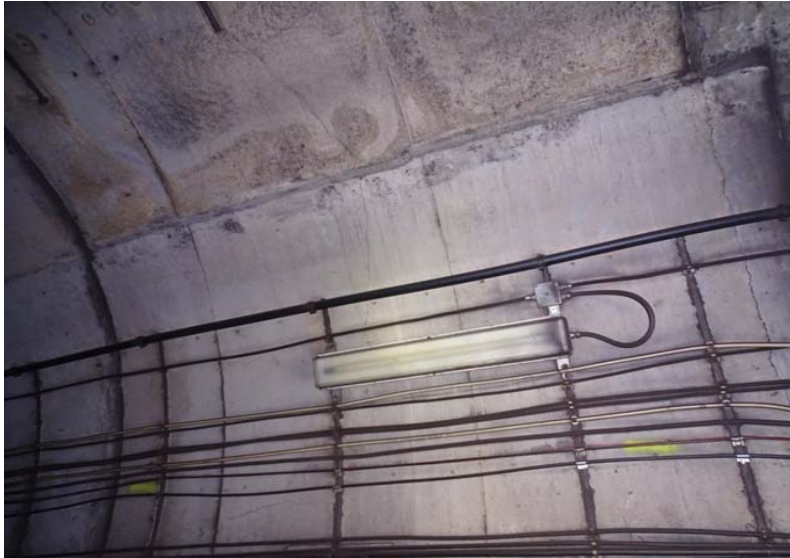
Photograph No. 305 Station 74+40, upper portion of west wall.
