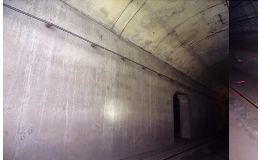
Photograph No. 386 Station 75+50, east wall.
