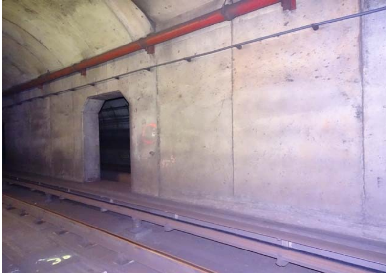
Photograph No. 177 Station 74+20, west wall.
