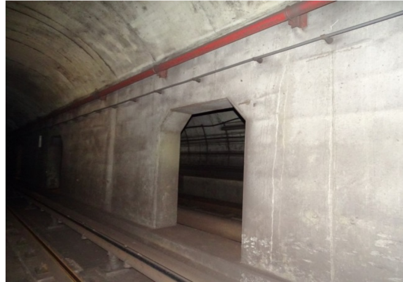
Photograph No. 278 Station 76+60, west wall.
