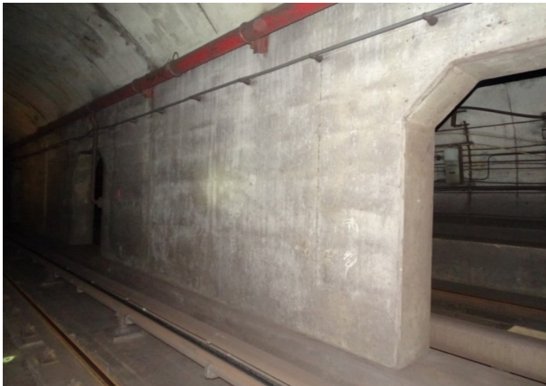
Photograph No. 215 Station 75+20, west wall.
