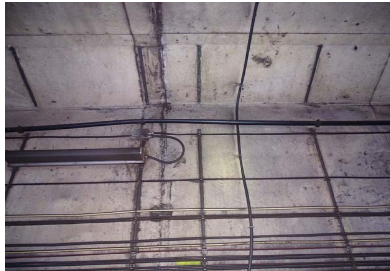
Photograph No. 200 Station 72+80, upper portion of west wall.
