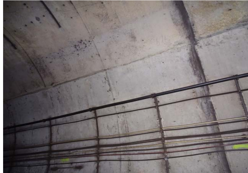
Photograph No. 314 Station 74+50, upper portion of west wall.
