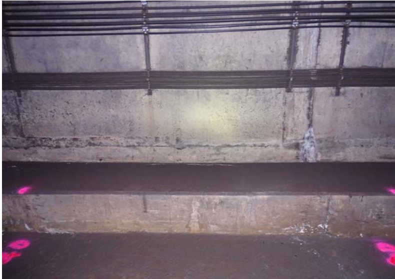
Photograph No. 169 Station 72+30, lower portion of west wall.
