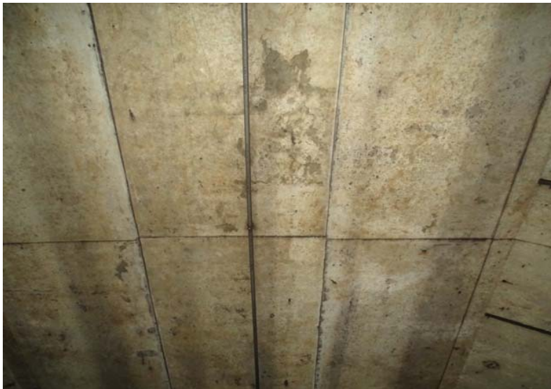
Photograph No. 159 Station 72+20, ceiling.
