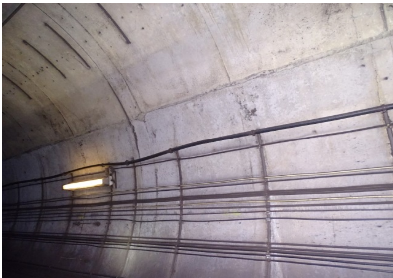
Photograph No. 415 Station 75+90, upper portion of west wall.
