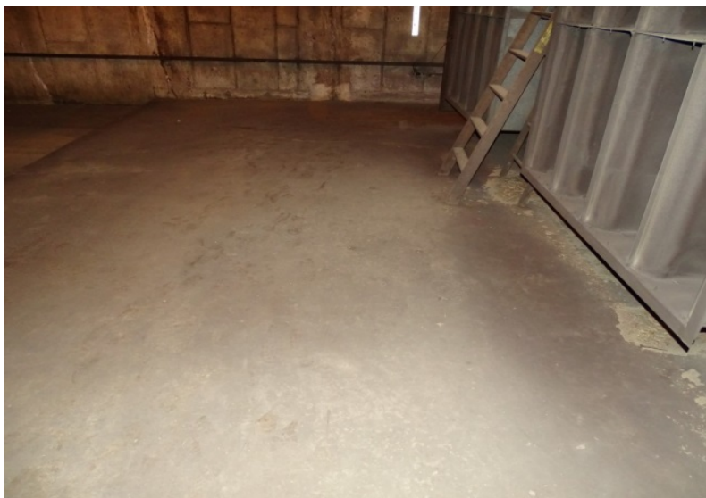
Photograph No. 175 Upper fan room floor, north section, east end.
