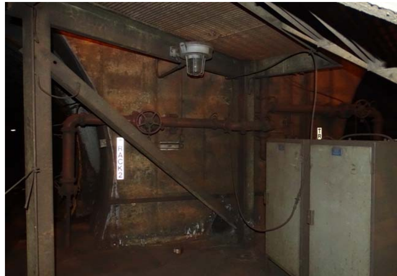
Photograph No. 52 Platform, north wall.
