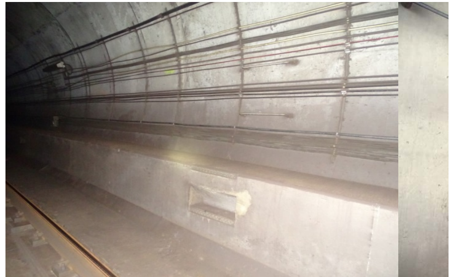
Photograph No. 536 Station 77+70, lower portion of west wall.
