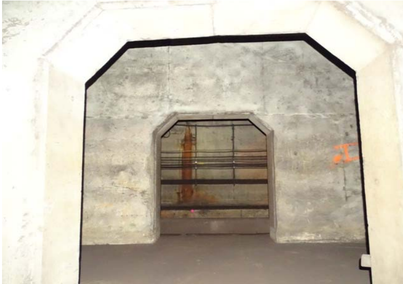
Photograph No. 5 Storage area, section 1, middle portion.
