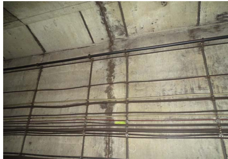
Photograph No. 260 Station 73+70, upper portion of west wall.
