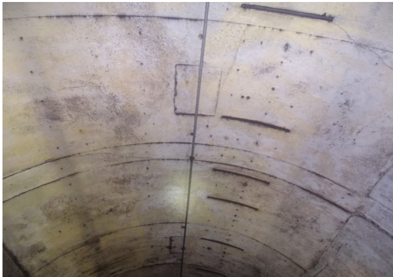
Photograph No. 387 Station 75+50, ceiling.
