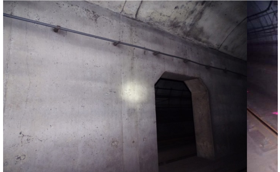
Photograph No. 358 Station 75+10, east wall.
