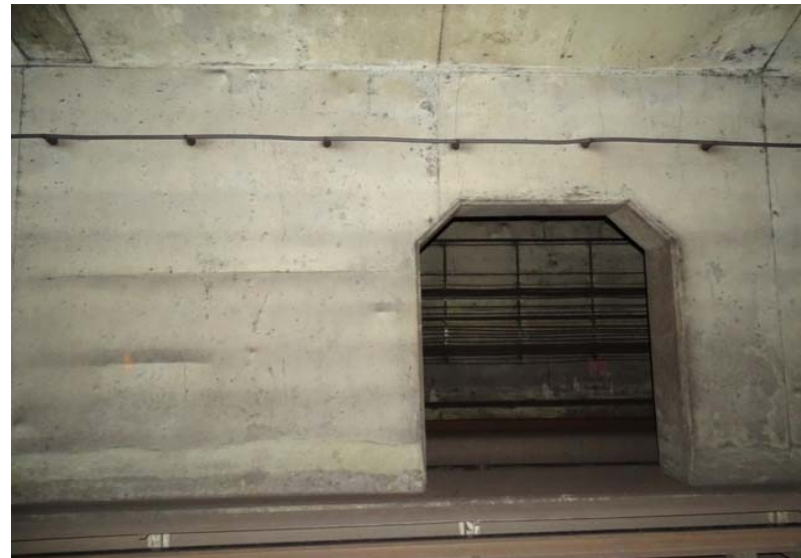
Photograph No. 148 Station 72+10, east wall.
