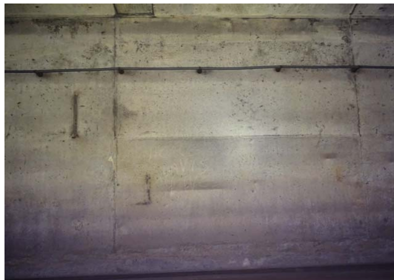
Photograph No. 276 Station 74+00, east wall.
