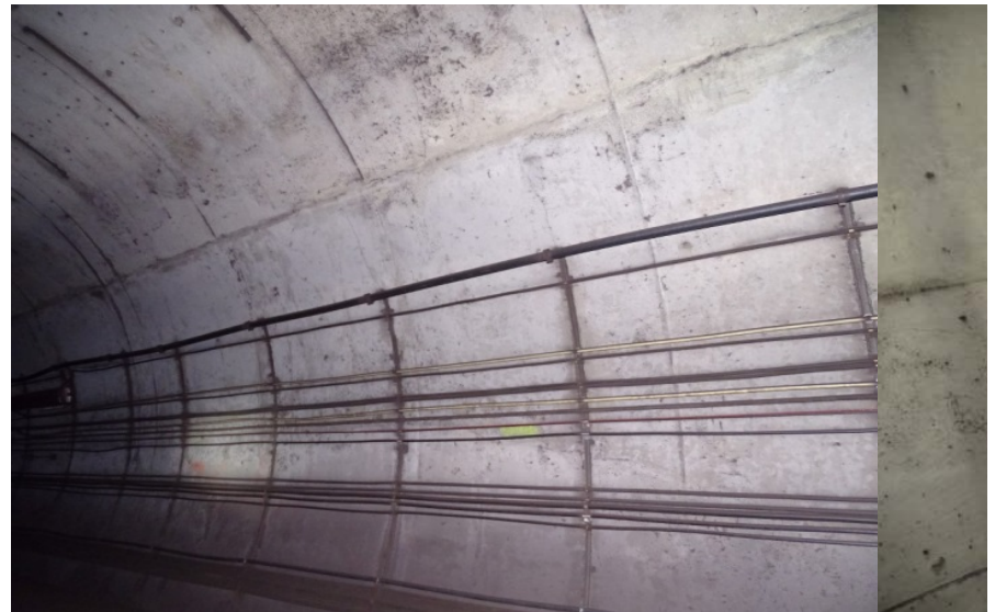
Photograph No. 352 Station 75+00, upper portion of west wall.
