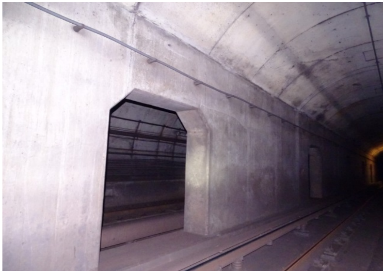
Photograph No. 431 Station 76+10, east wall.
