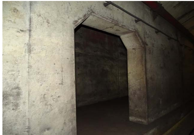
Photograph No. 12 Storage area, section 2, looking north toward arch 2.
