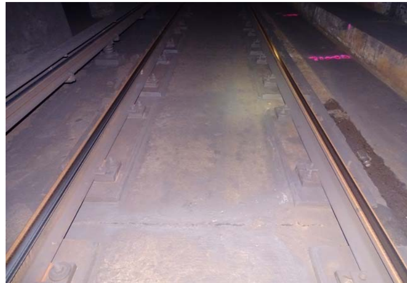
Photograph No. 92 Station 71+30, track bed.
