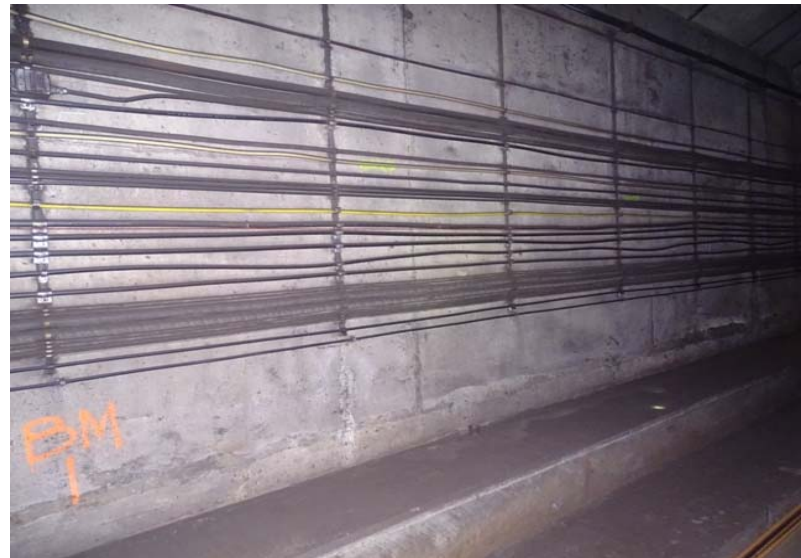
Photograph No. 168 Station 74+00, east wall.
