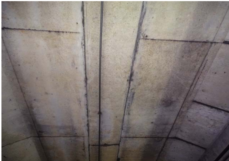
Photograph No. 265 Station 73+80, ceiling.
