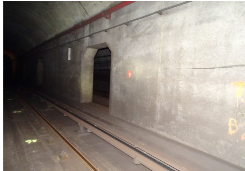
Photograph No. 240 Station 75+80, west wall.
