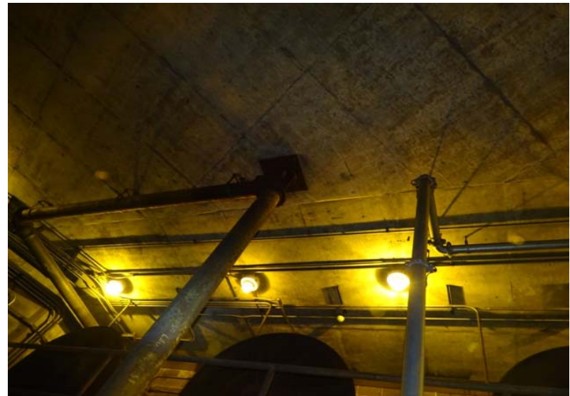
Photograph No. 108 Main room, ceiling, section 4, southwest corner.
