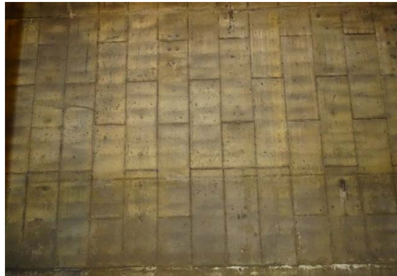
Photograph No. 68 Main room, east wall, upper north portion.
