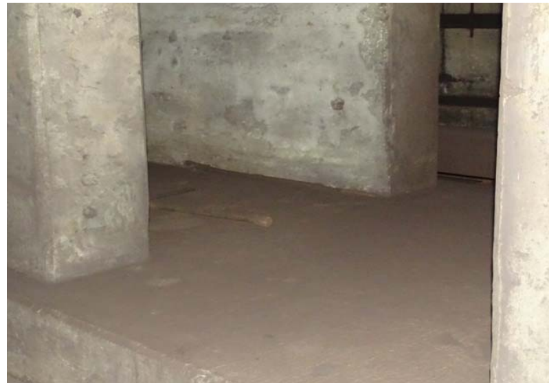
Photograph No. 32 Storage area, section 3, looking south at the floor.
