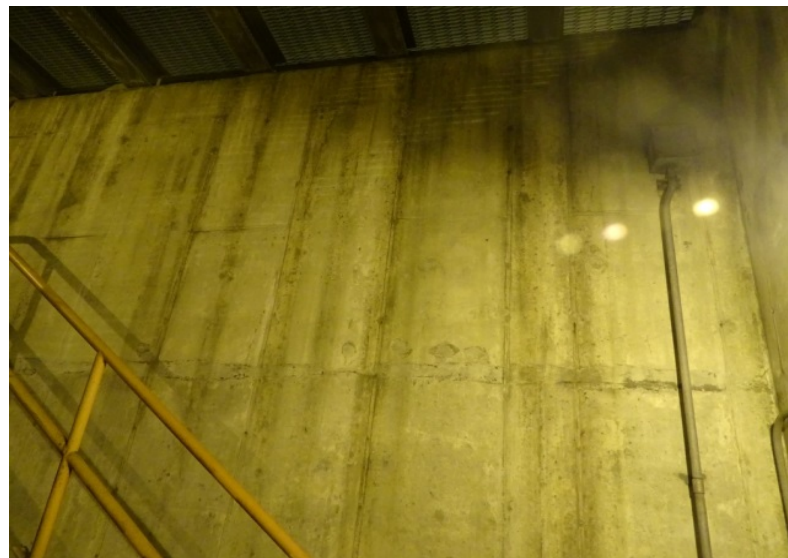
Photograph No. 150 Upper fan room, east wall, south end, upper portion.
