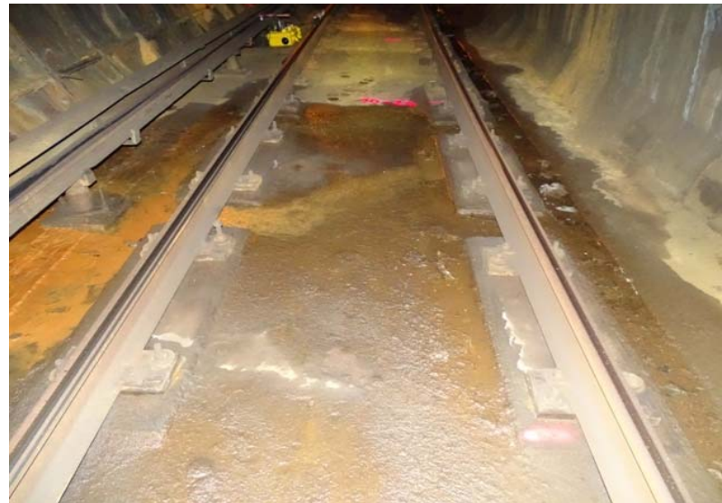
Photograph No. 20 Station 70+10, track bed.
