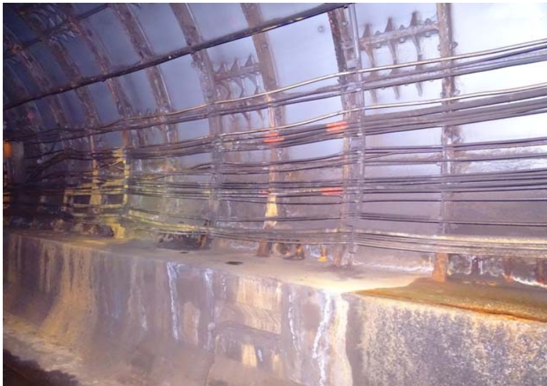
Photograph No. 23 Station 70+10, west wall.
