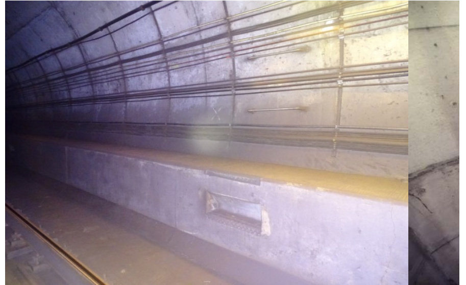
Photograph No. 506 Station 77+20, lower portion of west wall.
