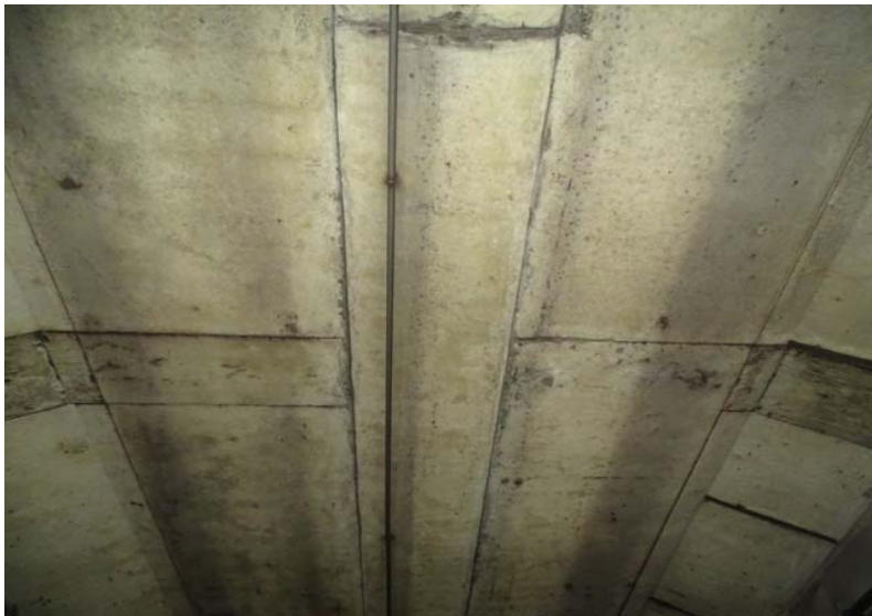
Photograph No. 211 Station 73+00, ceiling.
