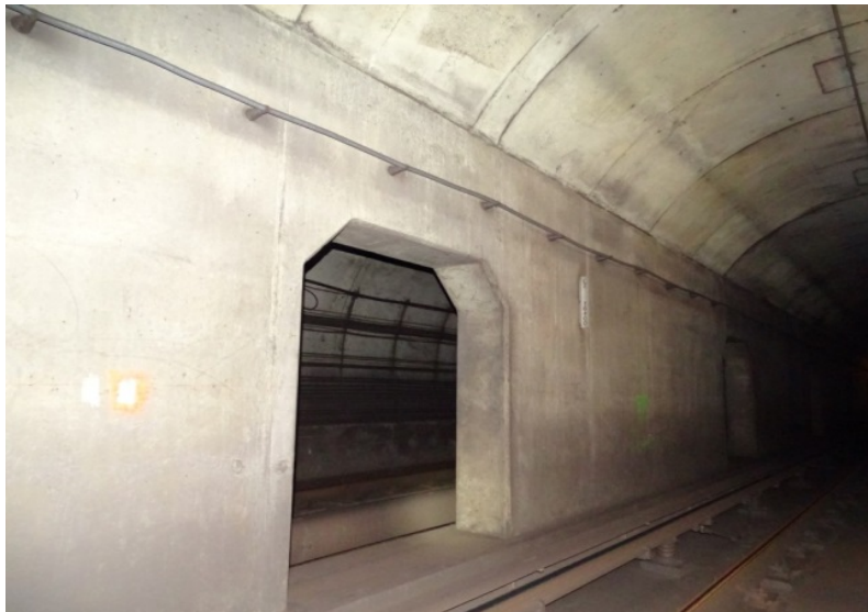
Photograph No. 413 Station 75+90, east wall.
