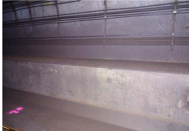
Photograph No. 322 Station 74+60, lower portion of west wall.
