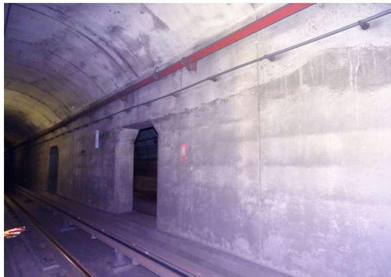
Photograph No. 366 Station 78+80, west wall.
