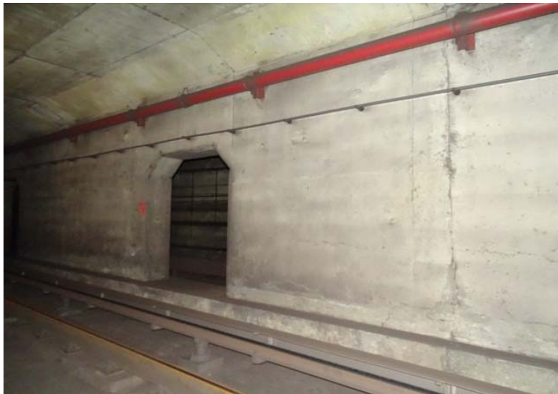
Photograph No. 95 Station 72+20, west wall.
