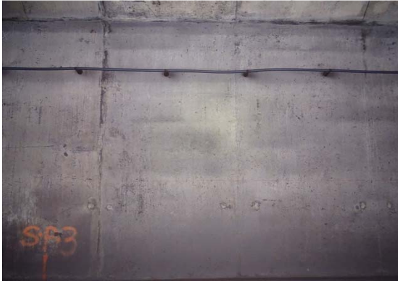
Photograph No. 309 Station 74+50, east wall.
