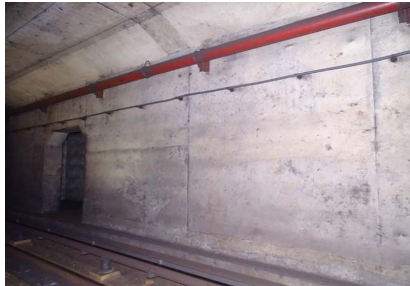
Photograph No. 60 Station 71+40, west wall.
