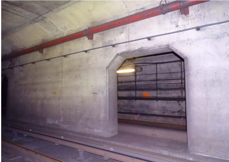
Photograph No. 165 Station 73+80, west wall.
