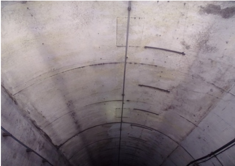
Photograph No. 571 Station 79+00, ceiling.
