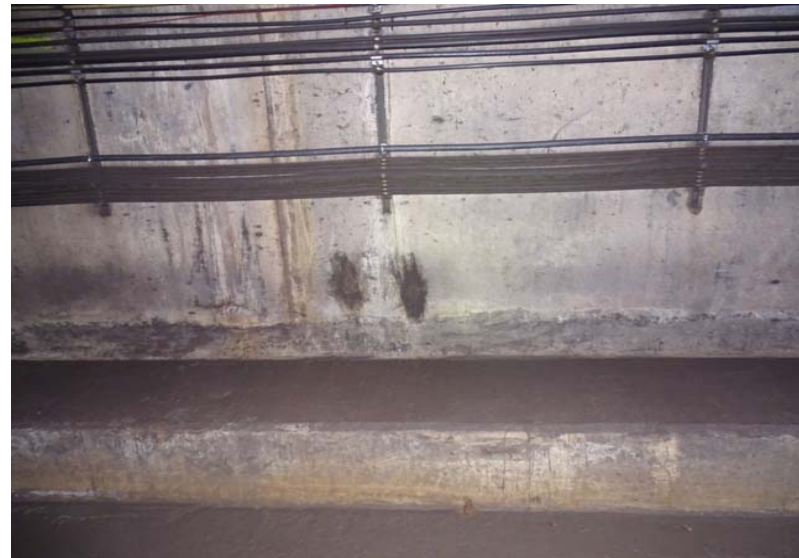
Photograph No. 292 Station 74+20, lower portion of west wall.
