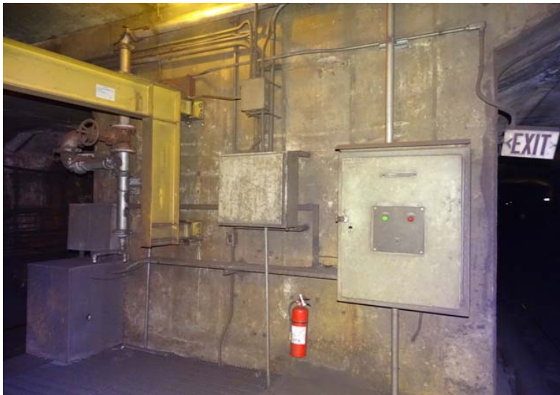
Photograph No. 39 Platform, south wall.
