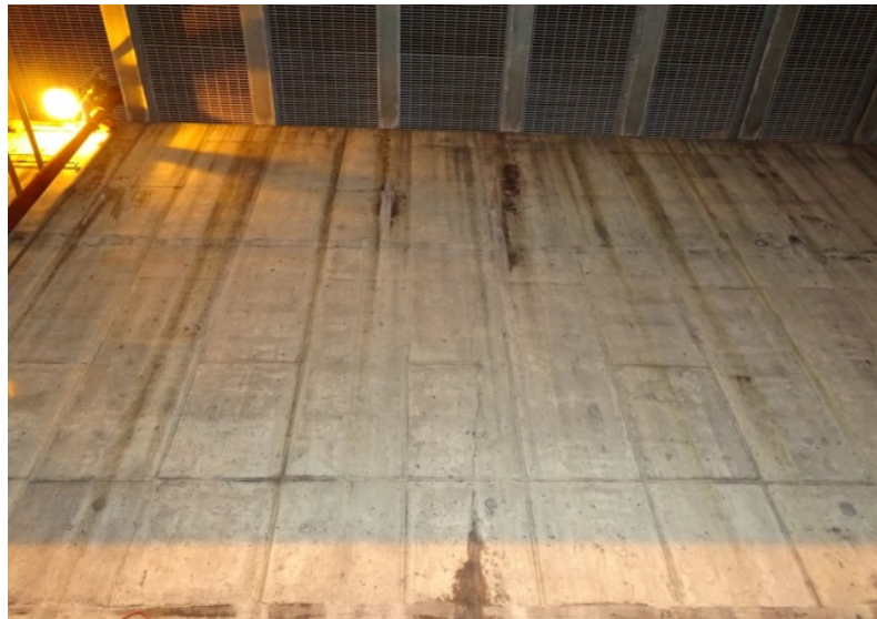
Photograph No. 167 Upper fan room, west wall, middle-south section, upper portion.
