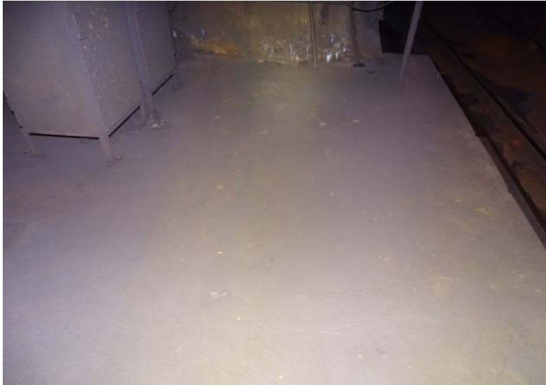
Photograph No. 57 Platform, floor, close up of northeast portion.
