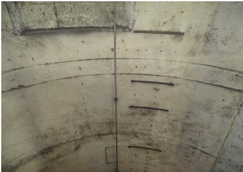
Photograph No. 327 Station 74+70, ceiling.
