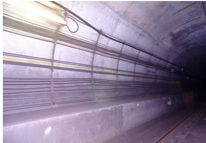
Photograph No. 288 Station 76+80, east wall.
