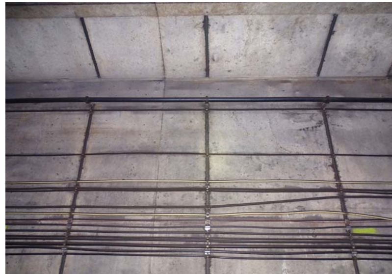
Photograph No. 152 Station 72+10, upper portion of west wall.
