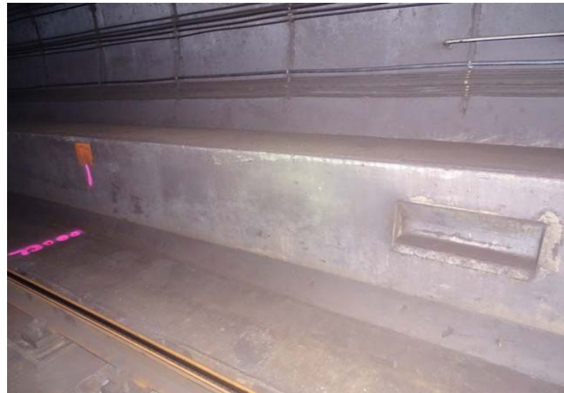
Photograph No. 344 Station 74+90, lower portion of west wall.
