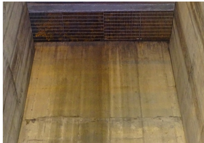
Photograph No. 132 Upper fan room, north wall, upper portion.
