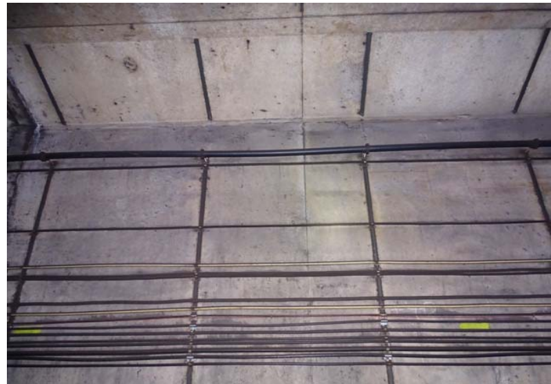
Photograph No. 160 Station 72+20, upper portion of west wall.
