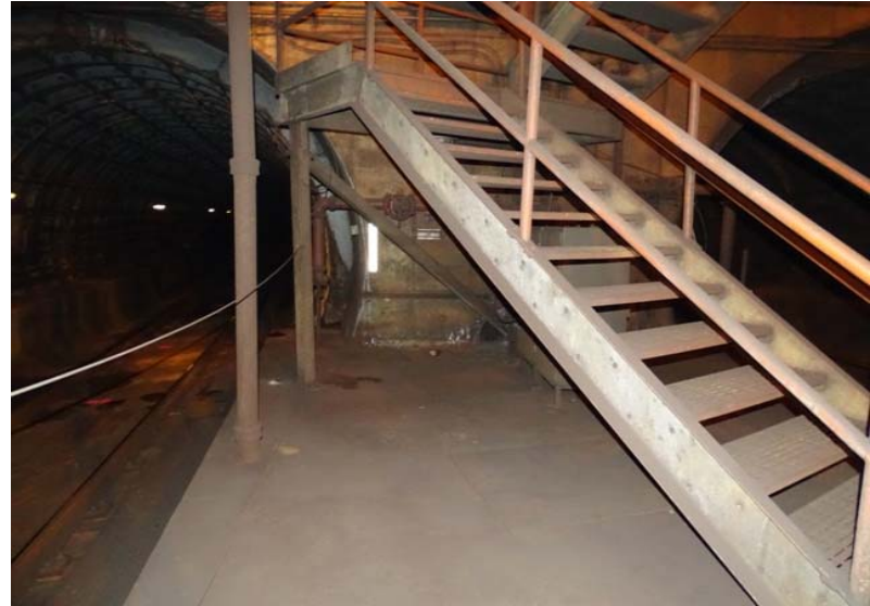
Photograph No. 50 Platform, looking north.
