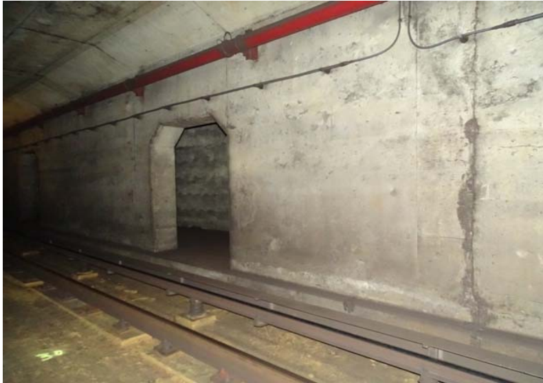
Photograph No. 53 Station 71+20, west wall.
