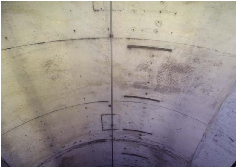
Photograph No. 335 Station 74+80, ceiling.
