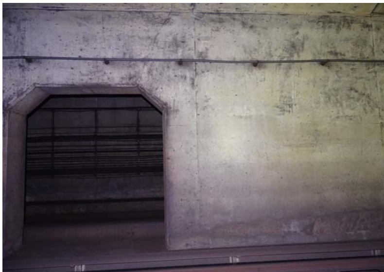
Photograph No. 239 Station 73+40, east wall.
