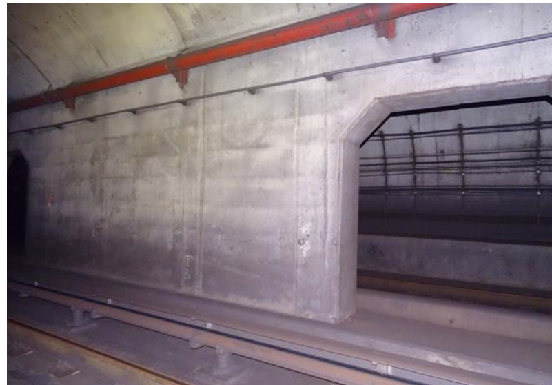
Photograph No. 196 Station 74+60, west wall.
