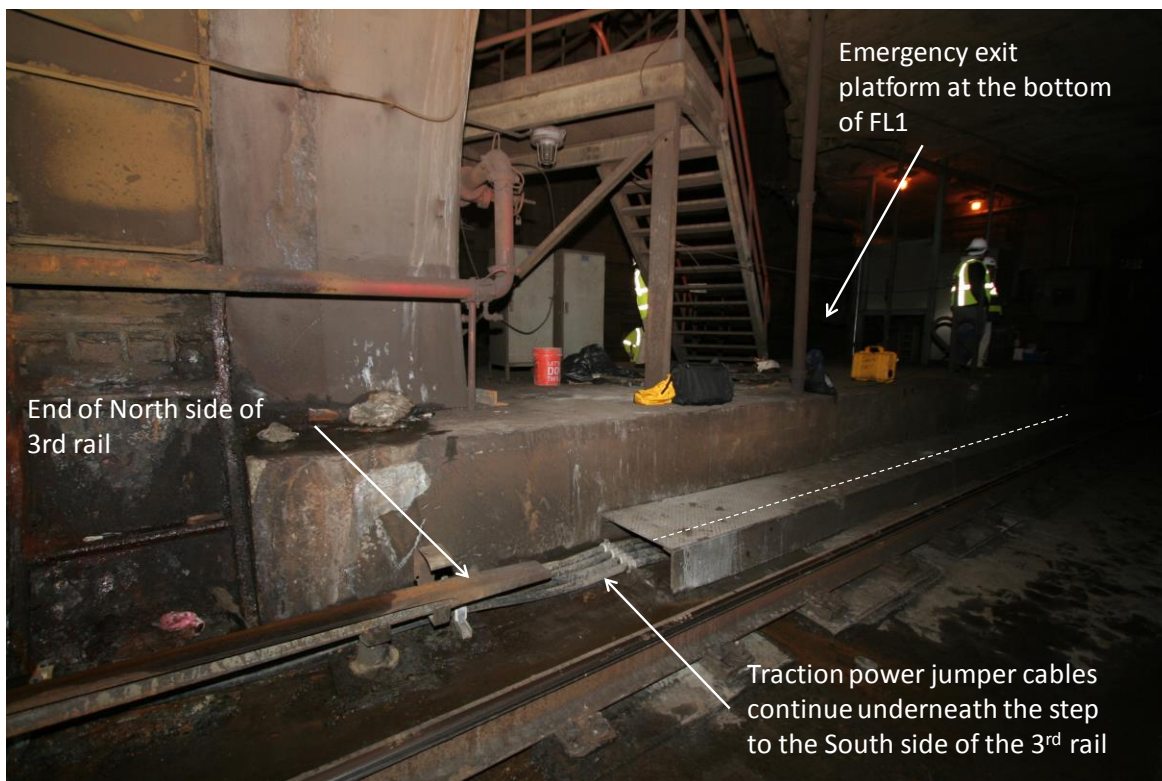
Figure 2: Emergency exit platform at the Intersection of L-line Track #2 and FL1.
