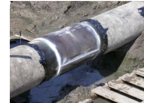
Carry out repairs)
