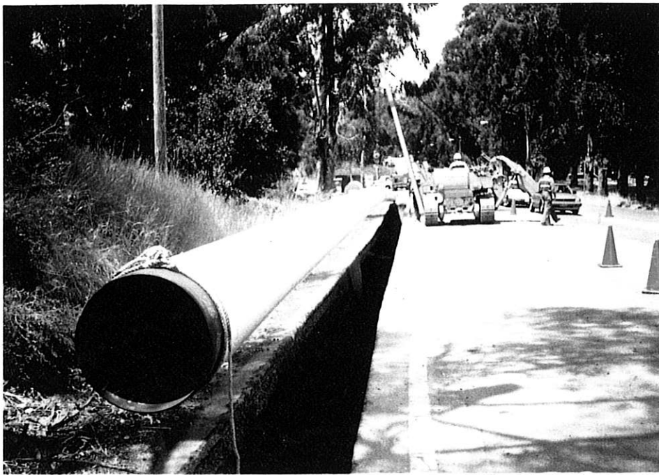
Lowering pipeline into trench
