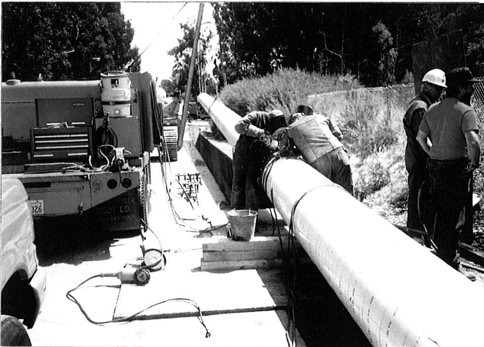
Welding pipeline segments together
