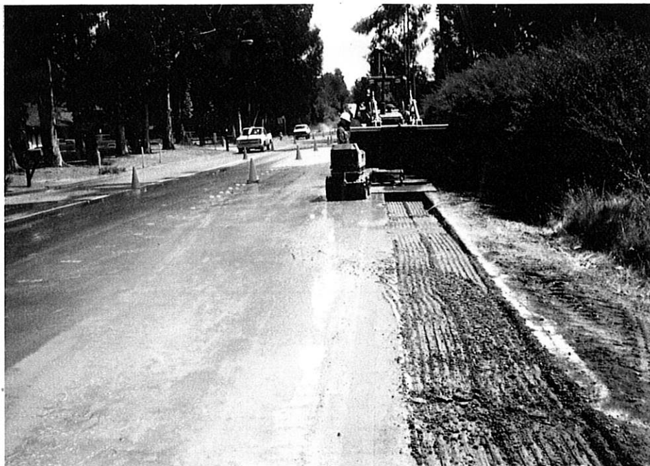
Backfilling and steel-plating trench
