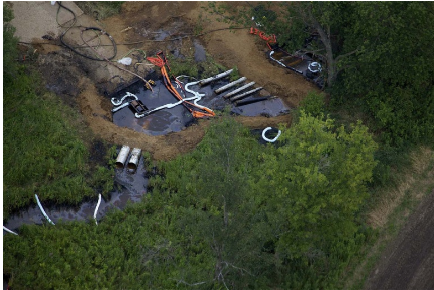
Figure 4: Underflow dam construction on Talmadge Creek, July 30, 2010. State of Michigan Photograph.
