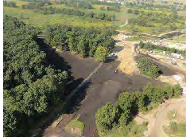
Insert 3-1 Source Area after re-grading with clean organic soils
