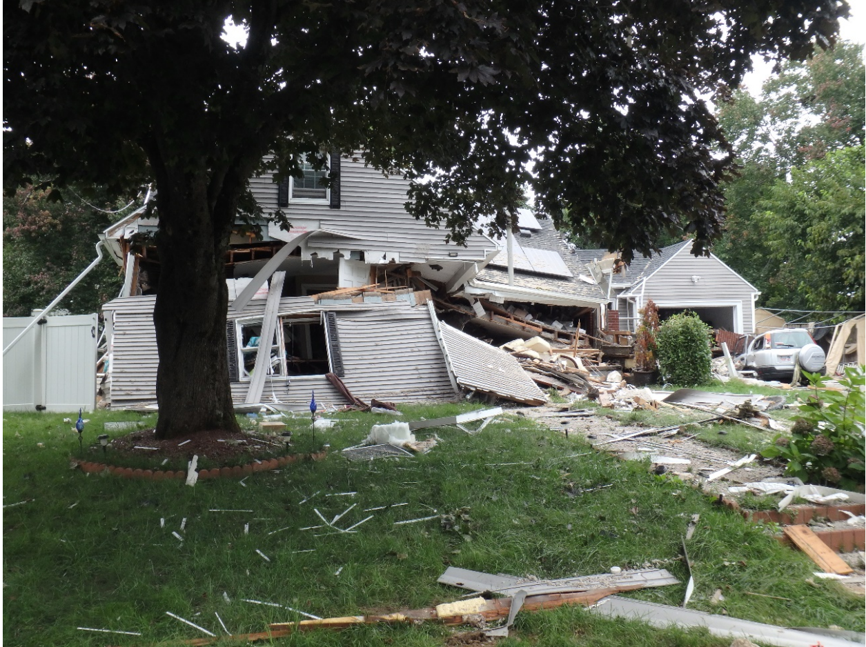
1 2 Figure 2: Exploded House where fatality occurred and two other severe injuries. 3
