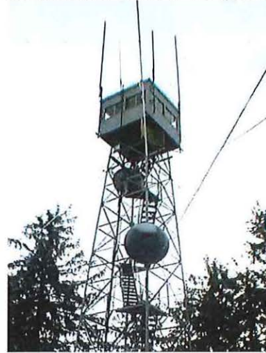
Figure 2-28: Typical Fire Tower
