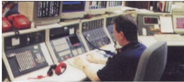
Figure 4-11: Metrofire Control Center
