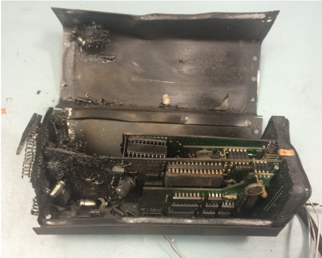
Figure 13. JPI EDM-700 internal inspection.
