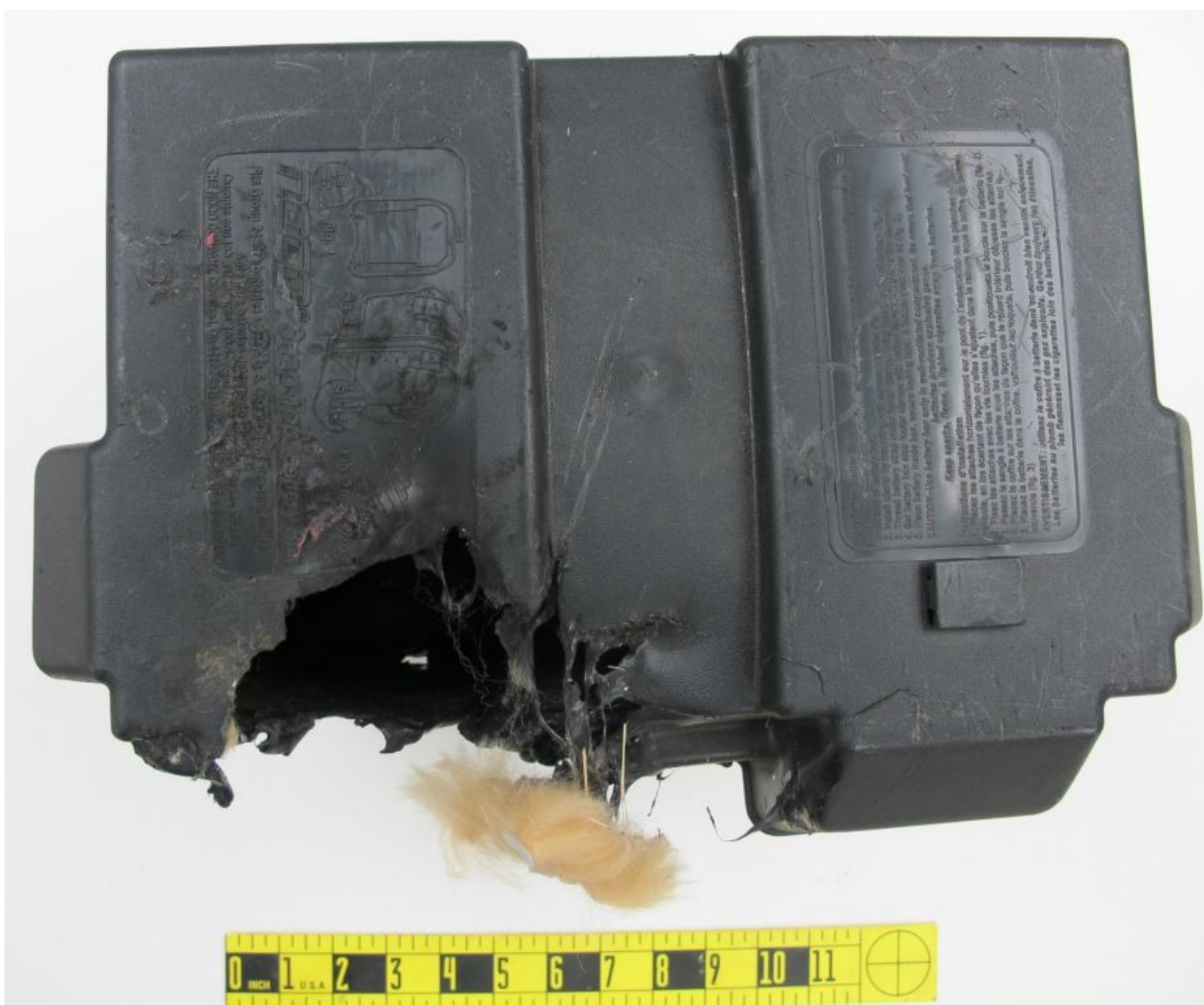
Figure 6 - Top View of Battery Box
