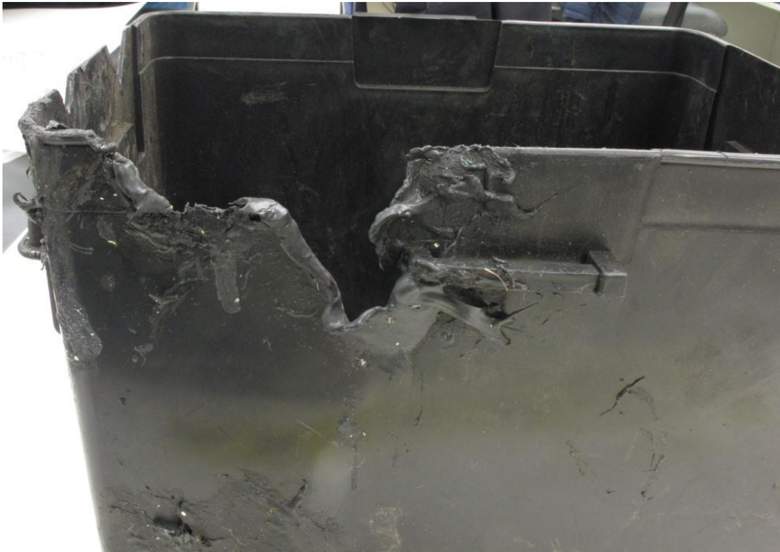
Figure 8 - Closeup of Front Side of Battery Box Melted Area
