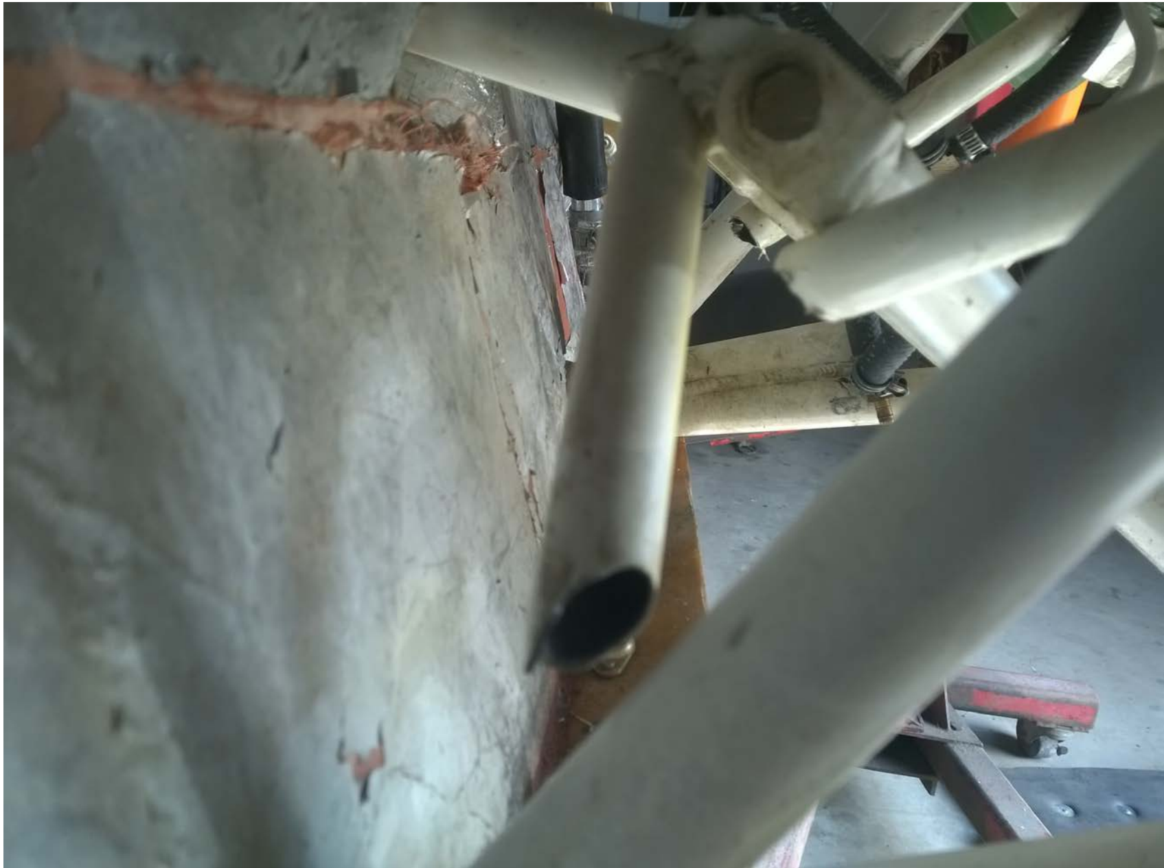
Photo 2 - View of engine mount damage (photo courtesy of the pilot).
