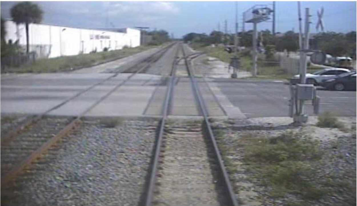
Figure-4 Depicts crossing gates in the up position as ATK 146 approached the crossing.
