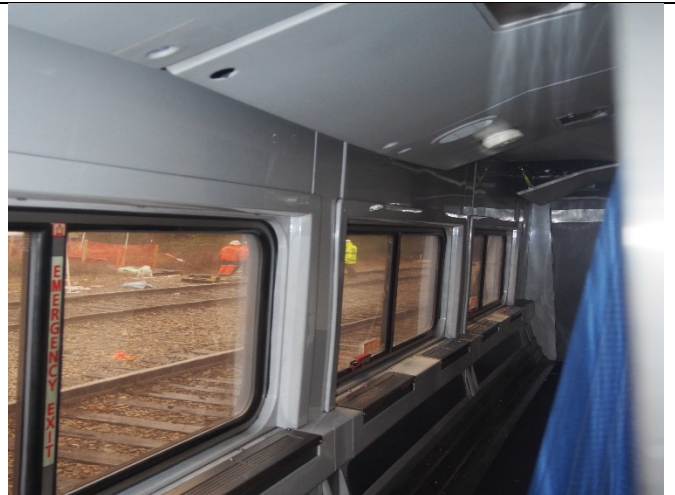
Figure 18- An example of dropped ceiling panels
