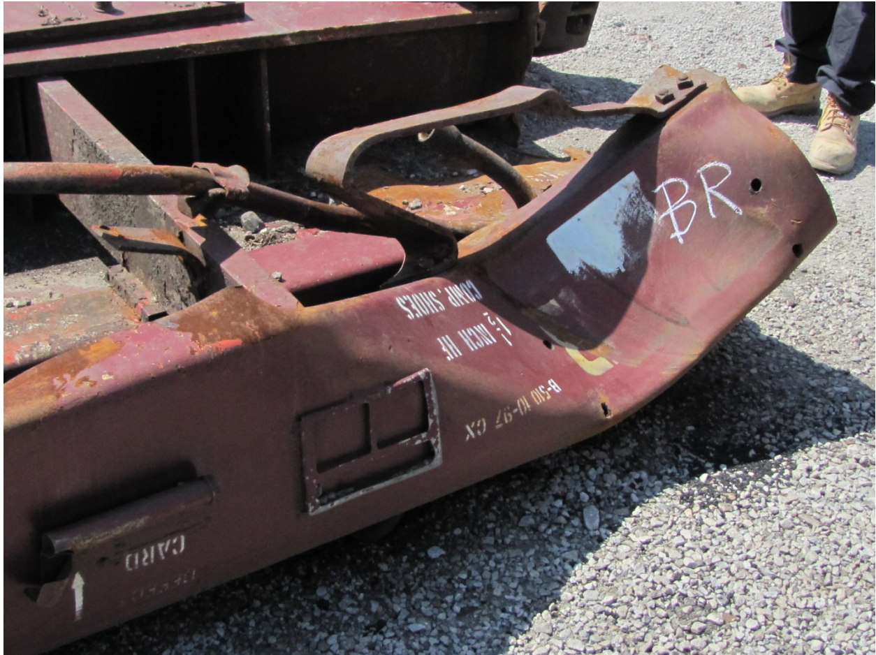
Exhibit 65-Photo Showing Damage to the Side Sill on BNSF 927022
