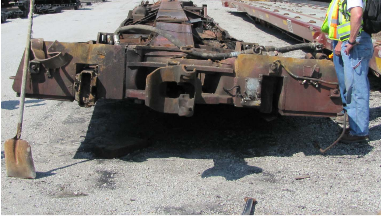
Exhibit 54-Photo Showing A-End Damage to BNSF 927022
