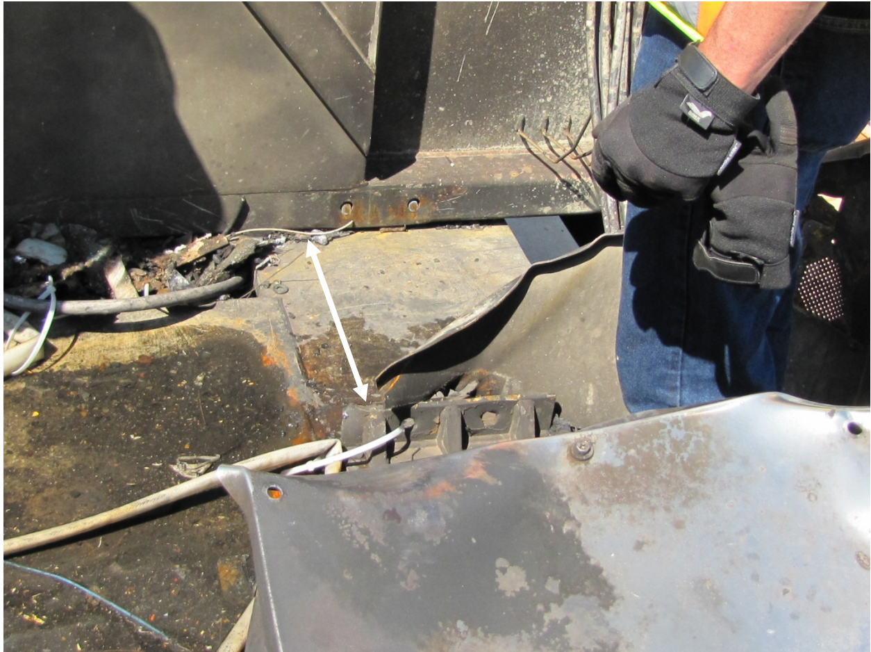
Exhibit 40-A-Photo Showing the Electrical Locker of BNSF 9159 Displaced 25 1/2" from Attachment Point
